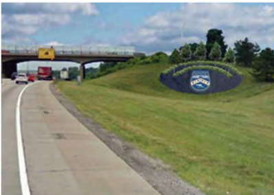
Hillside Signage and Landscaping
