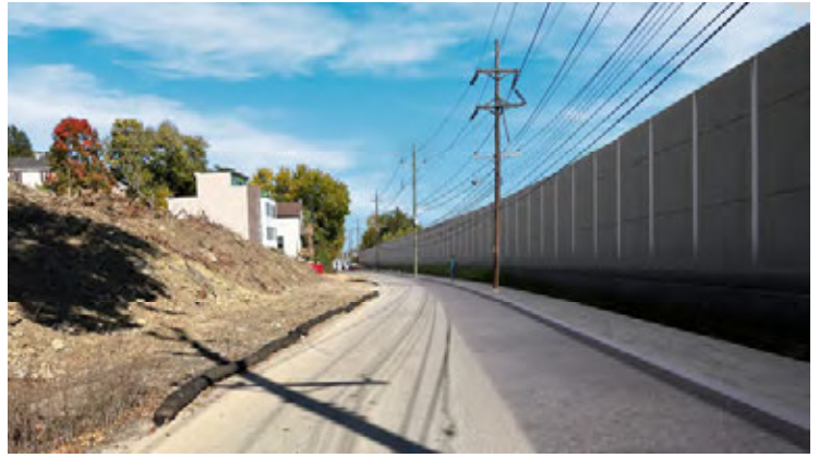
Crescent Avenue With Noise Wall 67 dBA (average)
