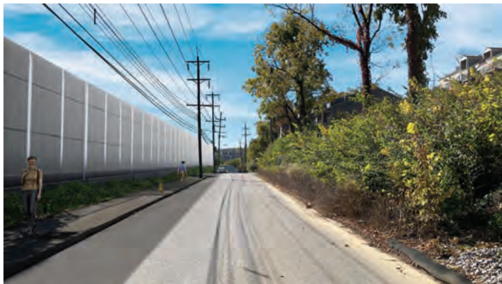
Crescent Avenue With Noise Wall - Kentucky (Looking South)
