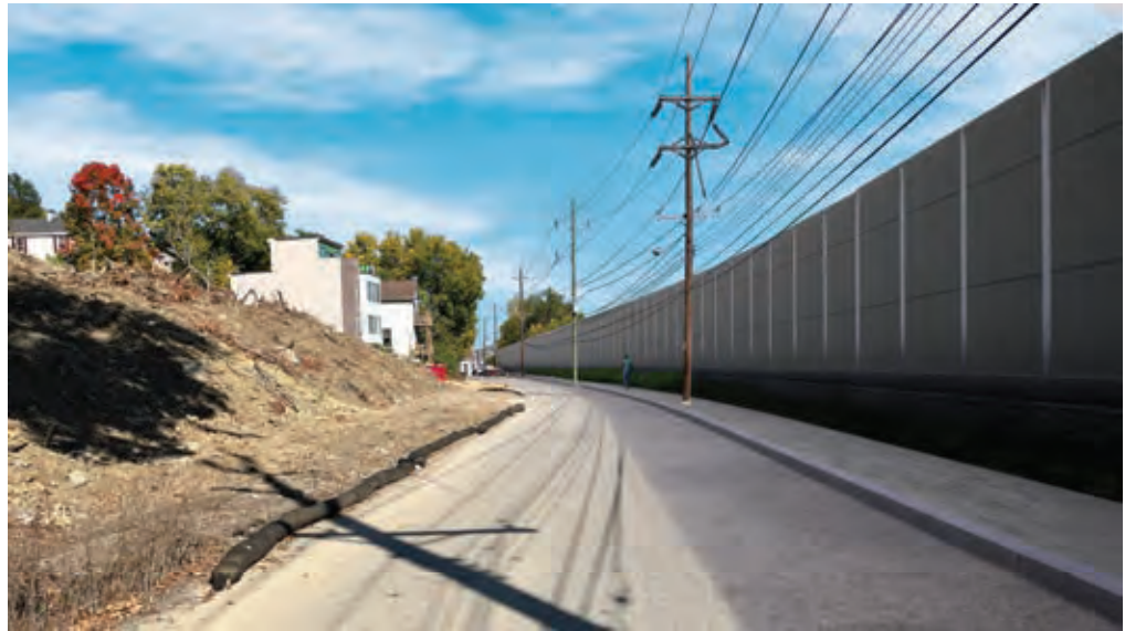
Crescent Avenue With Noise Wall - Kentucky (Looking North)
