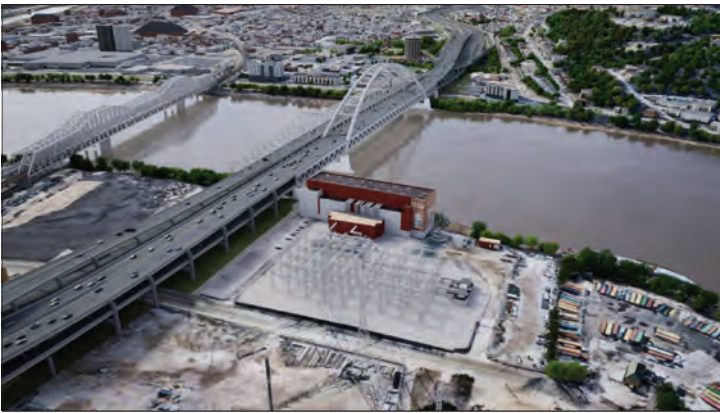
This drawing shows what the new companion bridge and the existing Brent Spence Bridge might look like after the project is built. Please note that the final design of the companion bridge will not be complete for a few years. It is possible it could be a cable-stayed design.
