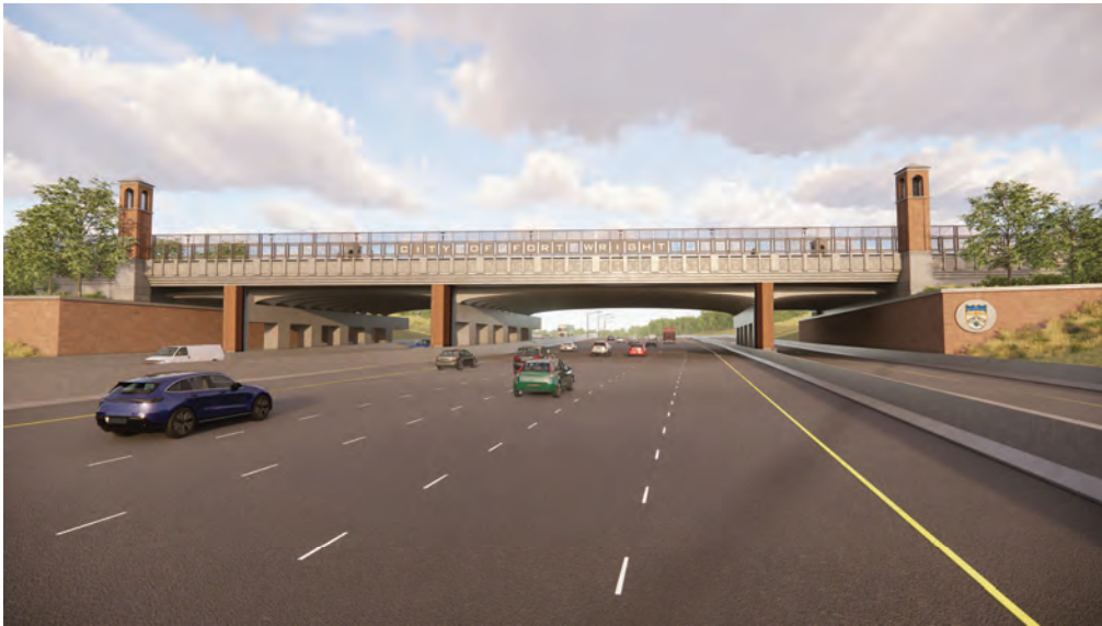
Kyles Lane Overpass (Looking South)
