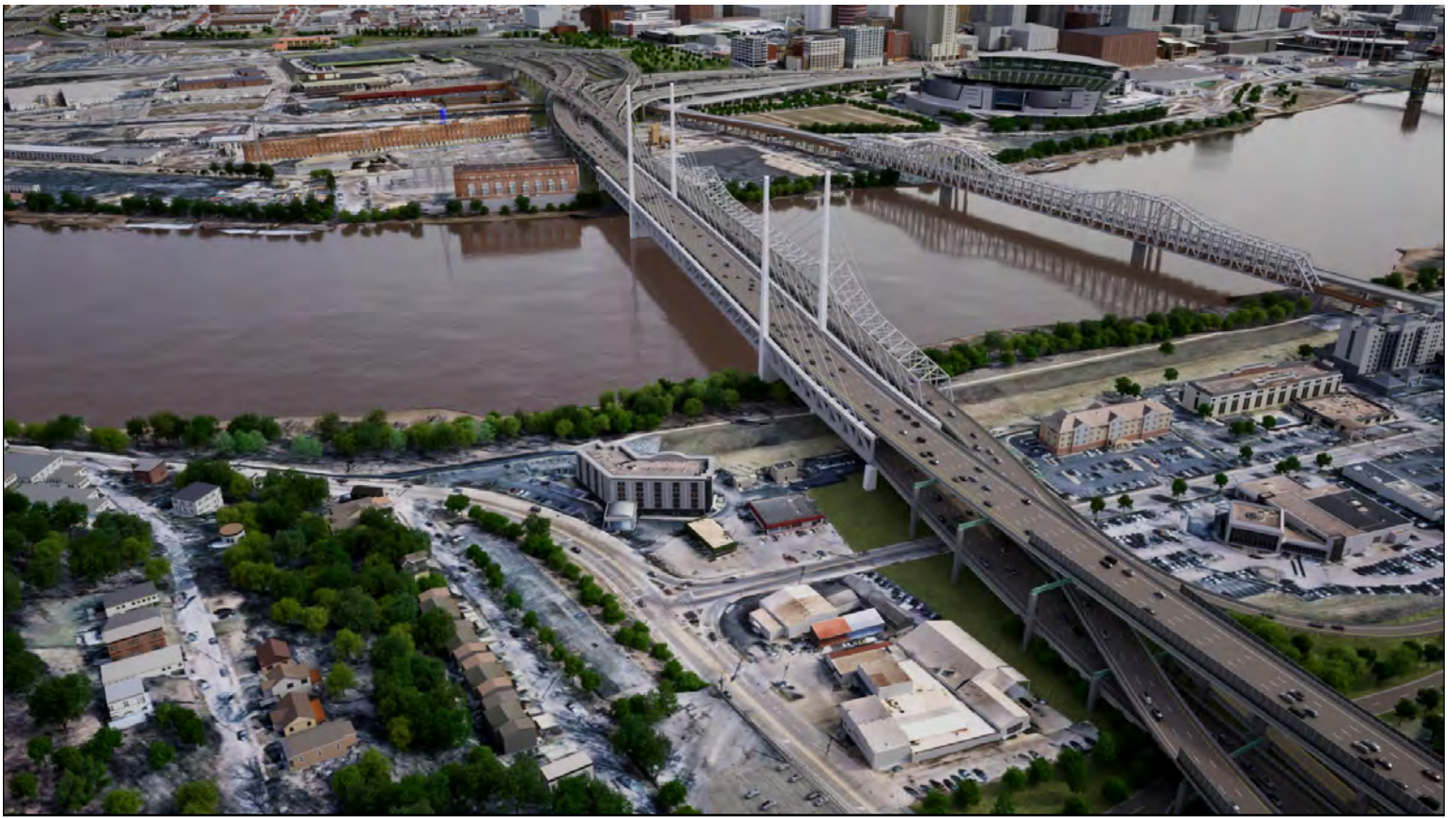
This rendering shows what a cable-stayed bridge might look like if that design is chosen.
