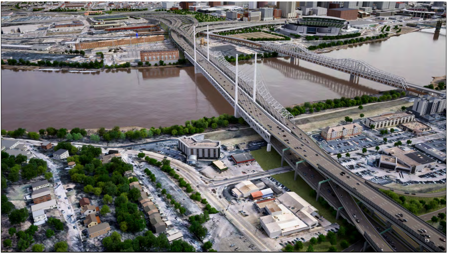
The other is a cable-stayed bridge, and this shows what a standard cable-stayed bridge looks like.
