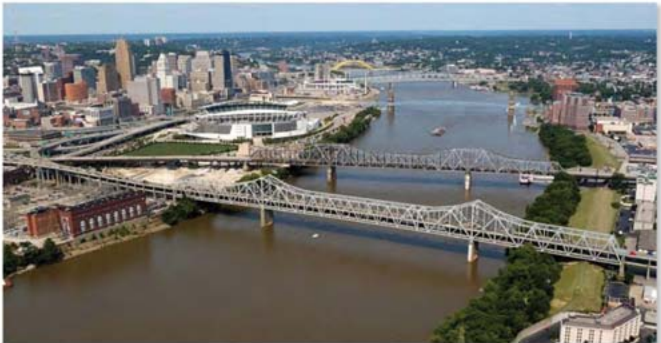
Existing Brent Spence Bridge
