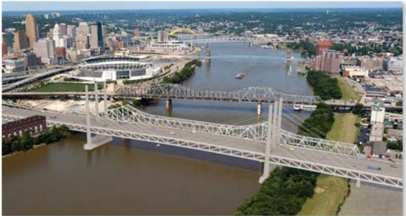
Alternative 3: Two Tower Cable Stayed Bridge
