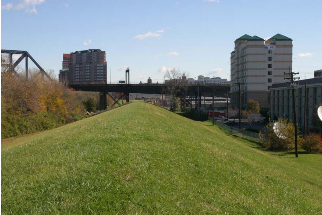
Figure 4. View Looking East from I-71/I-75 Showing Flood Control Levee in Covington, Kentucky
