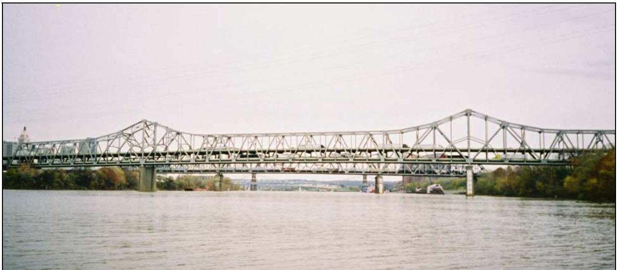
Figure 1. Elevation of main truss spans of Brent Spence Bridge facing upstream
