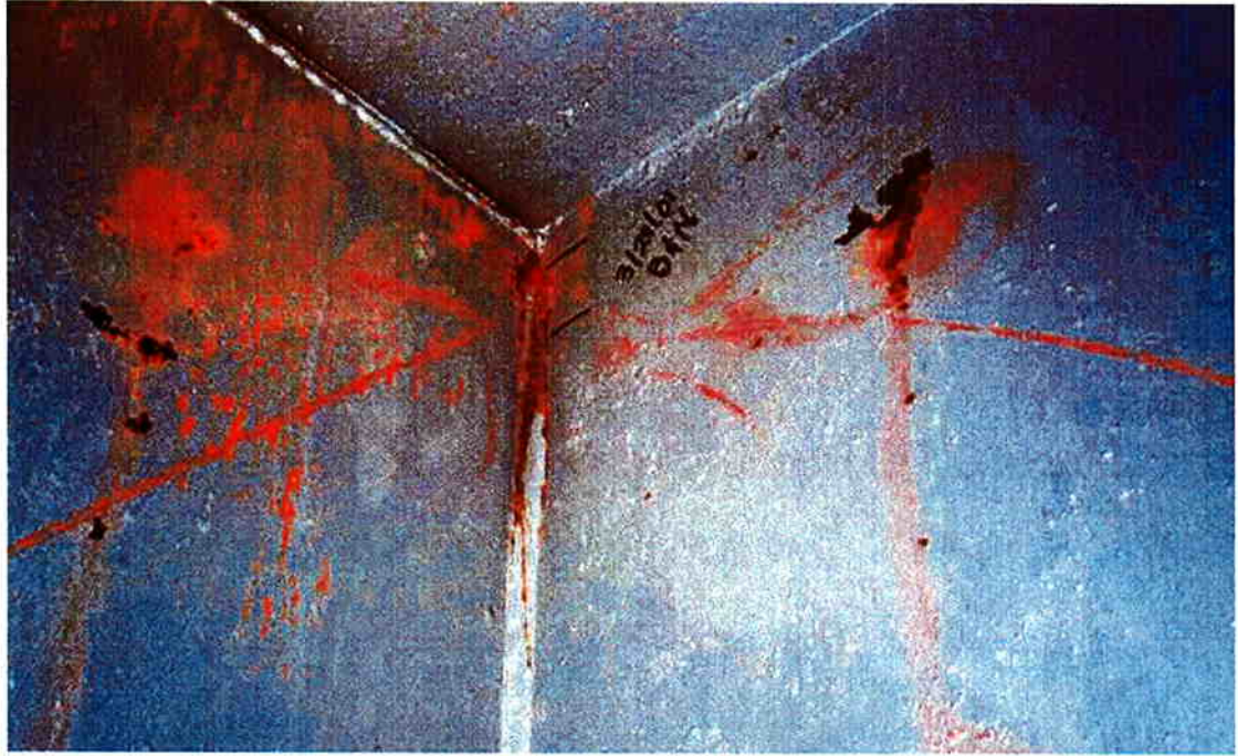
Photo 7: Looking south at the west face of diaphragm 5 and the south web plate in Pier Cap 4. Note 1-5/8 inch crack at top of weld from diaphragm to web plate.
