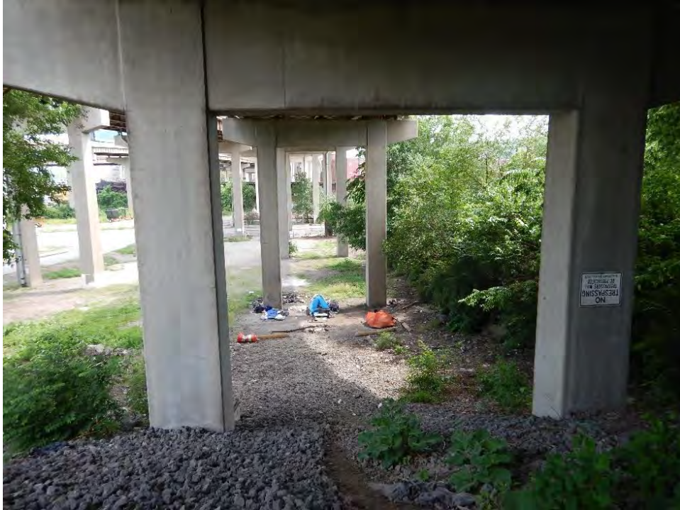
Photograph 22. View of I-75 right-of-way, looking south.
