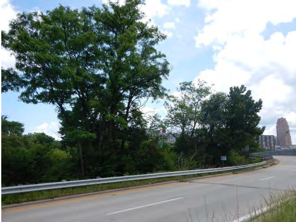
Photograph 66. View of I-75 right-of-way with SWH, looking east.
