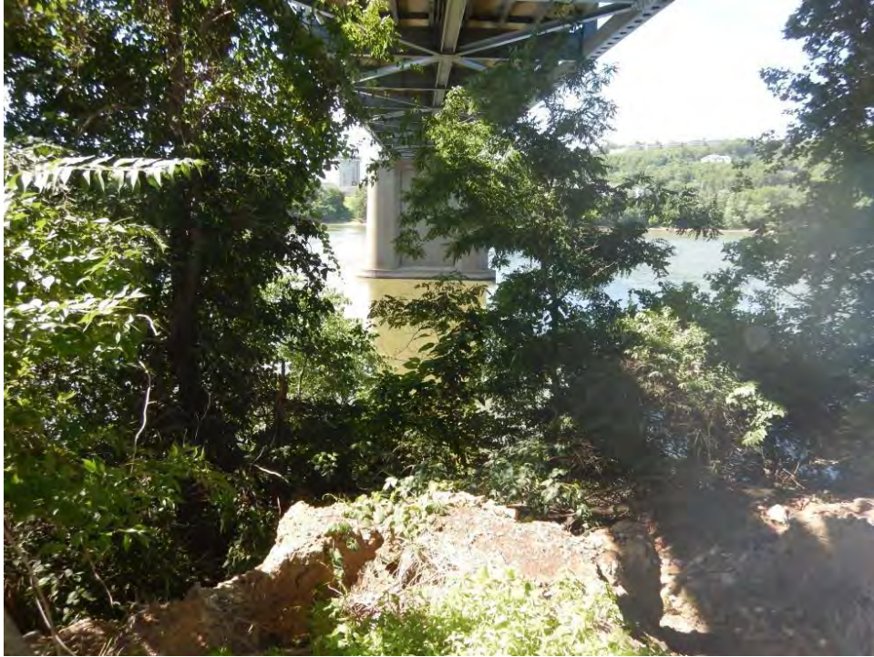
Photograph 6. View of SWH under the Brent Spence Bridge, looking south.
