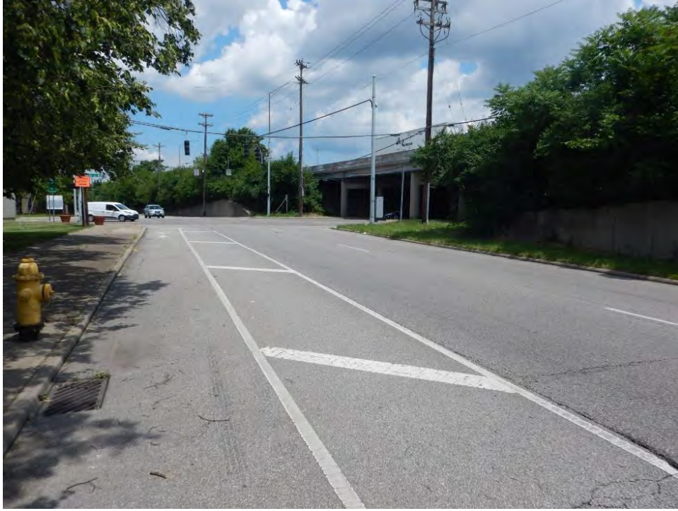
Photograph 100. View of I-75 right-of-way with SWH, looking northeast.
