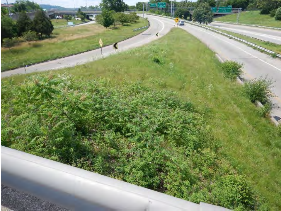
Photograph 34. View of I-75 right-of-way with mowed grass, looking northwest.
