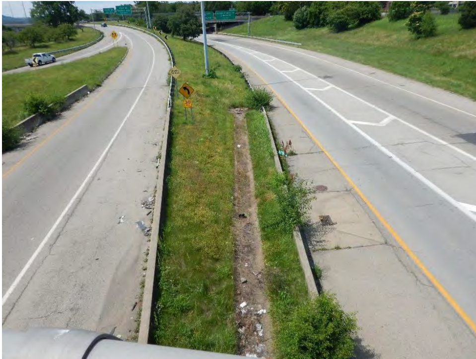
Photograph 33. View of I-75 right-of-way with mowed grass, looking northwest.
