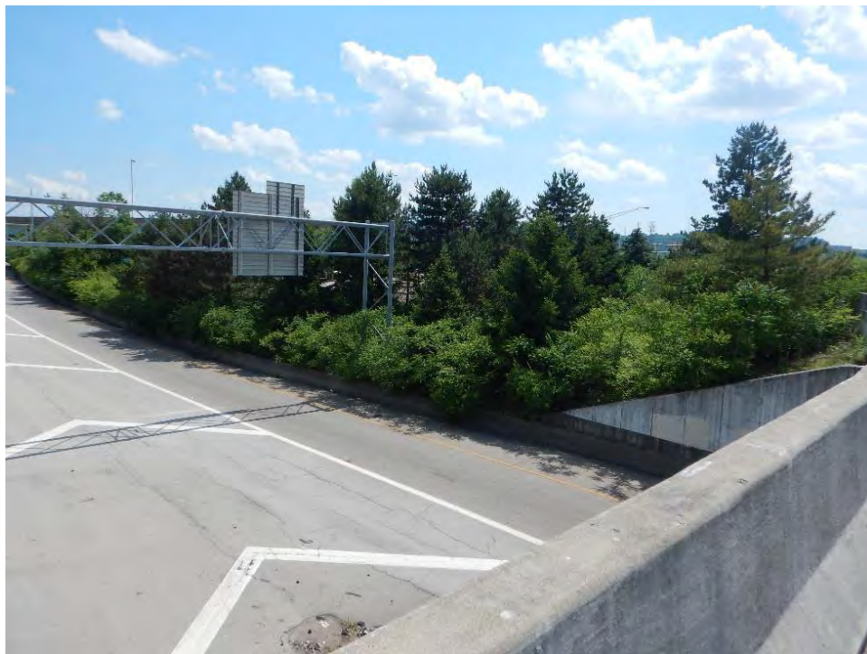
Photograph 30. View of I-75 right-of-way with pine trees and shrubby growth, looking southwest.
