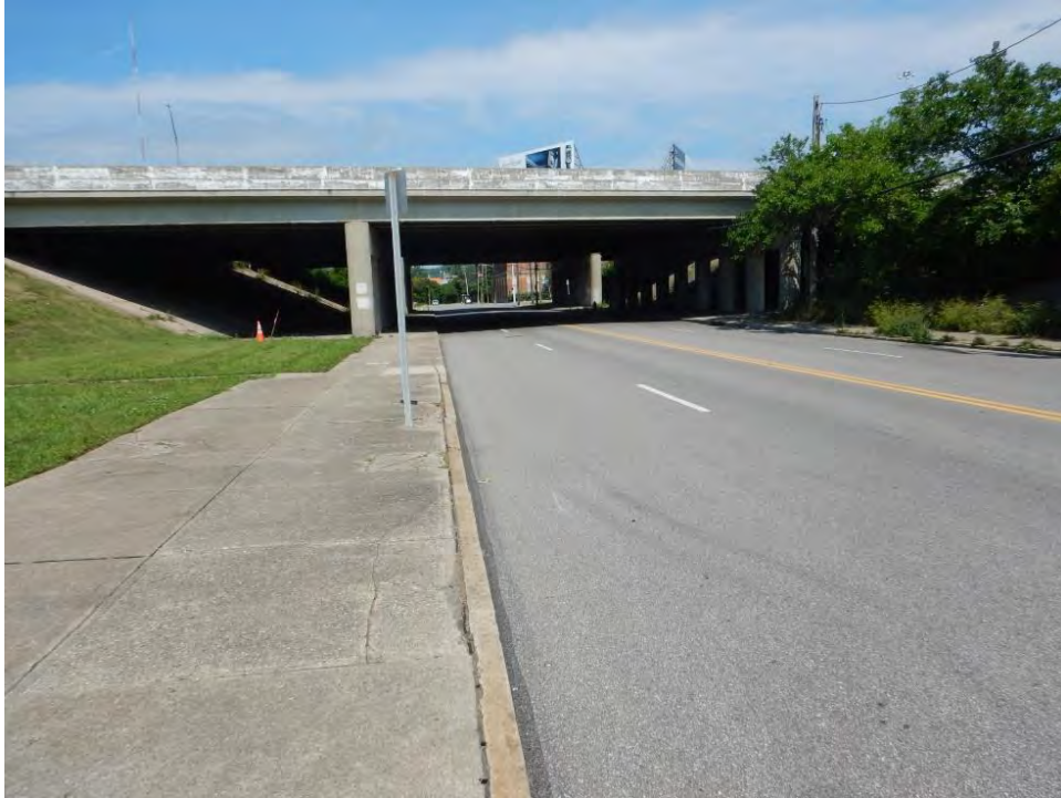
Photograph 129. View along Harrison Avenue, looking west.
