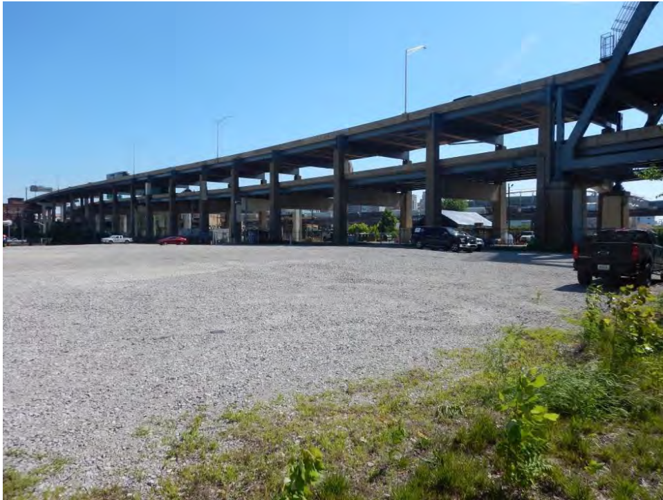
Photograph 5. View of the study area adjacent to the Brent Spence Bridge, looking northeast.
