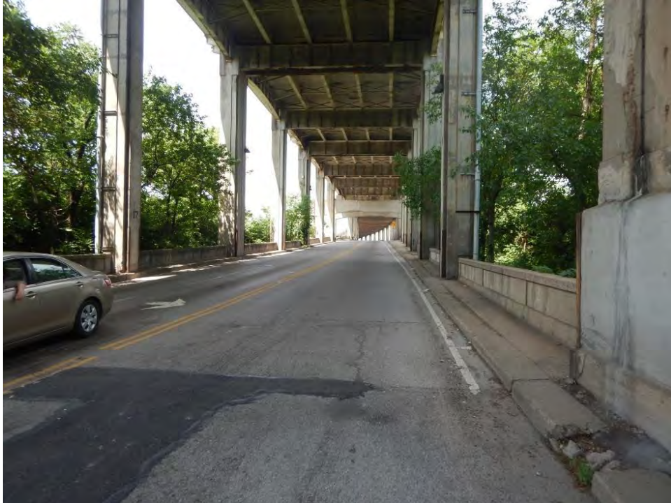
Photograph 140. View along Western Hills Viaduct, looking west.
