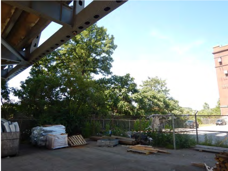
Photograph 7. View of SWH adjacent to the Brent Spence Bridge, looking southwest.
