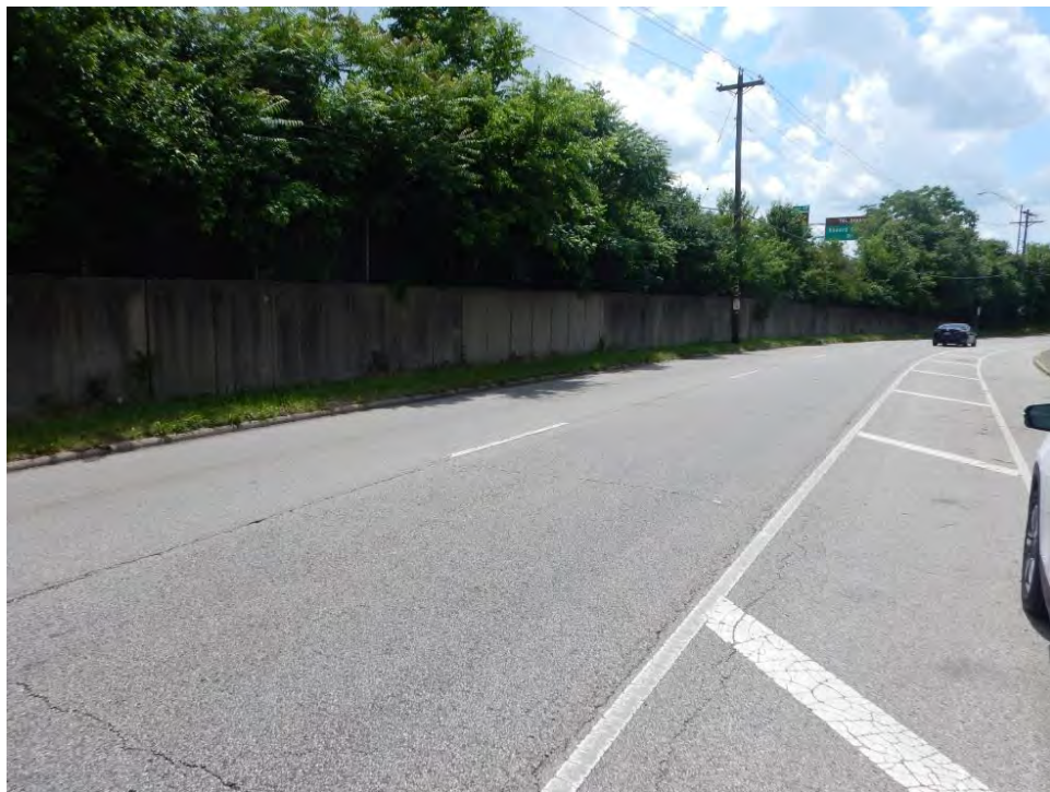
Photograph 96. View of Western Avenue with SWH, looking southeast.
