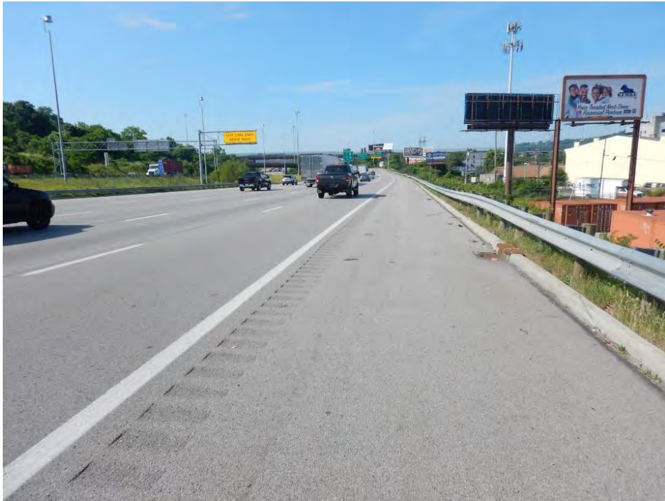
Photograph 153. View along I-75 and right-of-way, looking southwest.
