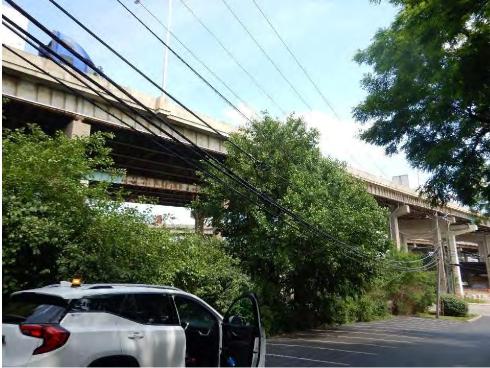
Photograph 20. View of I-75 right-of-way with SWH, looking southeast.
