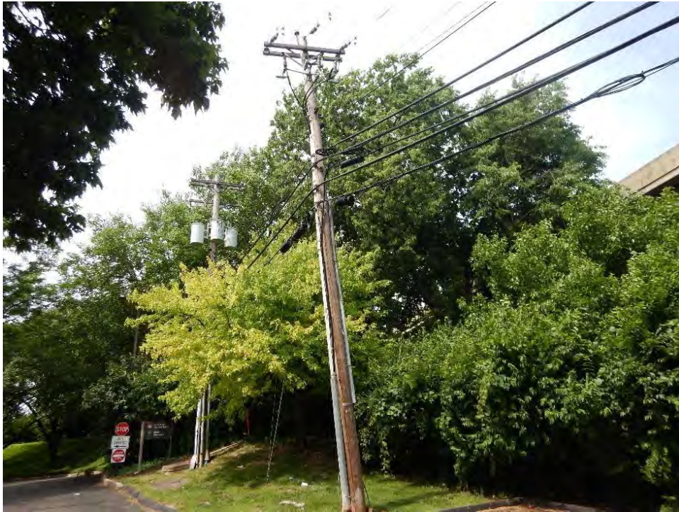
Photograph 21. View of I-75 right-of-way with SWH, looking northeast.
