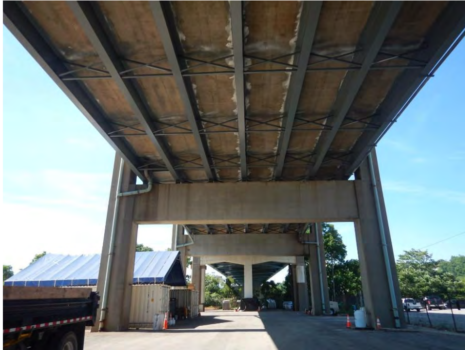
Photograph 9. View of the underside of the Brent Spence Bridge showing no signs of bat usage, looking south.
