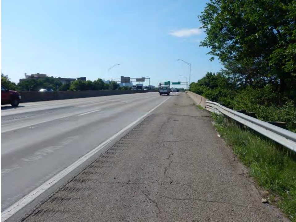
Photograph 114. View along I-75 and right-of-way with SWH, looking southeast.
