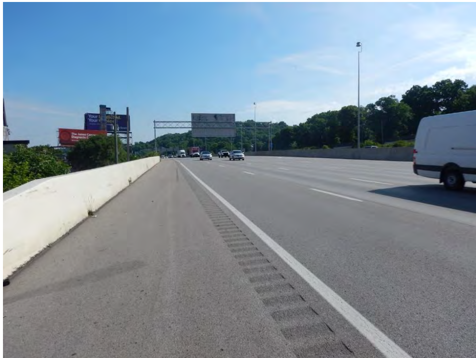
Photograph 155. View along I-75 and right-of-way, looking north-northeast.
