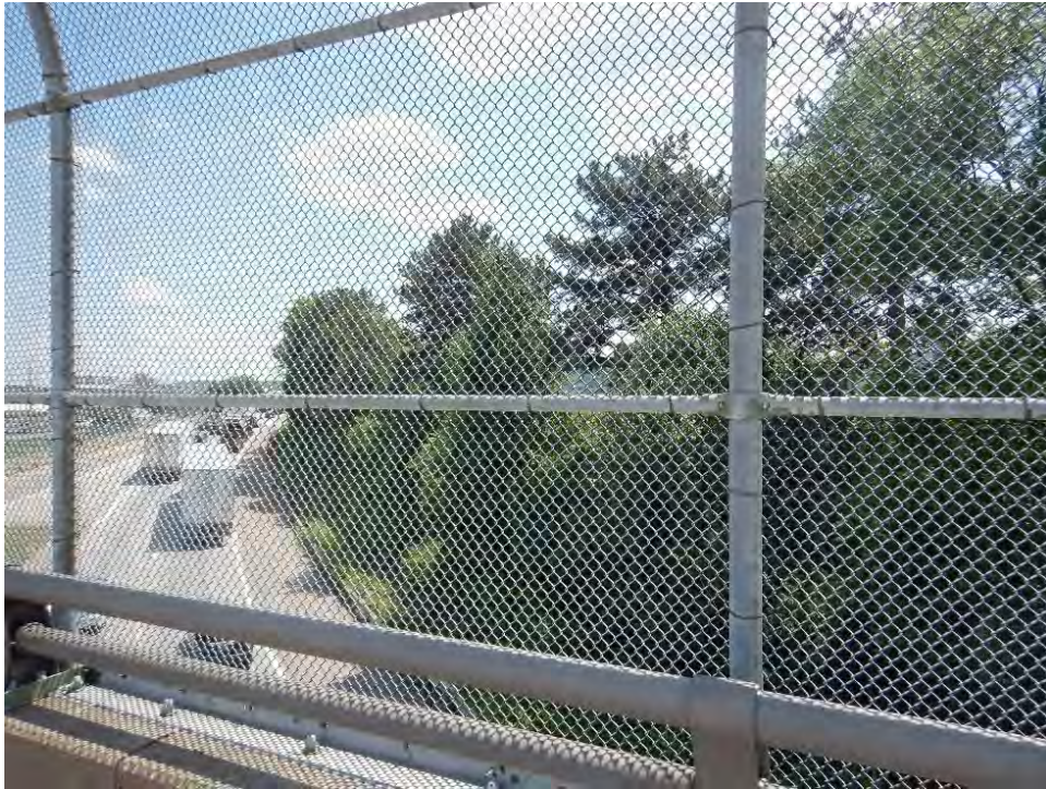
Photograph 45. View of I-75 right-of-way with SWH (right), looking south.
