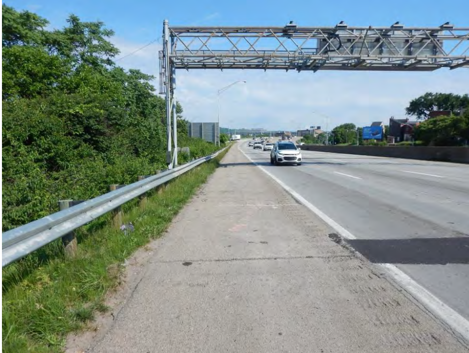
Photograph 115. View along I-75 and right-of-way with SWH, looking north-northwest.
