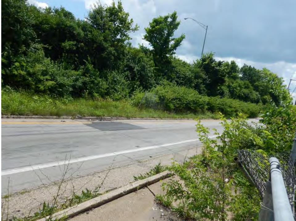
Photograph 116. View of I-75 right-of-way with SWH, looking southeast.
