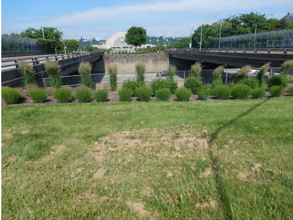
Photograph 90. View along I-75 and right-of-way, looking west.
