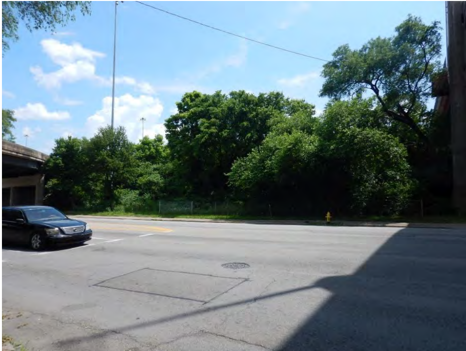
Photograph 141. View of I-75 right-of-way with SWH, looking east.
