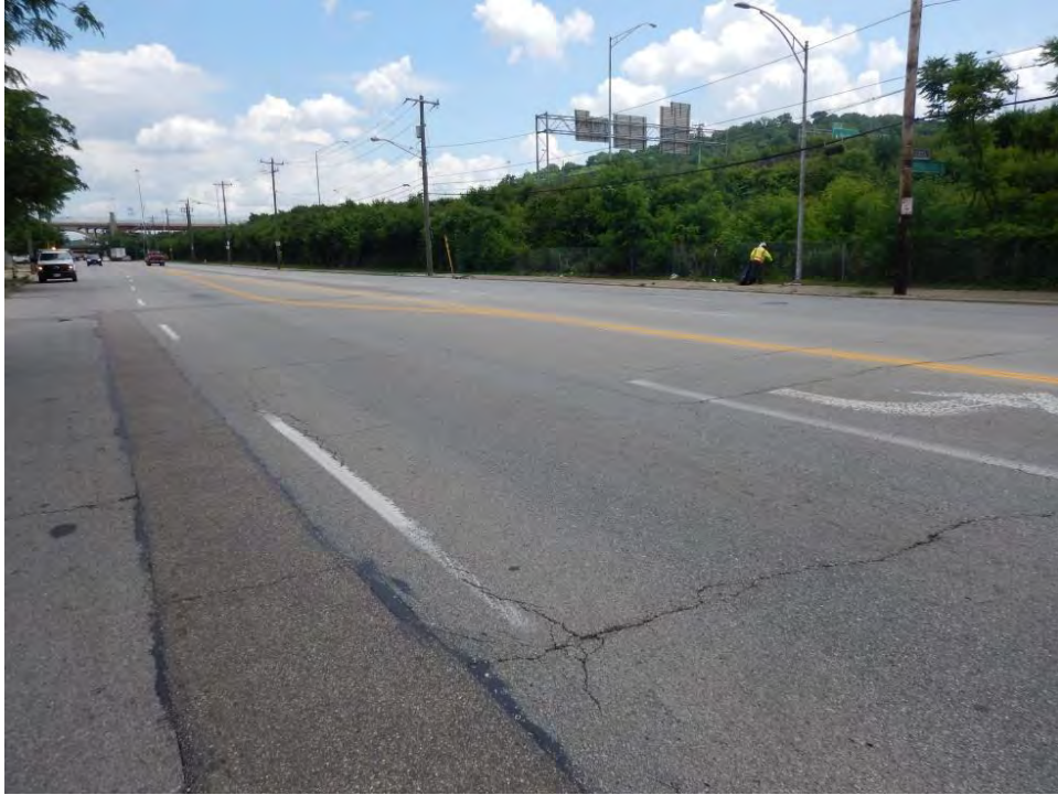
Photograph 126. View of I-75 right-of-way with shrubby vegetation, looking northeast.
