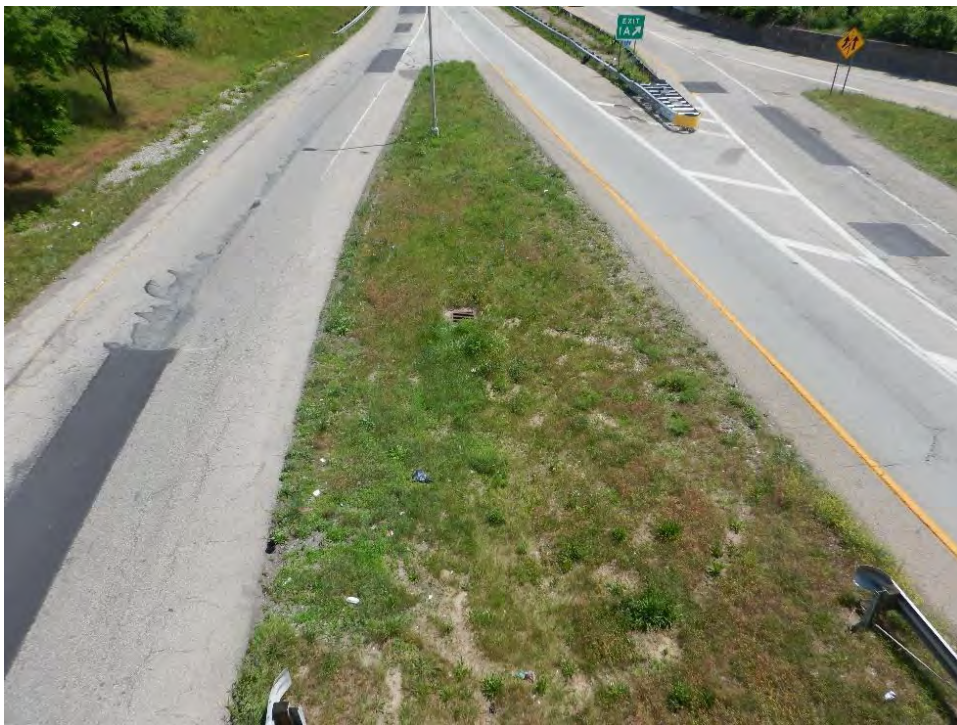
Photograph 40. View of I-75 right-of-way, looking south.
