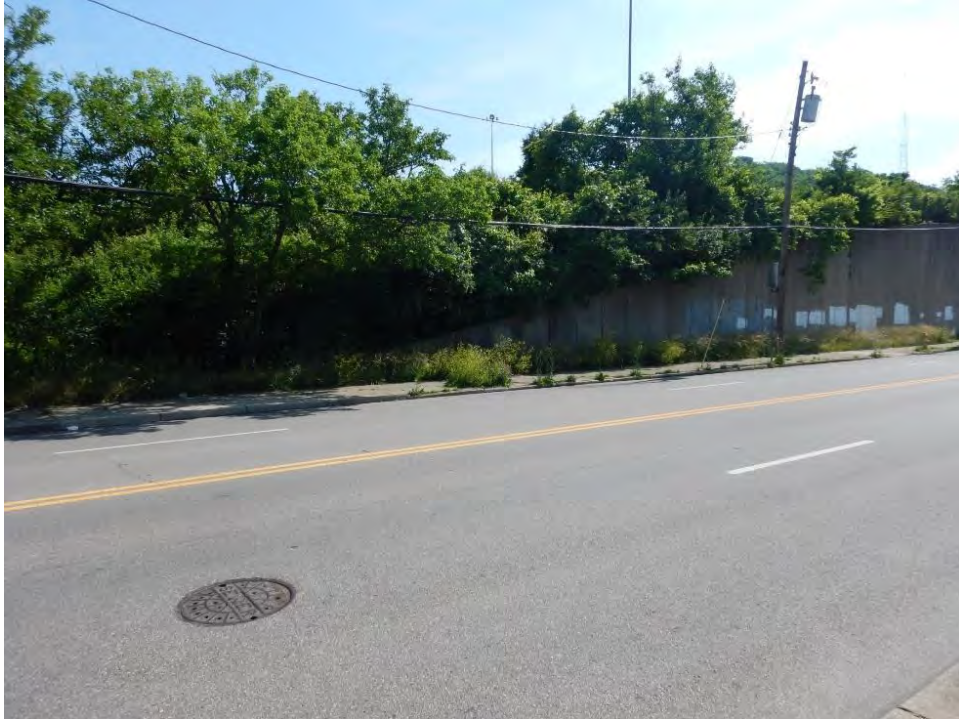
Photograph 128. View of I-75 right-of-way with SWH, looking northeast.
