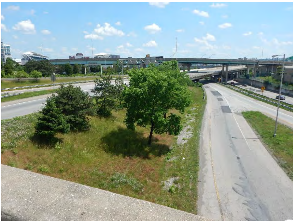
Photograph 38. View of I-75 right-of-way, looking south.
