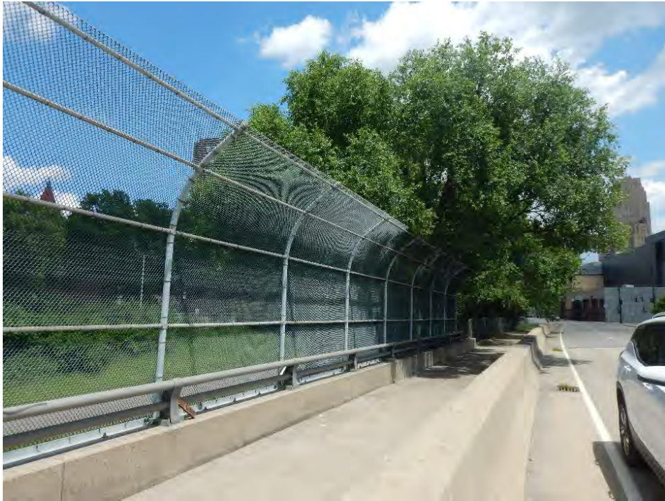
Photograph 53. View of along the 6 th Street Viaduct with SWH, looking east.
