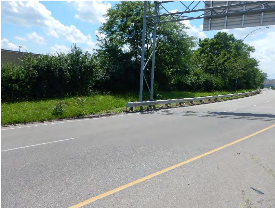
Photograph 51. View of SWH along Fort Washington Way, looking west-southwest.
