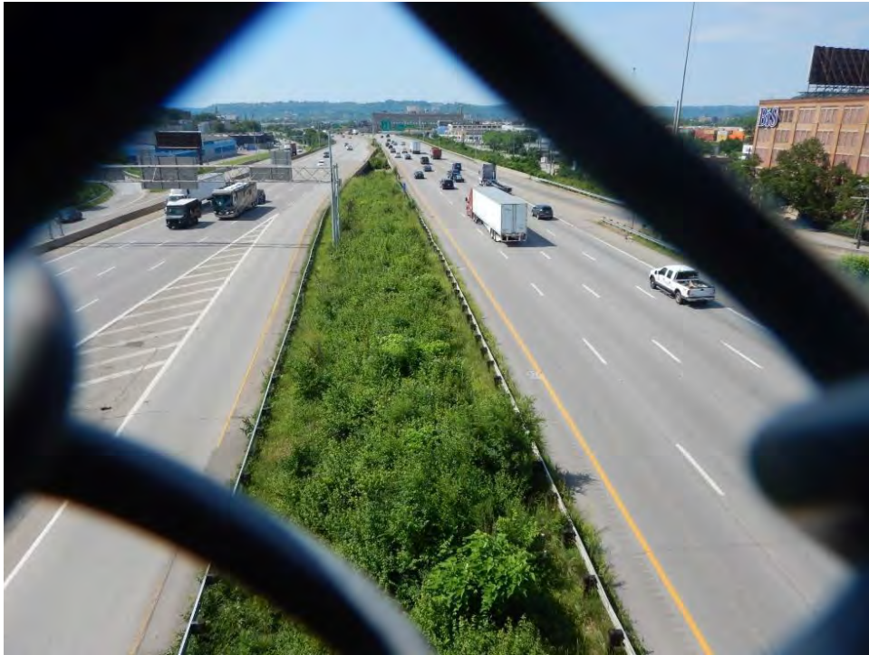
Photograph 139. View of I-75 right-of-way, looking south.
