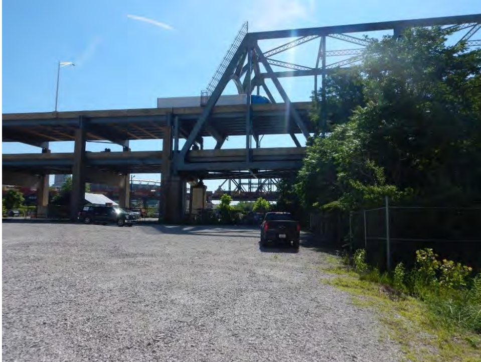
Photograph 3. View of SWH (right) adjacent to the Brent Spence Bridge, looking east.
