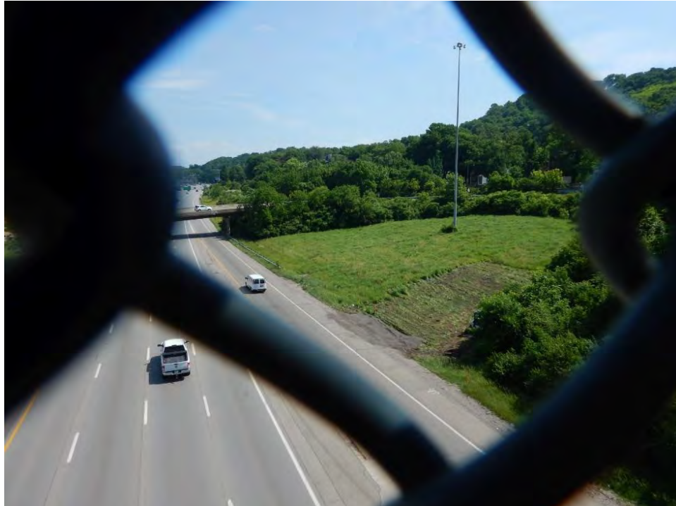
Photograph 143. View of I-75 right-of-way with SWH (along perimeter of interchange), looking northeast.
