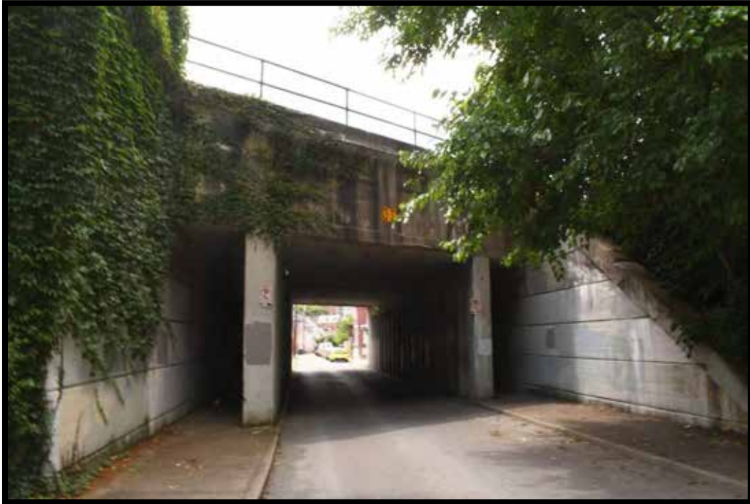
Plate 101. CSX Railroad Bridge No. 059R00626N, looking west.
