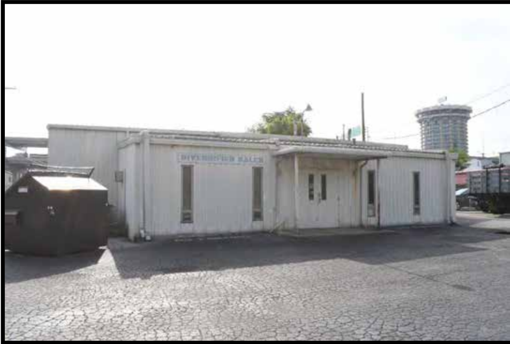
Plate 325. Commercial building, looking northeast.
