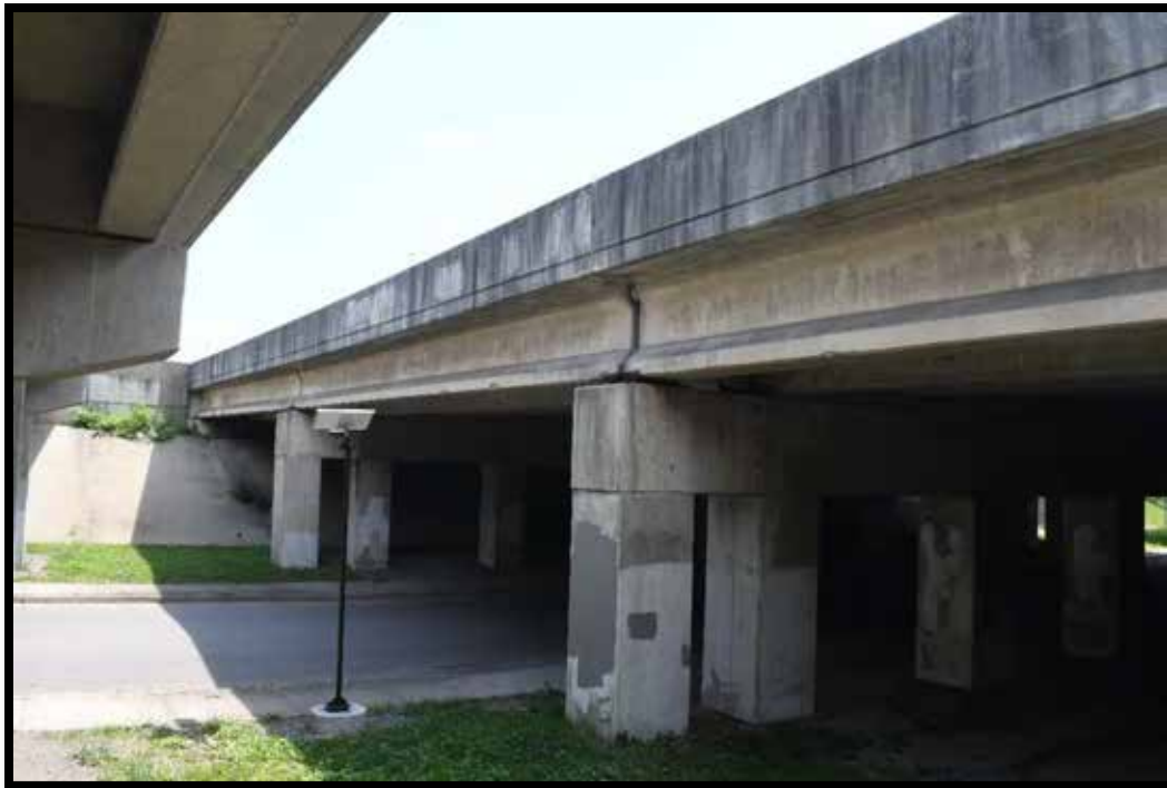
Plate 532. Bridge No. 059B00038R, looking north.
