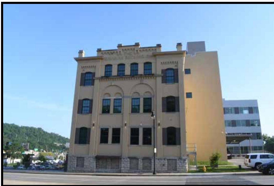
Plate 45. The Bavarian Brewing Co. / Kenton County Government Center looking north.
