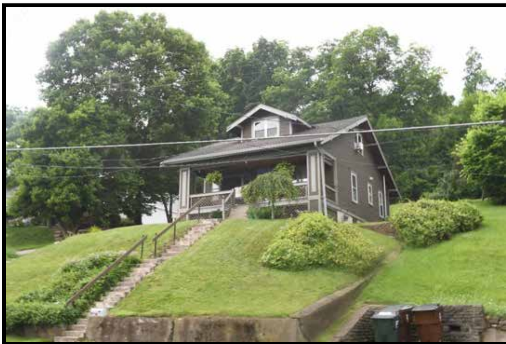
Plate 245. House, looking southwest.
