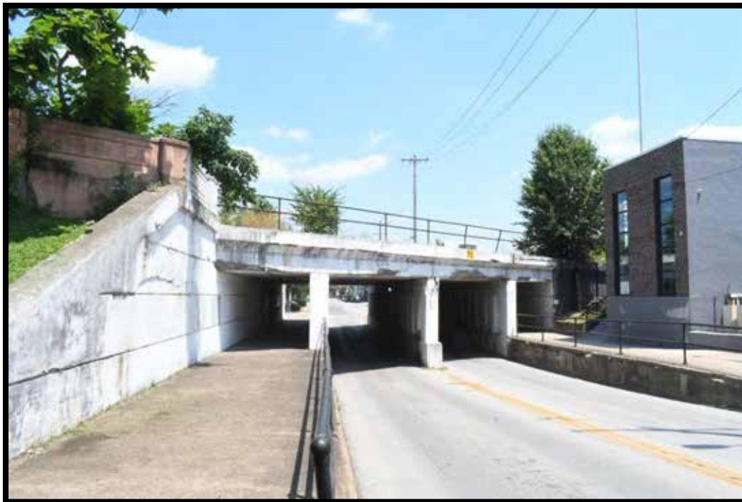
Plate 113. CSX Railroad Bridge No. 059R00621N, looking east.
