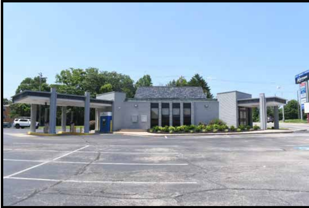
Plate 416. First National Bank Kentucky, looking northwest.
