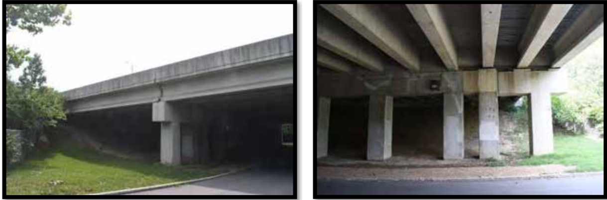
Plate 544. Bridge No. 059B0043R. Left: Bridge, looking west. Right: View of substructure.
