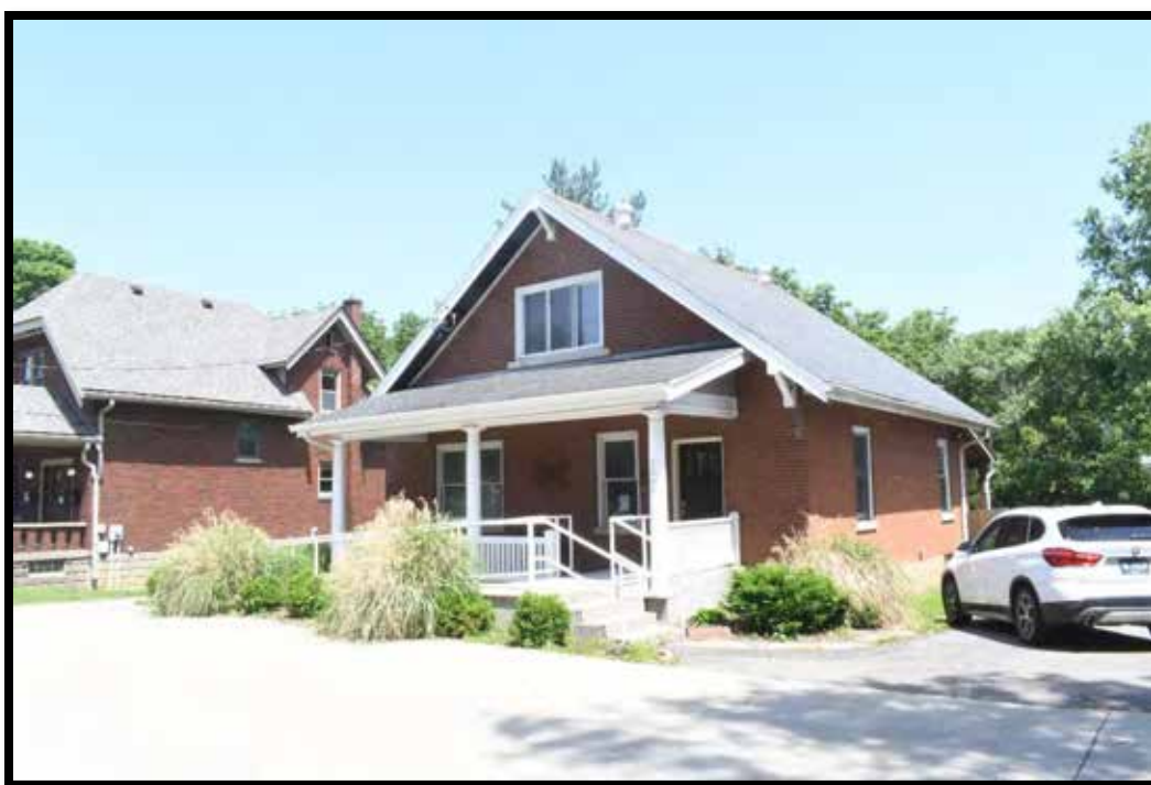
Plate 433. Office building, looking east.
