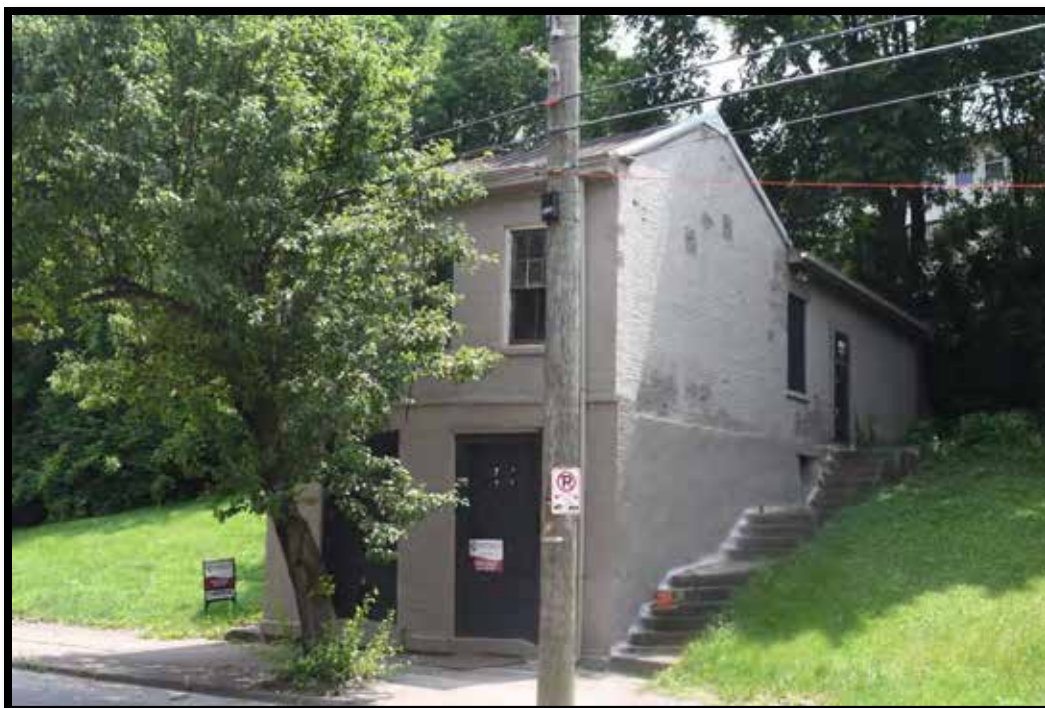
Plate 283. Commercial building, looking south.
