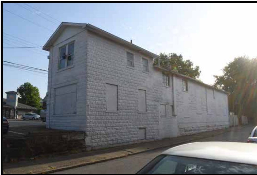
Plate 96. Commercial Building, looking northeast.
