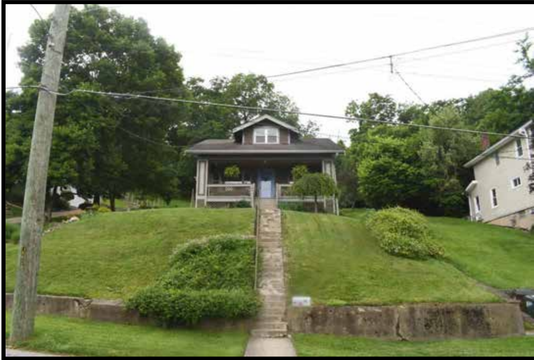
Plate 246. House and retaining wall, looking west.
