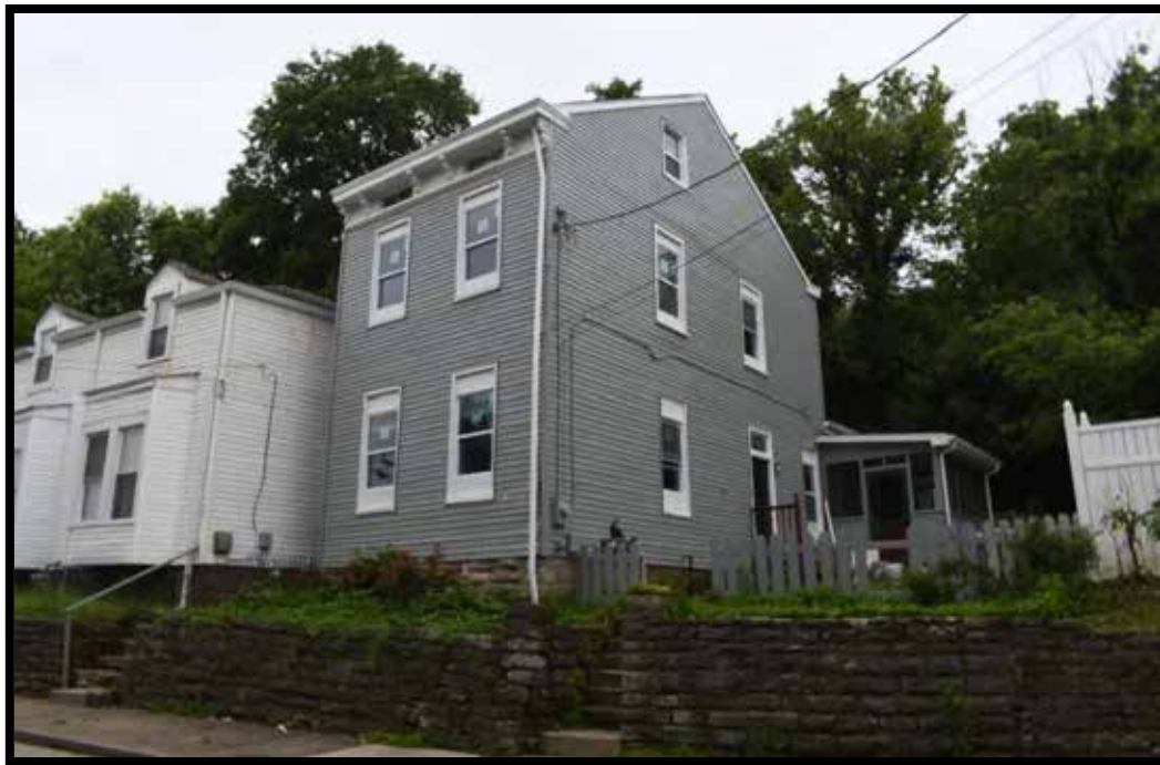
Plate 316. House and retaining wall (B), looking southwest.
