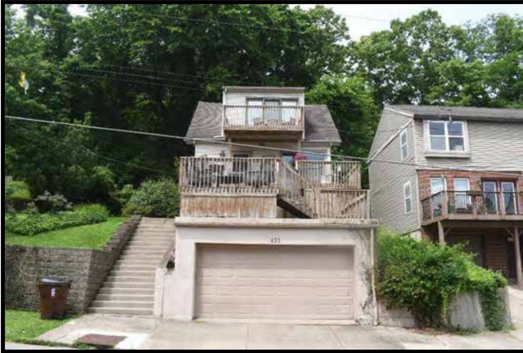
Plate 250. House, looking west.
