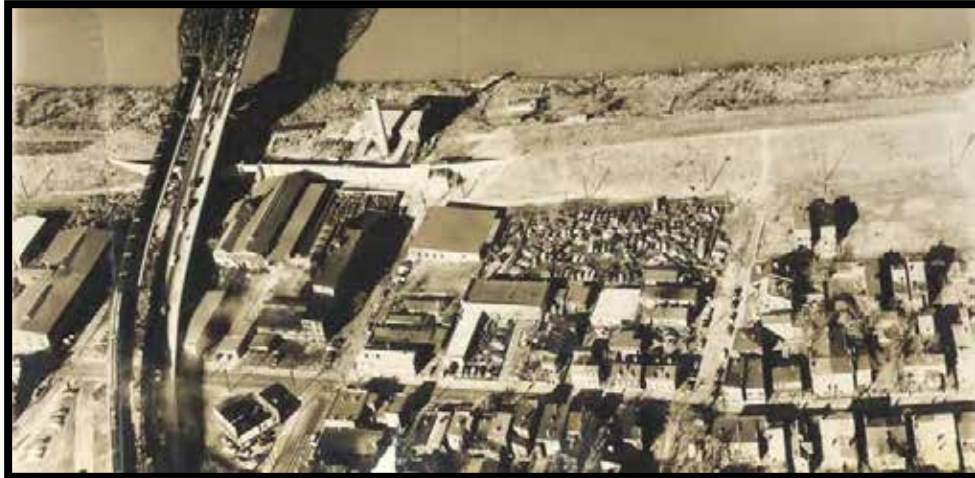
Figure 45. Covington Levee System. Circa 1956 aerial of earthen levee and concrete levee wall and gate between Bakewell and Johnson Streets. 197
