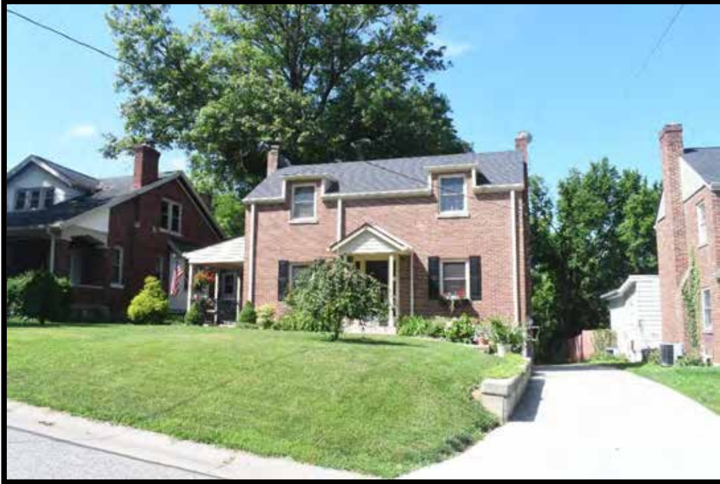
Plate 473. House, façade, looking southwest.
