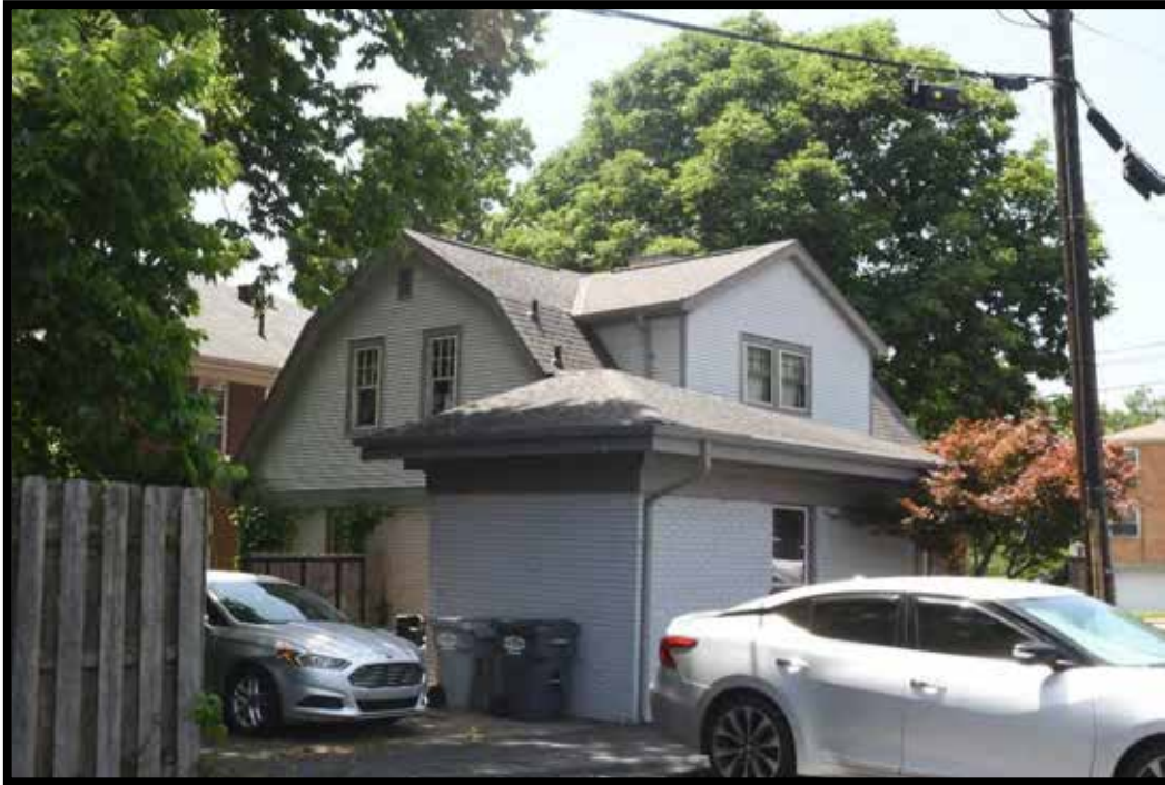
Plate 414. Office Building, looking west.
