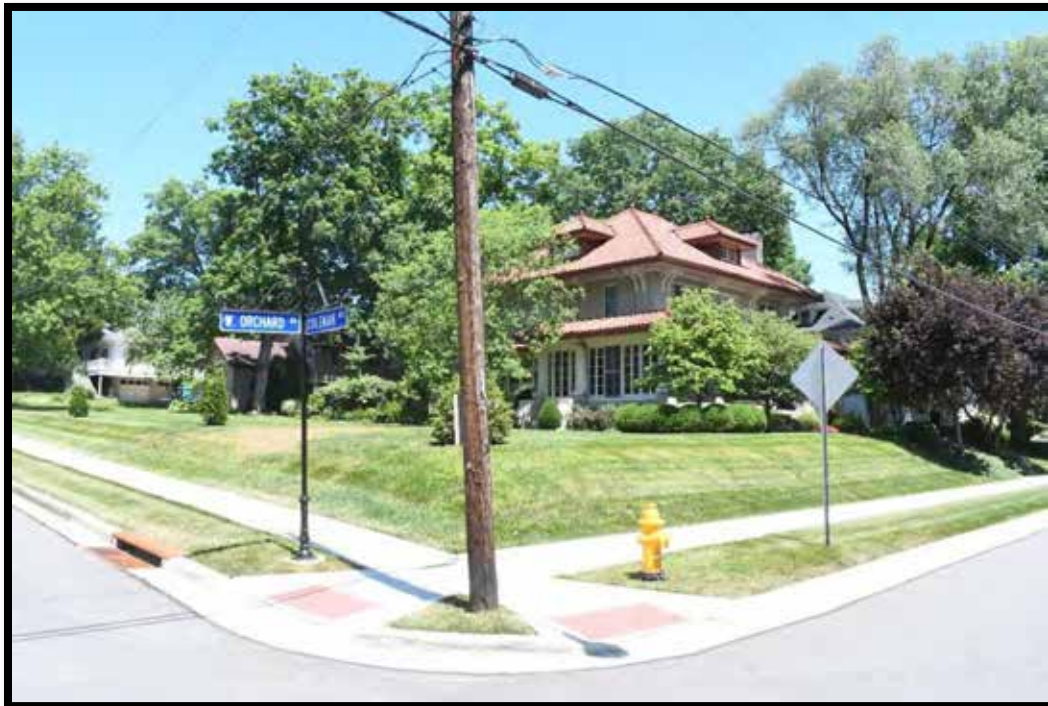
Plate 160. Looking NE at the Fred Hilker House (KEFM-222) at 36 West Orchard Road.
