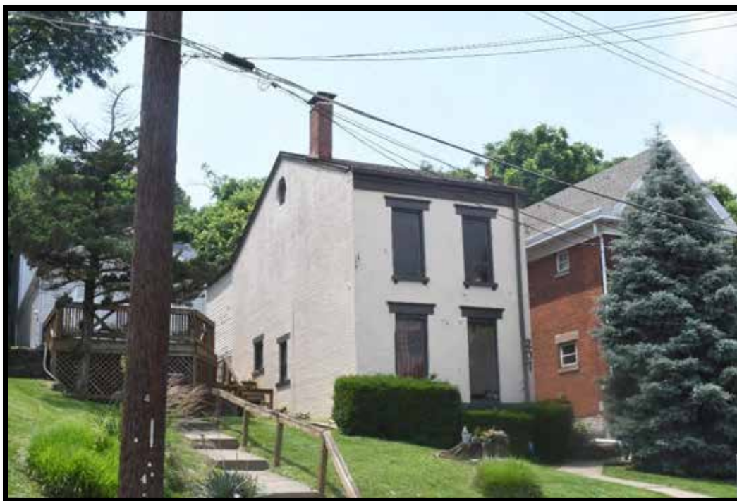
Plate 276. House, looking NW.
