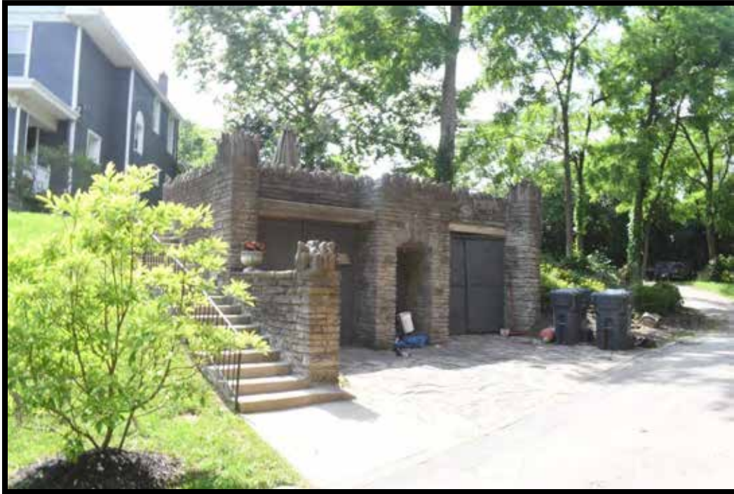
Plate 62. Garage (B), looking west.
