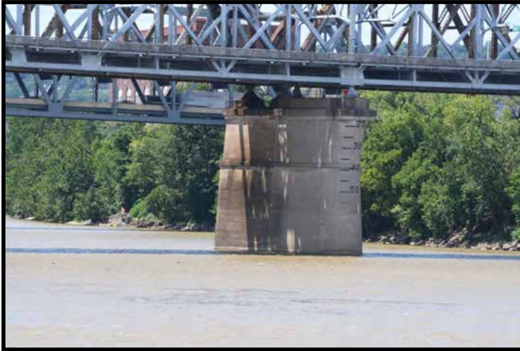
Plate 81. Detail of shared bridge pier showing depth markings, looking west
