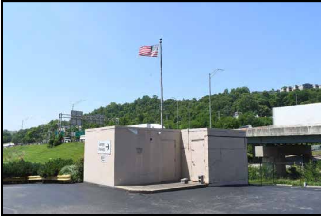
Plate 34. Outbuilding (B), looking southwest.
