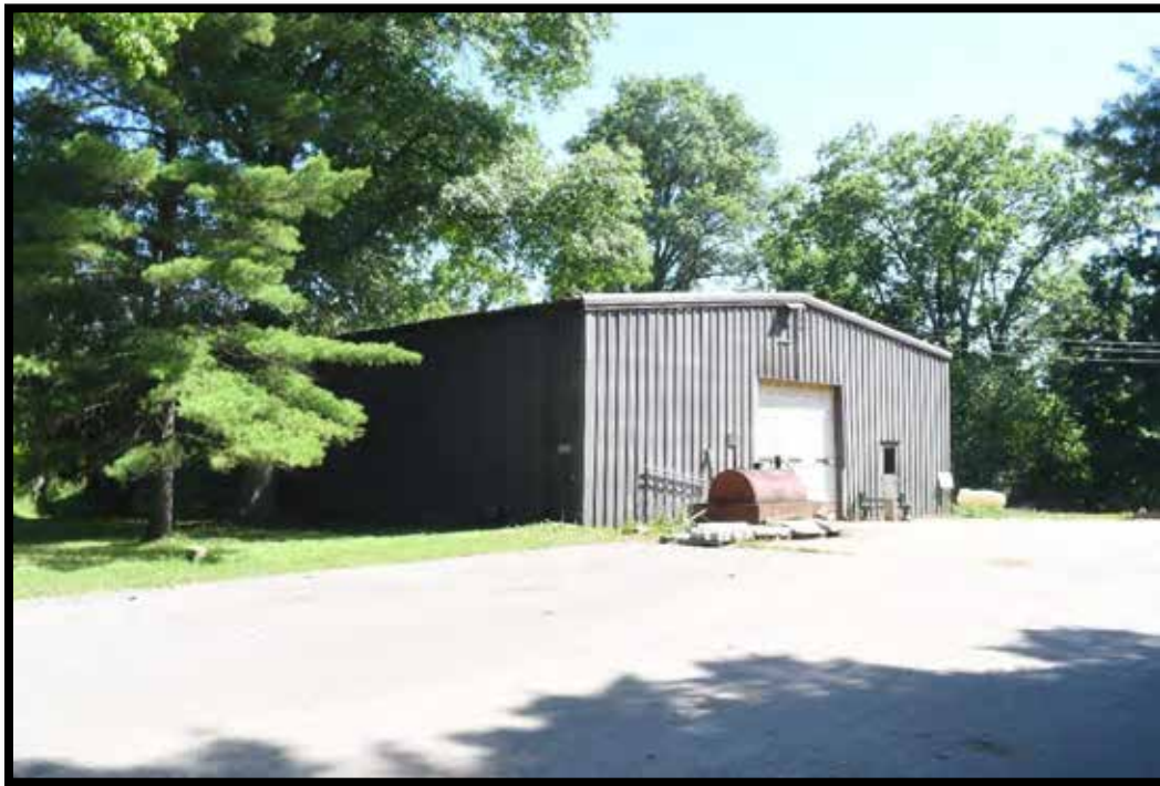
Plate 193. Highland Cemetery. Maintenance garage (G), looking south.
