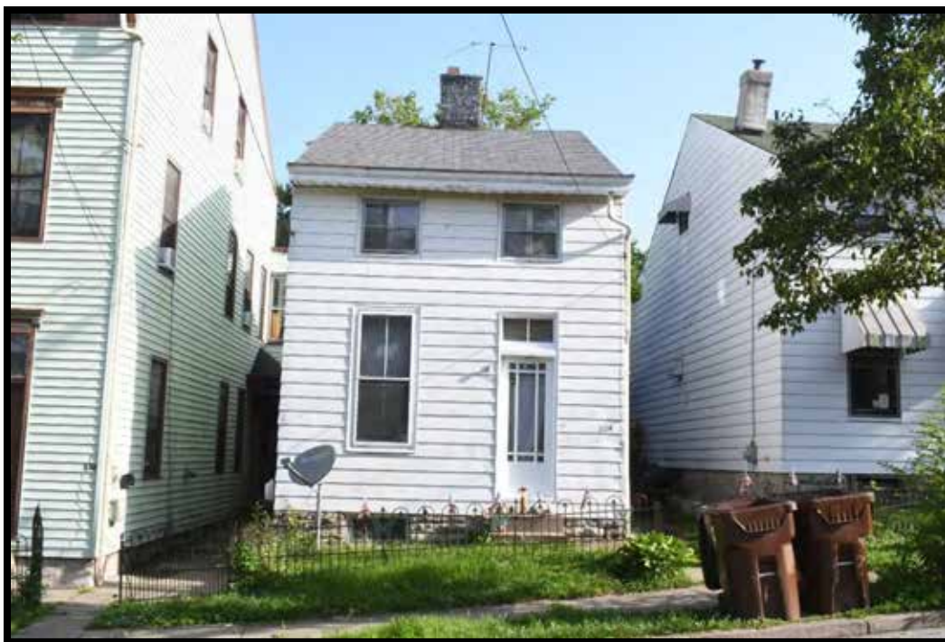
Plate 54. House and decorative wrought iron fence (B), looking north.
