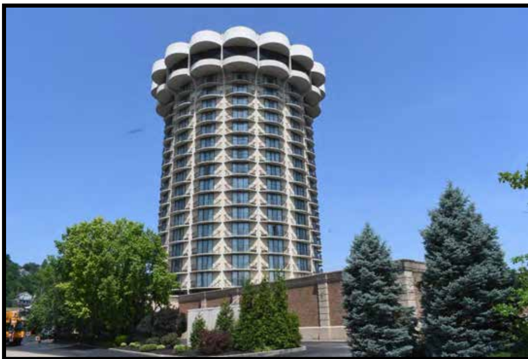
Plate 31. The Quality Inn / Radisson Hotel, looking northwest.
