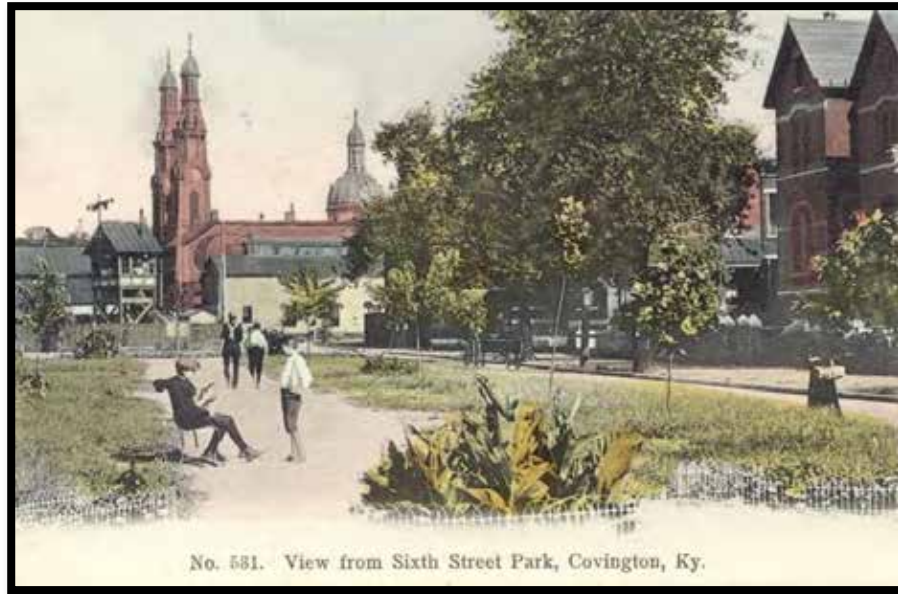
Figure 65. Circa 1900-postcard image of Sixth Street Park depicting the railroad prior it being elevated. 261
