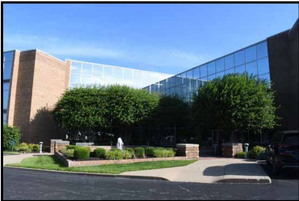
Plate 444. Triangular plaza (B), looking north.
