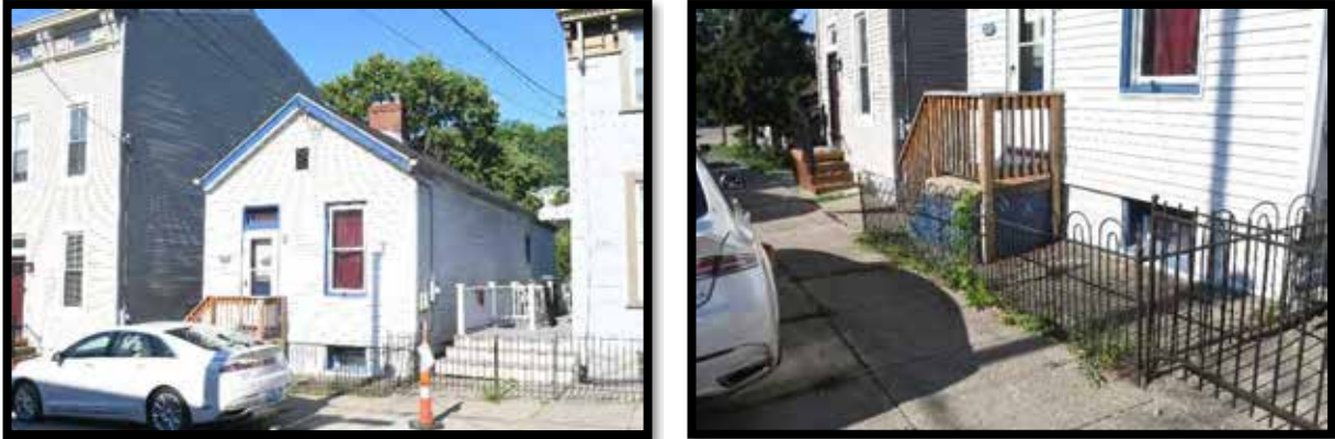
Plate 118. Left: House, looking southwest. Right: Fence (B), looking northwest.
