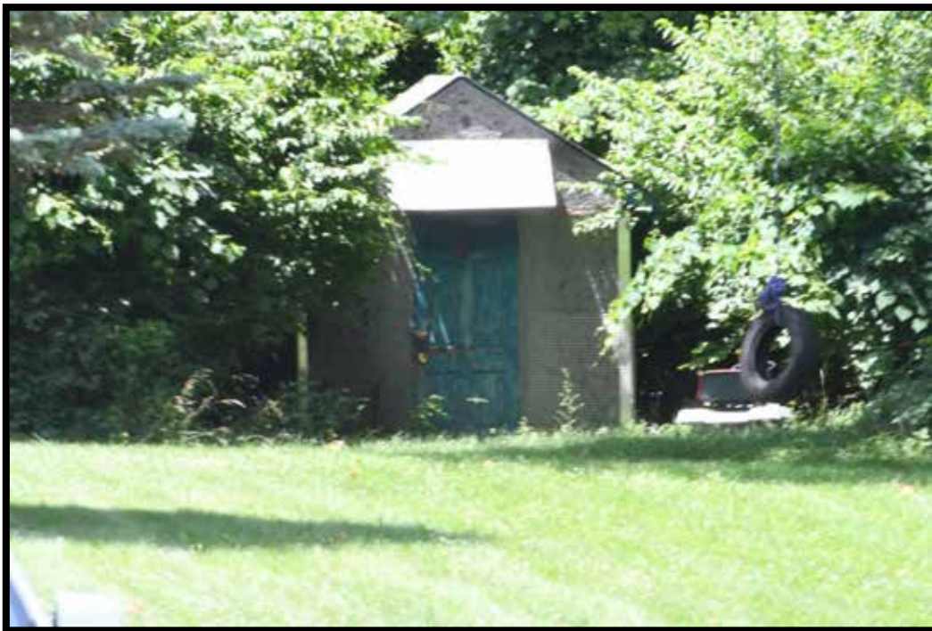
Plate 496. Storage shed (B), looking northwest.
