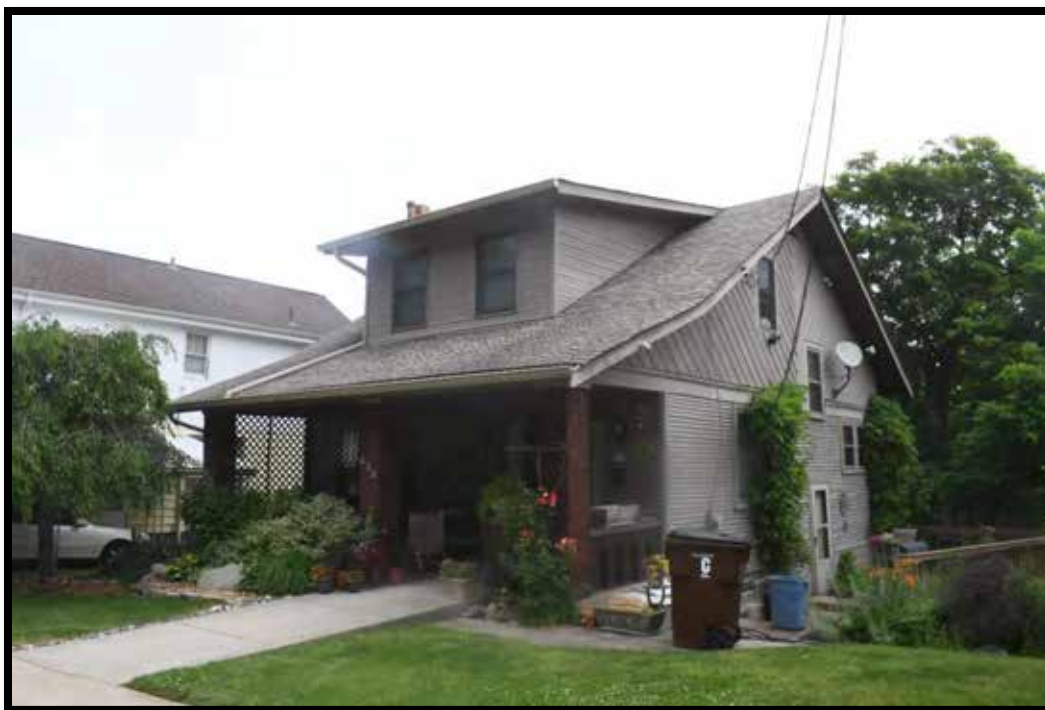
Plate 217. House, looking northeast.
