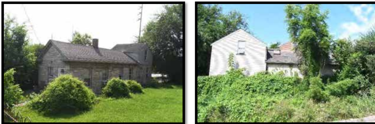
Plate 152. Left: View of façade and southwest side of house. Right: View of northeast side of house showing brick.
