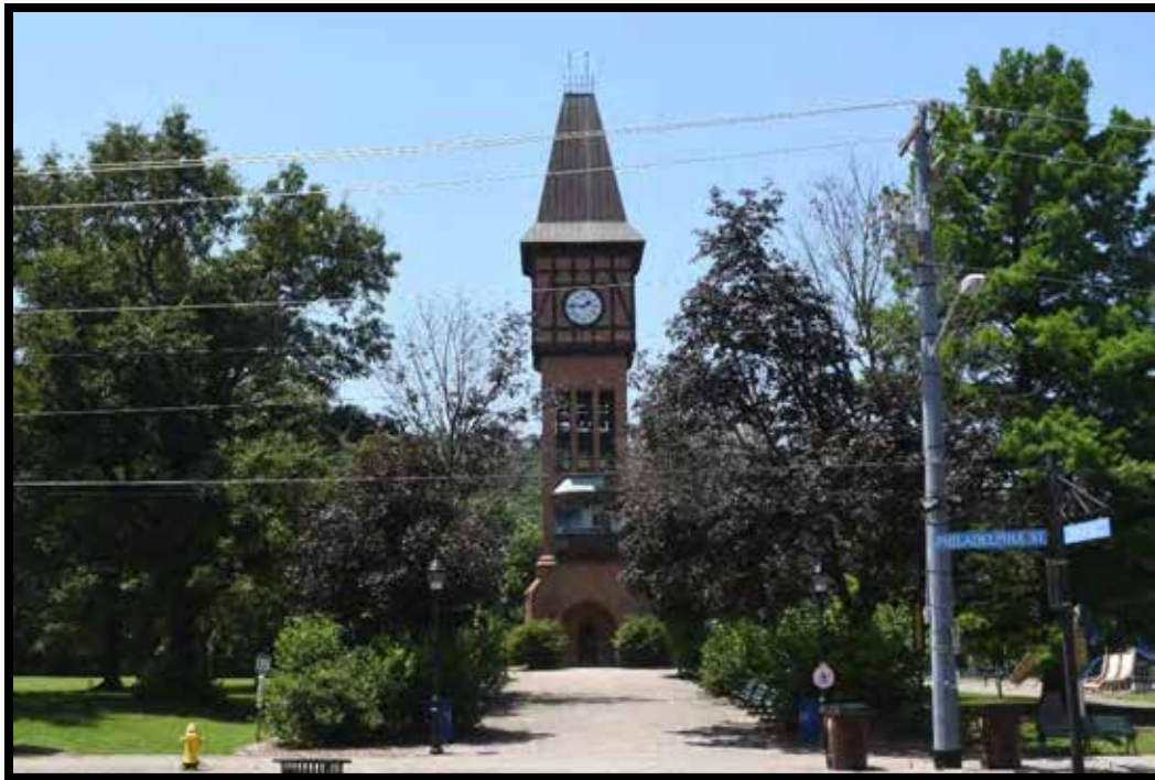
Plate 349. Carroll Chimes Bell Tower, looking west.
