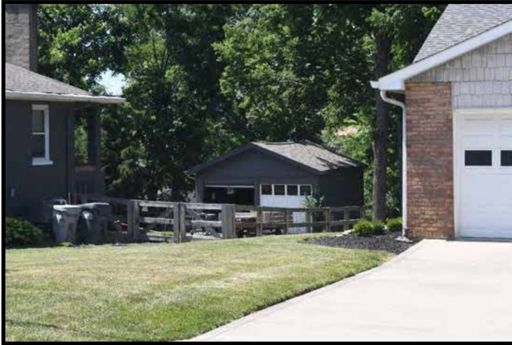
Plate 548. Garage, looking northwest.
