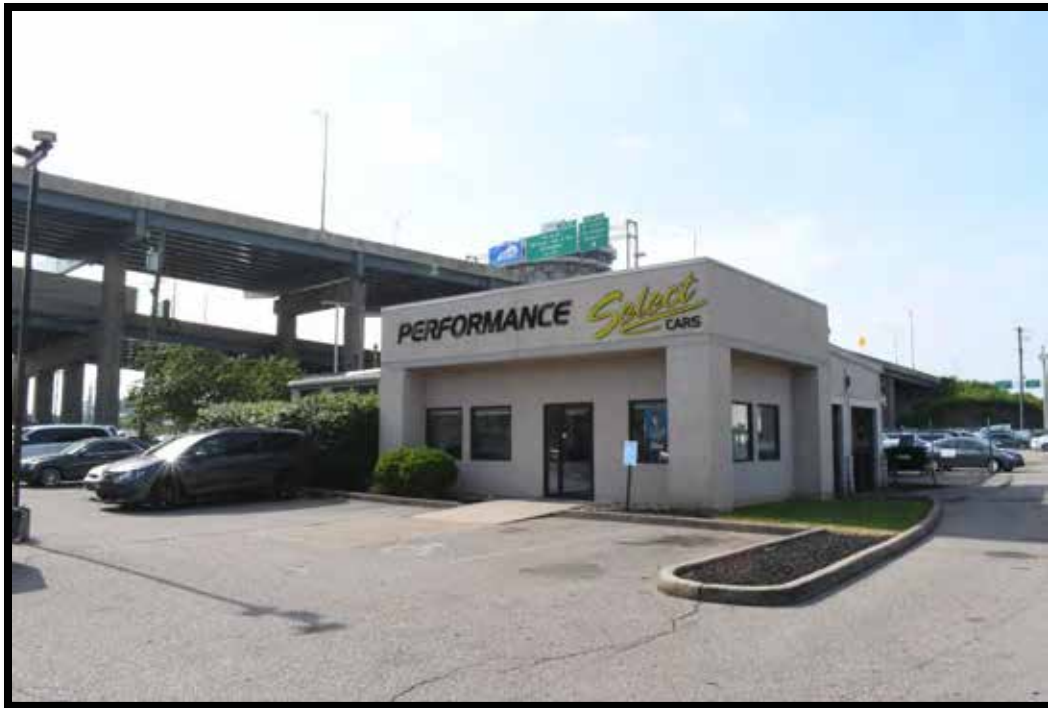
Plate 326. Commercial building, looking southeast.
