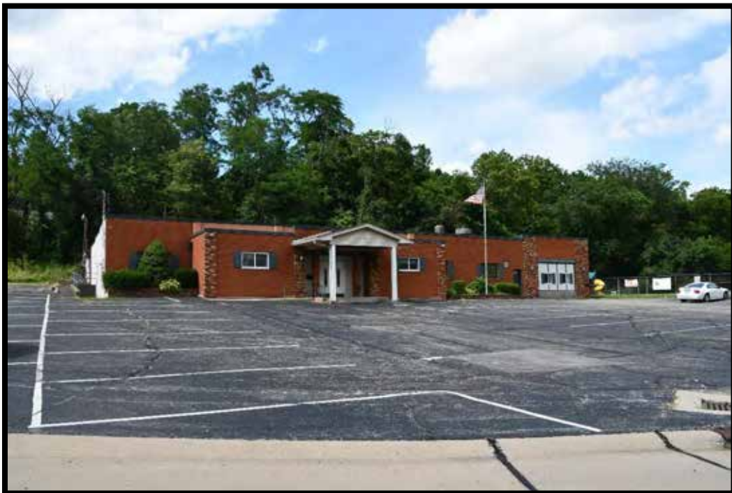
Plate 203. Fort Wright Civic Center, 115 Kennedy Road at east end of district, looking north
