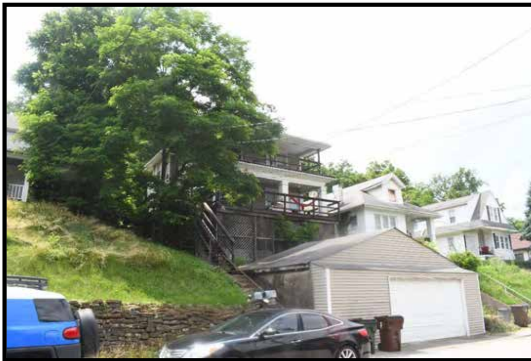
Plate 296. House and garage (B), looking NW.
