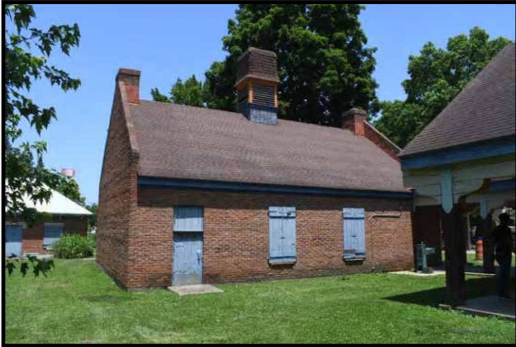
Plate 351. Outbuilding (D), looking north.
