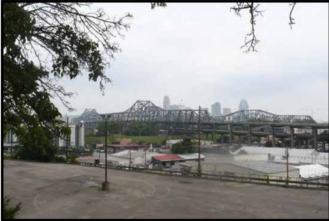
Plate 1. Northern section of the Project Area, looking NW from Western Avenue.
