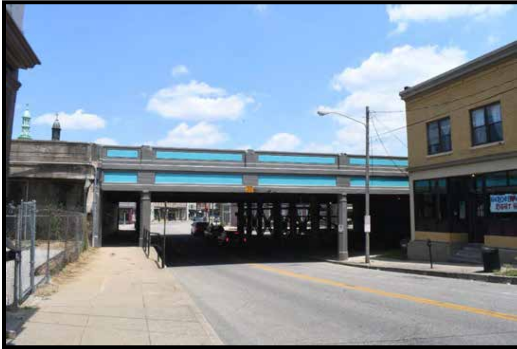
Plate 105. CSX Railroad Bridge No. 059R00617N, looking NE
