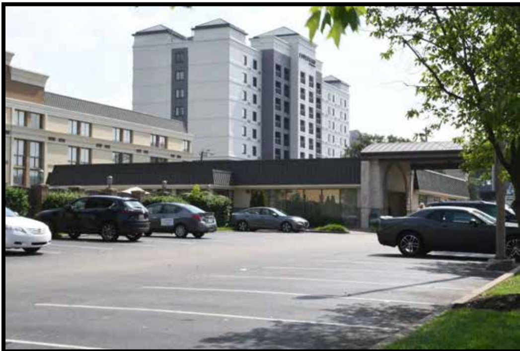
Plate 336. Commercial building breezeway, looking northeast.
