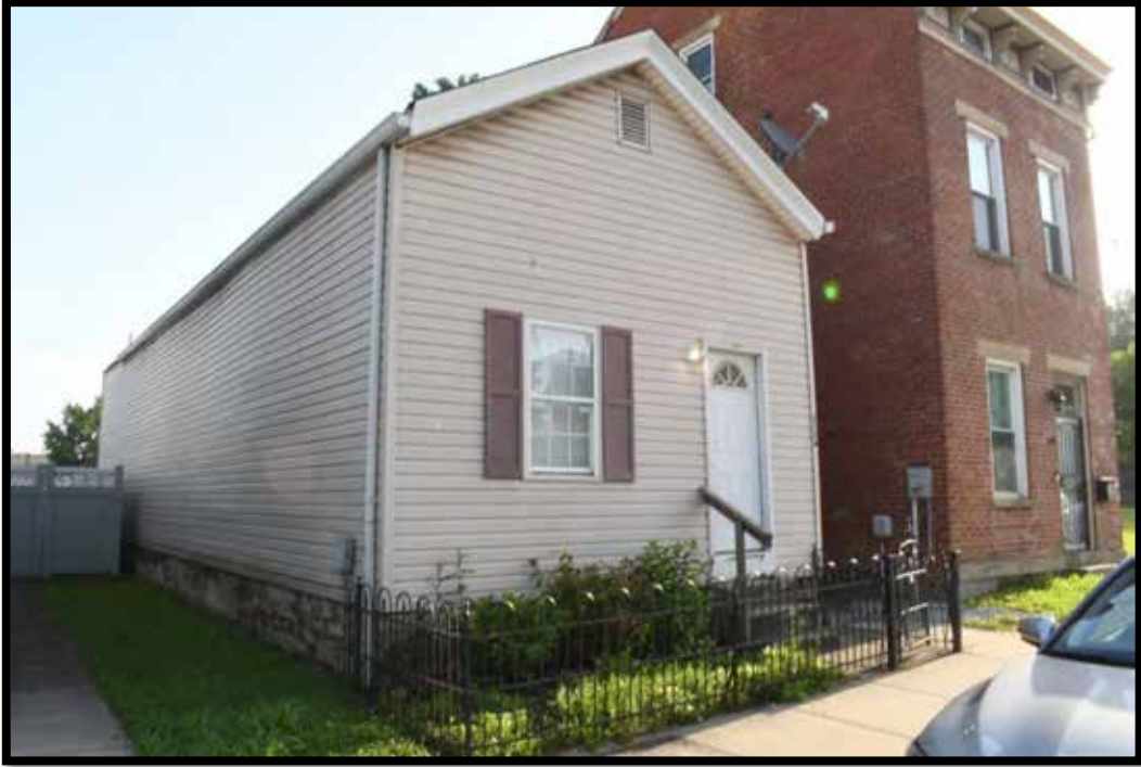
Plate 90. House, looking northeast.
