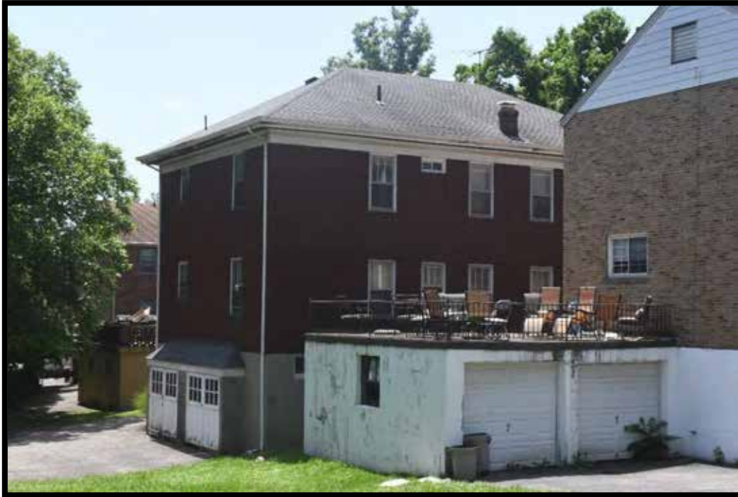
Plate 420. Apartment, looking southwest.
