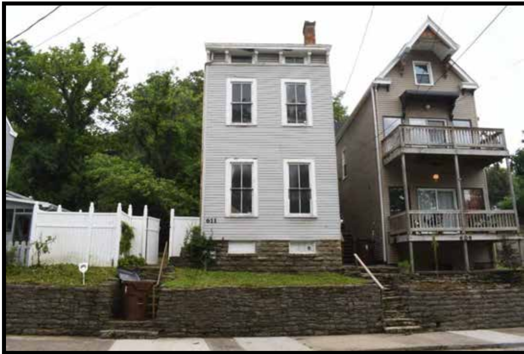
Plate 14. House and retaining wall (B), looking west.
