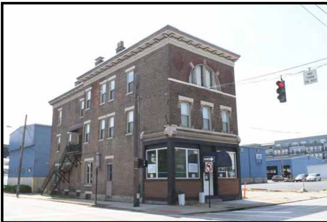
Plate 17. Commercial building, looking southeast.
