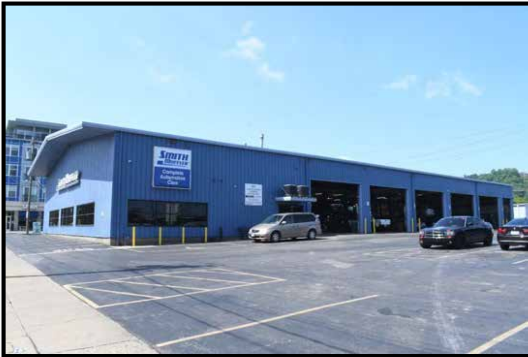
Plate 343. Commercial building, looking southwest.
