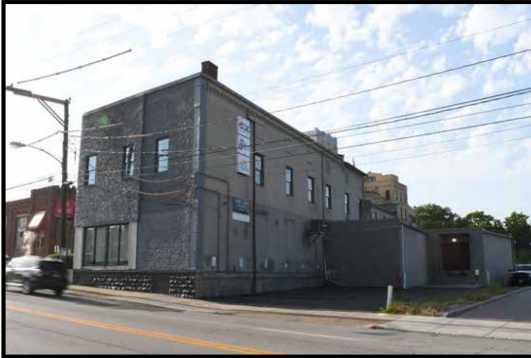
Plate 365. Commercial Building, looking southeast.
