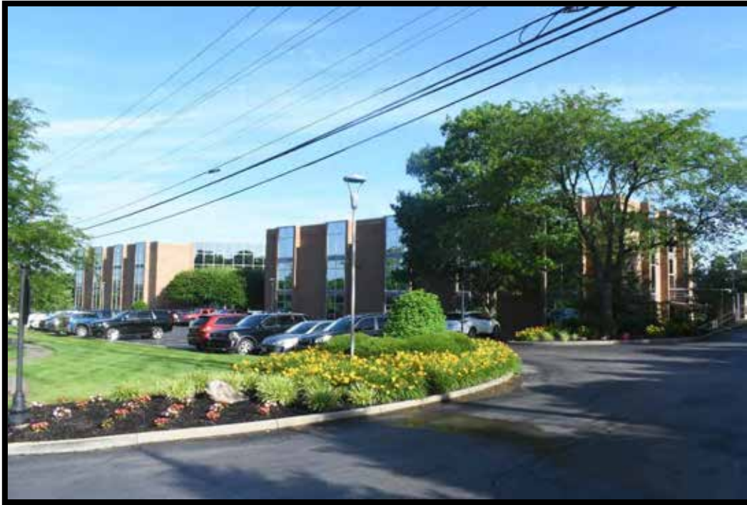
Plate 442. Fort Mitchell Executive Center, façade, looking northwest.
