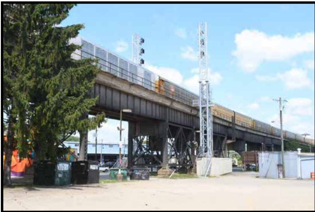
Plate 28. CSX Railroad Bridge No. 059R00610N (KEC-1065), looking NW.
