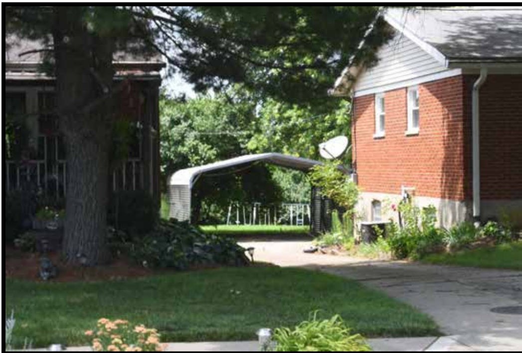
Plate 513. Carport (B), looking northwest.
