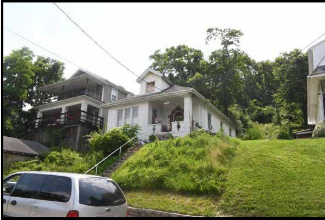
Plate 298. House, looking SW.
