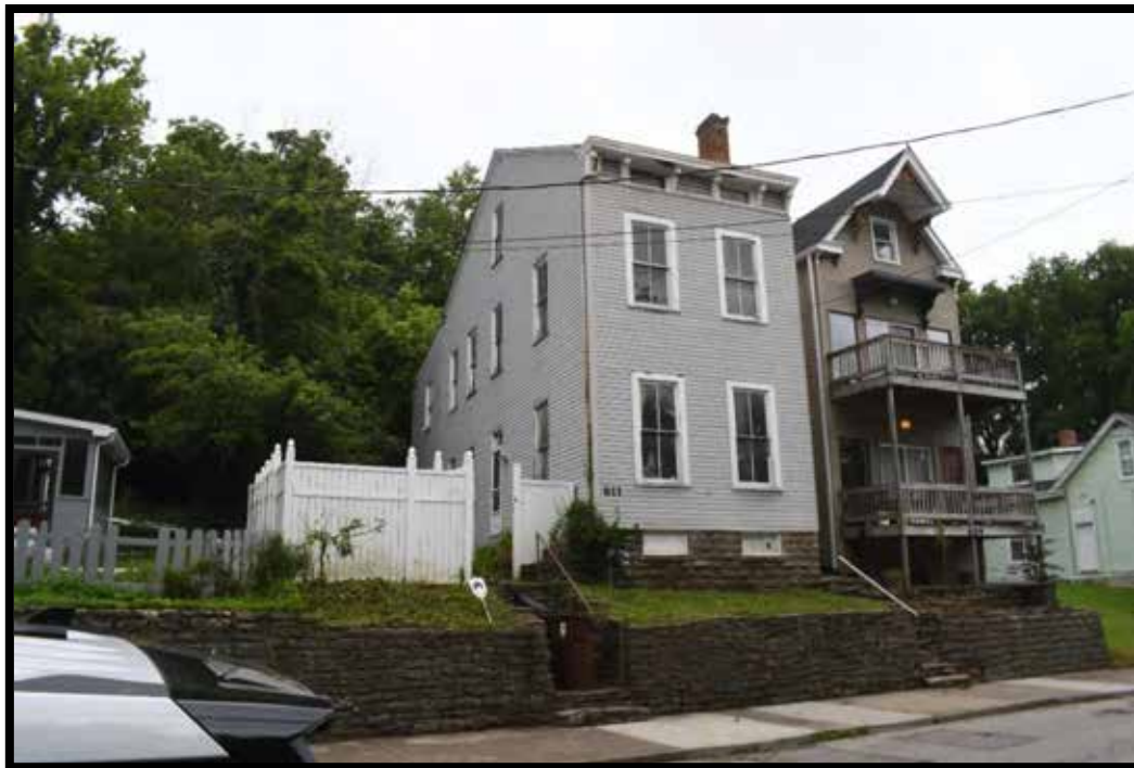
Plate 15. House and retaining wall (B), looking northwest.
