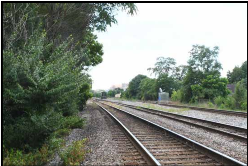
Plate 102. CSX Railroad Bridge No. 059R00626N. Sets of tracks over bridge, looking south.
