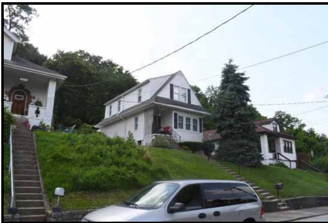
Plate 299. House, looking NW.
