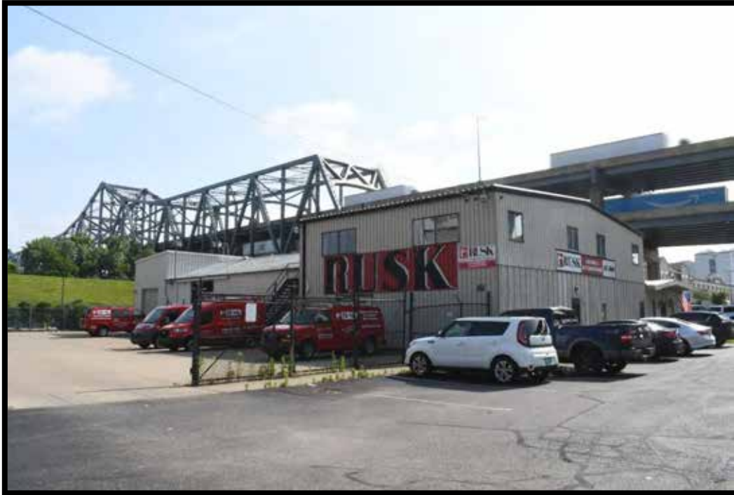
Plate 333. Commercial building, looking northeast.
