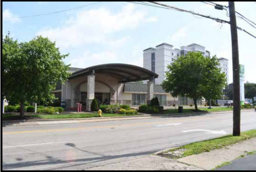
Plate 335. Commercial building entrance to lobby, looking northeast.
