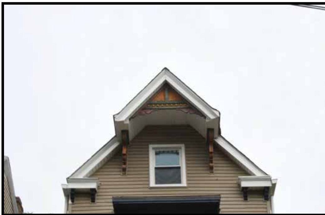
Plate 318. Detail of roof hood.
