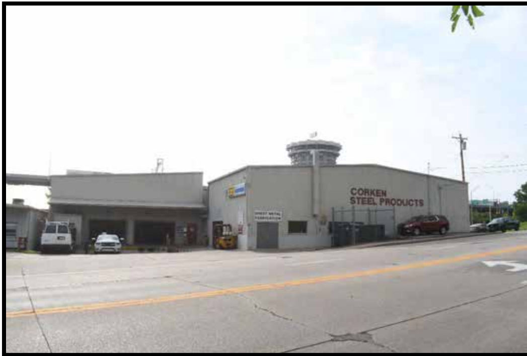
Plate 321. Commercial building, looking southeast.
