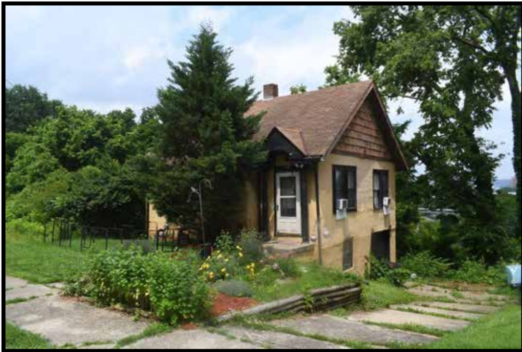
Plate 291. House, looking NE.
