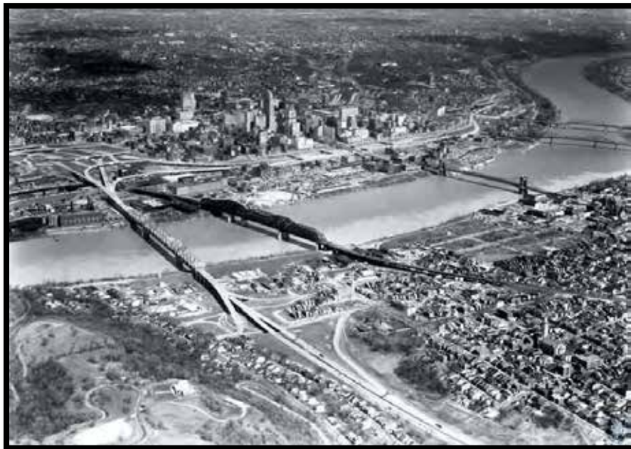
Figure 19. Circa 1964 aerial image of the Brent Spence Bridge and I-75, just after construction concluded. 92
