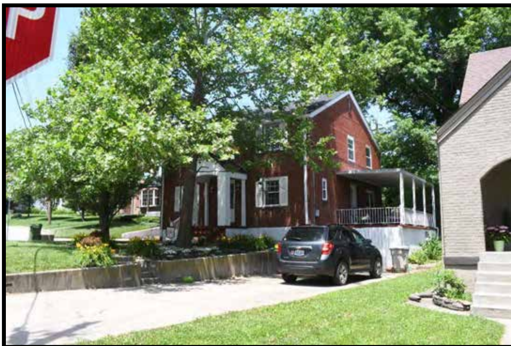
Plate 402. House, looking NE.
