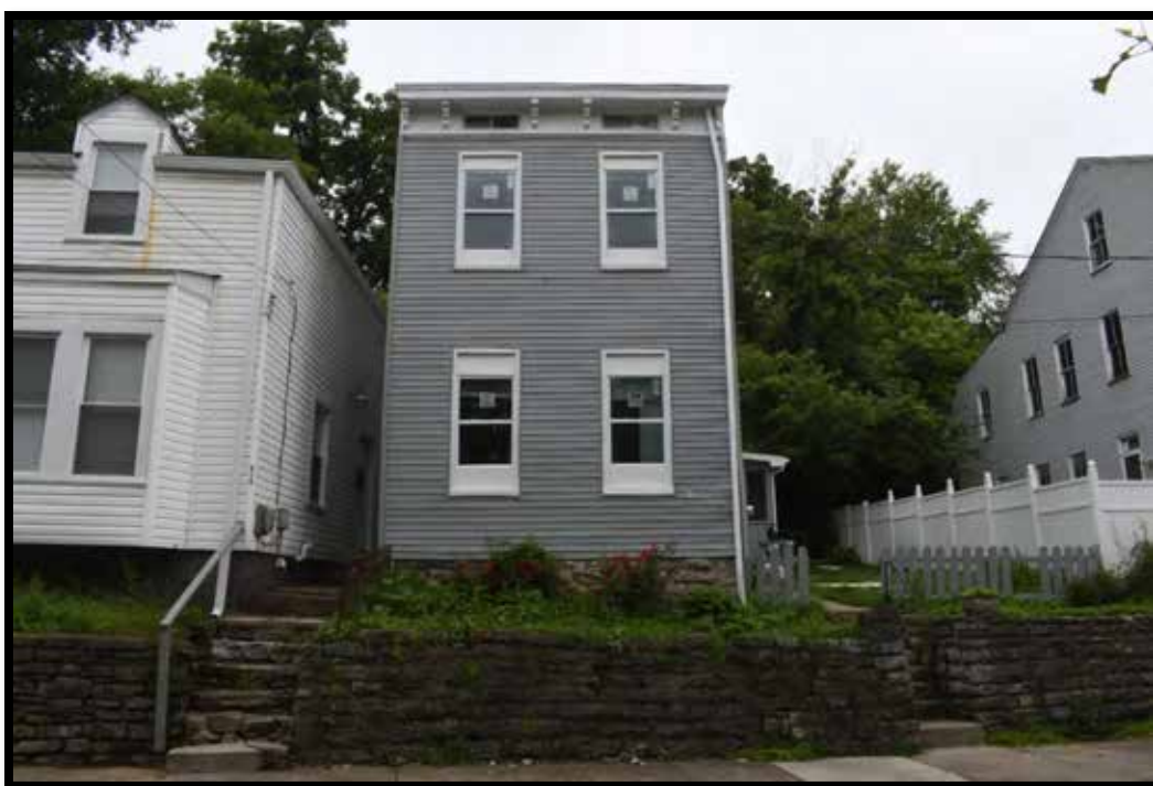
Plate 315. House and retaining wall (B), looking west.
