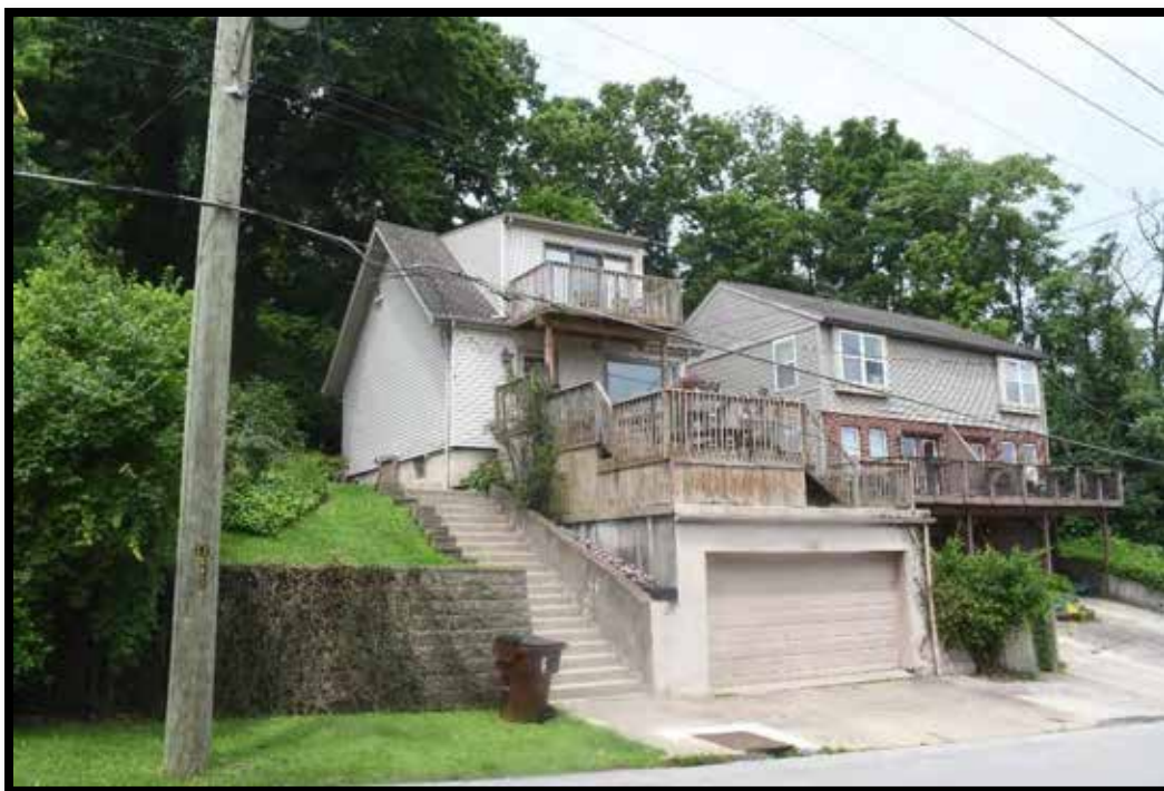
Plate 249. House, looking southwest.
