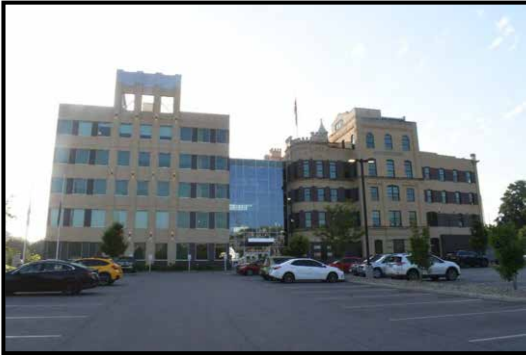
Plate 46. The Bavarian Brewing Co. / Kenton County Government Center, looking south.
