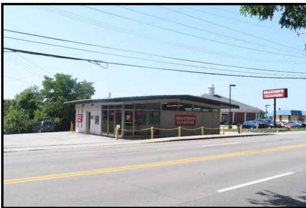
Plate 382. Commercial Building/Braxton's Cleaners, looking south.
