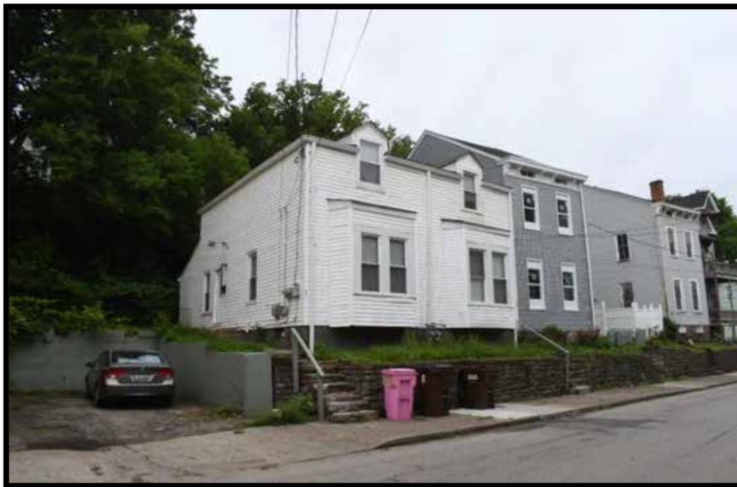
Plate 314. Duplex and retaining wall (B), looking northwest.
