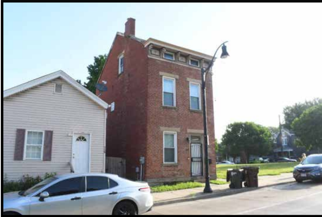
Plate 93. House, looking northeast.
