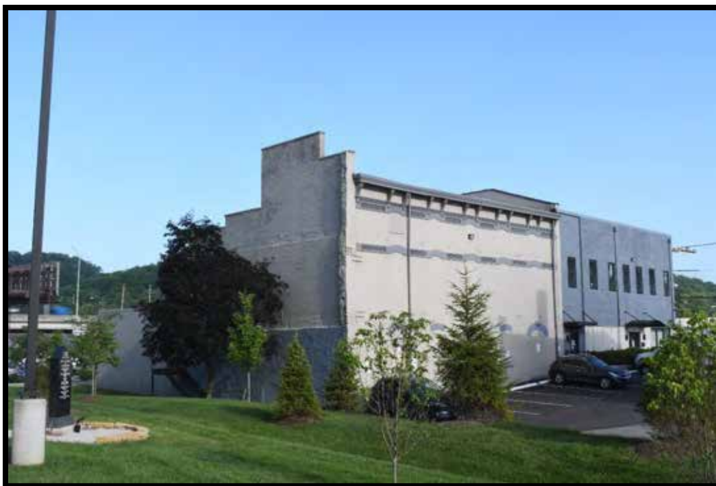
Plate 364. 533 Pike Street, looking northwest.
