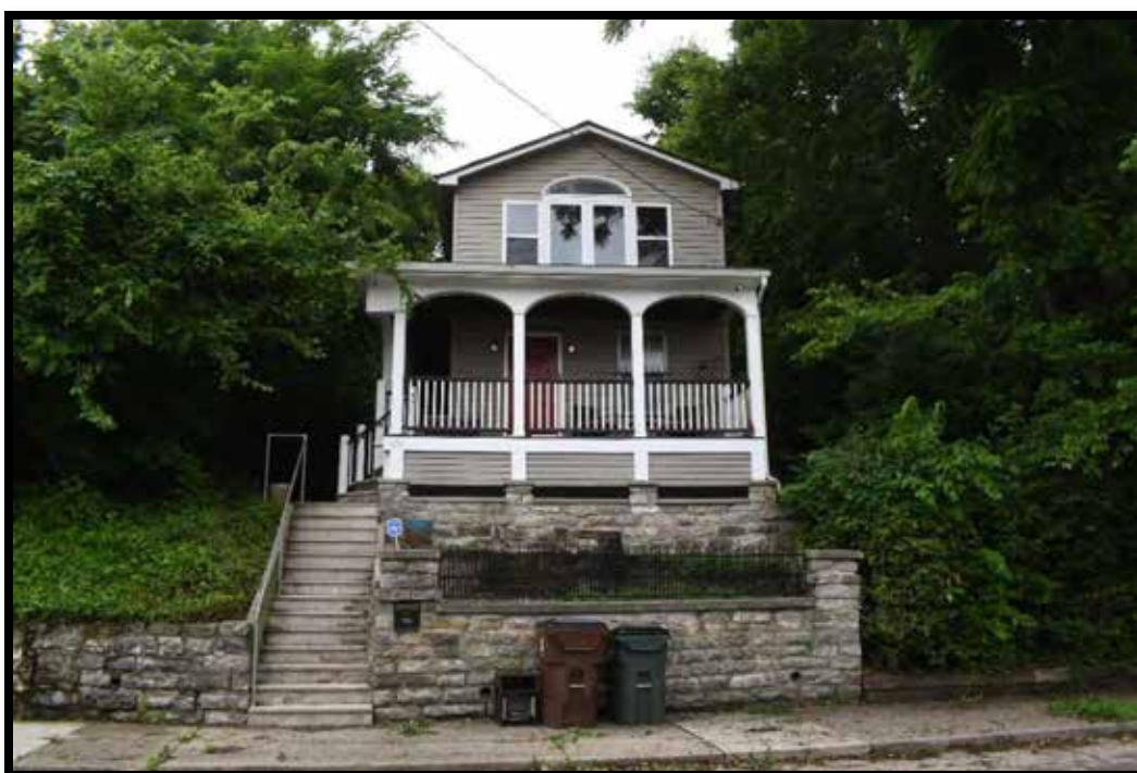
Plate 309. House and retaining wall (B), looking west.
