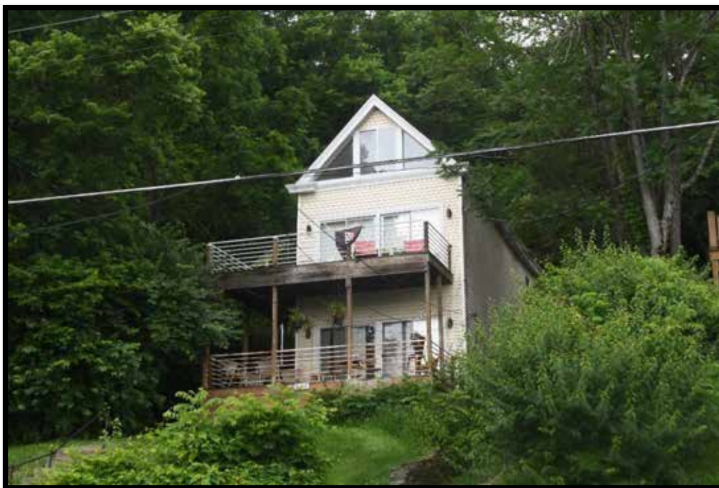
Plate 239. House, looking southwest.
