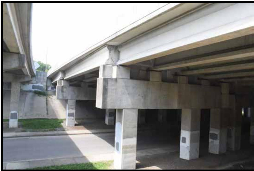
Plate 534. Bridge No. 059B00038L, looking north.
