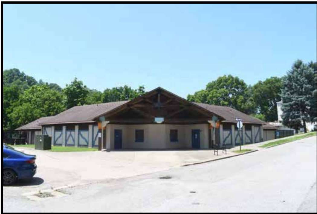
Plate 356. Bathhouse (I), looking northwest.
