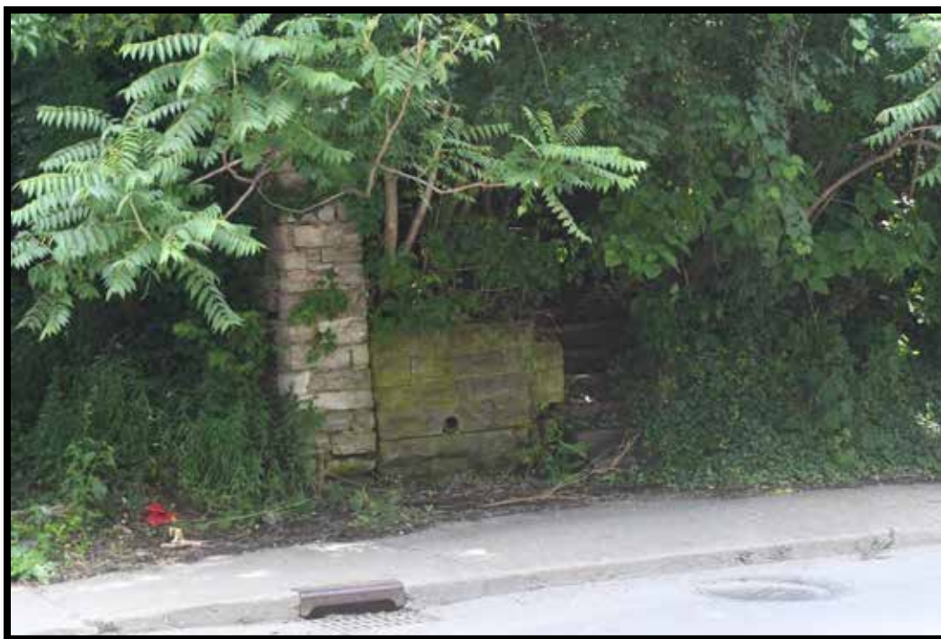
Plate 285. Stone wall, looking SW.
