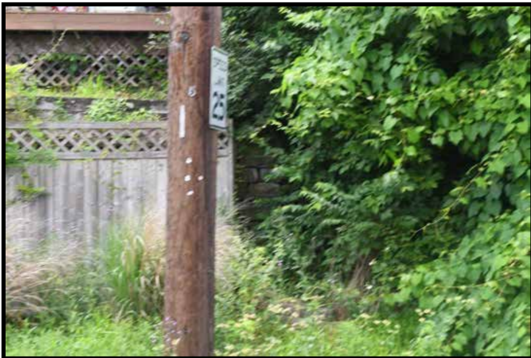
Plate 270. Stone Retention Wall (C), looking west.
