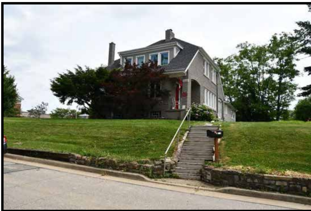
Plate 523. House, looking northeast.
