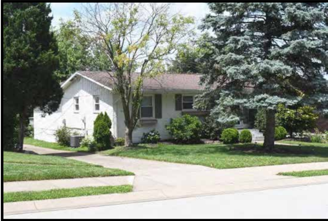
Plate 500. House, looking southwest.
