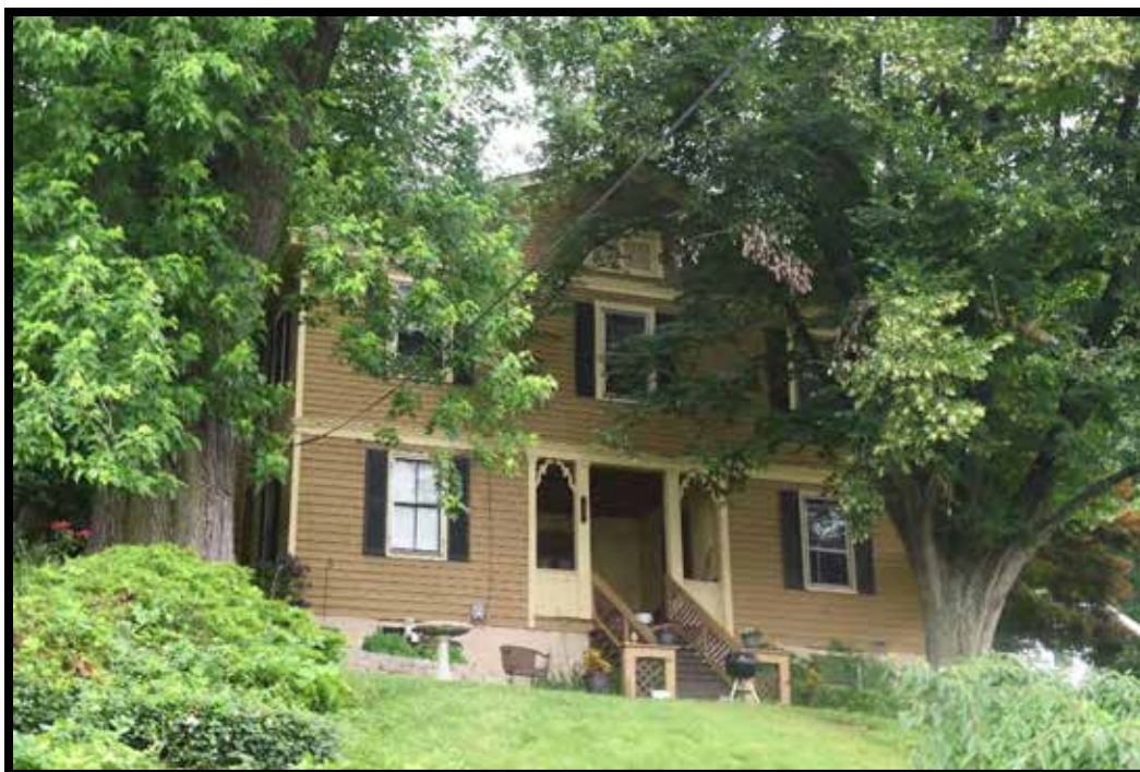
Plate 6. House, looking west.
