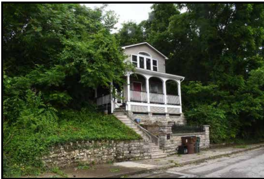
Plate 310. House and retaining wall (B), looking northwest.
