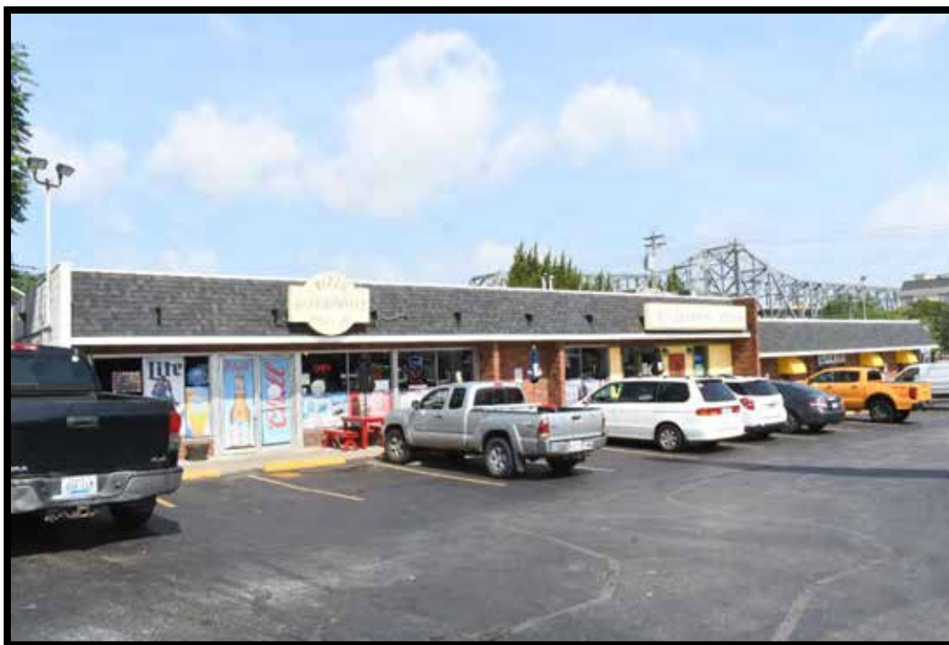
Plate 339. Commercial building, looking northeast.
