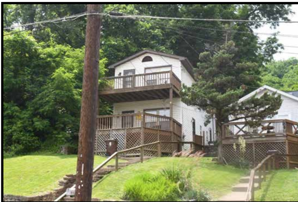
Plate 271. House, looking SW.
