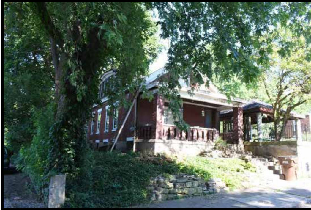
Plate 125. House and stone wall (B), looking northwest.
