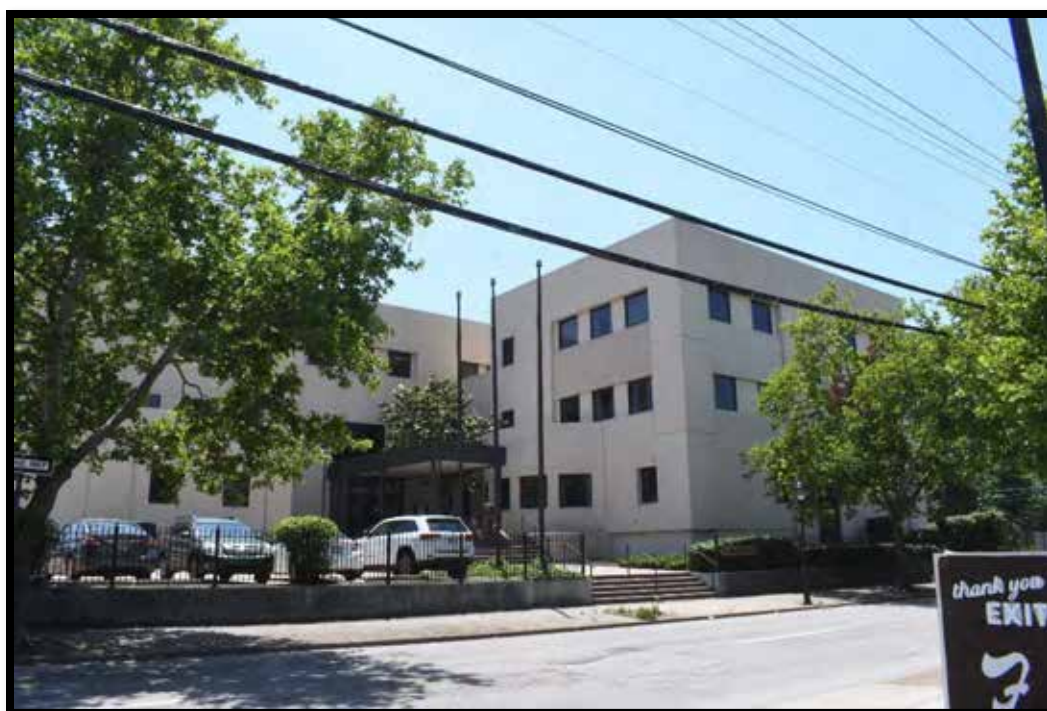
Plate 357. Fifth Street Center Office Building and Fence (B), looking southwest.
