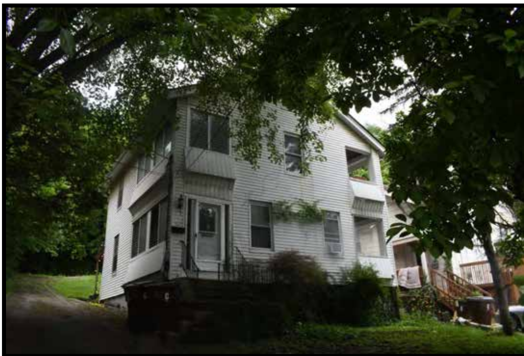
Plate 225. House, looking west.
