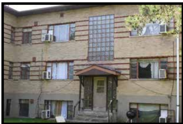
Plate 168. Left, St. Joseph Lane, Original Glass Block Sidelights, Multi-Story Glass Block Stairwell Window, and Steel Casement Windows; Right, Elberta Circle, Original Metal Front Canopy and Lighting
