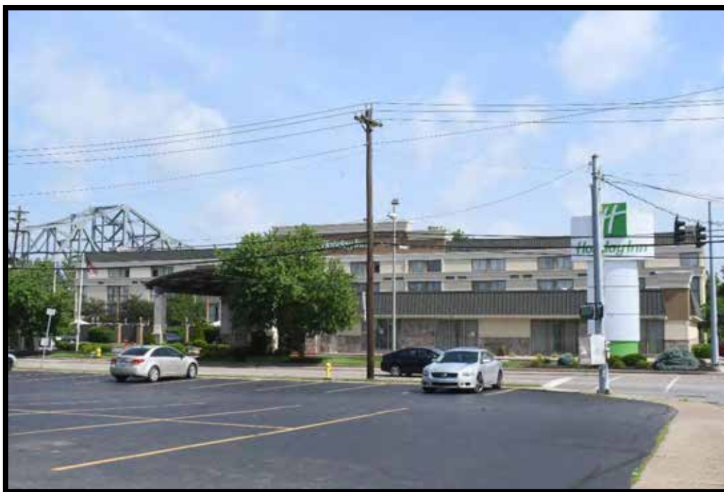
Plate 334. Commercial building, Holiday Inn Cincinnati-Riverfront, looking northwest.
