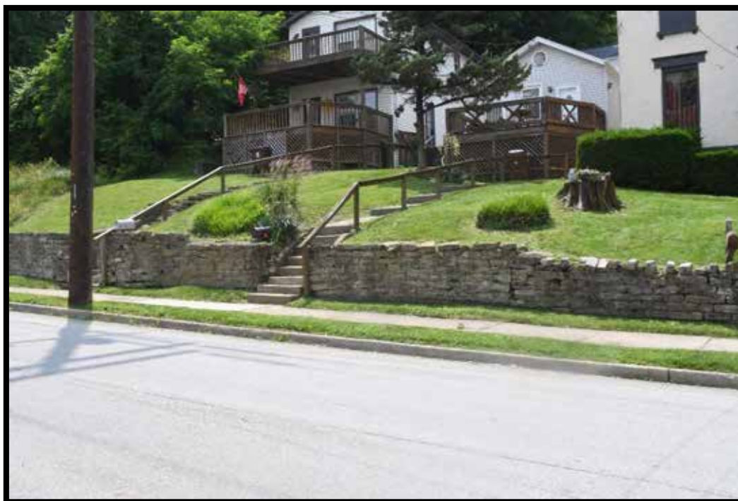
Plate 275. Stone retaining wall (B), looking SW.
