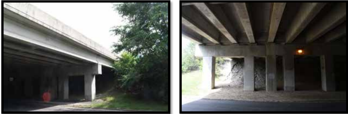
Plate 546. Bridge No. 059B00043L. Left: Bridge, looking north. Right: View of substructure.
