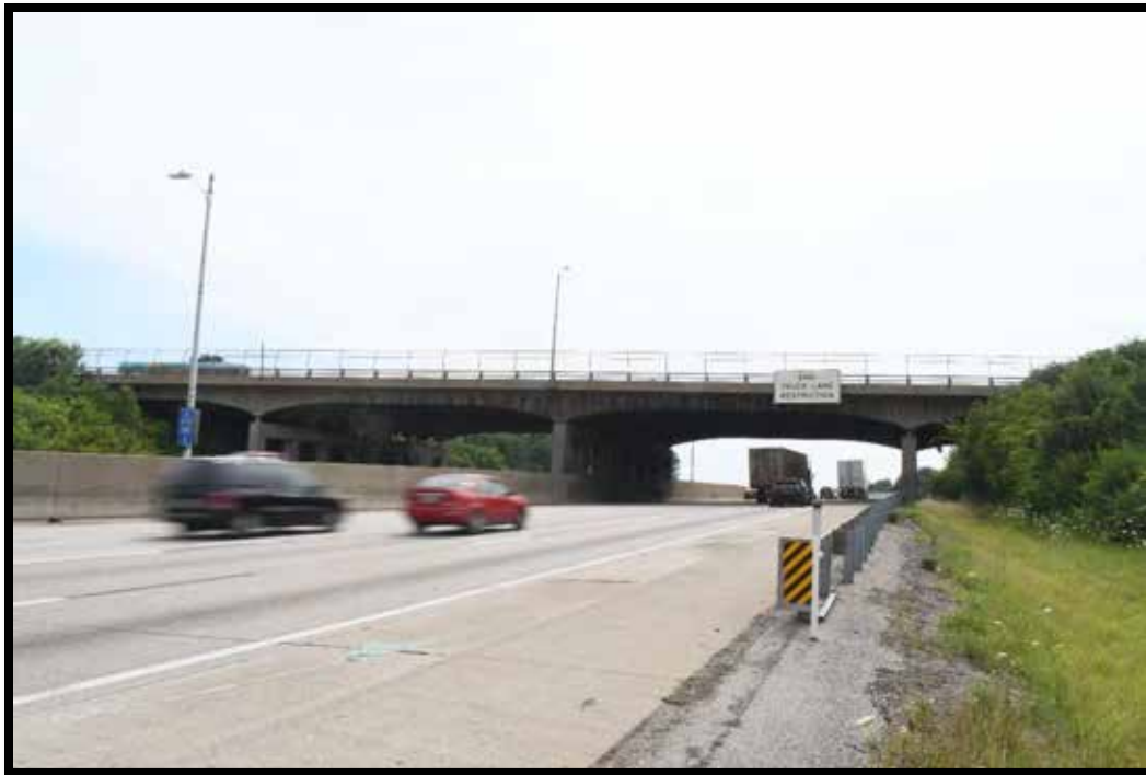
Plate 541. Bridge No 059B00047N, looking southwest.
