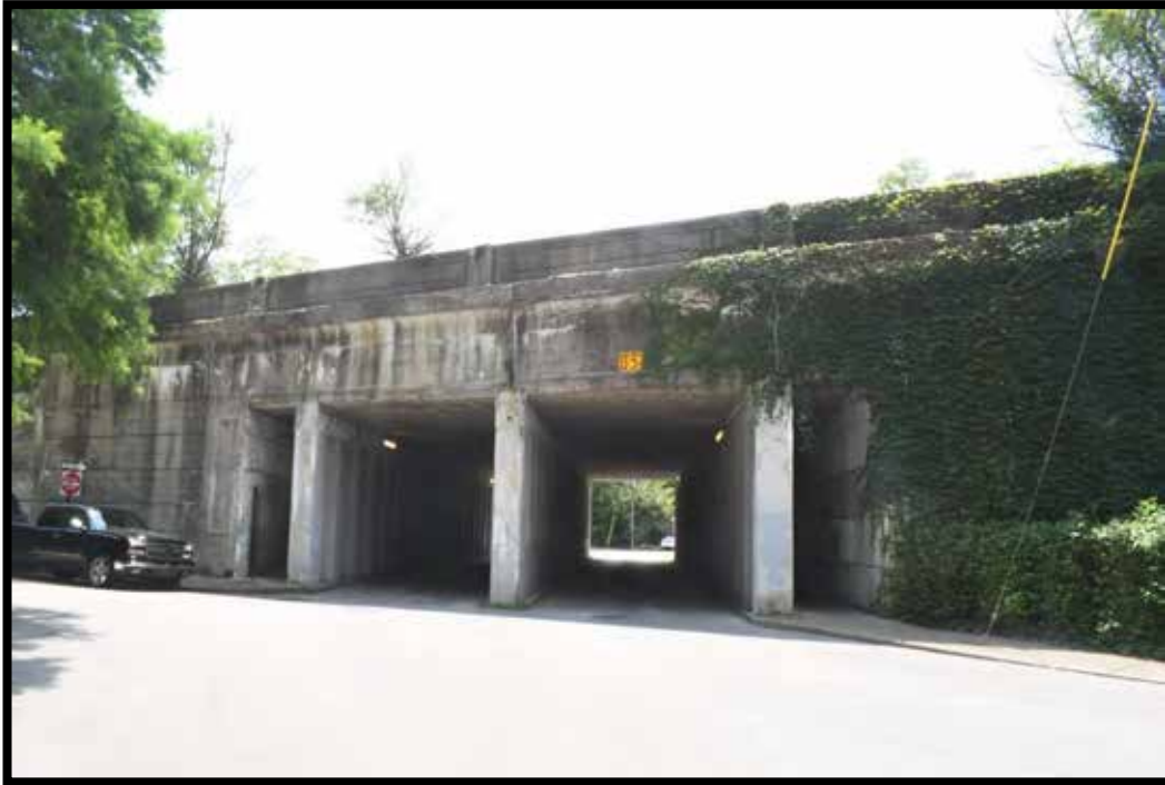
Plate 104. CSX Railroad Bridge No. 059R00627N, looking SW.
