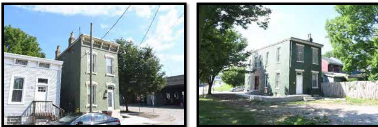
Plate 154. Left: House, looking southwest. Right: Rear of house, looking northwest.
