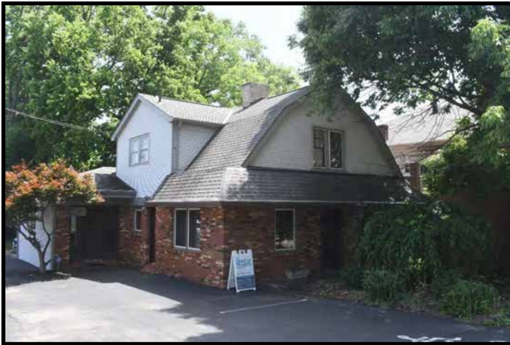
Plate 413. Office Building, looking south.
