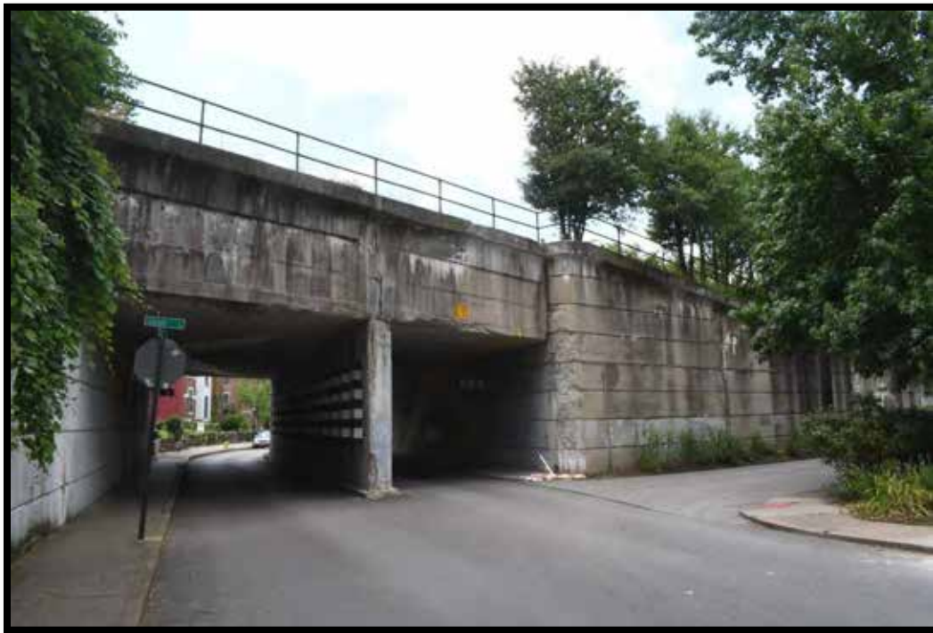
Plate 97. CSX Railroad Bridge No. 059R00622N, looking west.
