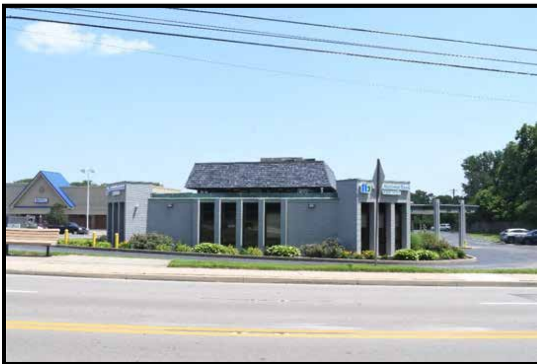
Plate 415. First National Bank Kentucky, looking southeast.
