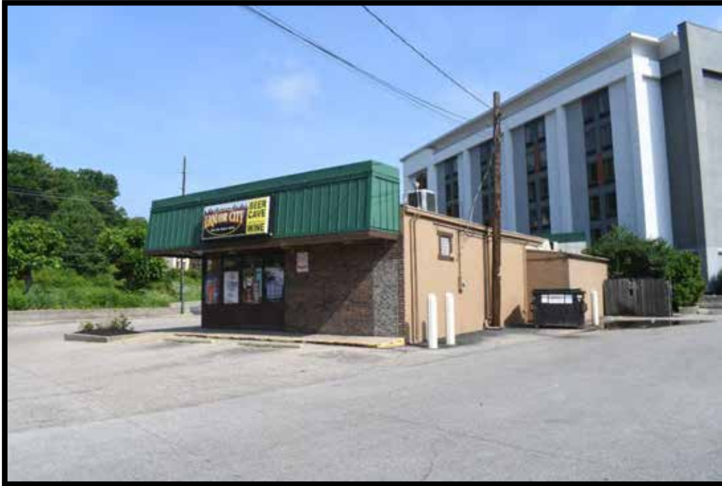
Plate 330. Rear of Commercial building, looking northeast.
