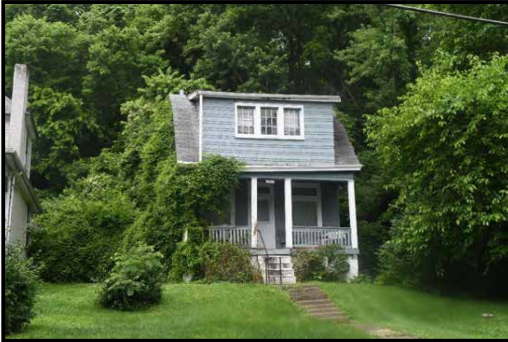
Plate 234. House, looking west.
