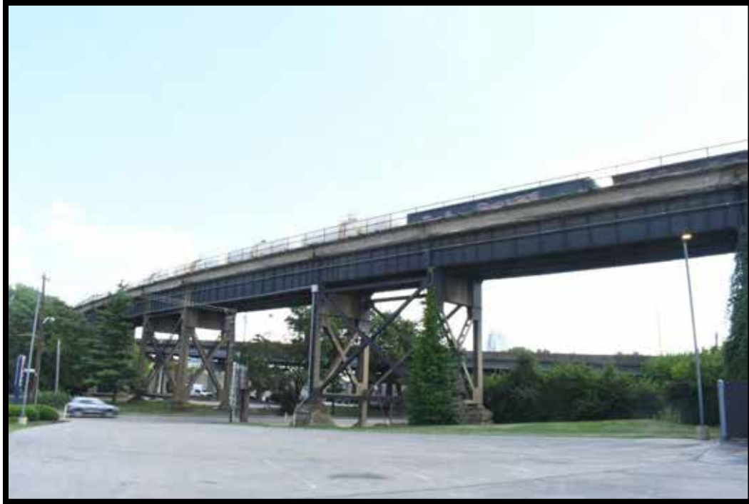
Plate 23. CSX Railroad Bridge No. 059R0062N (KEC-1063), looking east.
