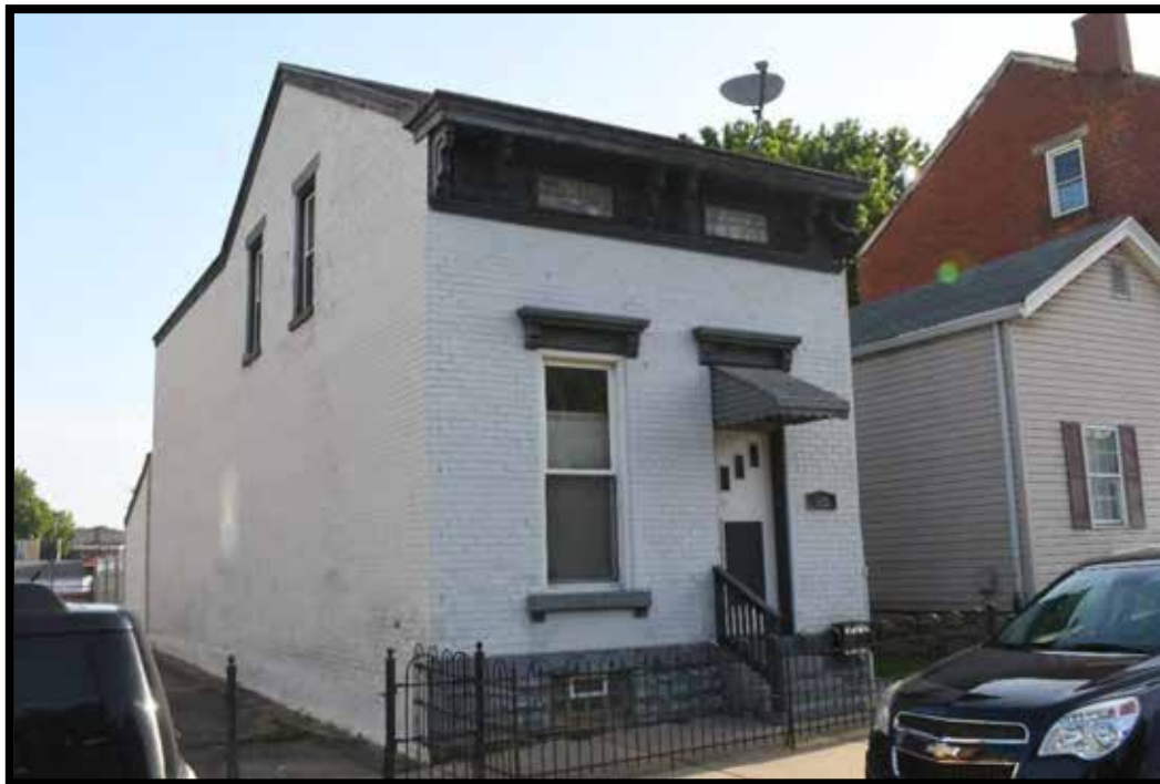
Plate 88. House and Fence (B), looking northeast.
