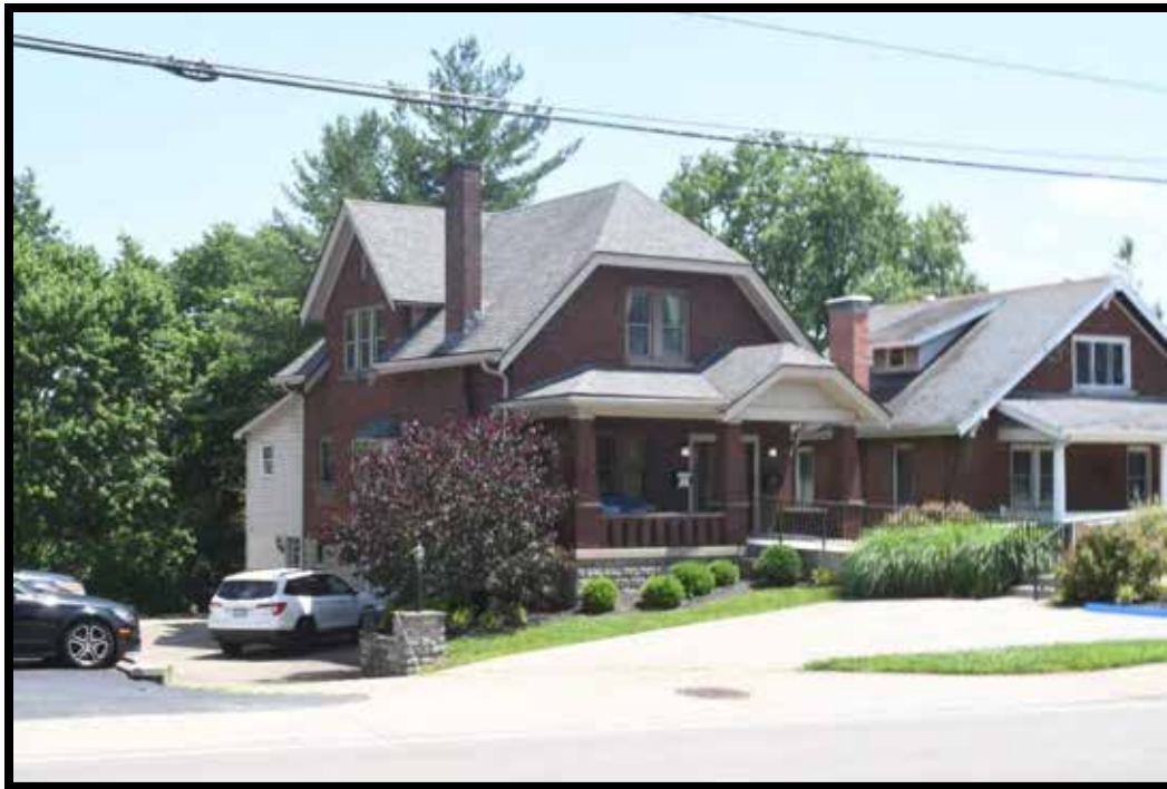
Plate 431. Office building, looking south.
