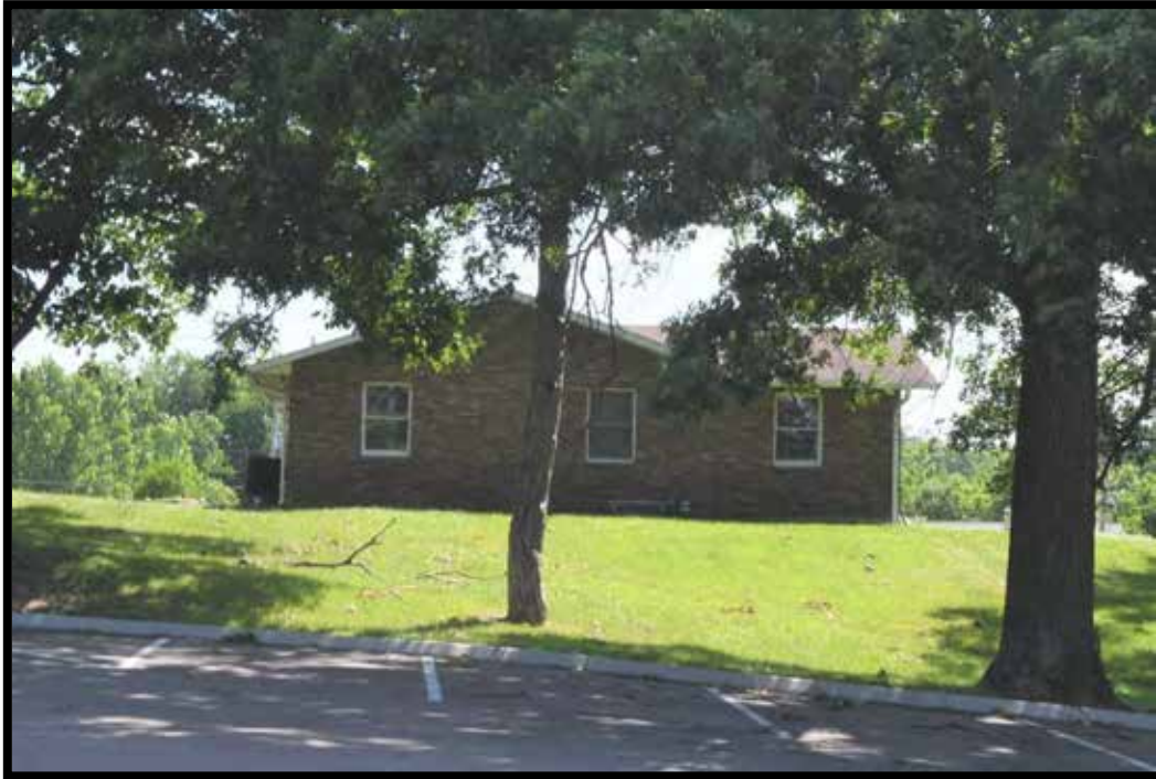
Plate 489. House, looking northeast.
