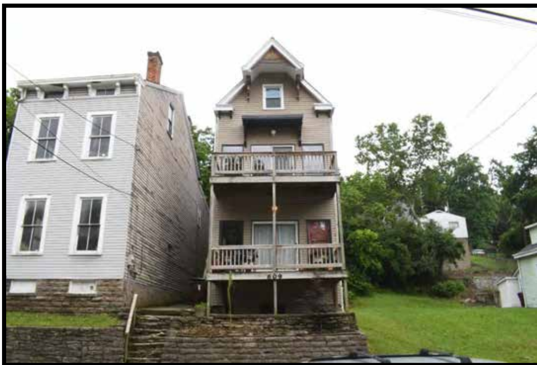
Plate 317. House and retaining wall (B), looking west.
