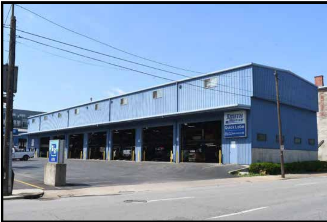
Plate 344. Commercial building. B, Garage/workshop, looking southwest.
