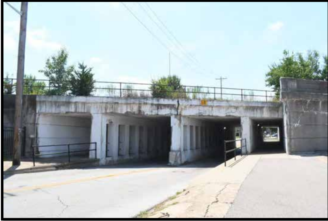
Plate 114. CSX Railroad Bridge No. 059R00621N, looking west.
