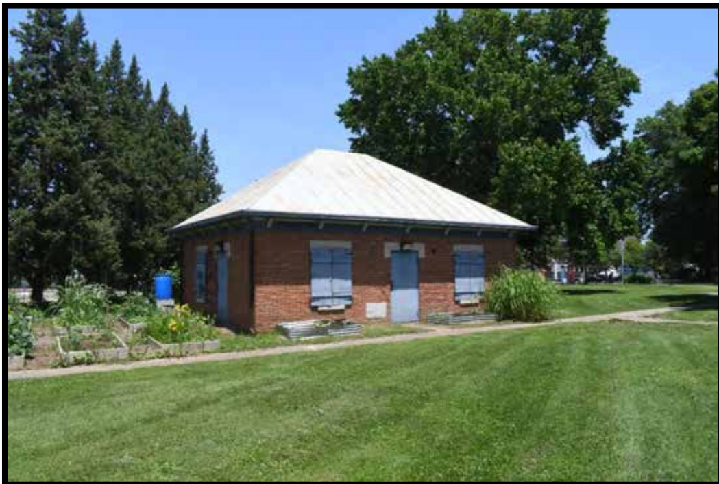
Plate 352. Outbuilding (E), looking northeast.
