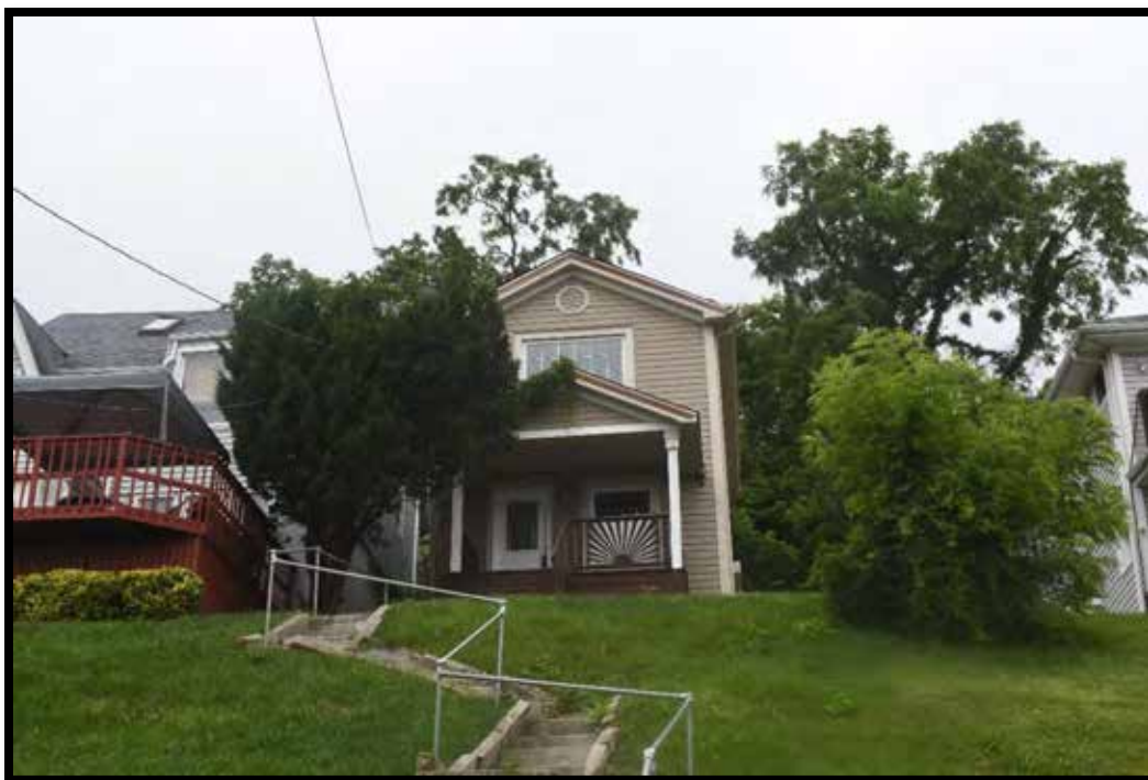
Plate 261. House, looking west.
