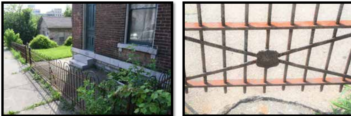
Plate 150. Left: Fence, looking southeast. Left: Stewart Iron Works Company badge on gate.
