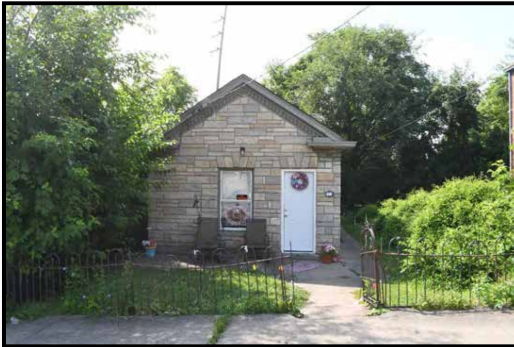
Plate 151. House, looking southwest.
