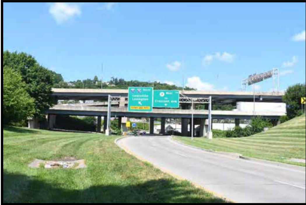
Plate 526. Bridge No. 059B00040N. Fourth Street overpass of Third, Fourth, and Fifth Street's approach of I-75/71 to Brent Spence Bridge (Bridge No. 059B00046N), looking west.
