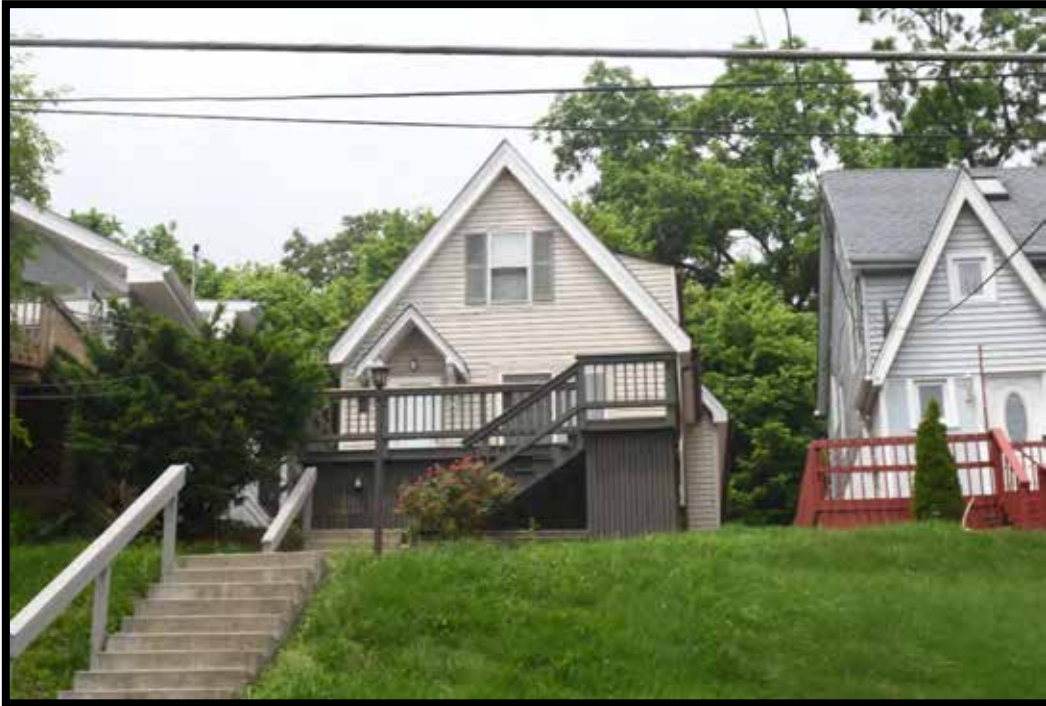
Plate 258. House, looking west.
