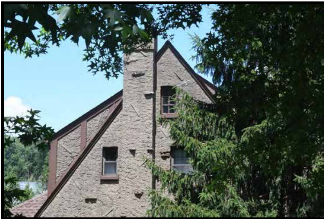
Plate 58. House, detail of stucco, ledges, and half-timbered detailing.
