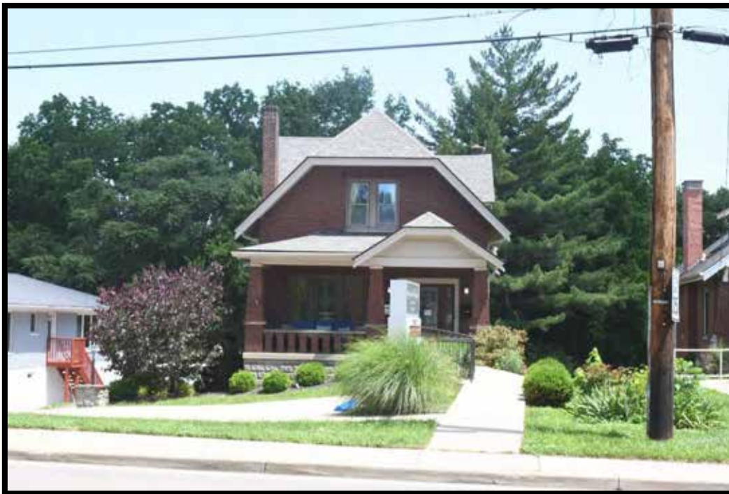
Plate 432. Office building, façade, looking southeast.
