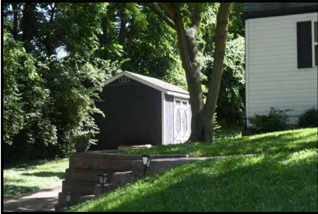
Plate 469. Storage shed (B), looking northeast.
