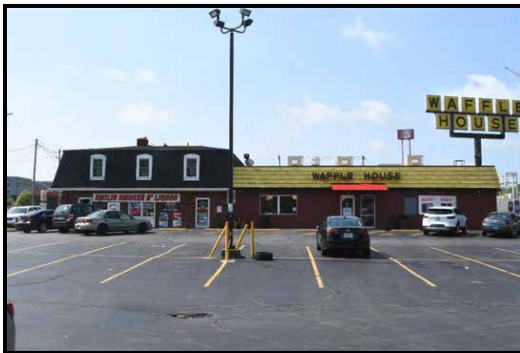
Plate 338. Commercial building, looking south.
