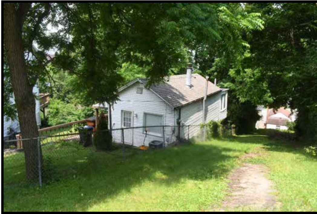
Plate 304. House, looking northeast.
