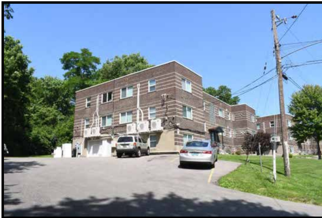
Plate 178. Apartment Building, looking north.
