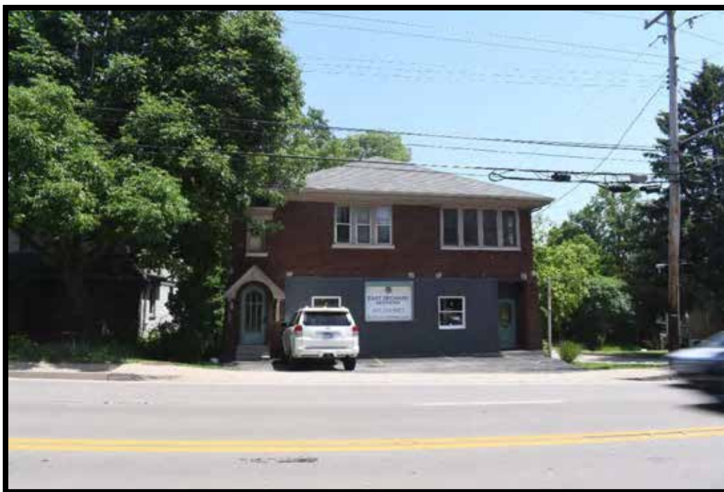
Plate 411. Office Building, looking southeast.
