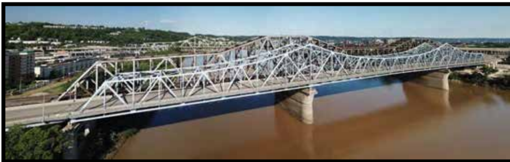
Figure 62. Clay Wade Bailey Bridge with 1929 C & O Railroad Bridge in background, 2018 255
