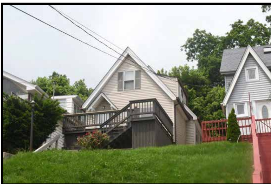
Plate 257. House, looking SW.
