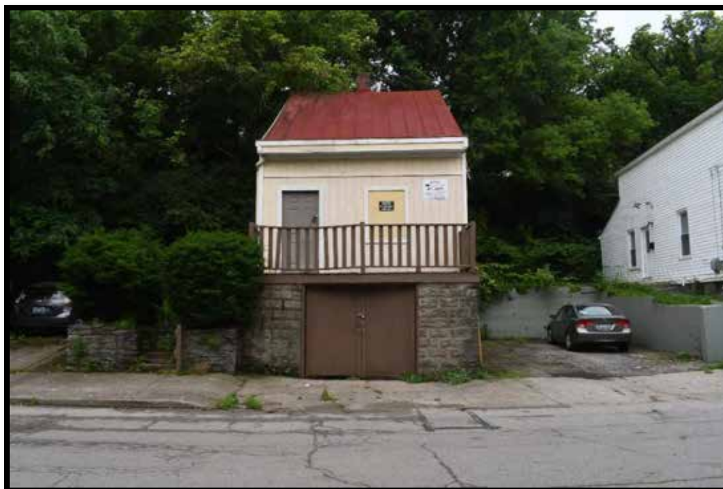
Plate 311. House and retaining wall (B), looking northwest.
