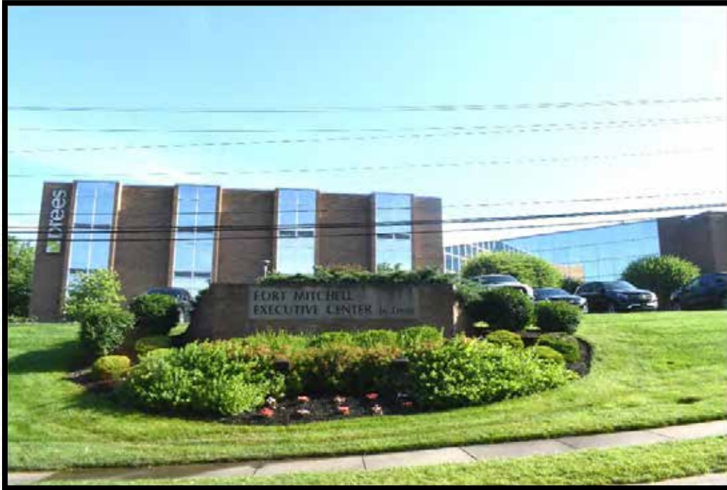
Plate 445. Fort Mitchell Executive Center business sign (C), looking north.
