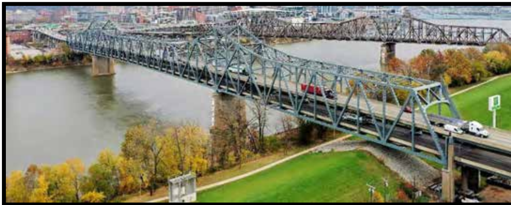
Plate 40. Brent Spence Bridge, looking NE.
