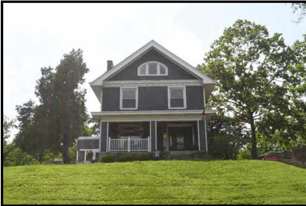
Plate 61. House, looking west.
