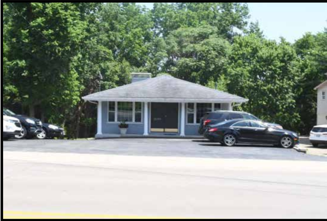
Plate 430. Office building, looking southeast.
