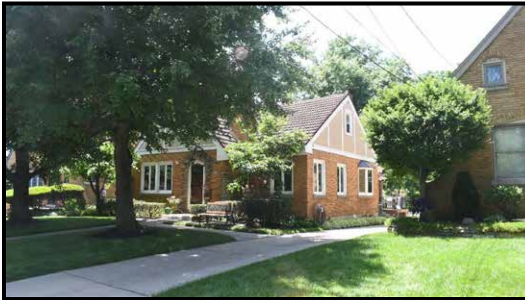
Plate 390. House, looking southwest.
