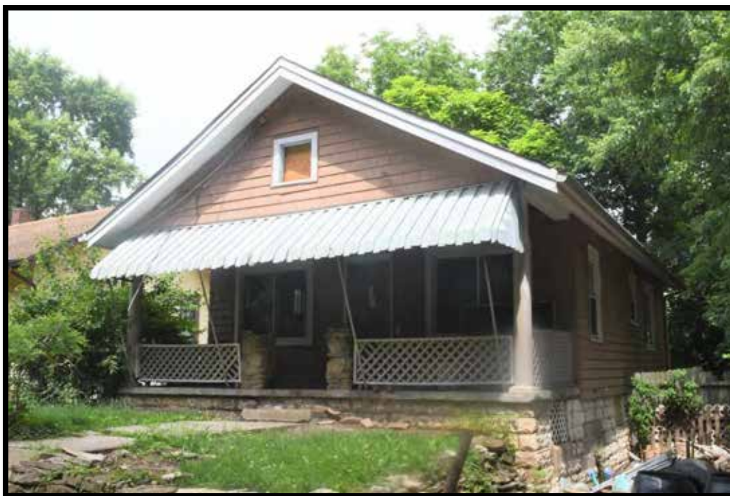
Plate 286. House, looking NE.
