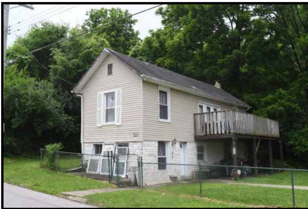
Plate 265. House, looking SW.
