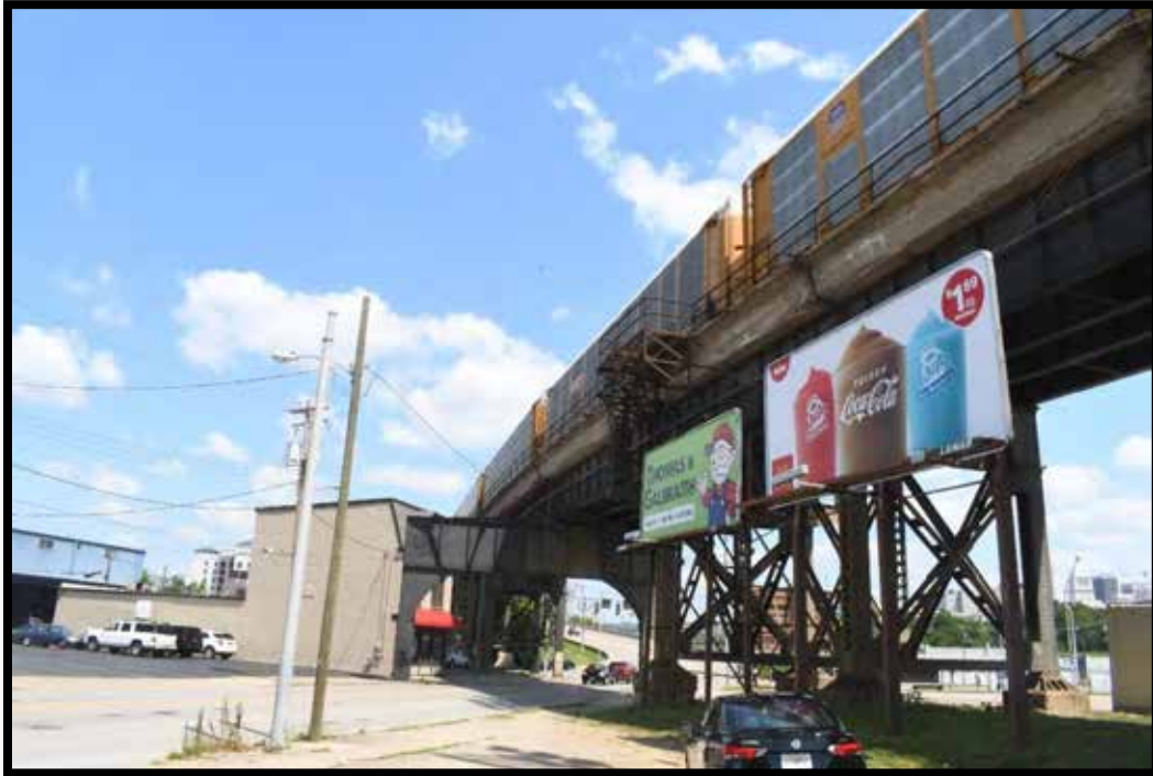
Plate 27. CSX Railroad Bridge No. 059R00610N (KEC-1065), looking north.
