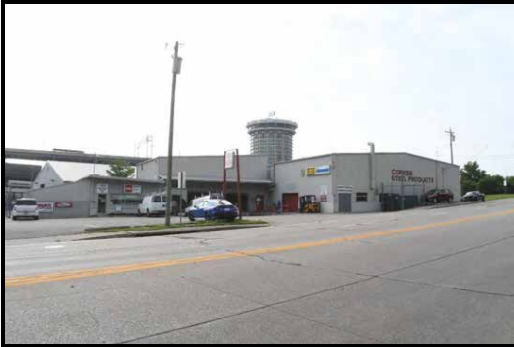
Plate 322. Commercial building, looking southeast.
