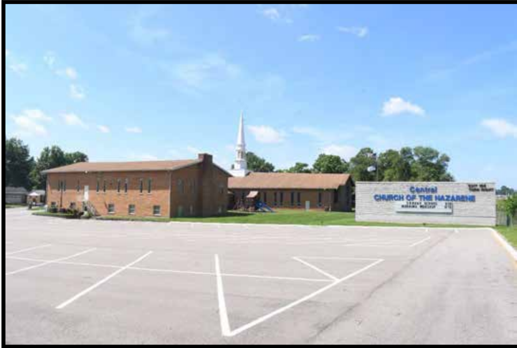
Plate 480. Church and storage building/Interstate sign (E), looking southwest.
