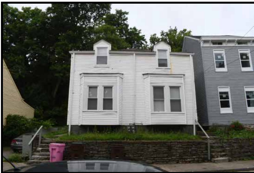
Plate 313. Duplex and retaining wall (B), looking west.
