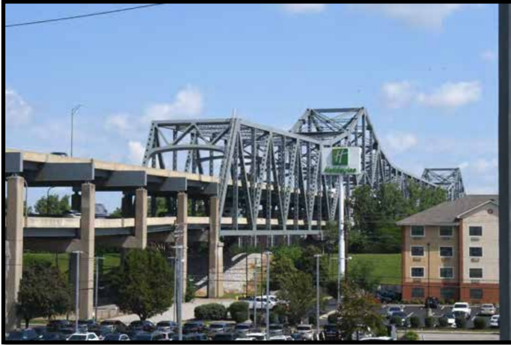
Plate 37. Brent Spence Bridge, looking north.
