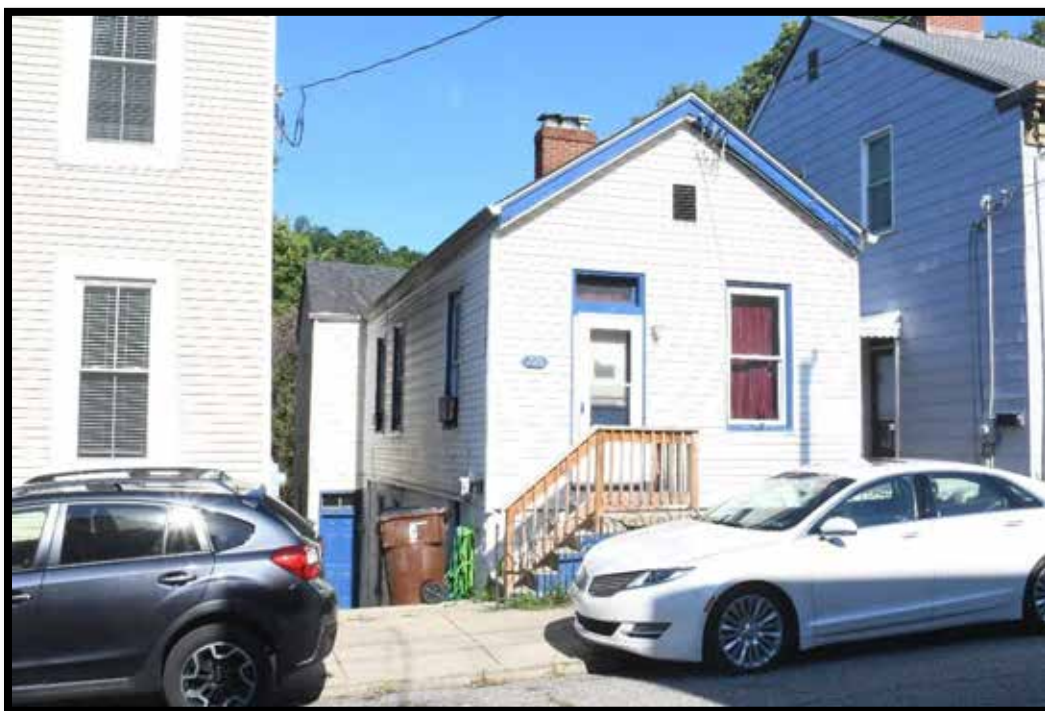
Plate 117. House, looking northeast.
