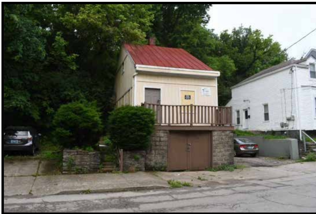
Plate 312. House and retaining wall (B), looking southwest.
