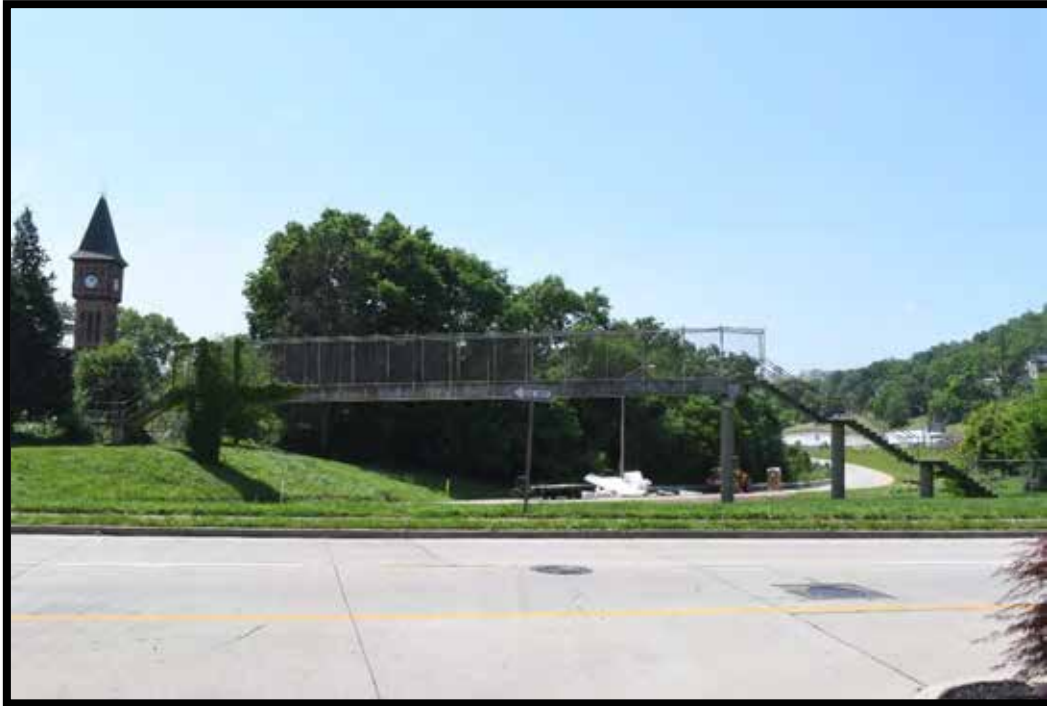
Plate 348. Bridge No. 059B00041N, looking south.
