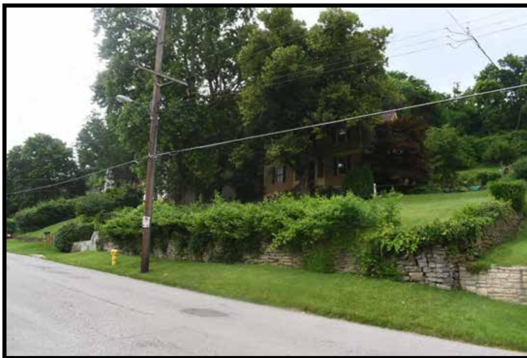
Plate 7. Dry-stone retaining wall, looking southwest.
