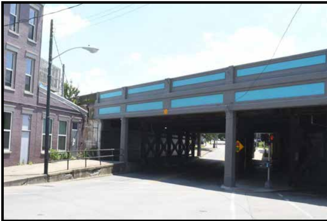
Plate 110. CSX Railroad Bridge No. 059R00620N, looking south.
