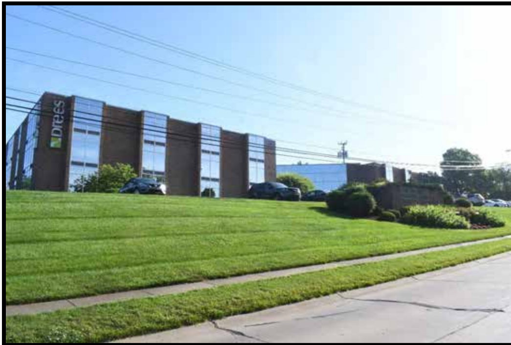
Plate 441. Drees Fort Mitchell Executive Center, façade, looking northeast.
