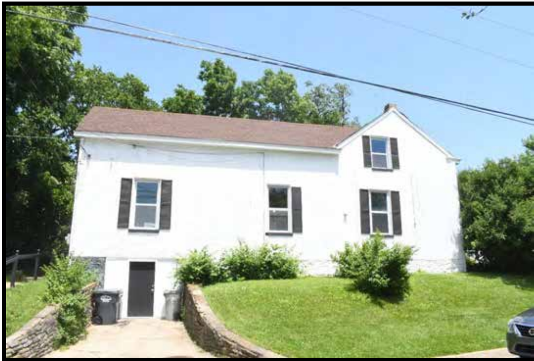
Plate 408. House, looking northeast.
