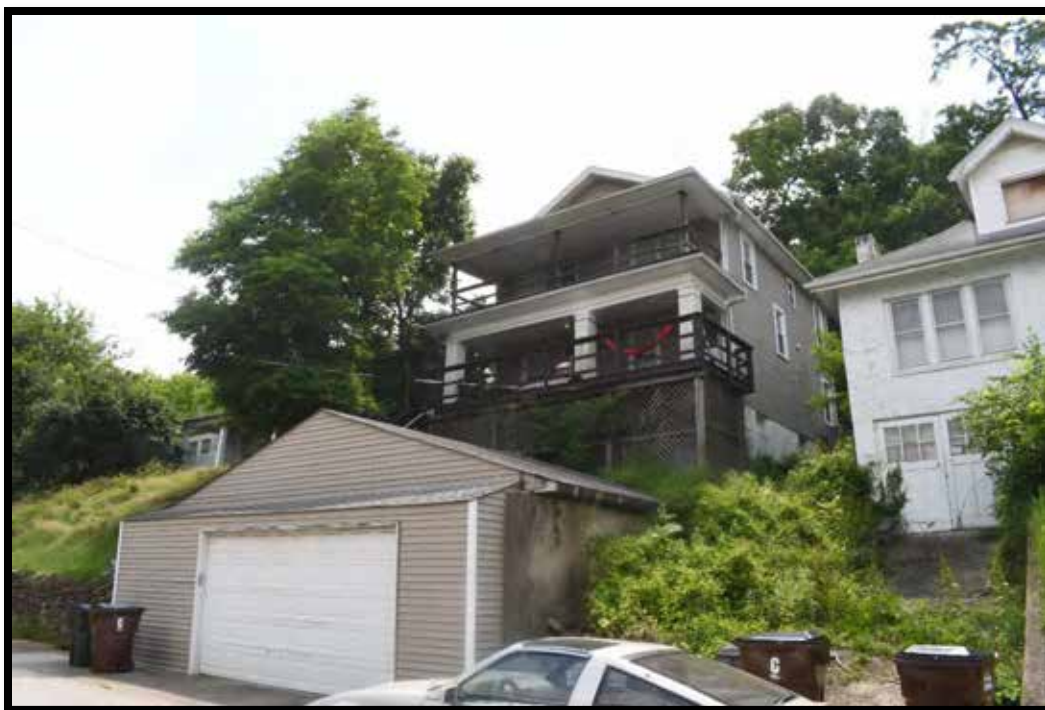
Plate 295. House and garage (B), looking SW.
