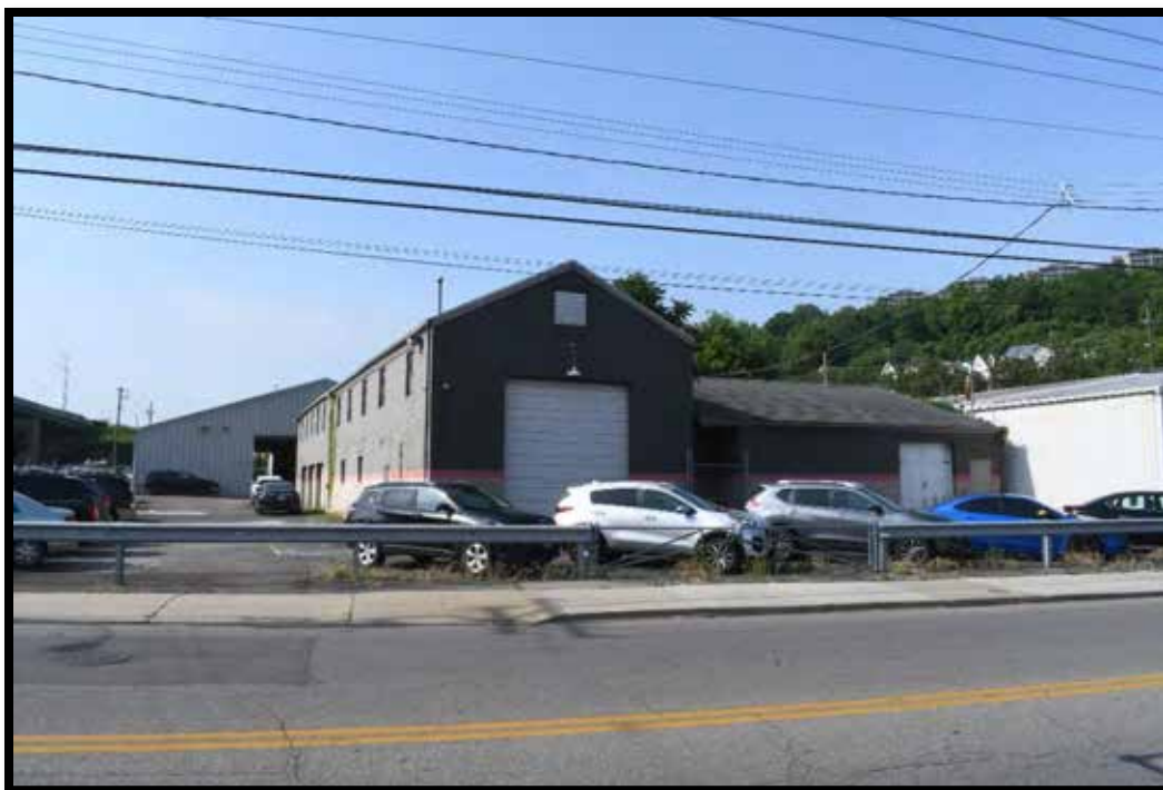
Plate 328. Garage/Workshop, looking southwest.
