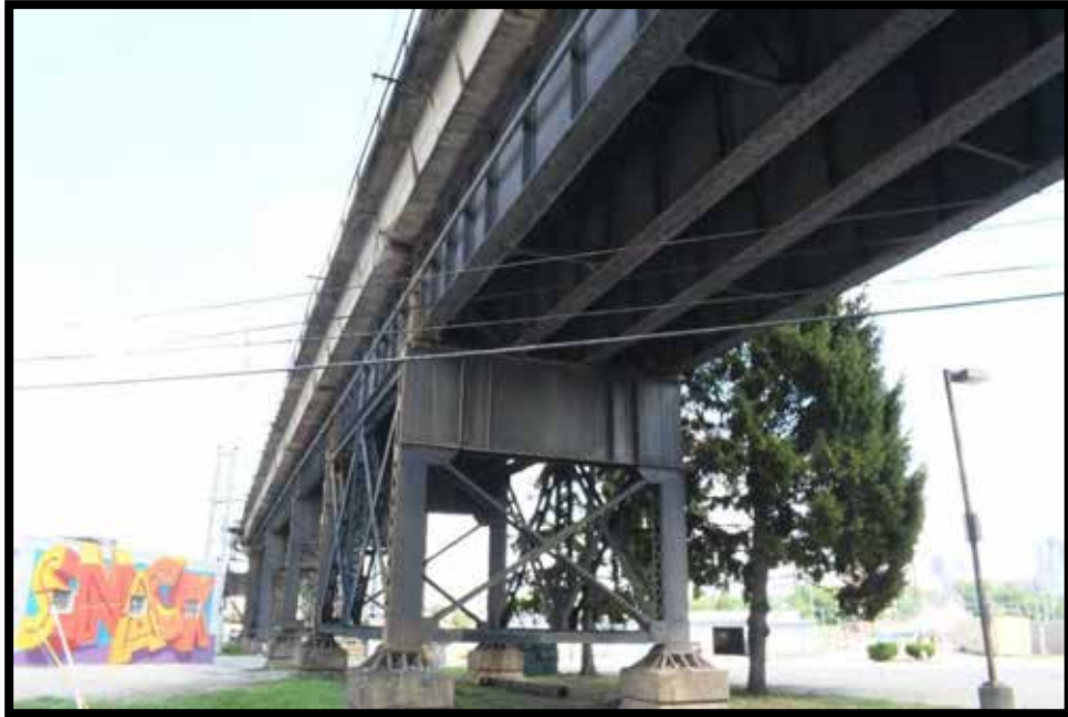
Plate 29. CSX Railroad Bridge No. 059R00610N (KEC-1065). Steel support truss and girders looking north.
