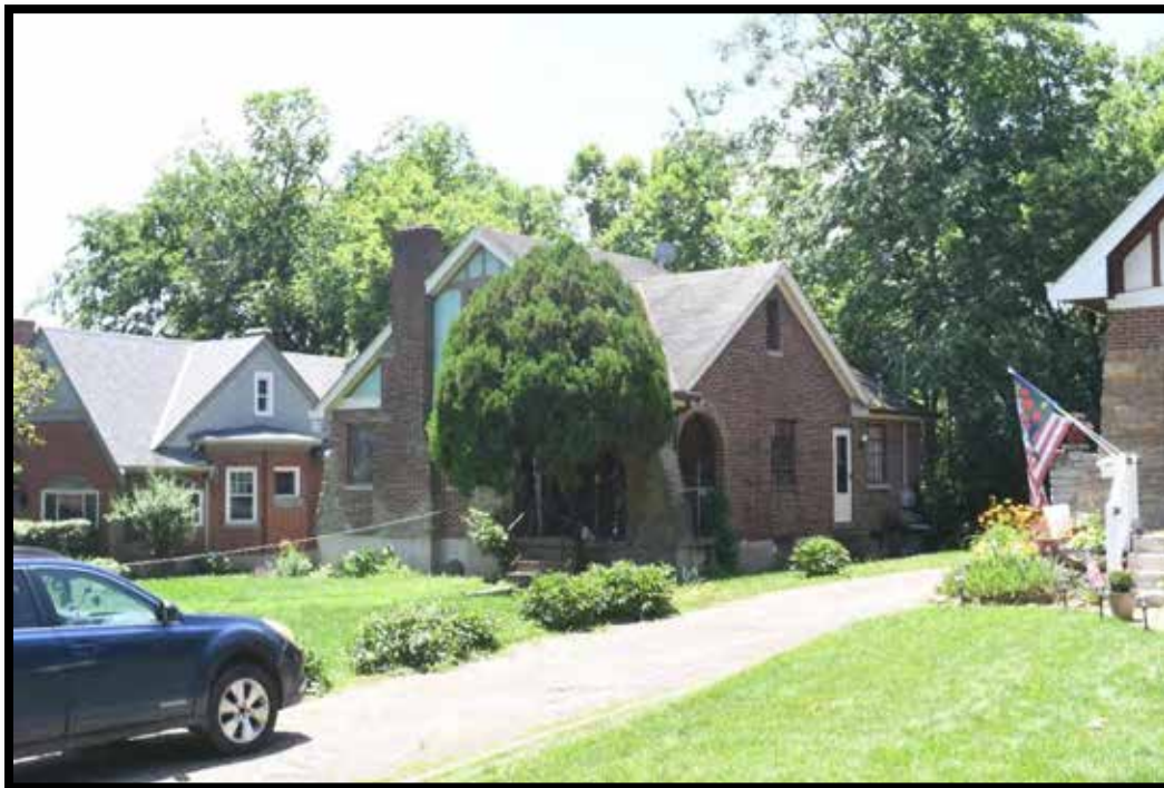
Plate 206. House, looking southwest.
