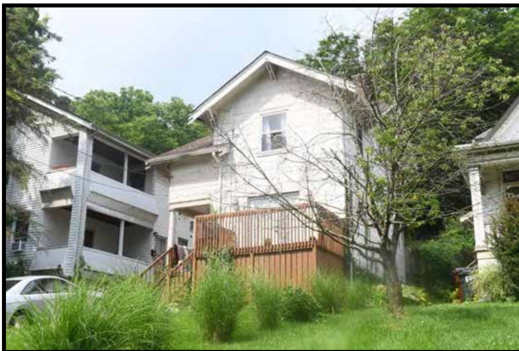
Plate 227. House, looking west.
