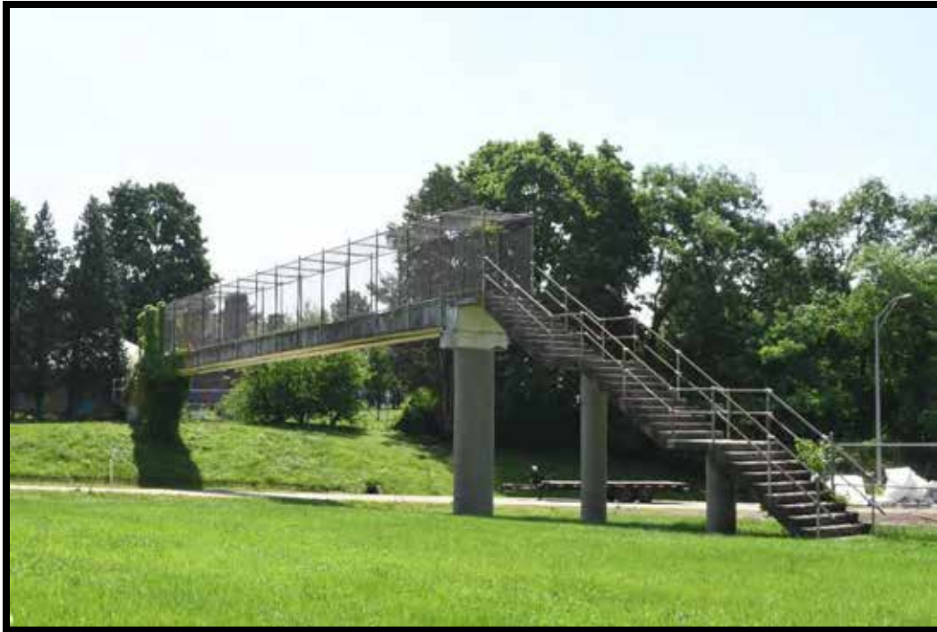
Plate 347. Bridge No. 059B00041N, looking northwest.
