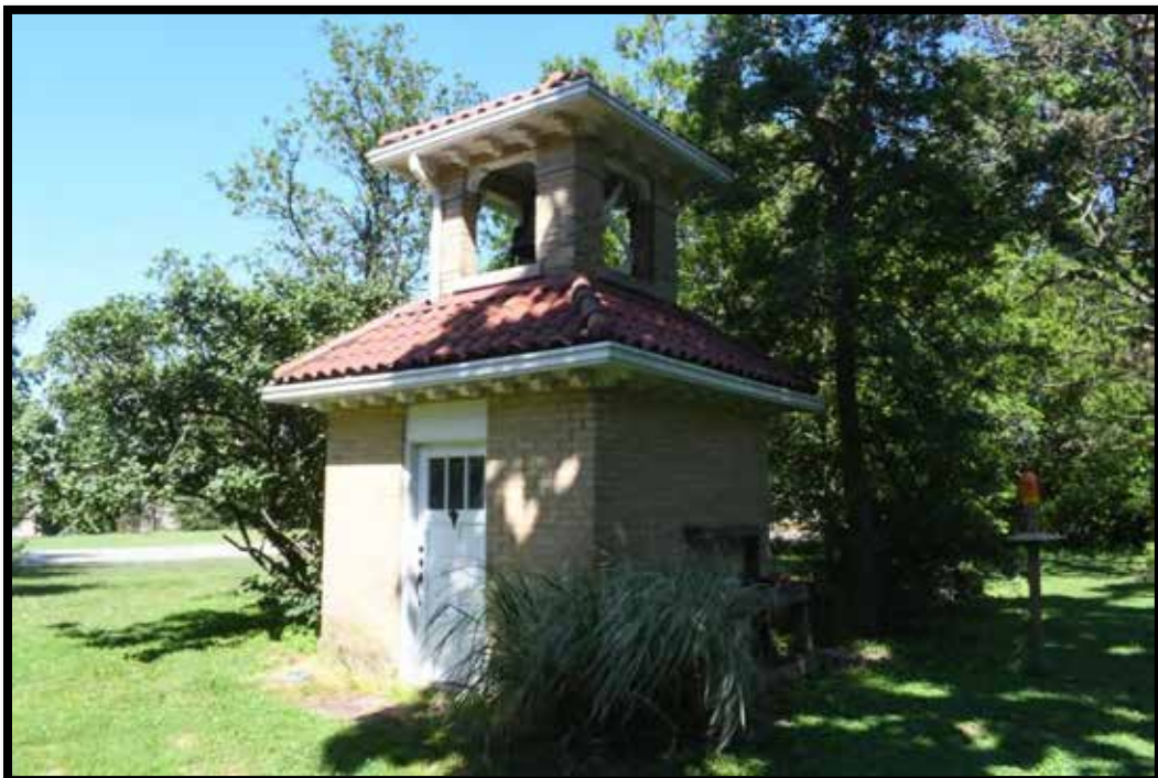
Plate 186. Highland Cemetery. Bell tower (D), looking NE.
