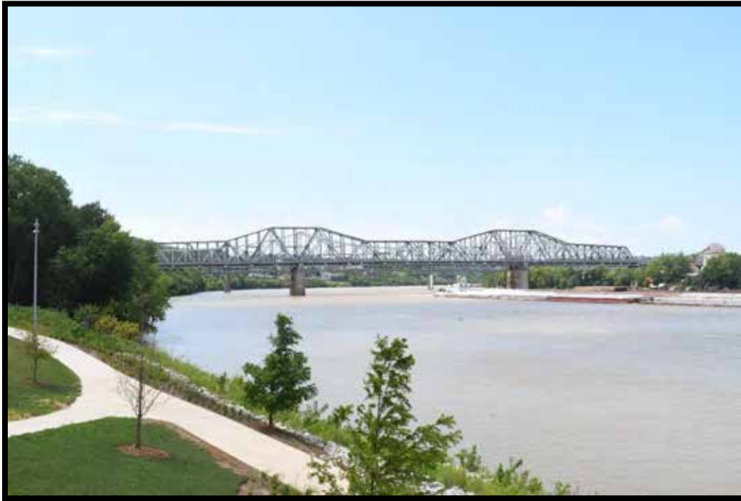
Plate 80. Clay Wade Bailey Bridge with 1929 C & O Railroad Bridge in background, looking west
