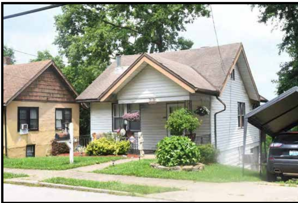
Plate 289. House, looking NE.
