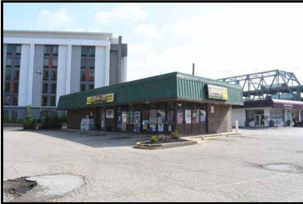
Plate 329. Commercial building, looking northeast.
