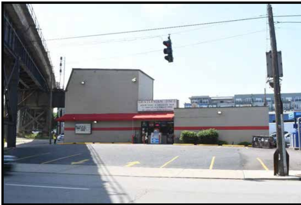
Plate 342. Commercial building, looking south.
