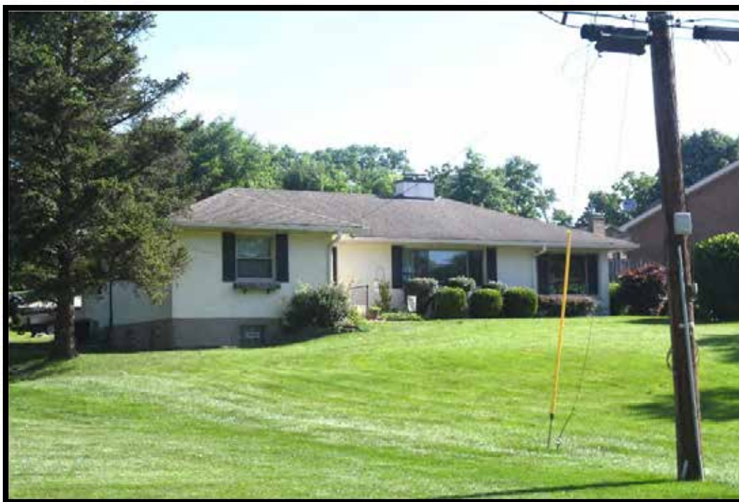
Plate 446. House, looking northeast.
