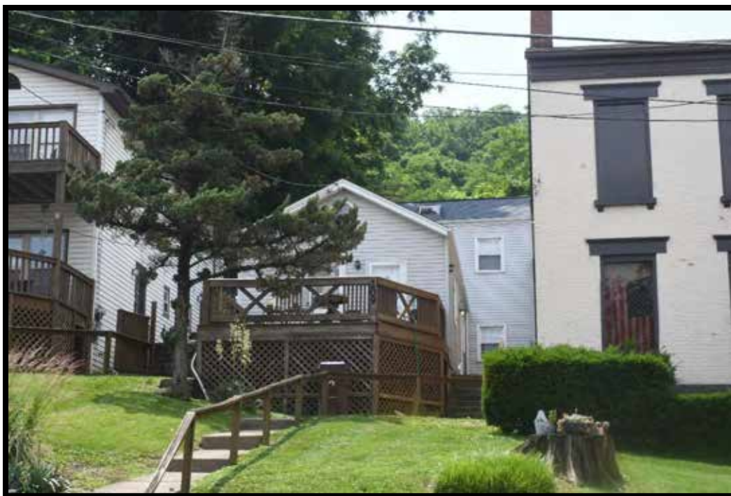
Plate 274. House, looking west.
