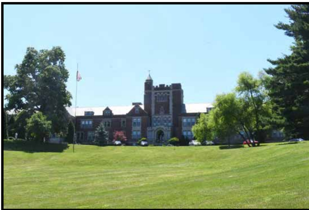
Plate 63. Sisters of Notre Dame Provincial House and Convent, looking SW.
