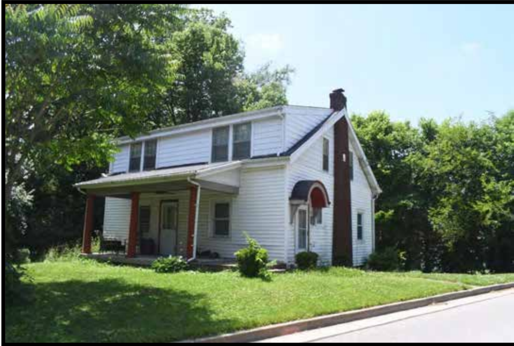
Plate 407. House, looking west.
