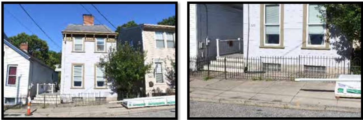
Plate 120. Left: House, looking west. Right: Fence (B), looking west.
