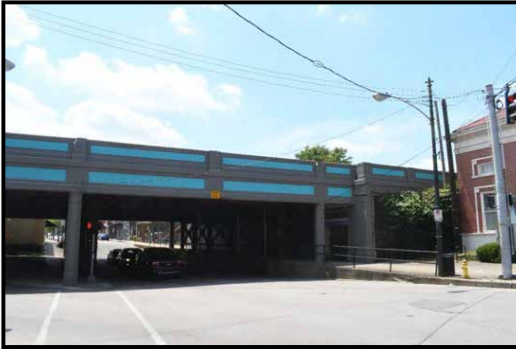
Plate 106. CSX Railroad Bridge No. 059R00617N, looking south.
