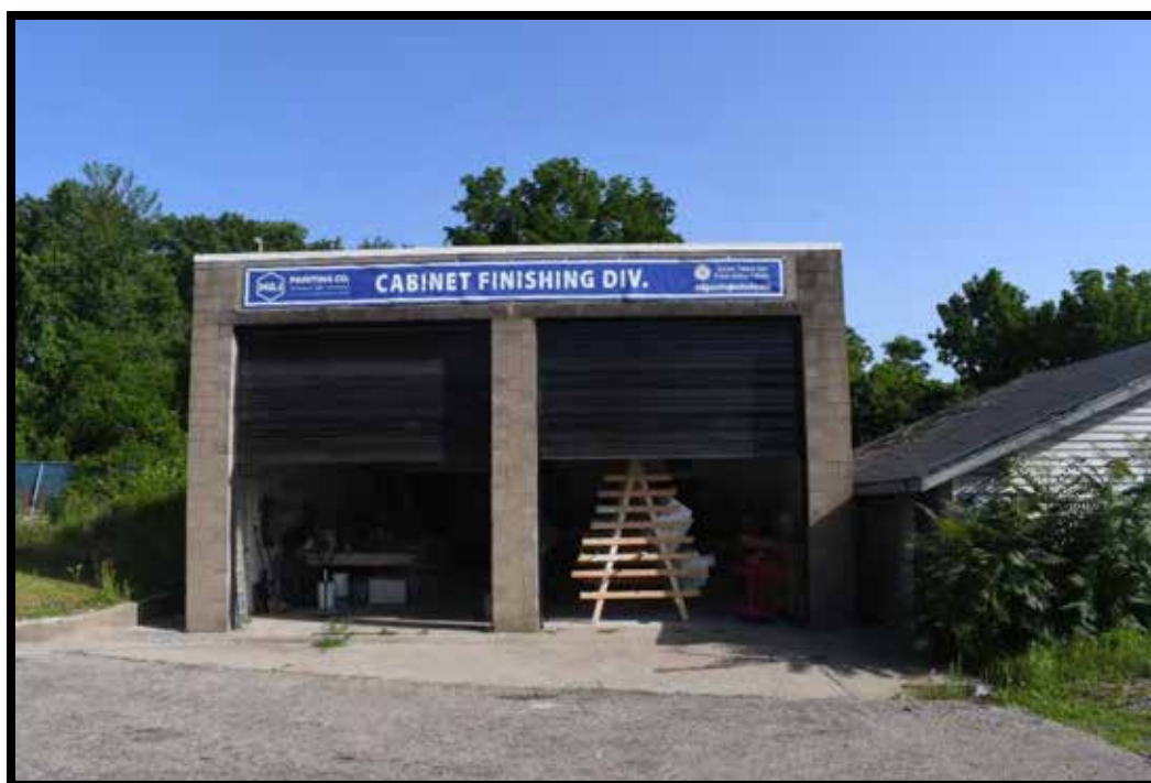
Plate 369. Garage, looking northwest.
