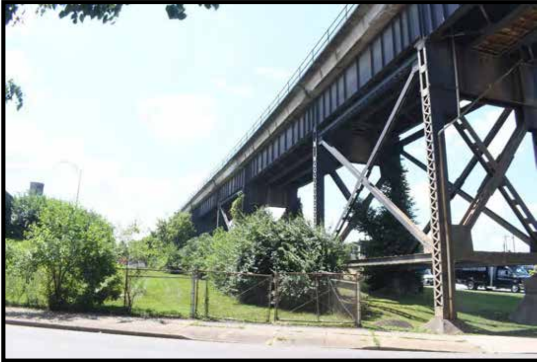
Plate 24. CSX Railroad Bridge No. 059R0062N (KEC-1063), looking south.
