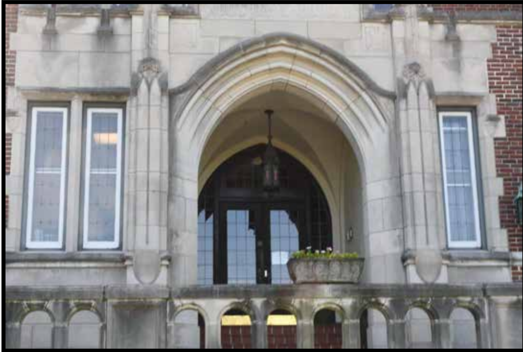
Plate 67. SND Provincial House and Convent. Entry detail of original 1927 building, looking south.
