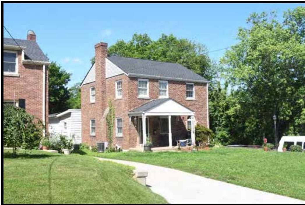
Plate 475. House, looking west.
