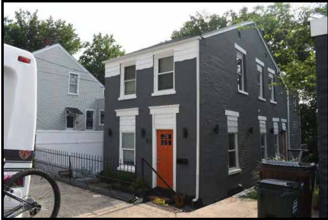
Plate 143. House, looking northeast.
