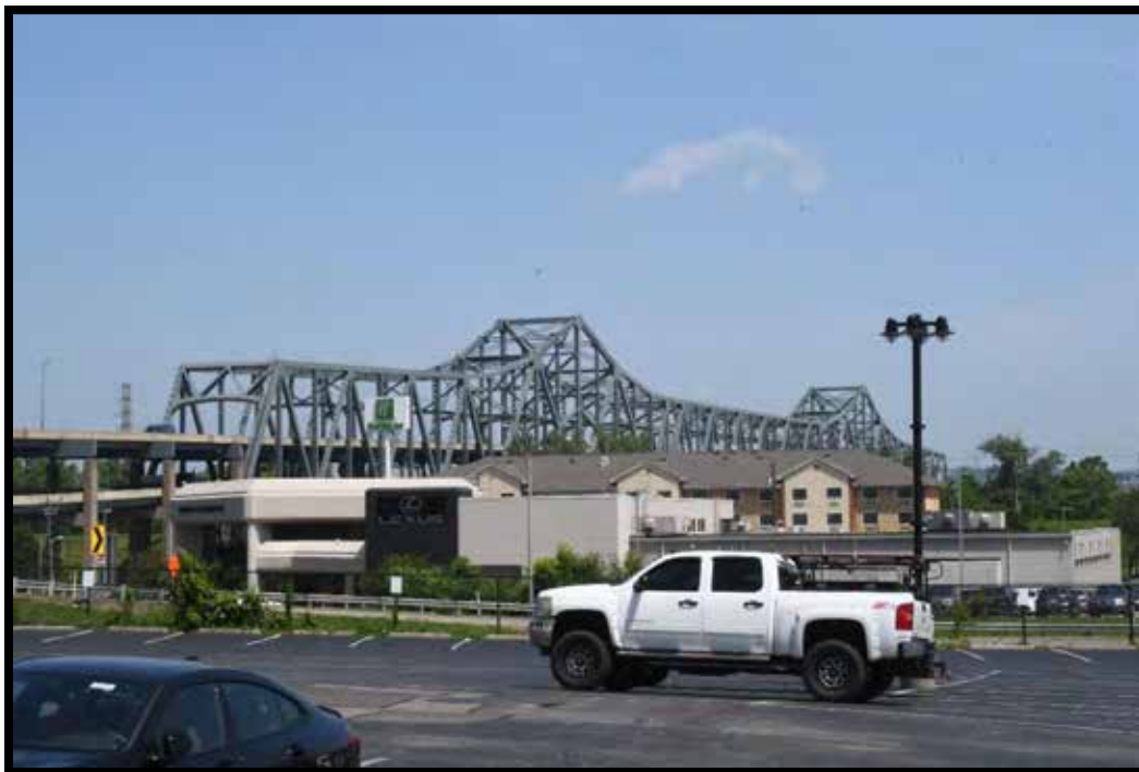
Plate 36. Brent Spence Bridge, looking NW.
