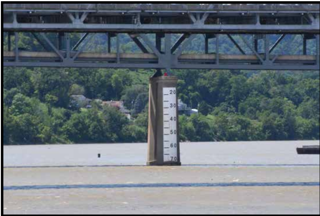
Plate 39. Detail of Brent Spence Bridge pier showing depth markings, looking west.
