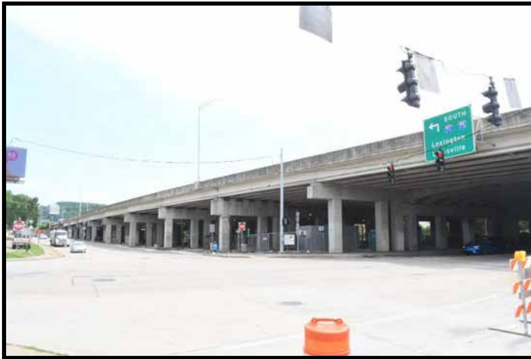
Plate 536. Bridge No. 059B00044R, looking west.
