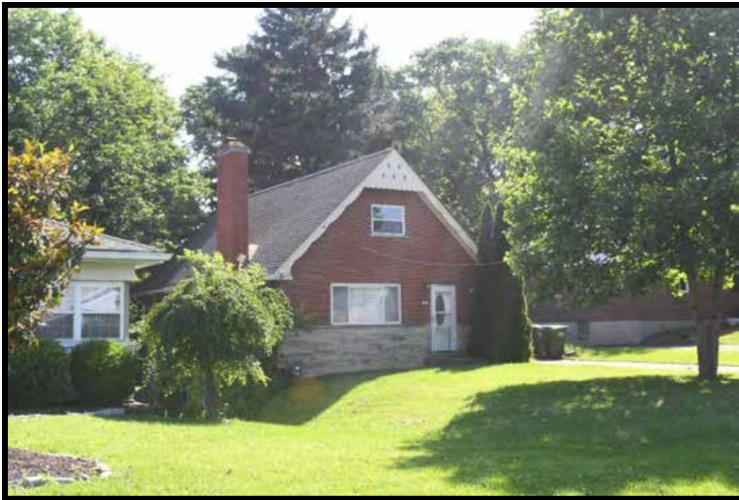
Plate 460. House, looking northeast.
