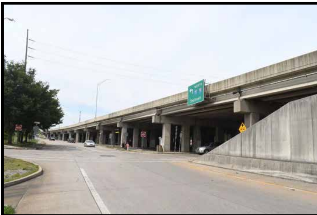
Plate 539. Bridge No. 059B00044L, looking north.
