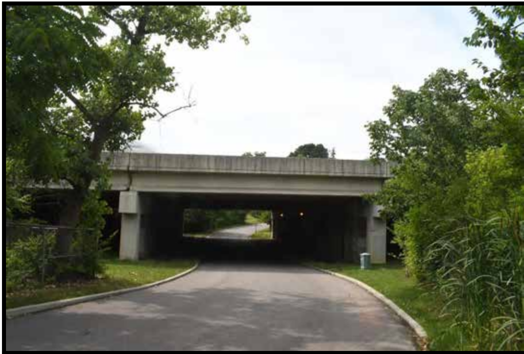
Plate 543. Bridge No. 059B00043R, looking northwest.
