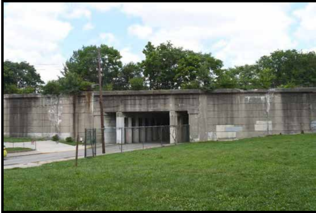
Plate 100. CSX Railroad Bridge No. 059R00626N, looking NE.
