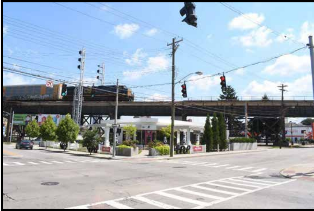
Plate 26. CSX Railroad Bridge No. 059R00610N (KEC-1065), looking NE.
