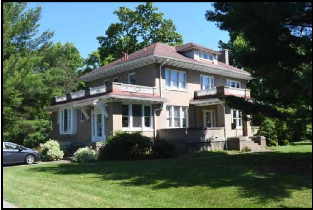
Plate 185. Highland Cemetery. Superintendent's house (D), looking SE.
