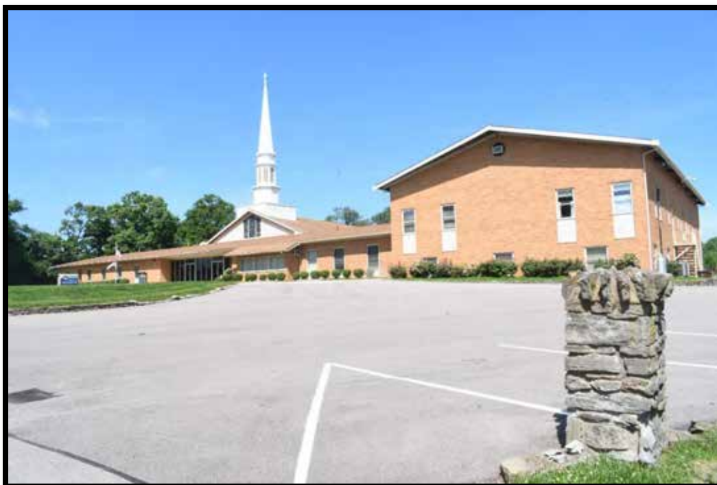
Plate 478. Church and (B) stone entrance posts, looking west.
