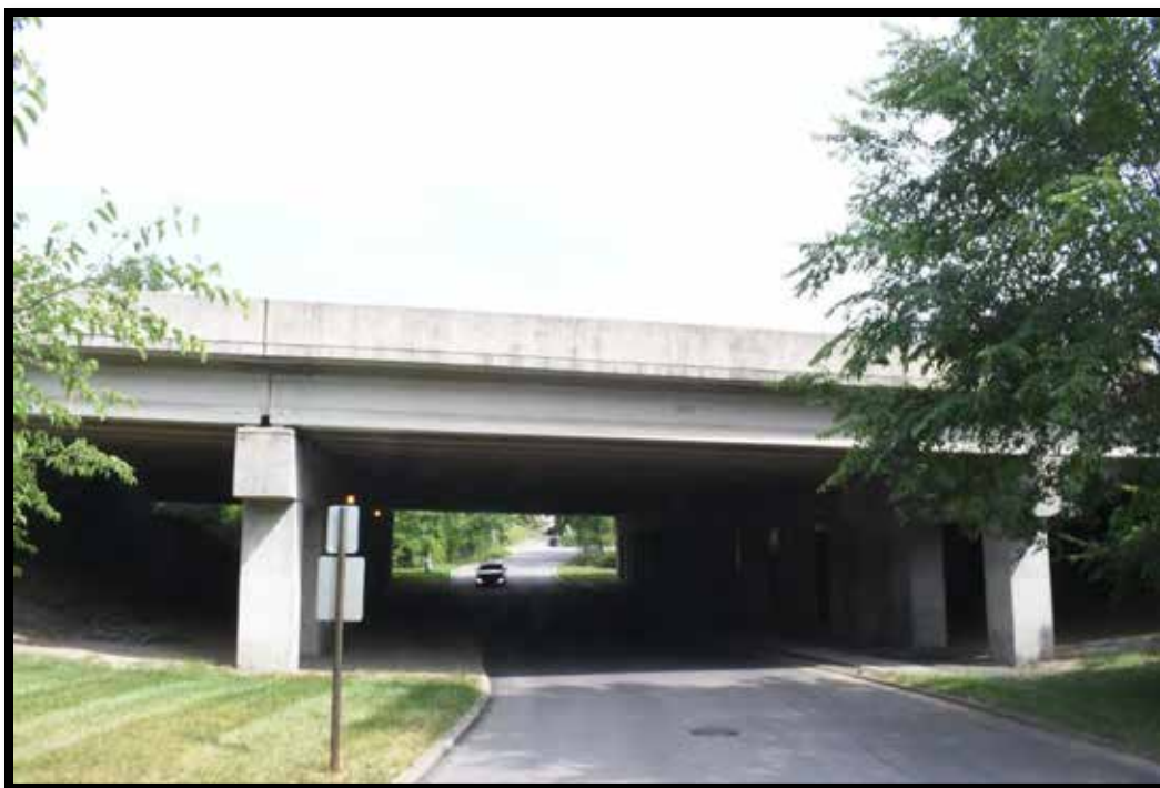
Plate 545. Bridge No. 059B00043L, looking northwest.
