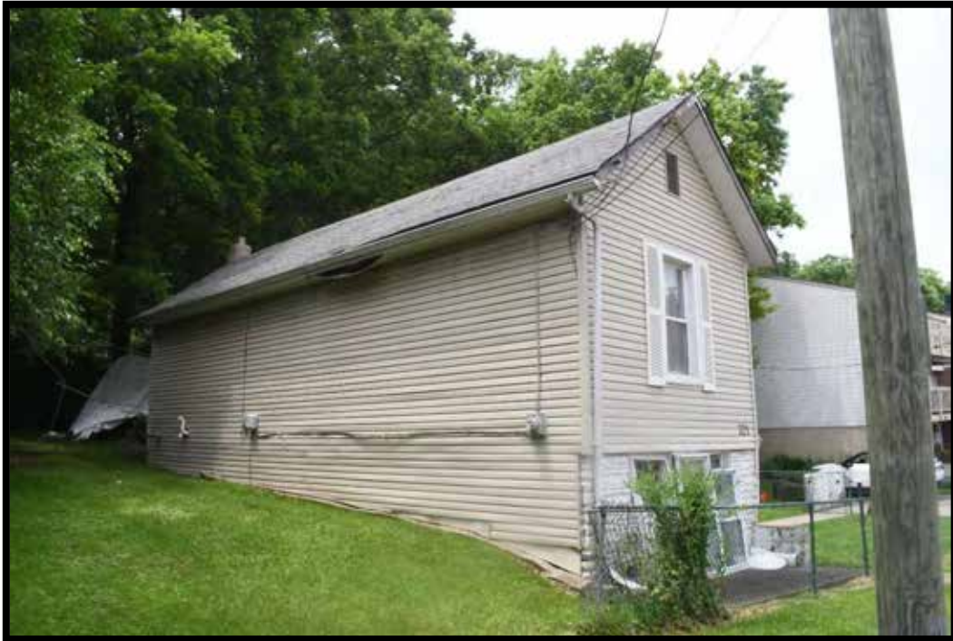
Plate 266. House, looking NW.
