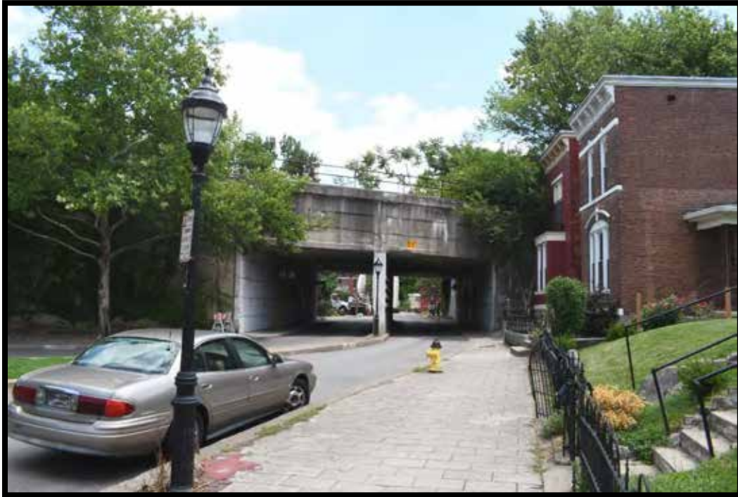
Plate 98. CSX Railroad Bridge No. 059R00622N, looking east.
