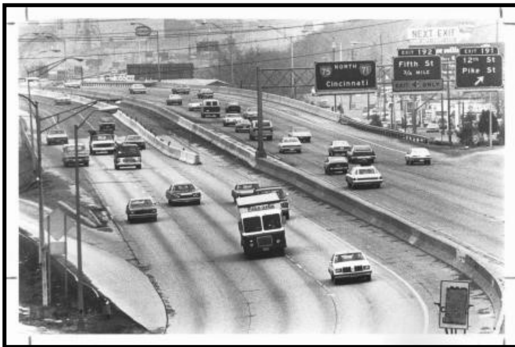
Figure 91. Bridge No. 059B00044L. Photograph depicting this bridge being widened, April 3, 1981, looking north. 472
