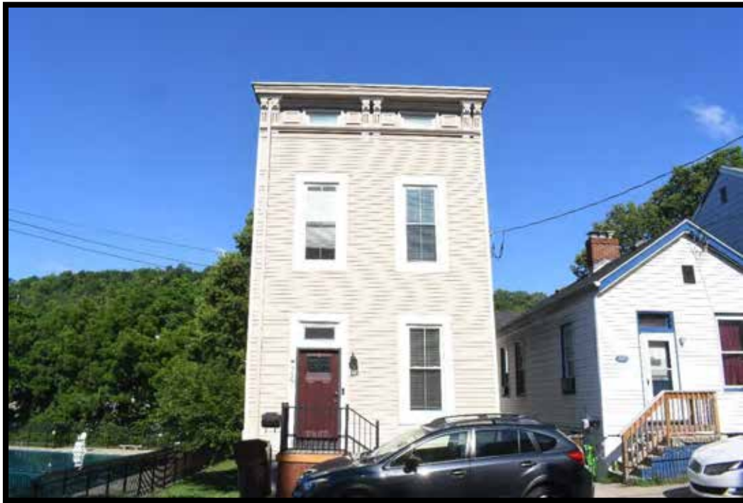
Plate 115. House, looking west.
