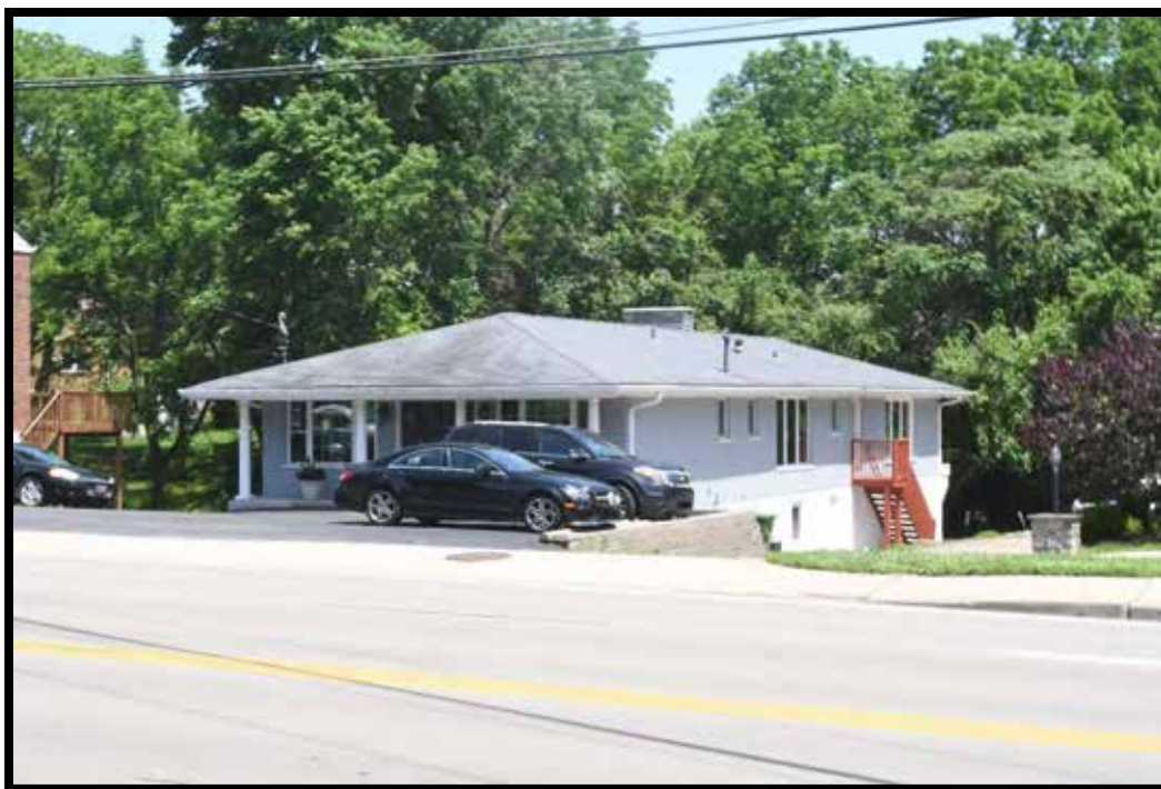
Plate 429. Office building, looking east.
