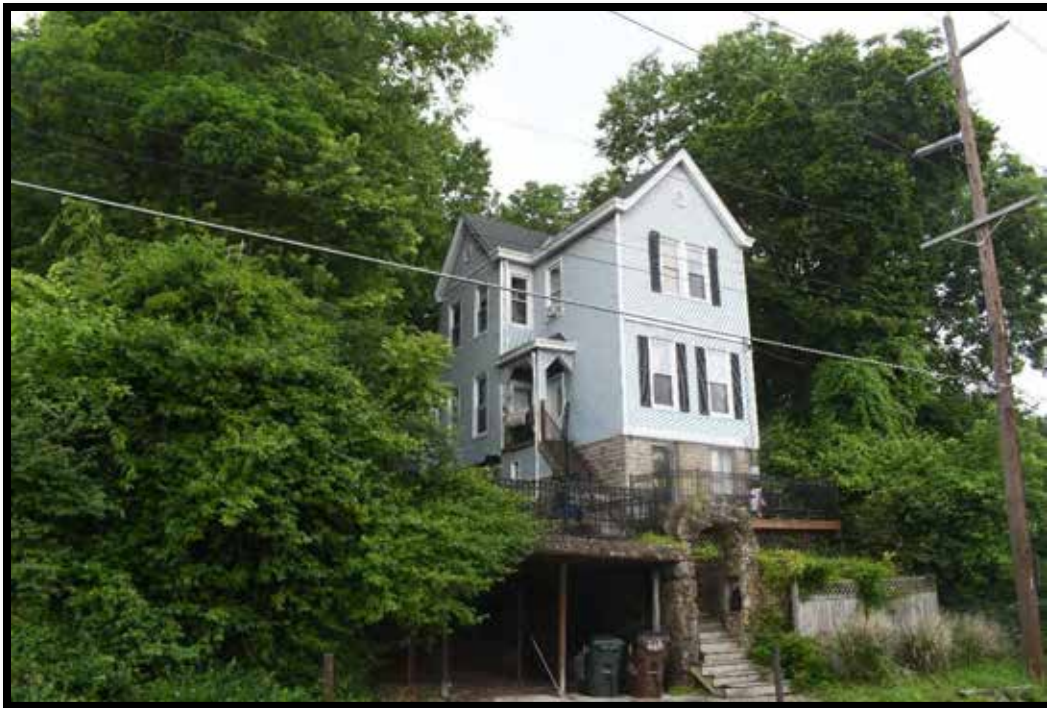
Plate 267. House, looking NW.
