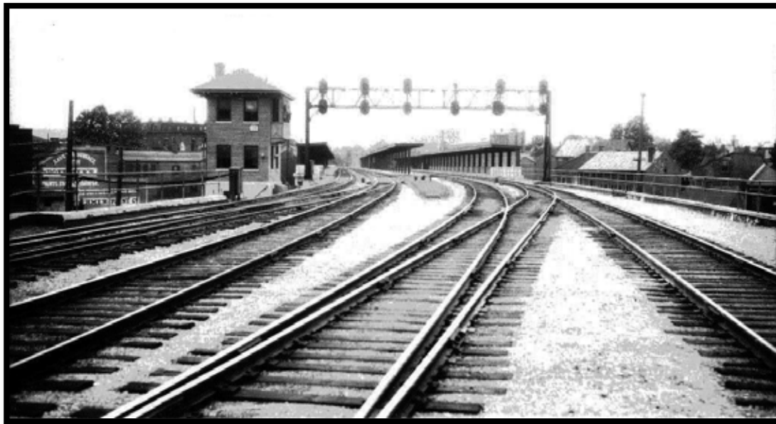
Figure 13. Approach to the C&O RR Bridge at OB Interlocking, June 1930. 54
