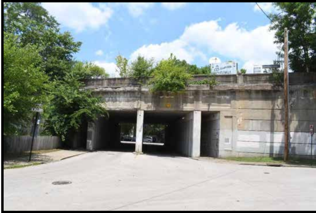
Plate 103. CSX Railroad Bridge No. 059R00627N, looking NE.
