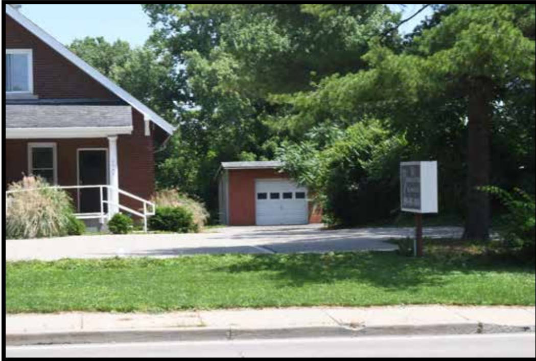
Plate 435. Garage (B), looking southeast.
