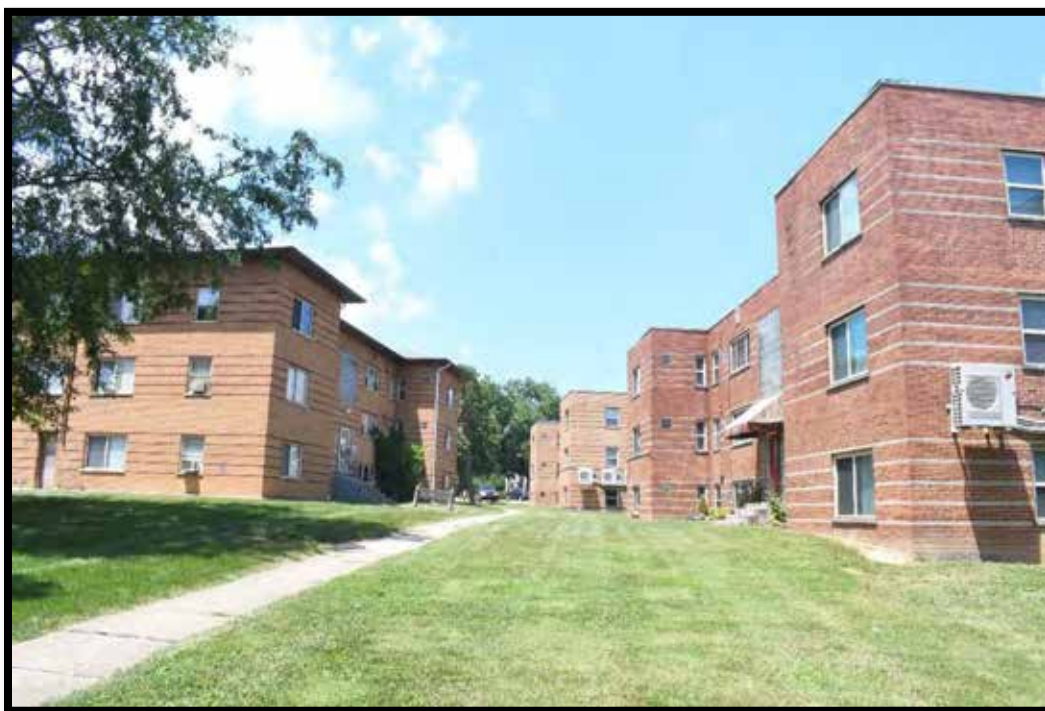
Plate 167. Courtyard at Elberta Circle, looking northwest
