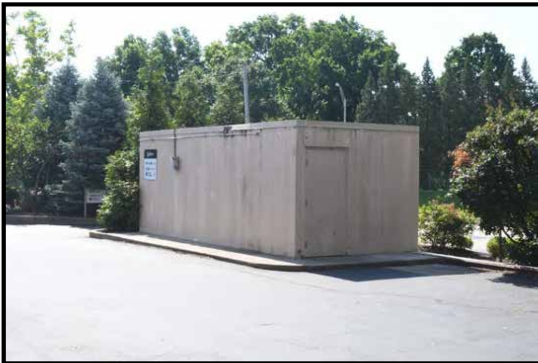
Plate 35. Outbuilding (C), looking southeast.
