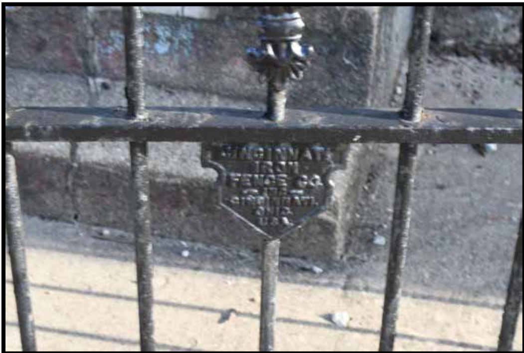
Plate 91. Fence (B), looking north.
