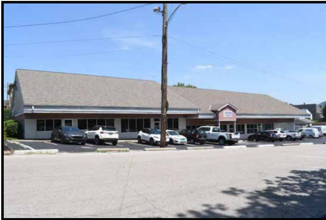
Plate 361. Commercial Building, looking northeast.
