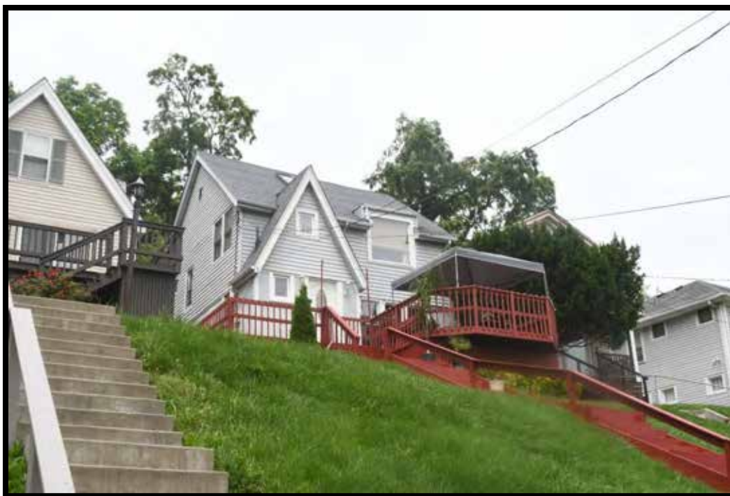
Plate 259. House, looking NW.
