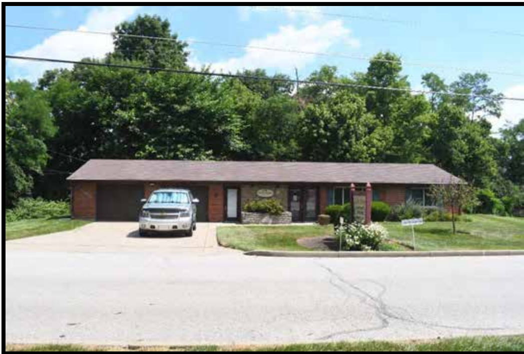
Plate 170. Apartment Leasing Office on Far Hills Drive, looking northeast
