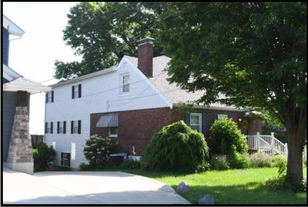
Plate 377. House, looking northeast.
