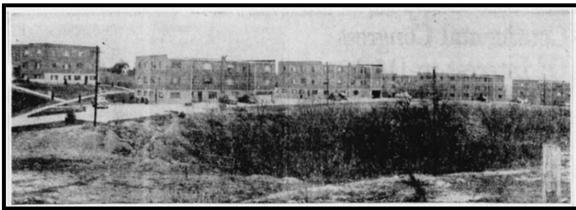
Figure 71. Elberta Apartments, Elberta Circle looking north, showing former lake 286
