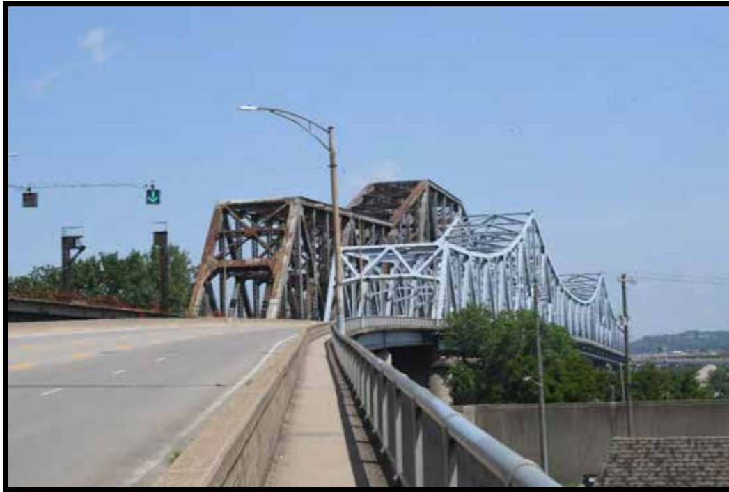
Plate 79. 1929 C & O Railroad Bridge (Left) and 1974 Clay Wade Bailey Bridge (Right)
