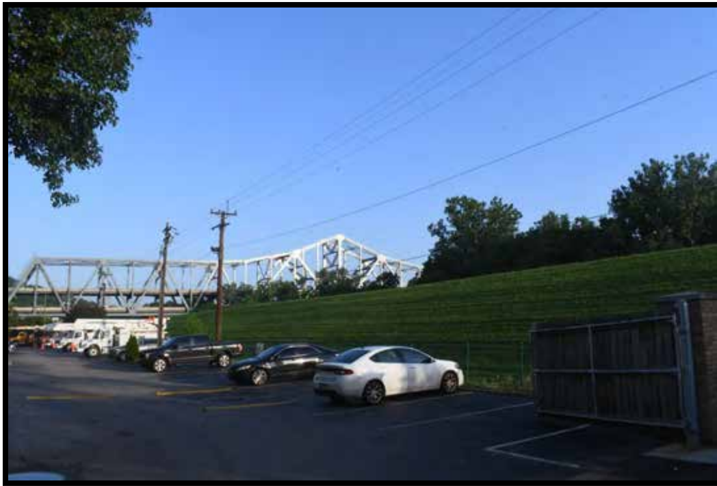
Plate 41. Covington Levee System. Southside of earthen levee wall, looking northwest from the rear (northern) parking lot of KEC-1060.
