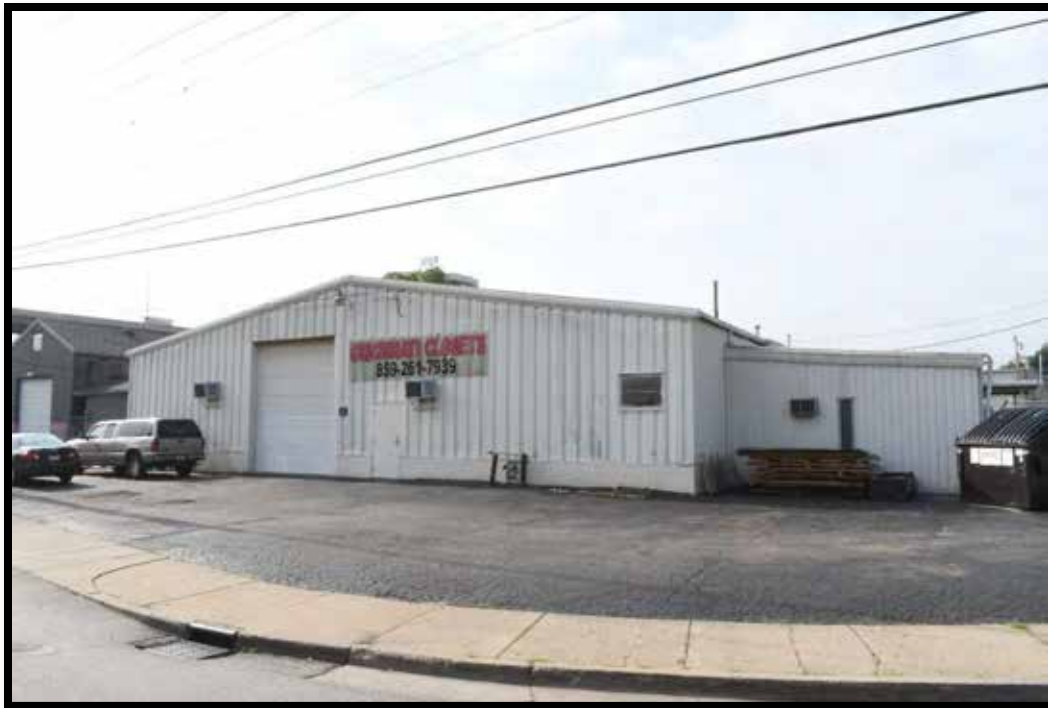
Plate 324. Commercial building, looking southeast.
