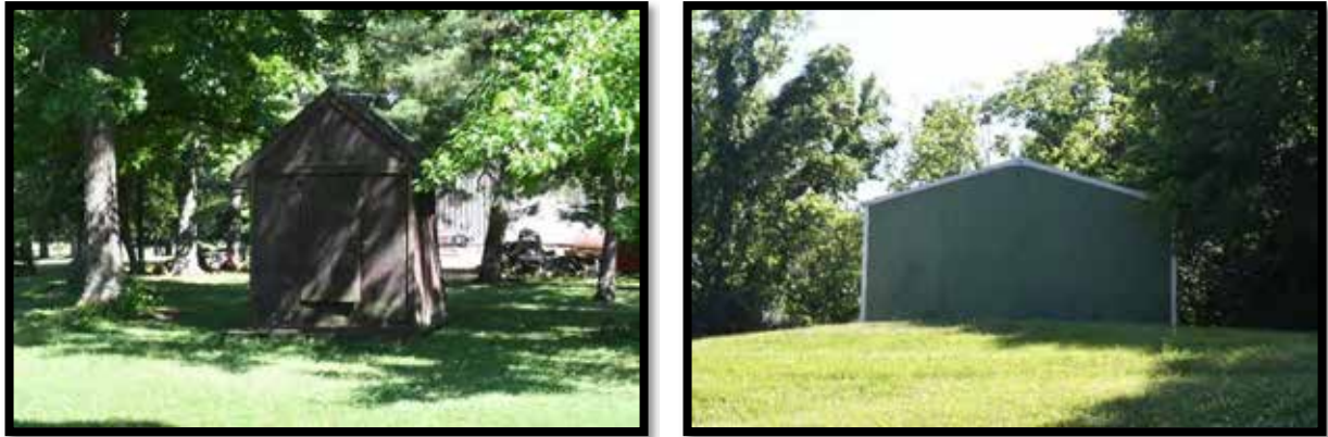
Plate 194. Highland Cemetery. Left: storage shed (F), looking east. Right: Maintenance garage (J), looking SW.
