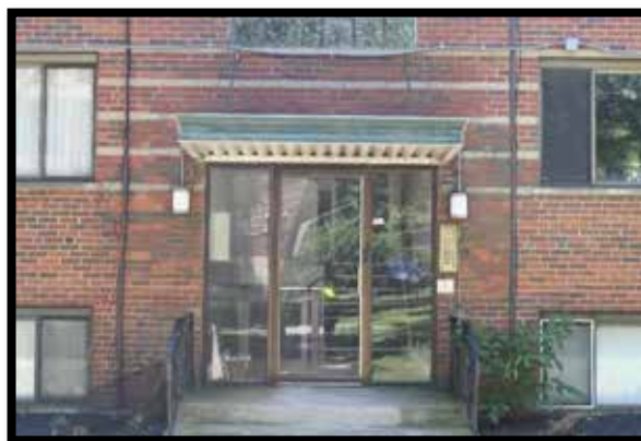
Plate 168. Left, St. Joseph Lane, Original Glass Block Sidelights, Multi-Story Glass Block Stairwell Window, and Steel Casement Windows; Right, Elberta Circle, Original Metal Front Canopy and Lighting
