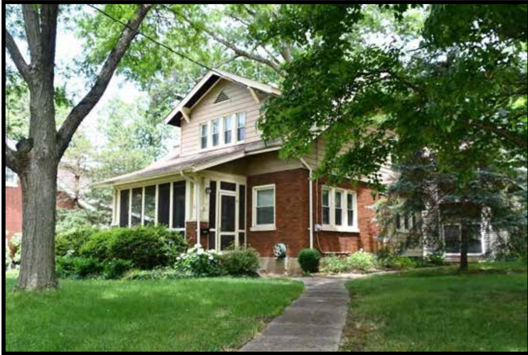
Plate 166. Looking NE at 16 Woodlawn Avenue. This bungalow is representative of early twentieth century middle-class housing in the Beechwood Historic District, most of which is located on Woodlawn Avenue or the east side of Beechwood Road.
