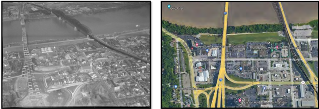
Figure 47. Covington Levee System between Crescent Avenue and Bakewell Street. Left: Historic aerial of Levee circa 1963, looking northwest. 199 Right: Circa 2022 aerial map, looking north. 200
