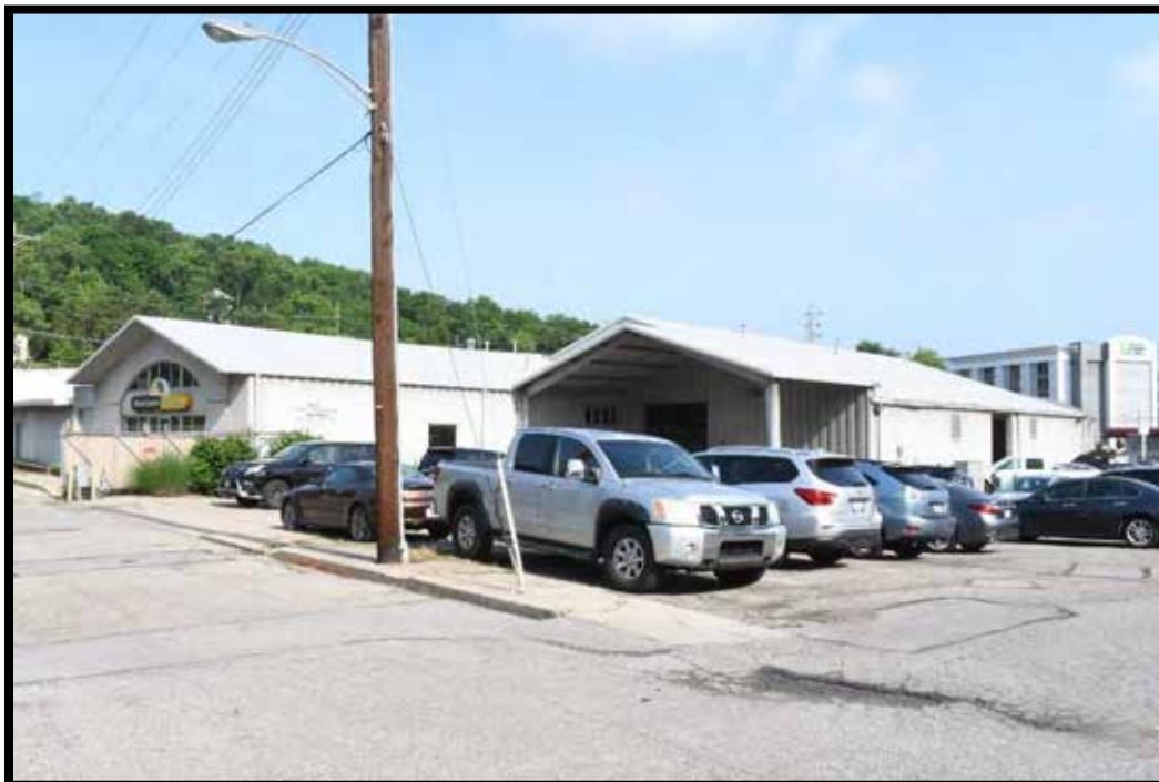
Plate 323. Commercial building addition, looking northwest.
