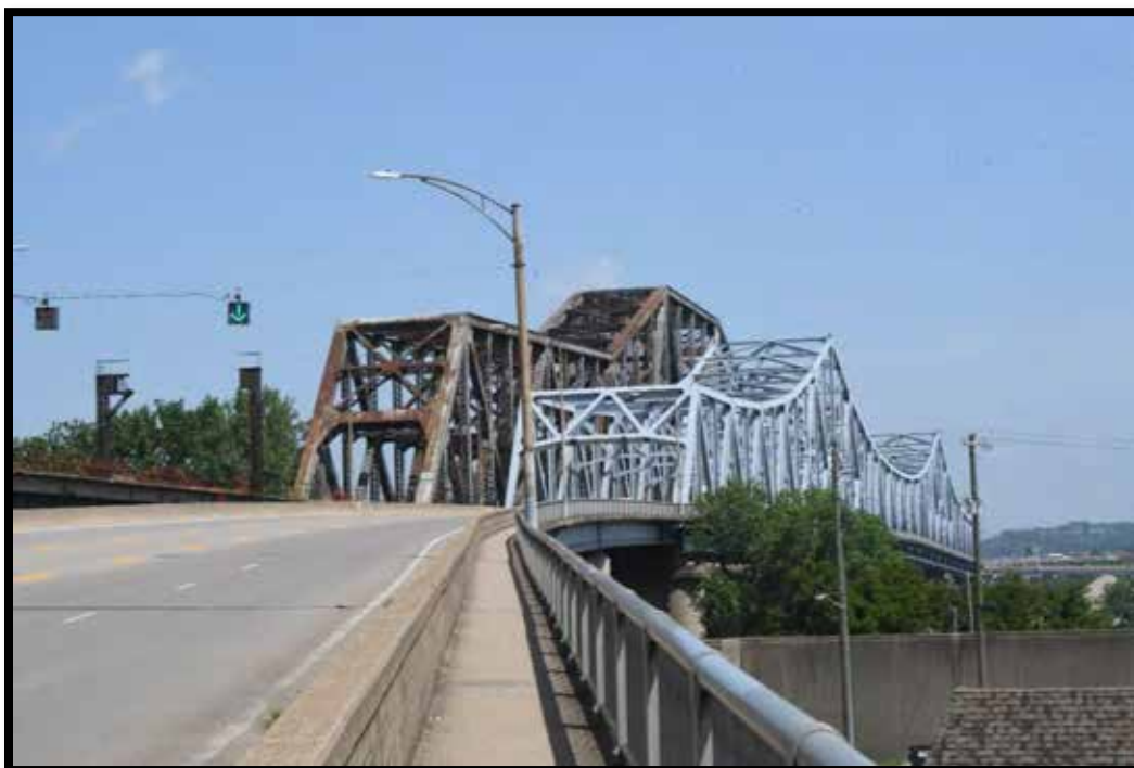
Plate 18. C & O Railroad Bridge (left) and Clay Wade Bailey Bridge (right), looking northwest.
