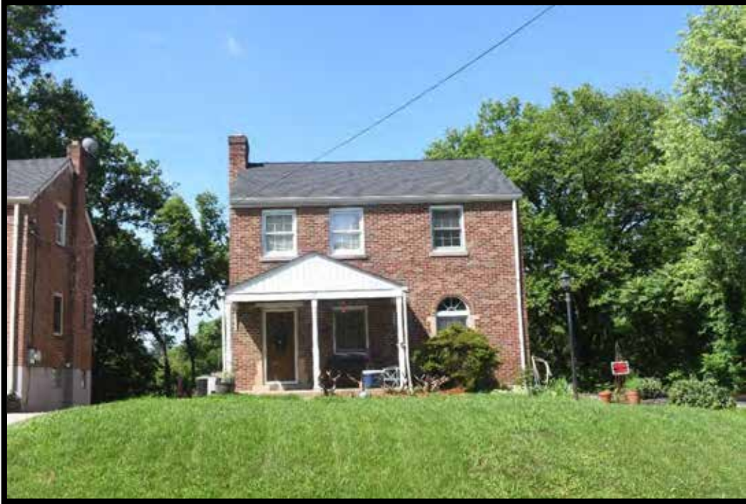
Plate 476. House, façade, looking southwest.
