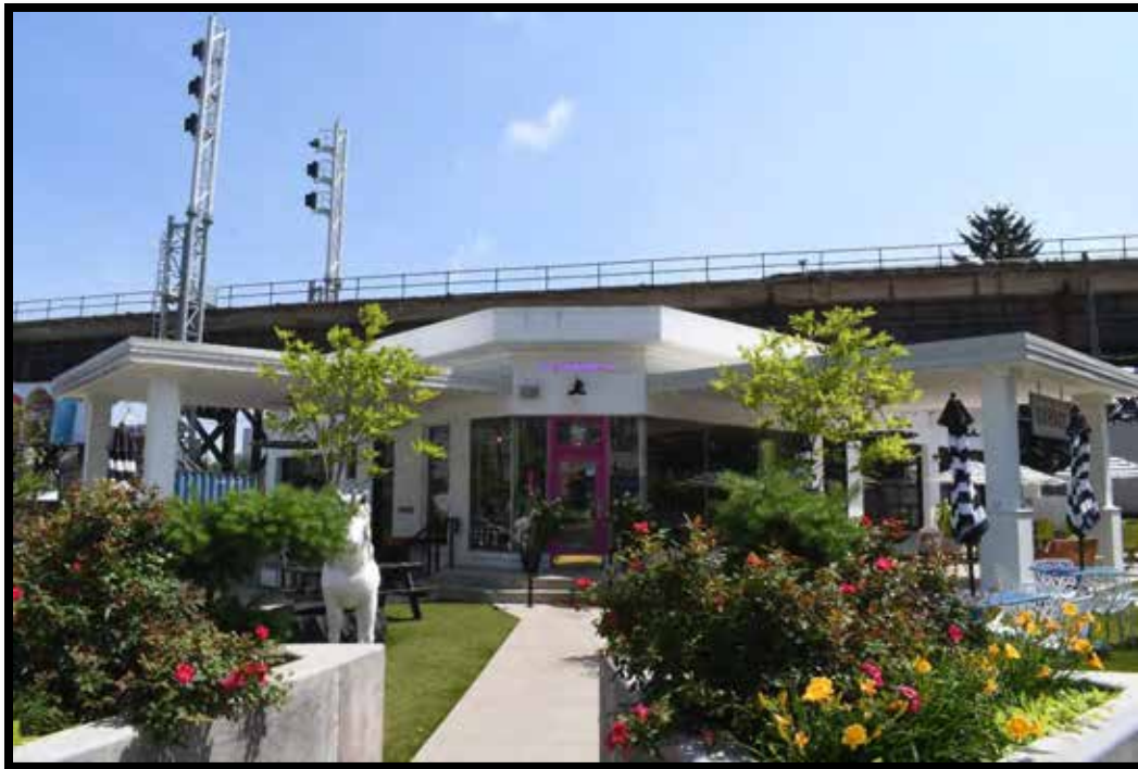
Plate 345. Commercial building, looking northeast.
