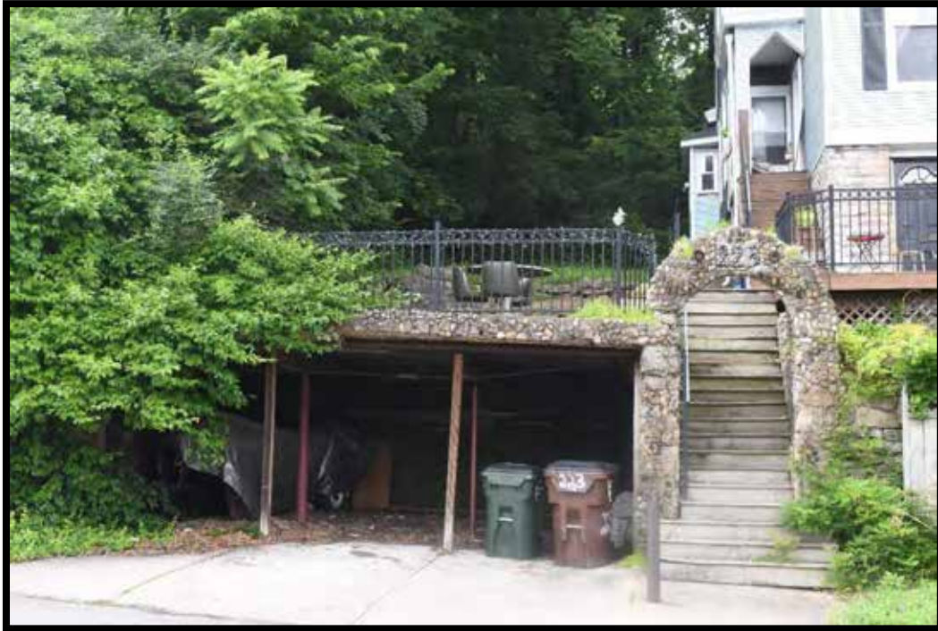
Plate 269. Garage (B), looking west.
