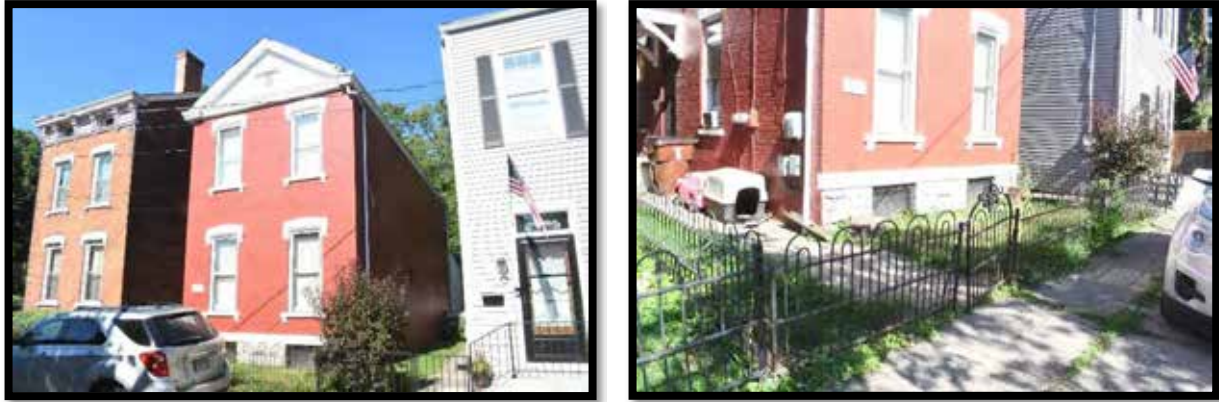
Plate 130. Left: House, looking southwest. Right: Fence (B), looking northwest.
