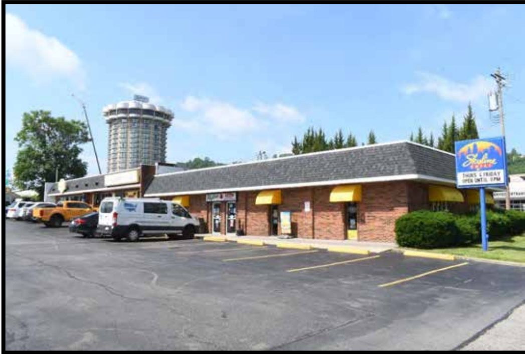
Plate 340. Commercial building, looking southwest.
