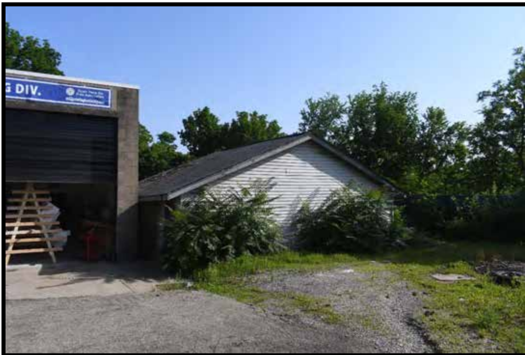
Plate 371. Outbuilding (95B), looking northwest.
