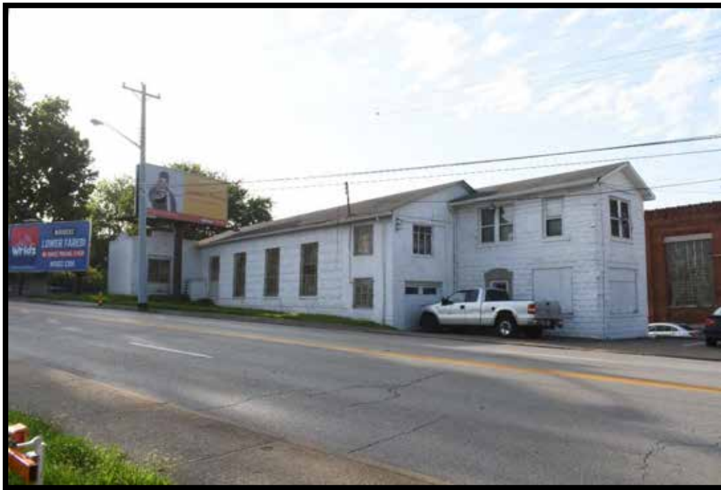
Plate 95. Commercial Building, looking southeast.
