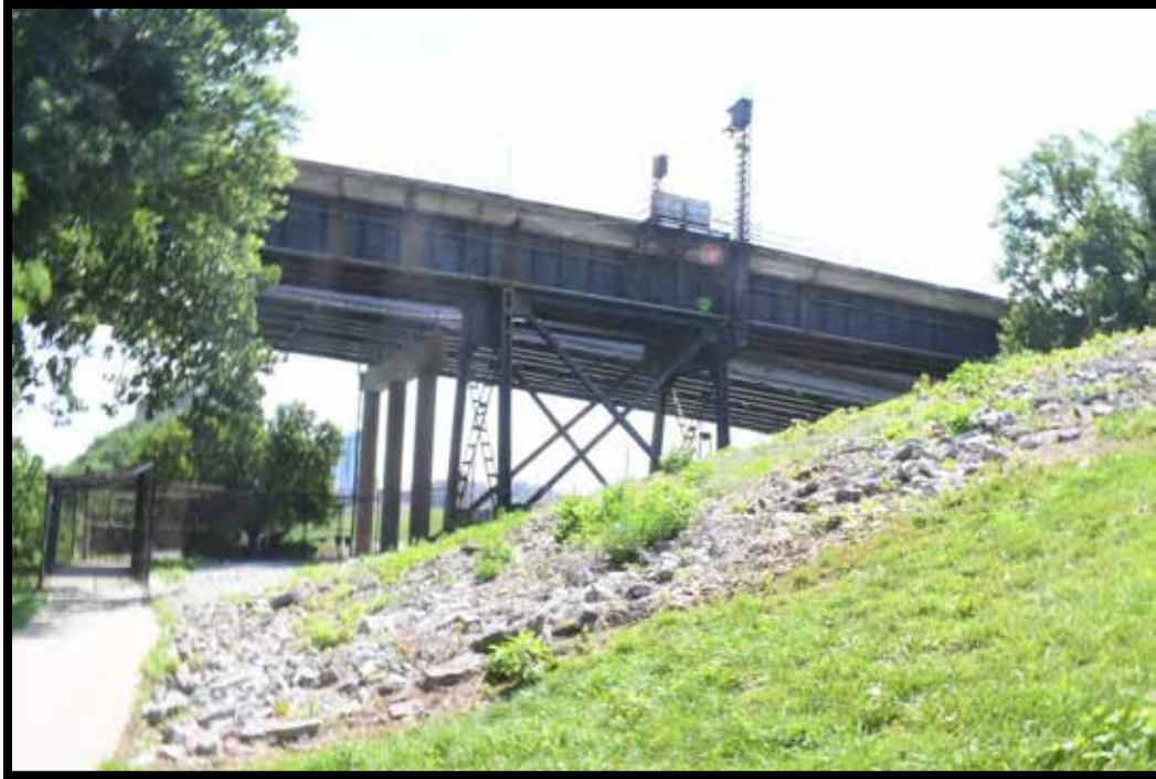
Plate 20. CSX Railroad Bridge No. 059R00633N (KEC-1062), looking east.
