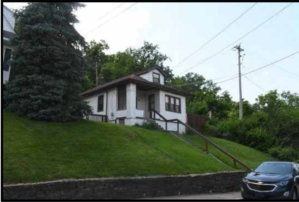
Plate 302. House and stone wall, looking NW.
