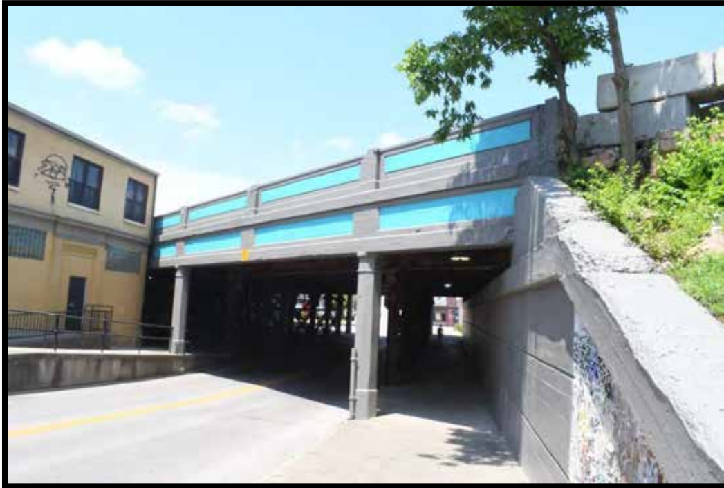
Plate 111. CSX Railroad Bridge No. 059R00620N, looking north.
