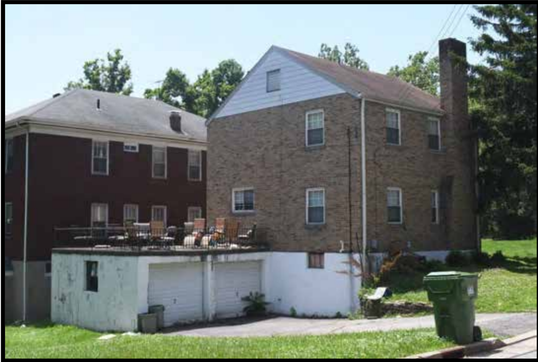
Plate 418. House, looking west.
