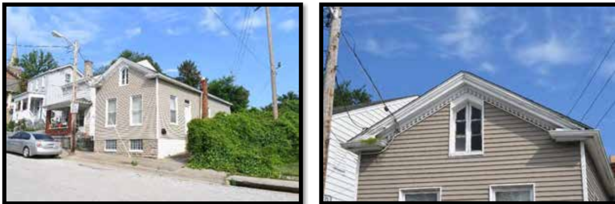
Plate 146. Left: House, looking northwest. Right: Detail of gable returns, box gutters, dentiled cornice, and pentagon window.
