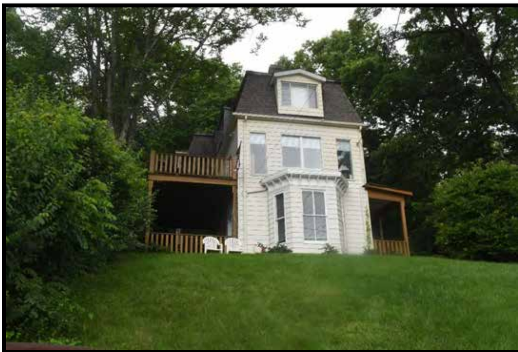
Plate 241. House, looking west.
