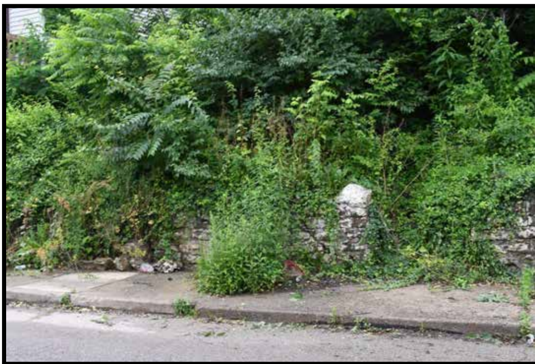
Plate 308. Mortared stone wall, looking west.
