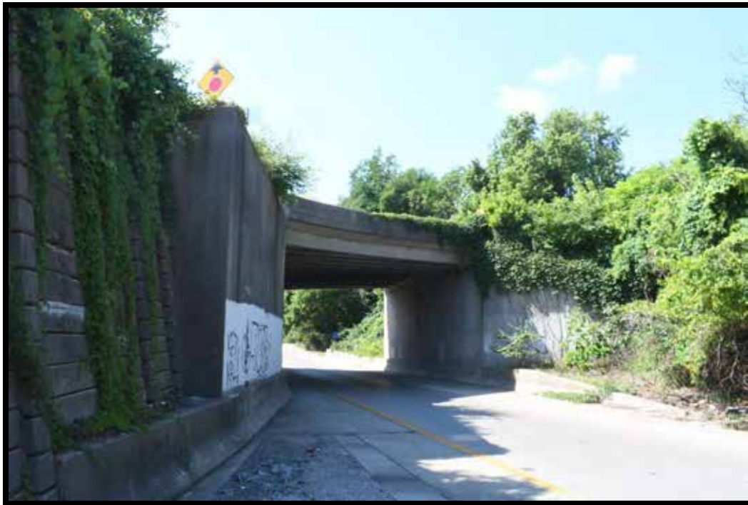
Plate 530. Bridge No. 059B00039N, looking south.
