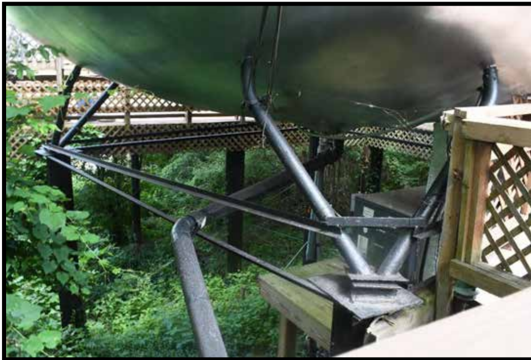
Plate 13. Steel support piers of Covington Futuro, looking SE.
