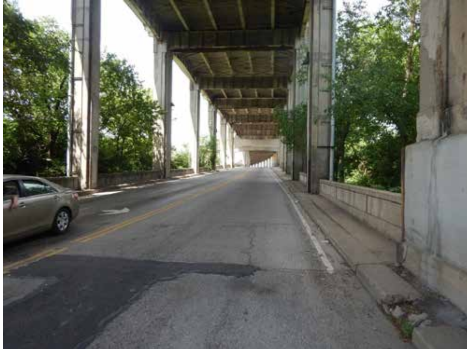
Photograph 140. View along Western Hills Viaduct, looking west.
