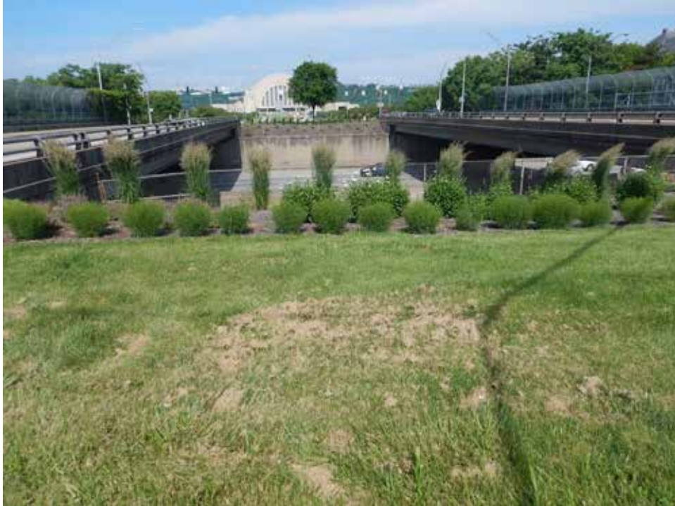
Photograph 90. View along I-75 and right-of-way, looking west.
