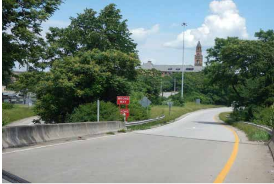
Photograph 85. View of I-75 right-of-way with SWH, looking north-northwest.
