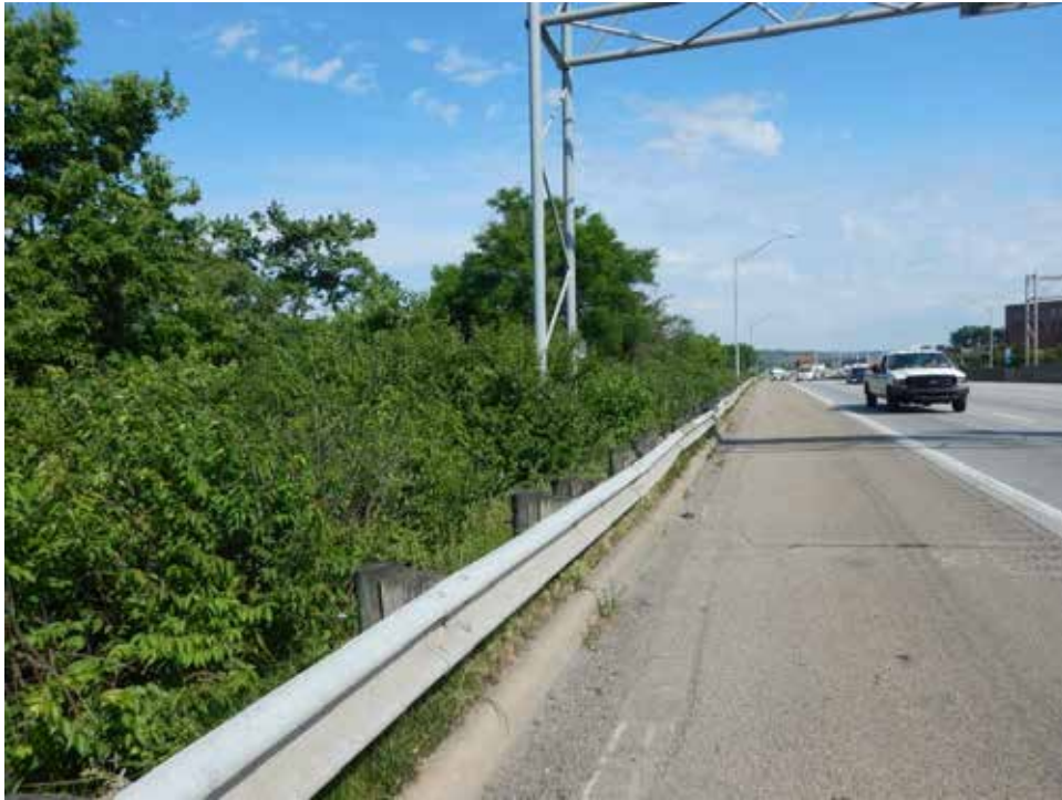
Photograph 105. View along I-75 and right-of-way with SWH, looking north-northwest.
