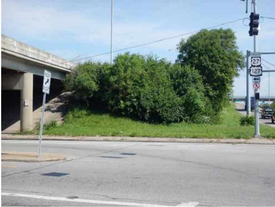
Photograph 122. View of I-75 right-of-way with SWH, looking north.
