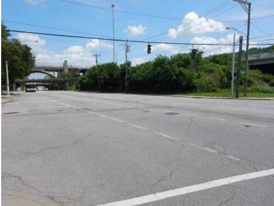
Photograph 131. View of I-75 right-of-way with shrubby vegetation, looking northeast.
