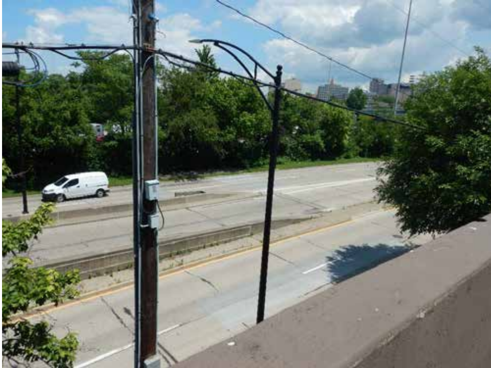
Photograph 72. View of I-75 right-of-way with SWH (distant), looking northeast.
