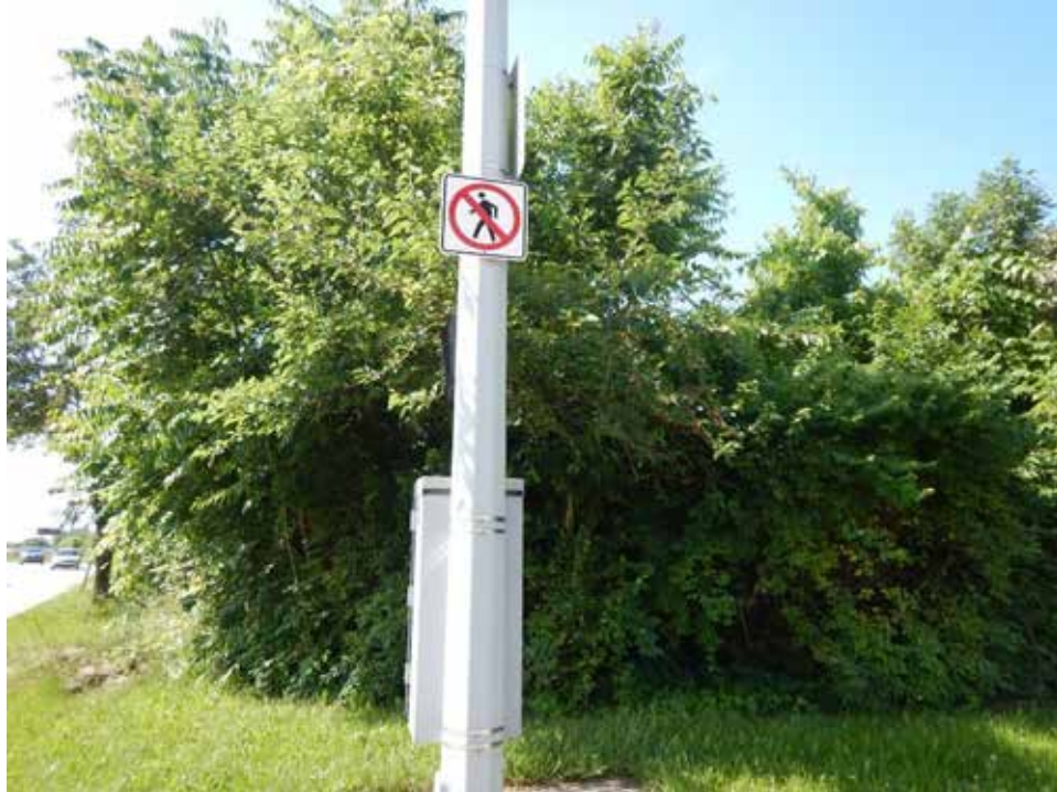
Photograph 120. View of I-75 right-of-way with SWH, looking south
