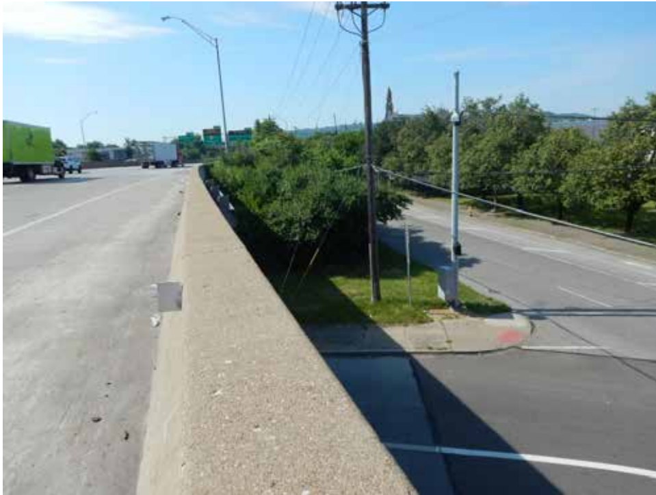
Photograph 101. View along I-75 and right-of-way with SWH, looking south.
