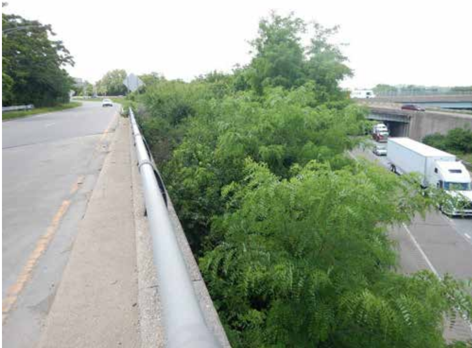
Photograph 47. View of I-75 right-of-way with SWH, looking north.
