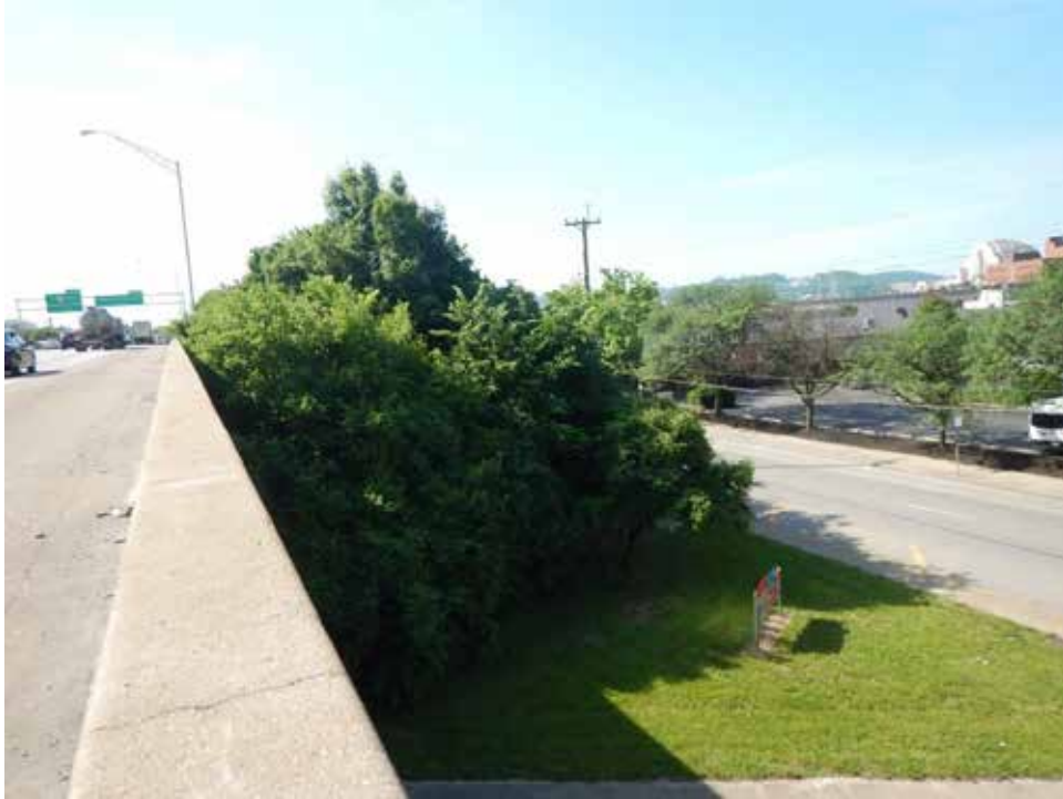
Photograph 111. View along I-75 and right-of-way with SWH, looking south.
