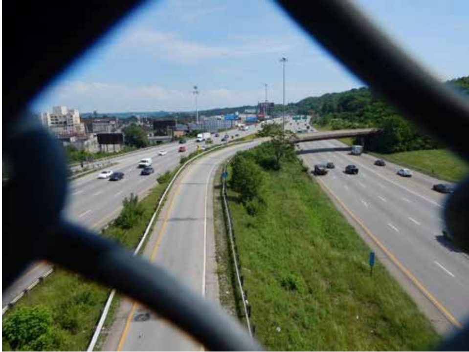
Photograph 142. View of I-75 right-of-way, looking north.
