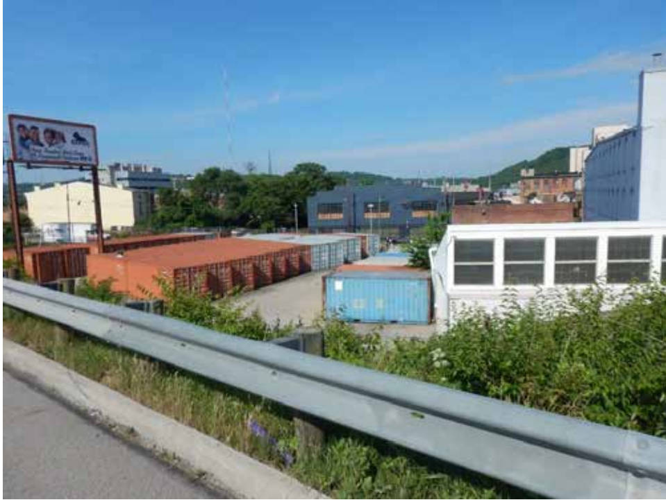
Photograph 154. View of adjacent right-of-way and properties, looking west.
