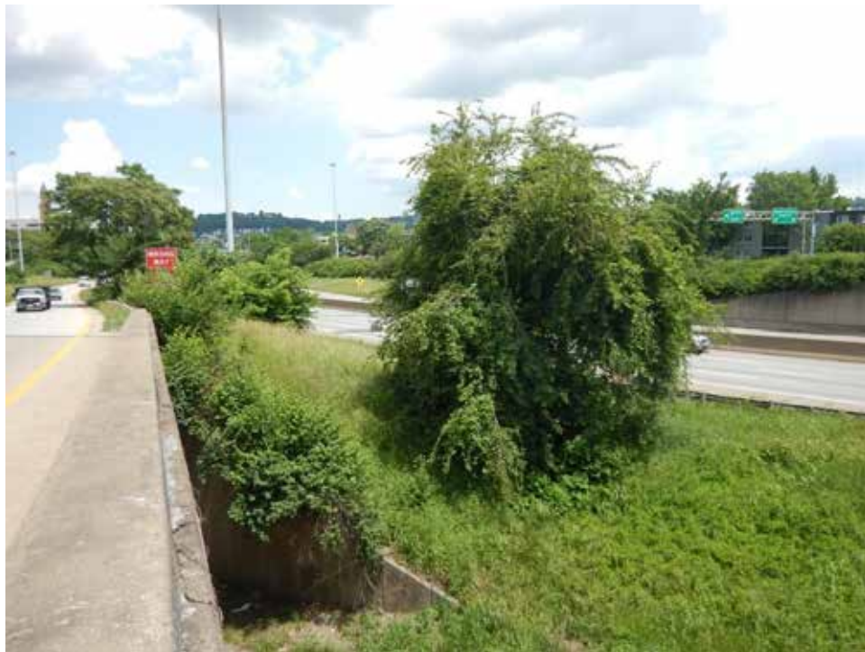
Photograph 86. View of I-75 right-of-way, looking north
