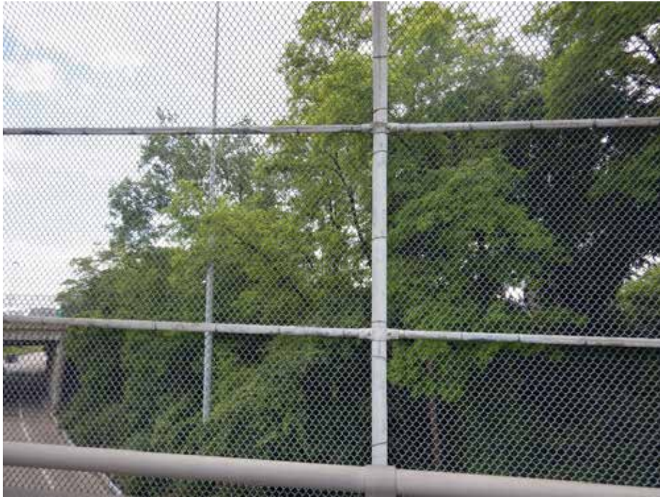
Photograph 63. View of I-75 right-of-way with SWH, looking south.
