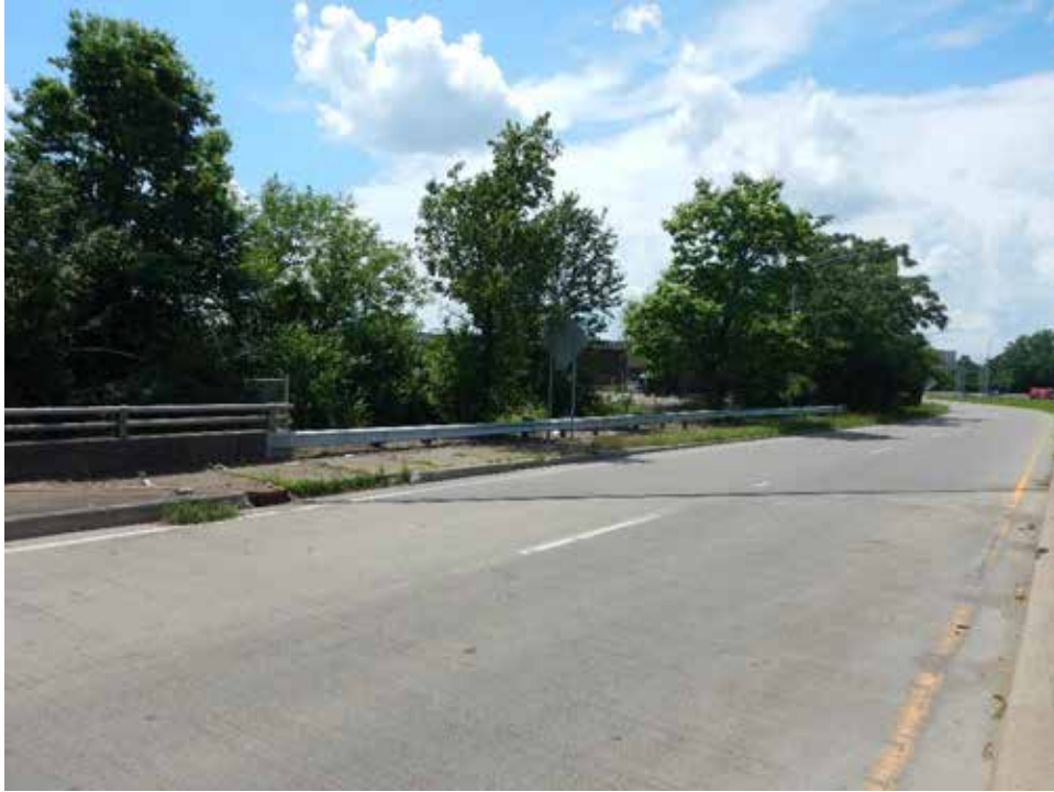
Photograph 46. View of SWH along the 6 th Street Expressway, looking northwest.
