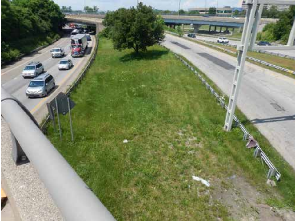
Photograph 44. View of I-75 right-of-way, looking north.
