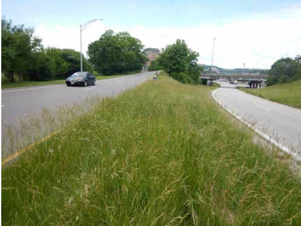
Photograph 68. View of I-75 right-of-way with SWH (distant), looking northwest.
