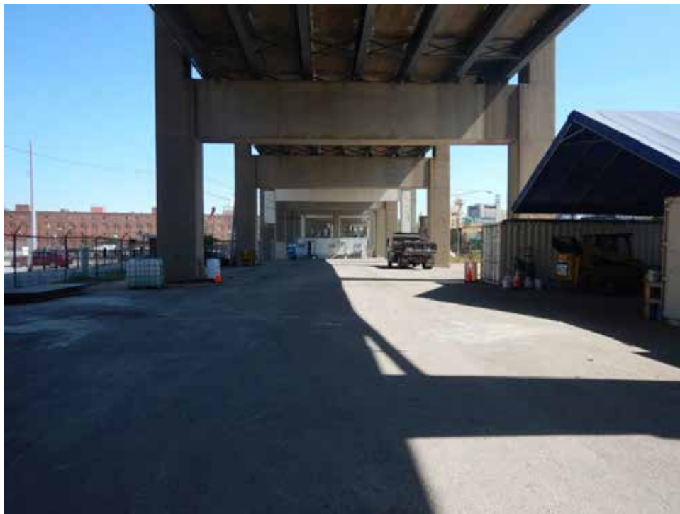
Photograph 10. View of the underside of the Brent Spence Bridge showing no signs of bat usage, looking north.
