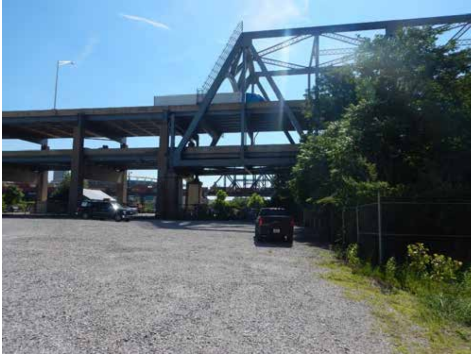
Photograph 3. View of SWH (right) adjacent to the Brent Spence Bridge, looking east.
