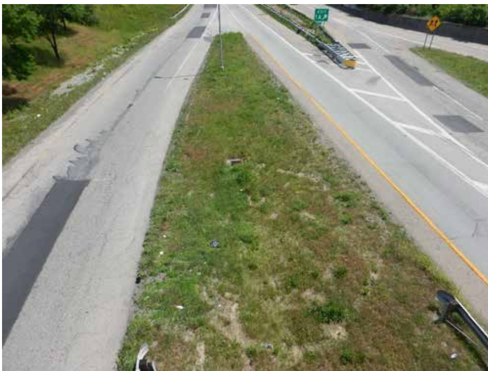
Photograph 40. View of I-75 right-of-way, looking south.
