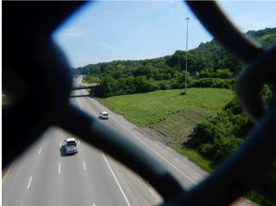
Photograph 143. View of I-75 right-of-way with SWH (along perimeter of interchange), looking northeast.
