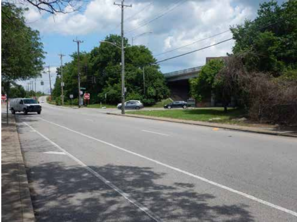
Photograph 110. View of I-75 right-of-way with SWH, looking north
