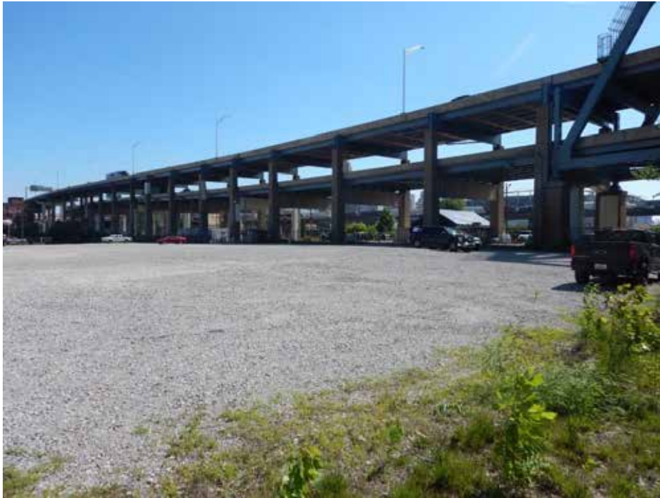
Photograph 5. View of the study area adjacent to the Brent Spence Bridge, looking northeast.
