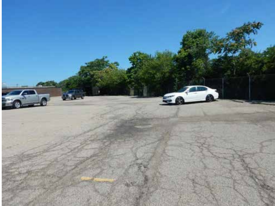
Photograph 28. View of SWH along the I-75 right-of-way and UPS parking area, looking north.
