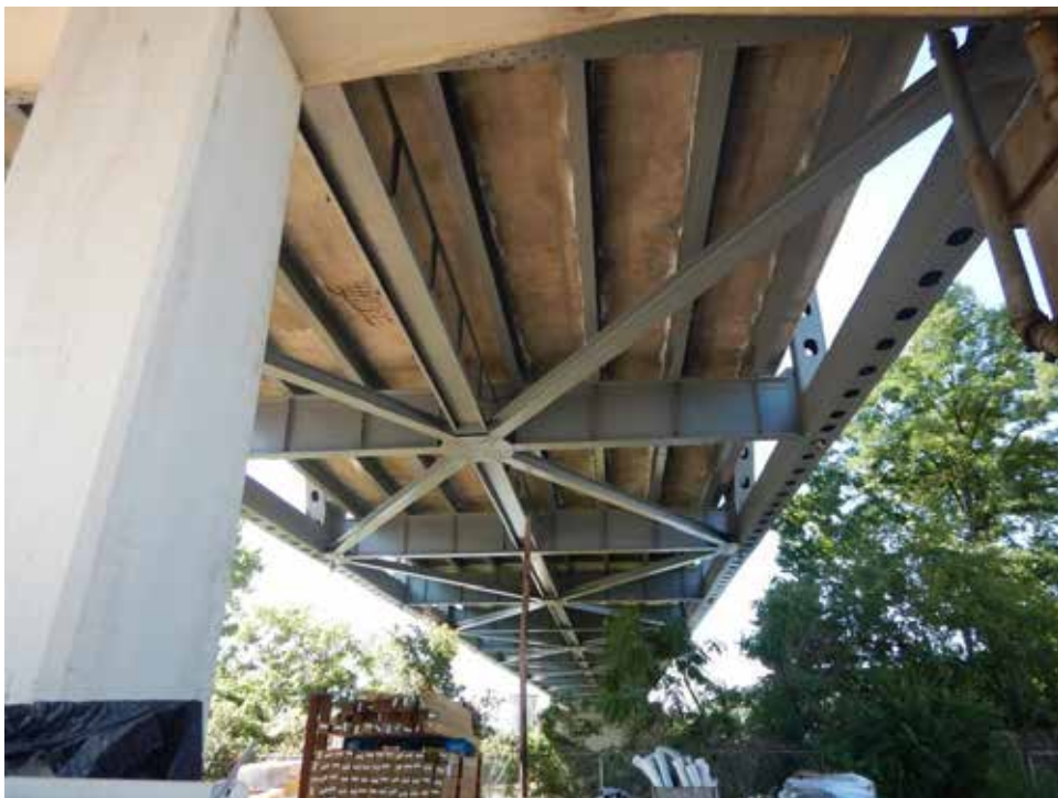
Photograph 8. View of the underside of the Brent Spence Bridge showing no signs of bat usage, looking south.
