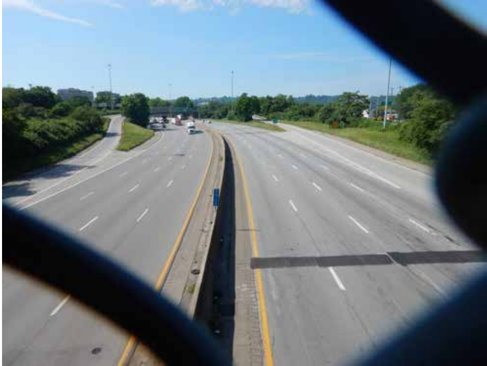
Photograph 91. View along I-75 and right-of-way with SWH, looking south.
