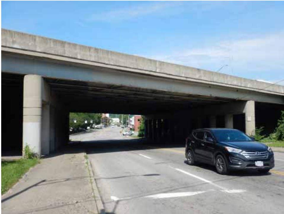
Photograph 107. View along Findlay Street, looking west.
