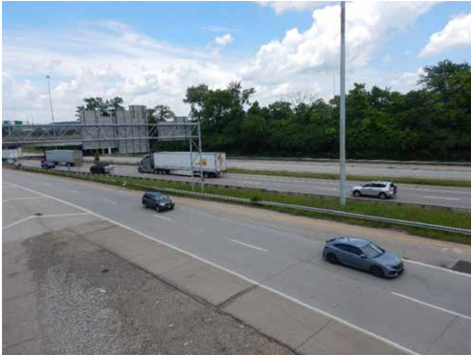
Photograph 65. View of I-75 right-of-way with SWH (distant), looking north.
