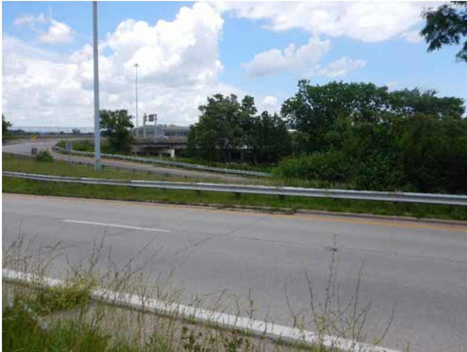
Photograph 67. View of I-75 right-of-way with SWH (distant), looking northeast.
