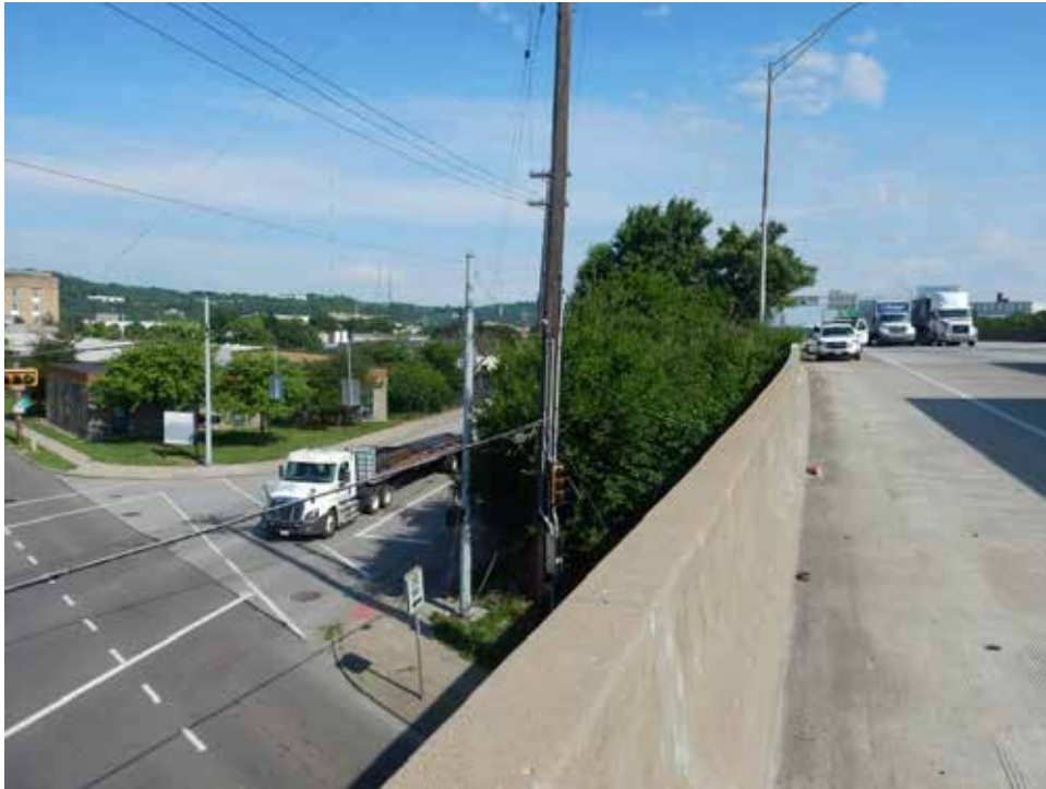
Photograph 103. View along I-75 and right-of-way with SWH, looking northwest.
