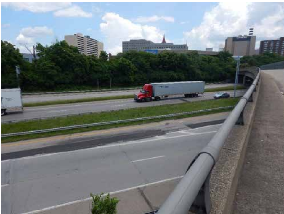
Photograph 64. View of I-75 right-of-way with SWH (distant), looking northeast.
