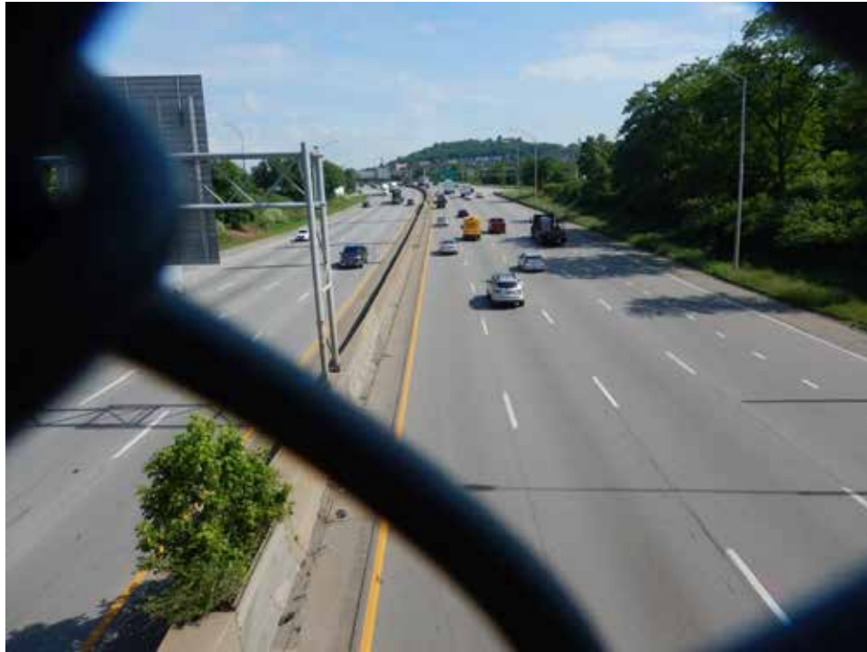
Photograph 95. View along I-75 and right-of-way with SWH (right side), looking north.
