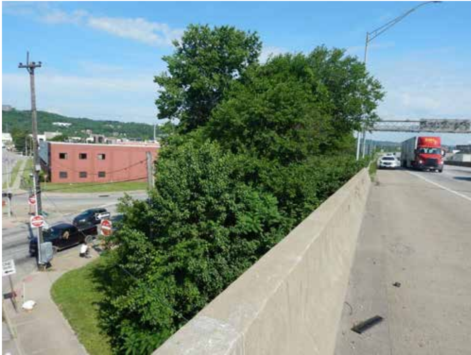
Photograph 113. View along I-75 and right-of-way with SWH, looking northwest.
