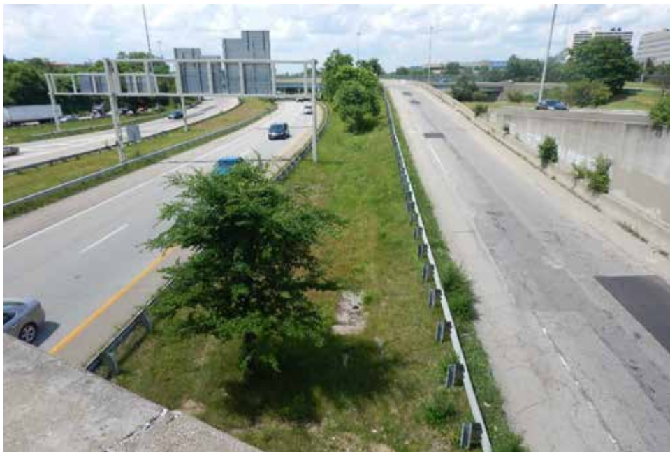
Photograph 42. View of I-75 right-of-way, looking north.
