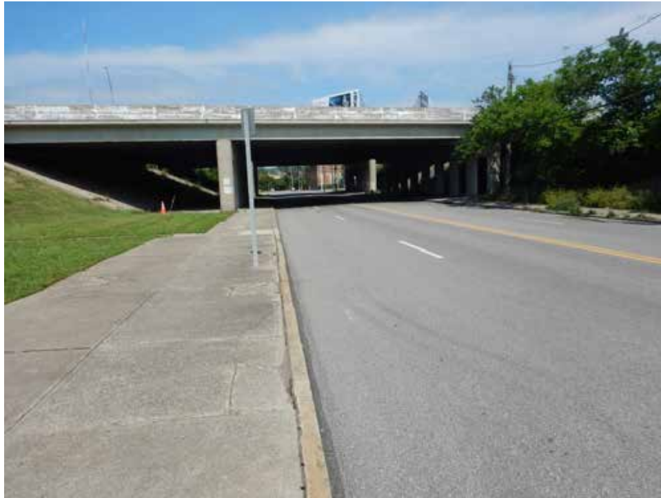
Photograph 129. View along Harrison Avenue, looking west.
