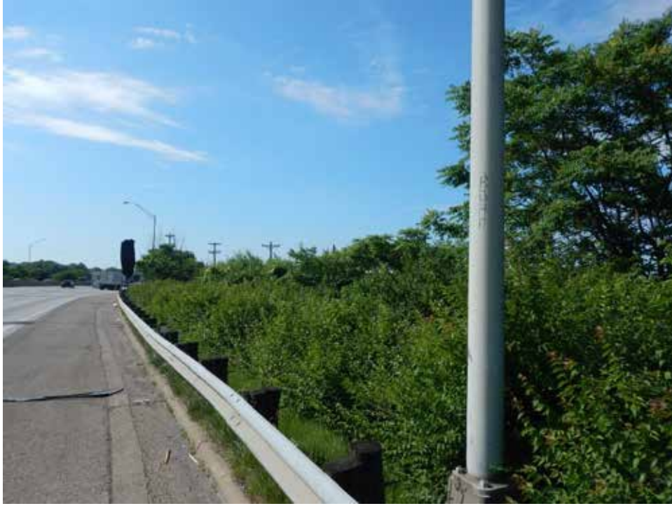
Photograph 104. View along I-75 and right-of-way with SWH, looking southeast.
