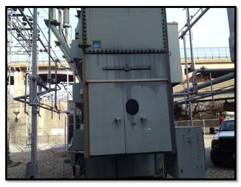
Photo #21 View of transformer, note blue "Non-PCB" label.
