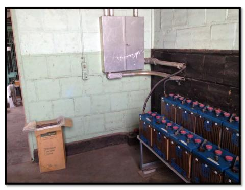
Photo #31 Backup battery storage of 2229 Spring Grove Avenue. First Floor.
