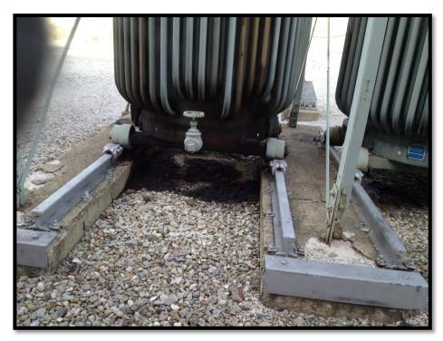
Photo #17 View of oil staining beneath transformers.
