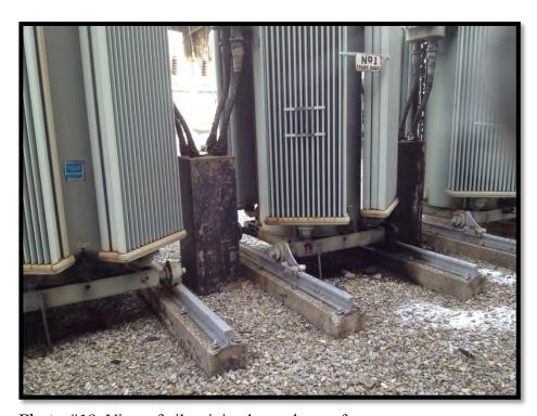
Photo #18 View of oil staining beneath transformers.
