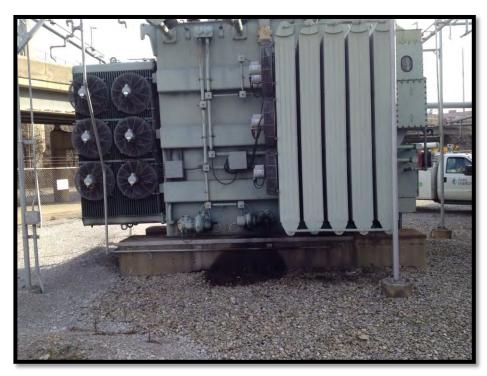
Photo #19 View of control panel and transformer, note staining.
