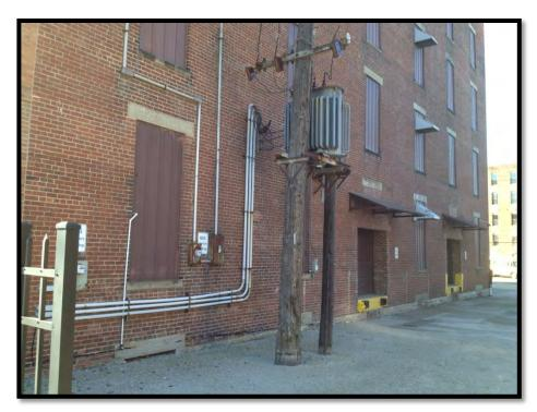
Photo #4 View of pole-mounted transformer located on north side of building at 2201 Spring Grove Avenue.
