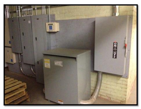
Photo #9 View of electrical panels and pad-mounted transformer located in basement of 2201 Spring Grove Avenue.
