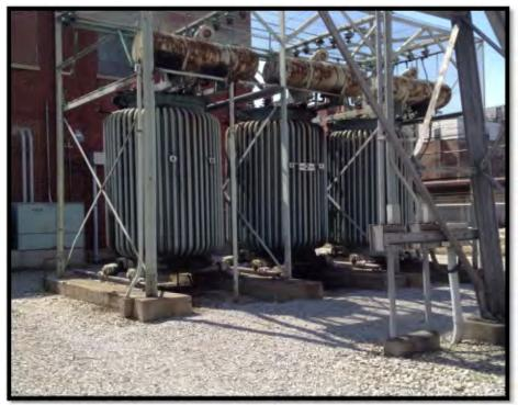
Photo #17 Transformers located in substation yard.
