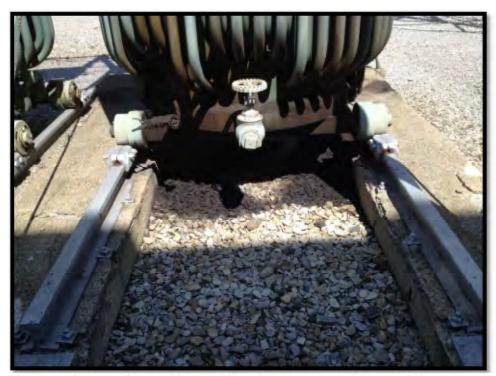
Photo #10 Transformers located in substation yard. Note staining.
