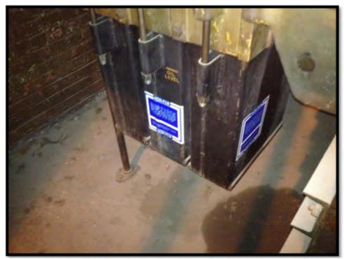
Photo #27 Blue NON-PCB label located on circuit breakers on 1<sup>st</sup> floor of building.
