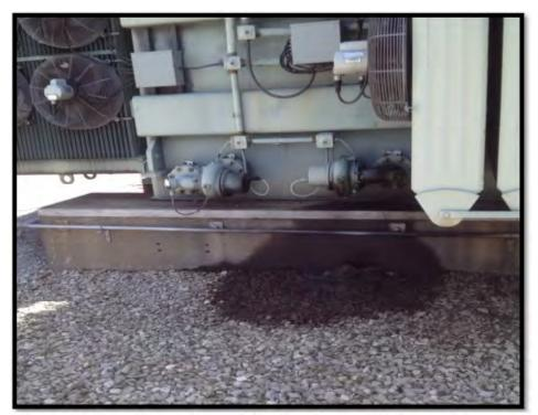
Photo #14 Transformers located in substation yard. Note staining.
