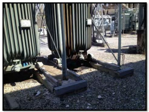
Photo #9 Transformers located in substation yard. Note staining.
