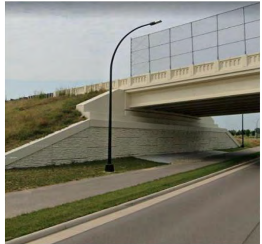
Concrete girder example
