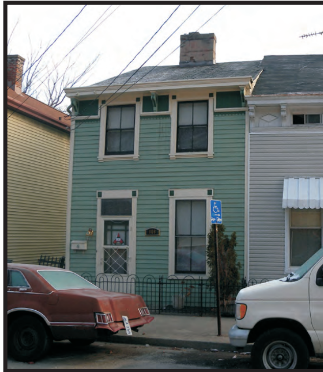
Plate A28. View of KY-123, 806 Crescent Avenue, facing east.
