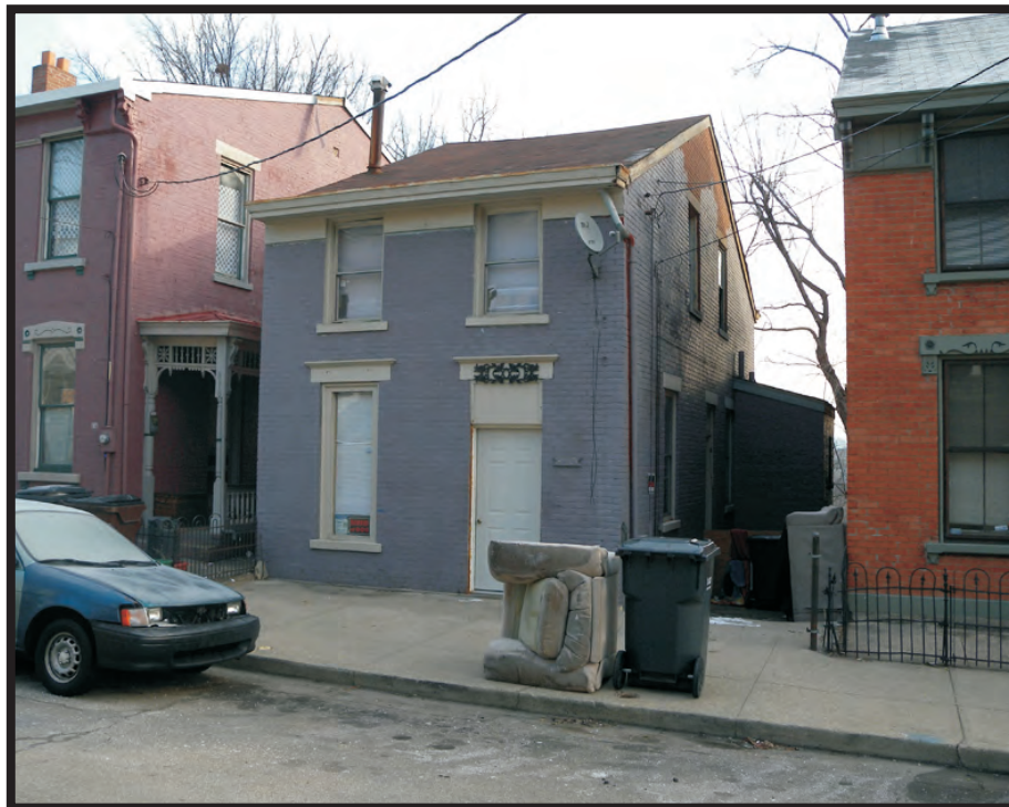
Plate A23. View of KY-117, 820 Crescent Avenue, facing northeast.
