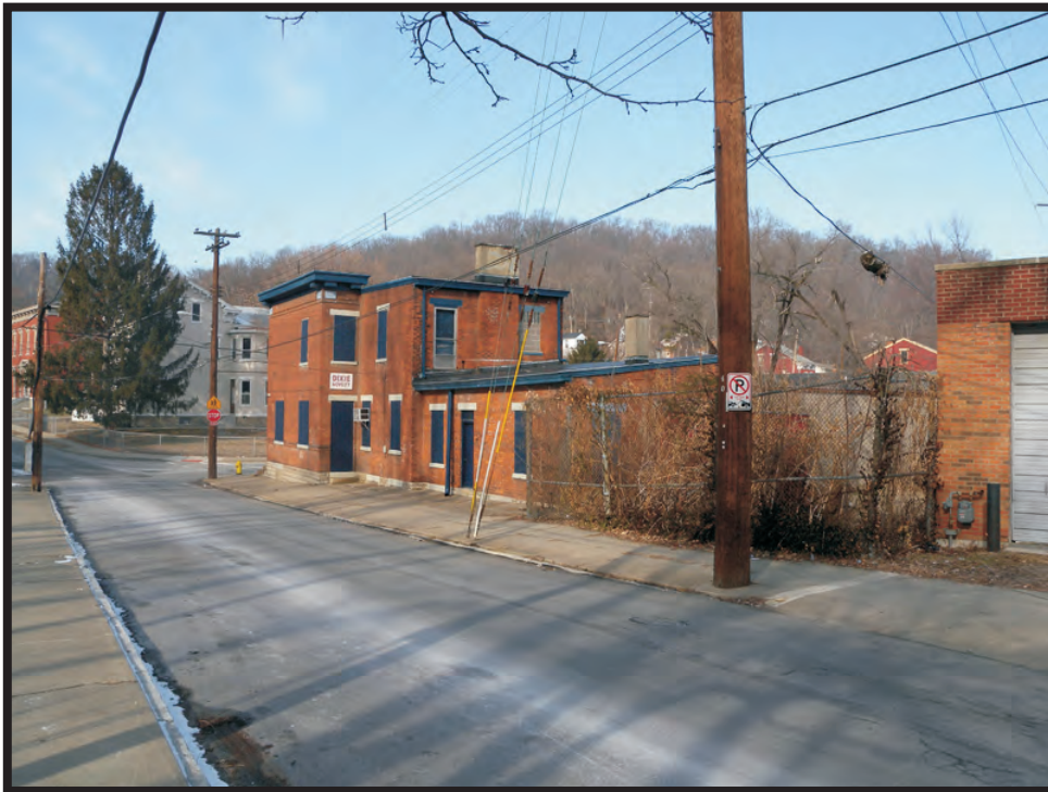
Plate A16. View of KY-73, 636-640 Lewis Street, facing west.
