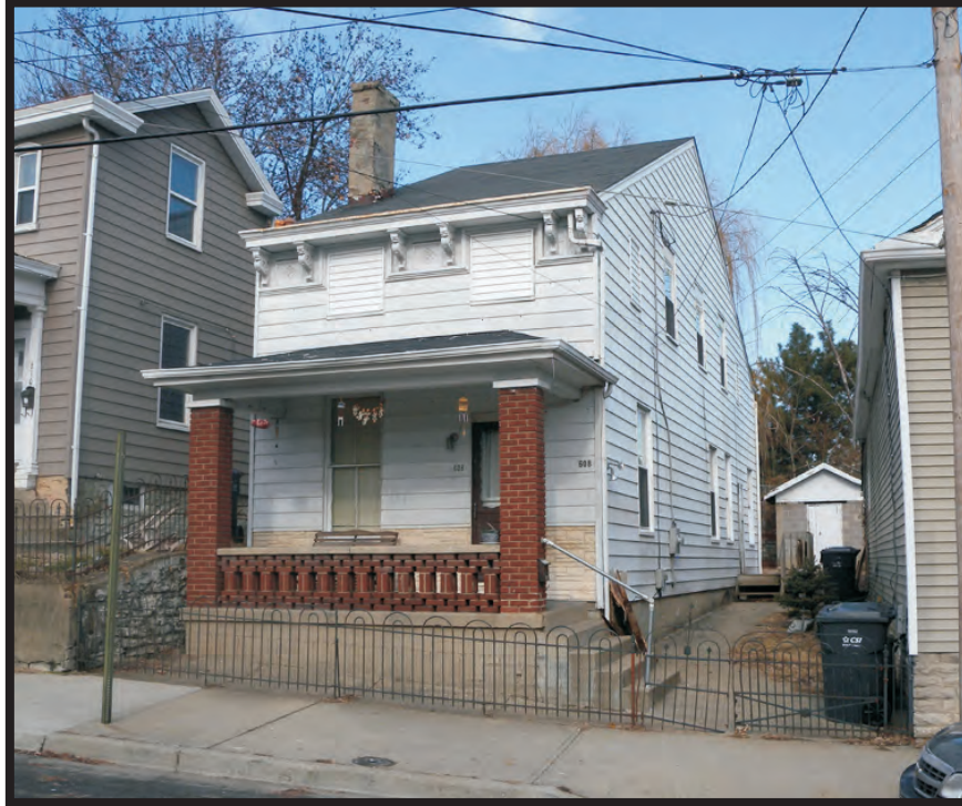
Plate A9. View of KY-56, 608 West 11th Street, facing northwest.
