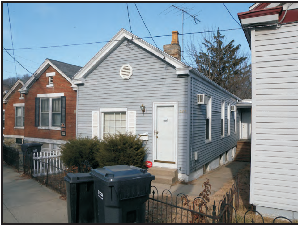
Plate A12. View of KY-68, 624 Lewis Street, facing northwest.
