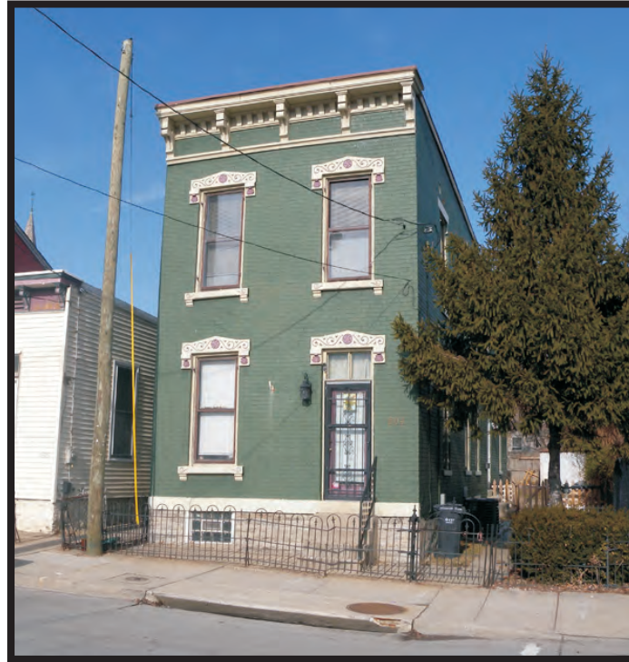
Plate A5. View of KY-52, 604 West 12th Street, facing northwest.
