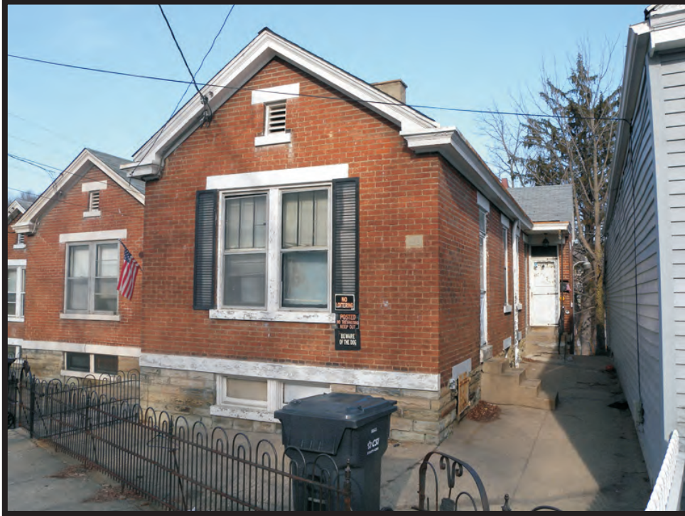
Plate A13. View of KY-69, 626 Lewis Street, facing northwest.
