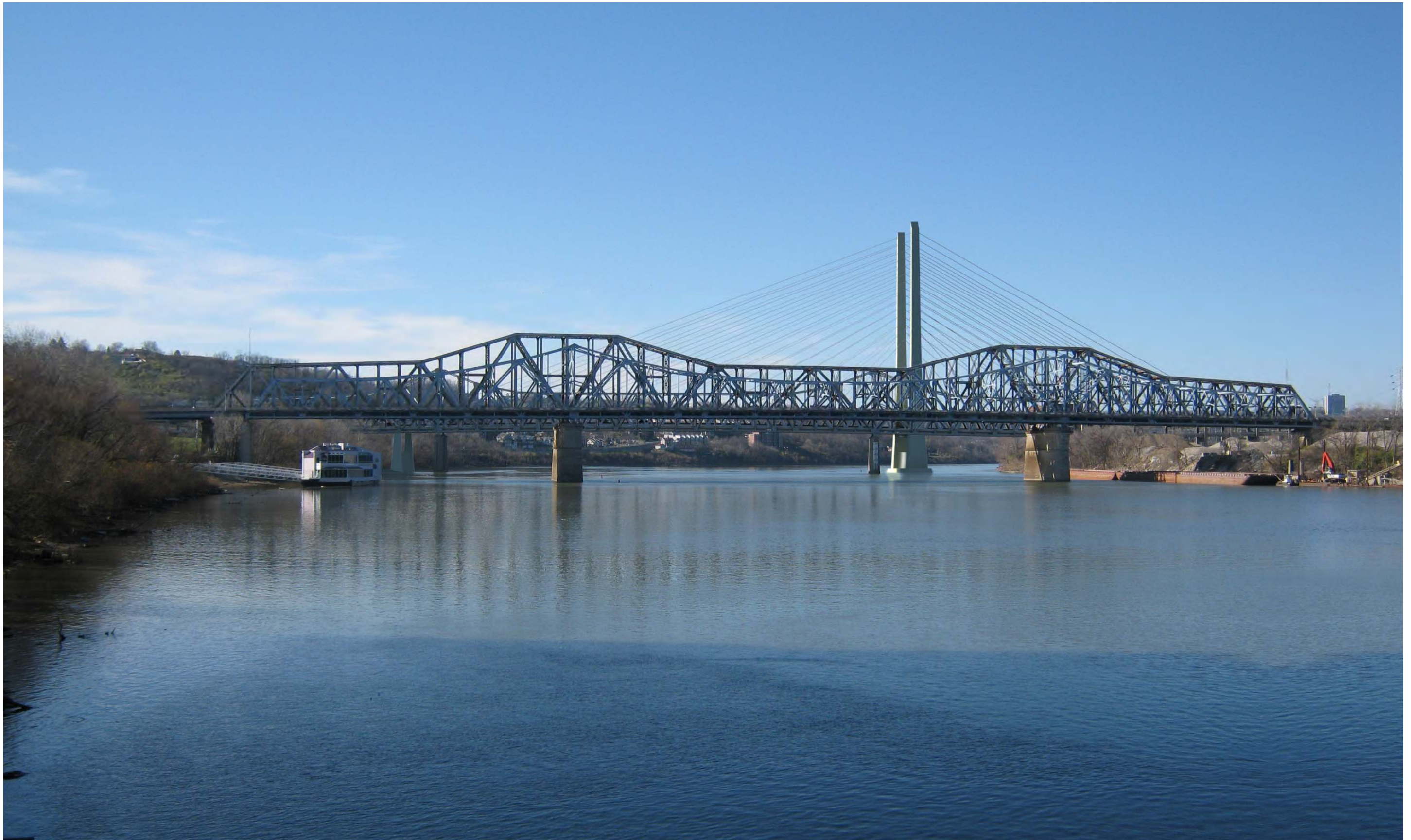
ALTERNATIVE 6 – ONE TOWER CABLE STAYED
