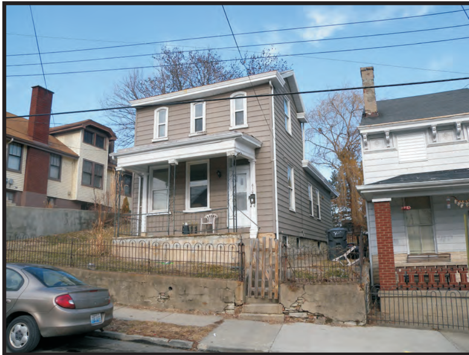
Plate A10. View of KY-57, 610 West 11th Street, facing northwest.
