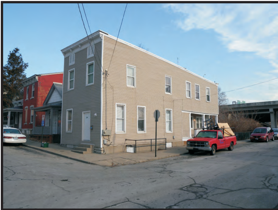
Plate A20. View of KY-96, 872 Crescent Avenue, facing northeast.
