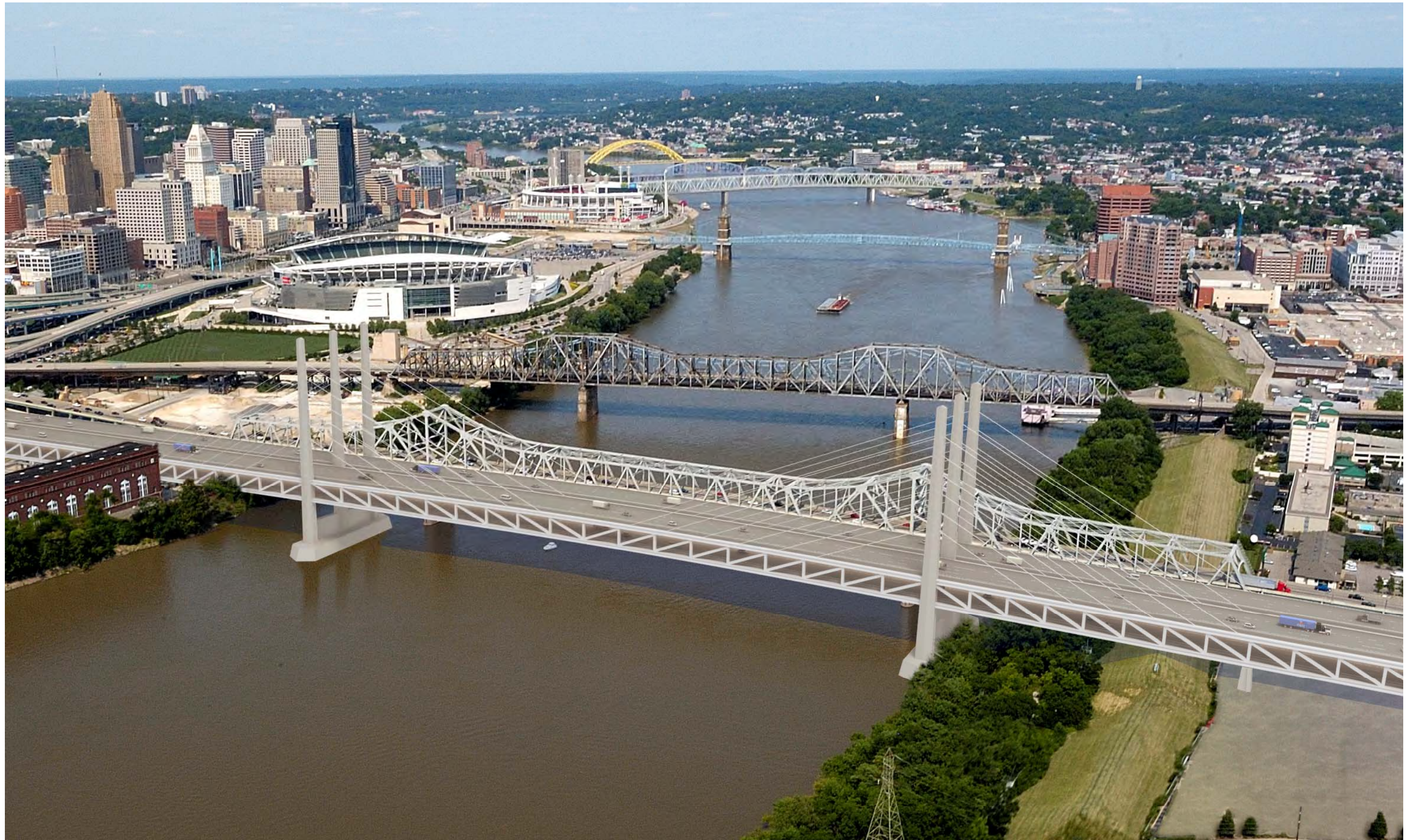
ALTERNATIVE 3 – TWO TOWER CABLE STAYED
