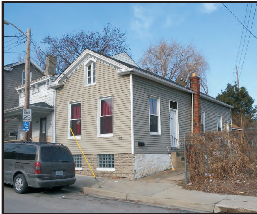
Plate A8. View of KY-55, 606 West 11th Street, facing northwest.
