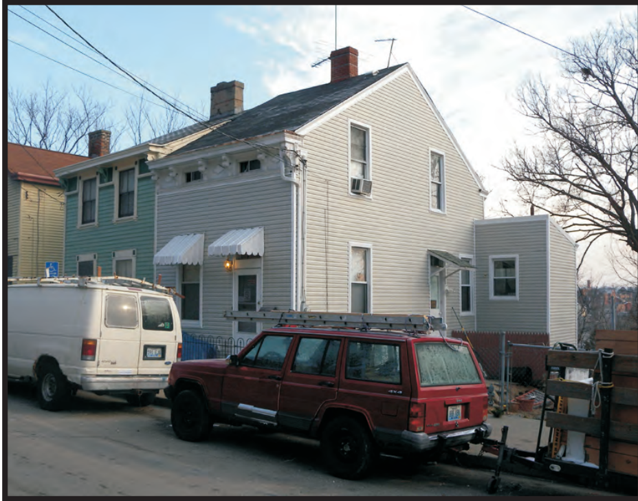
Plate A27. View of KY-122, 808 Crescent Avenue, facing northeast.
