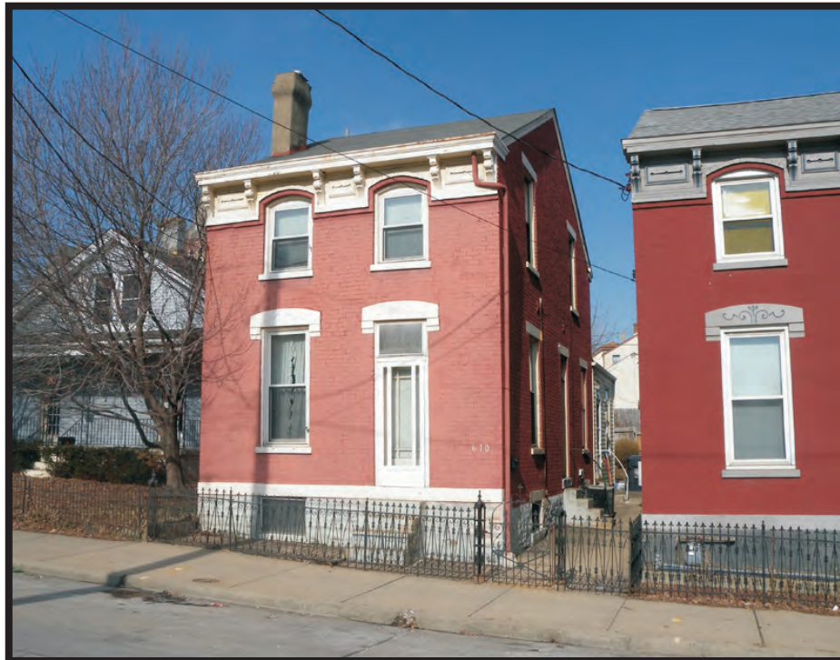
Plate A2. View of KY-49, 610 West 12th Street, facing northwest.
