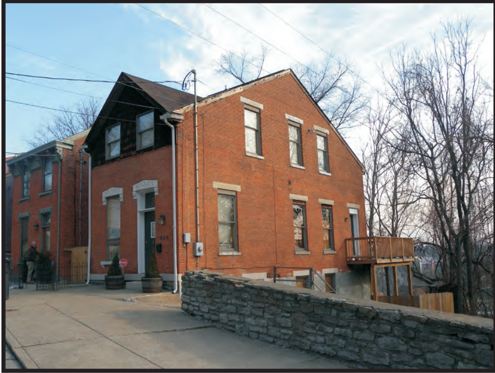
Plate A21. View of KY-115, 824 Crescent Avenue, facing northeast.
