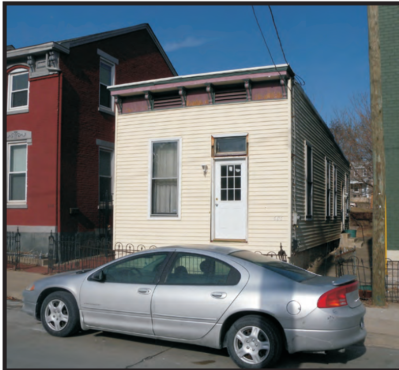
Plate A4. View of KY-51, 606 West 12th Street, facing northwest.
