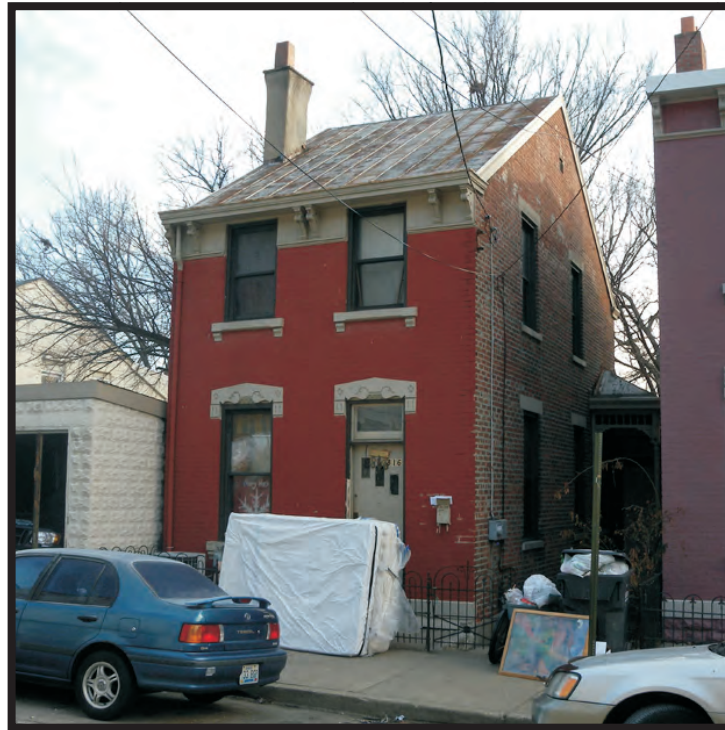
Plate A25. View of KY-119, 816 Crescent Avenue, facing northeast.
