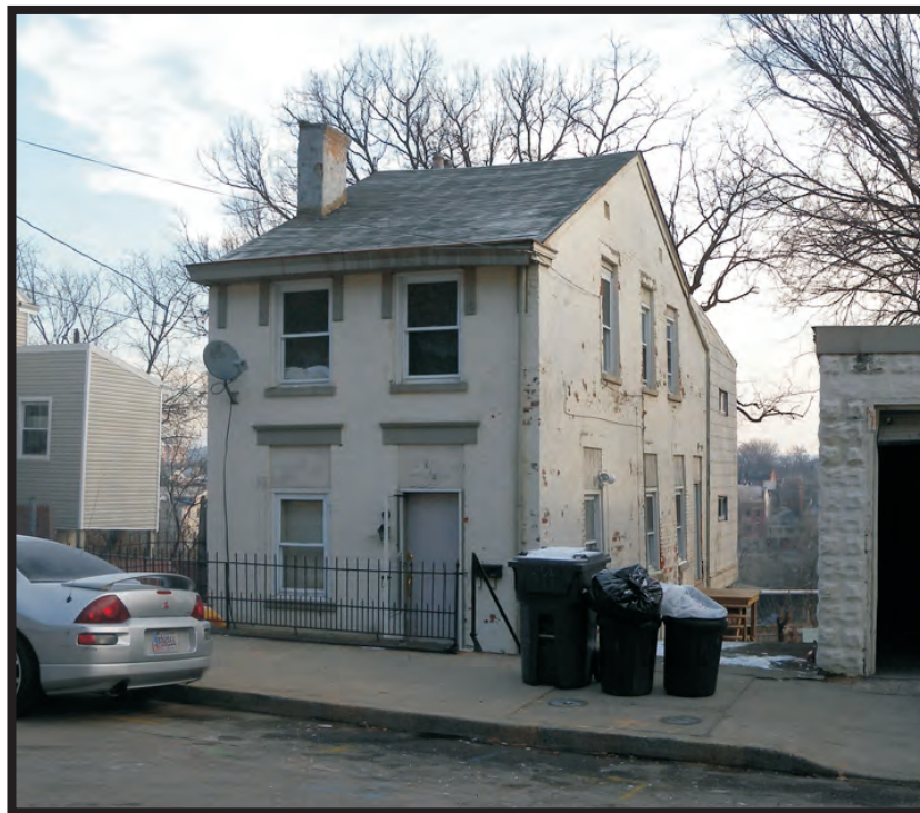
Plate A26. View of KY-120, 812 Crescent Avenue, facing northeast.
