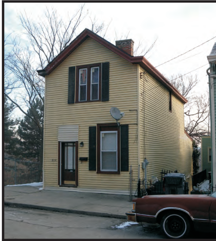
Plate A29. View of KY-124, 804 Crescent Avenue, facing northeast.
