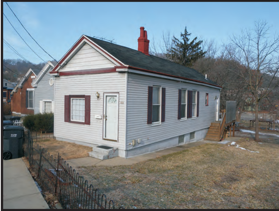
Plate A11. View of KY-67, 622 Lewis Street, facing northwest.
