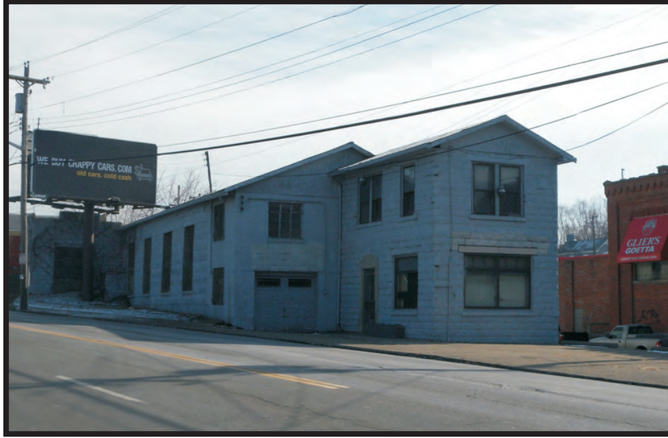
Plate A31. View of 511-519 Pike Street, facing southeast.
