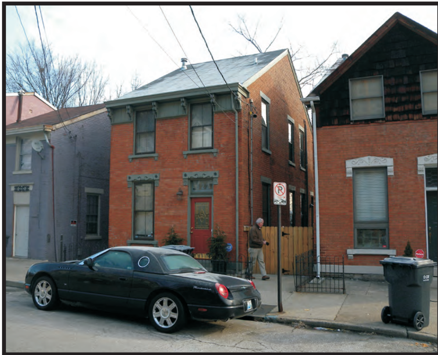
Plate A22. View of KY-116, 822 Crescent Avenue, facing northeast.
