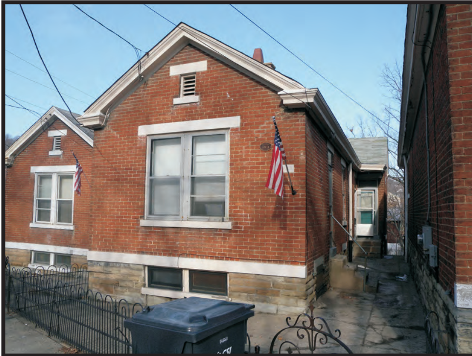
Plate A14. View of KY-70, 628 Lewis Street, facing northwest.
