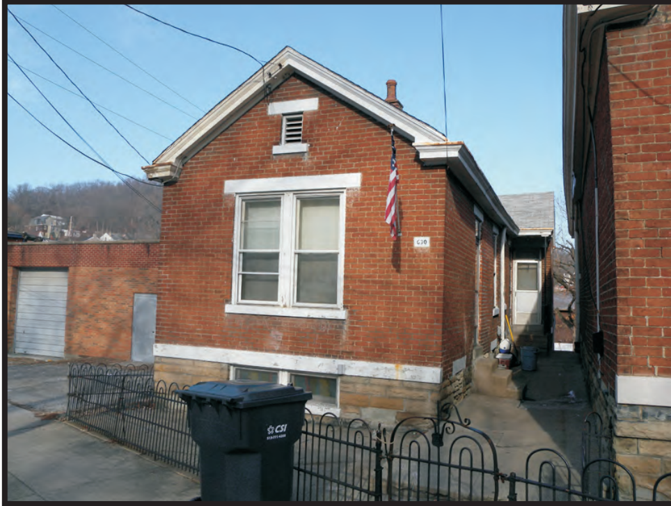
Plate A15. View of KY-71, 630 Lewis Street, facing northwest.
