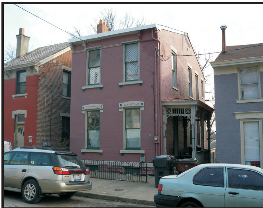
Plate A24. View of KY-118, 818 Crescent Avenue, facing northeast.
