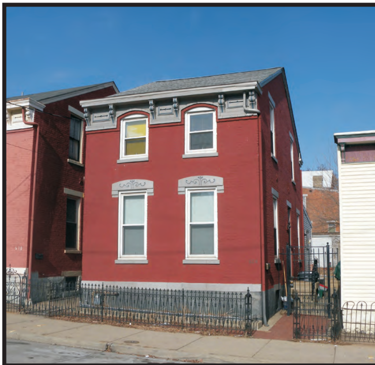
Plate A3. View of KY-50, 608 West 12th Street, facing northwest.
