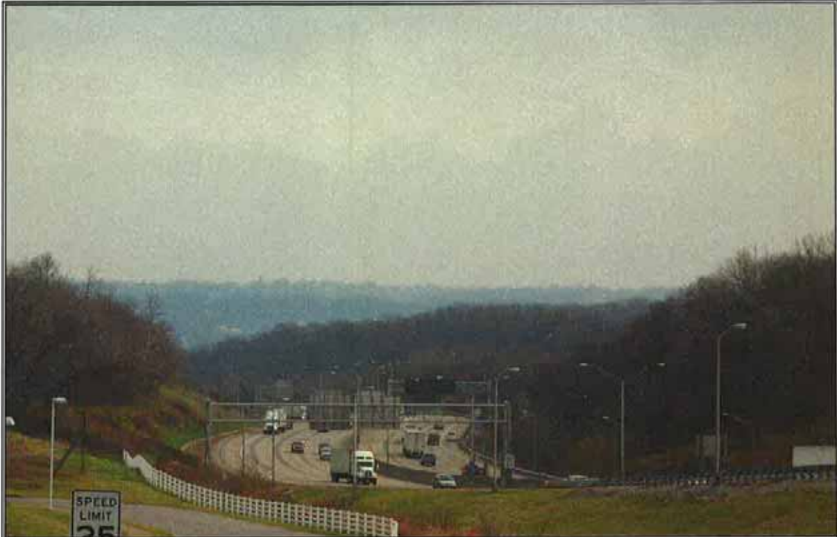
Photograph 1: General view of I-75/I-71 study area from near the Kyles Lane overpass looking northeast. Brent Spence Bridge Replacement and Rehabilitation Project. November 29, 2006.
