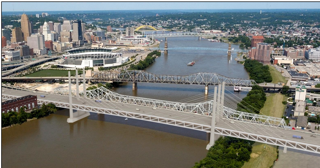
Alternative 3: Two Tower Cable Stayed Bridge
