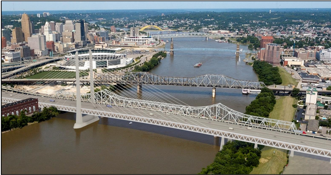
Alternative 6: One Tower Cable Stayed Bridge
