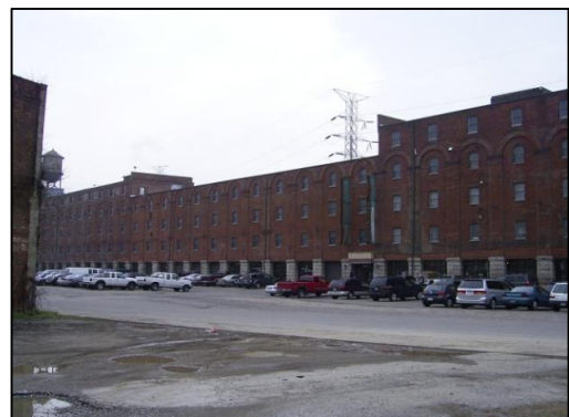
View of Longworth Hall
