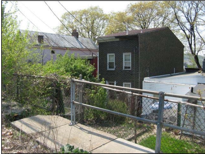
Residential Structures Along Central Parkway (rear view, to be impacted)
