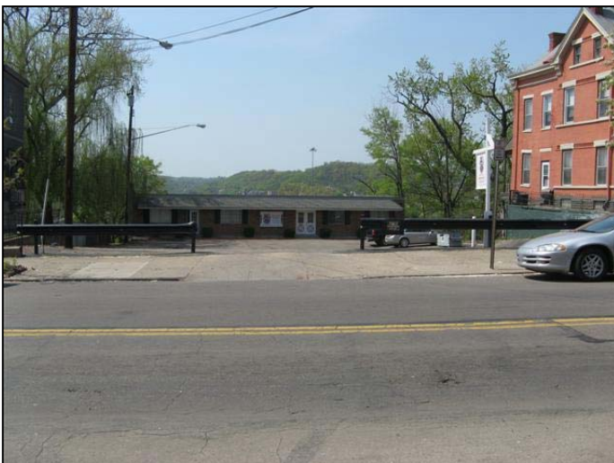
Property To Be Impacted Along McMicken
