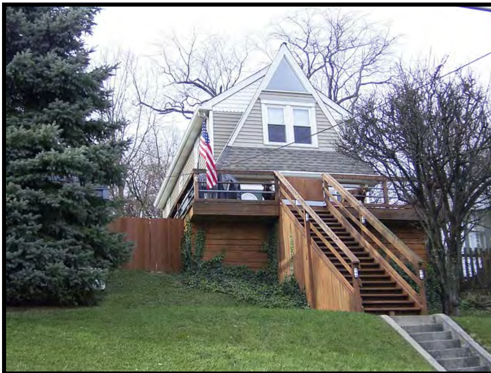
Plate 51. View of 411 Western Avenue, facing west.
