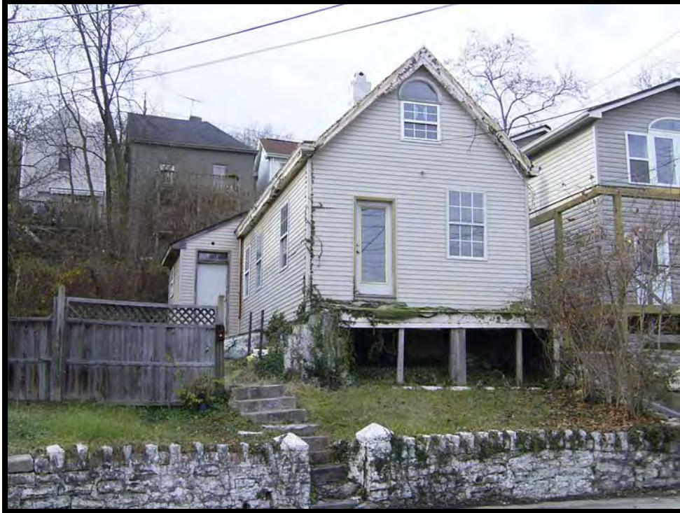
Plate 82. View of 637 Crescent Avenue, facing west.
