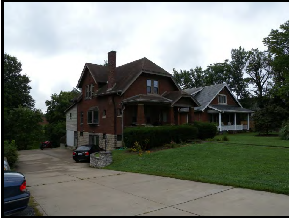
Plate 129. View of 2045 Dixie Highway, facing south.
