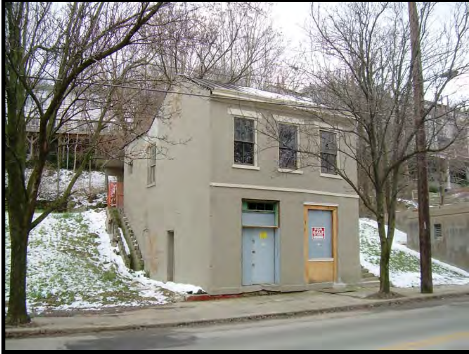
Plate 36. View of 841 Highway Avenue, facing southwest.
