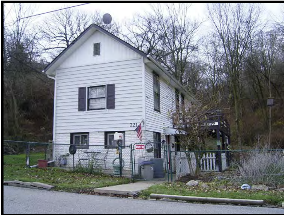
Plate 45. View of 321 Western Avenue, facing west.
