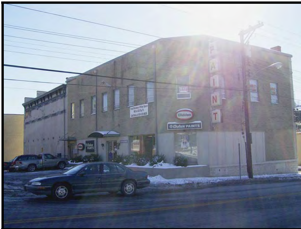
Plate 12. View of 533 Pike Street (KECL 817), facing southwest.
