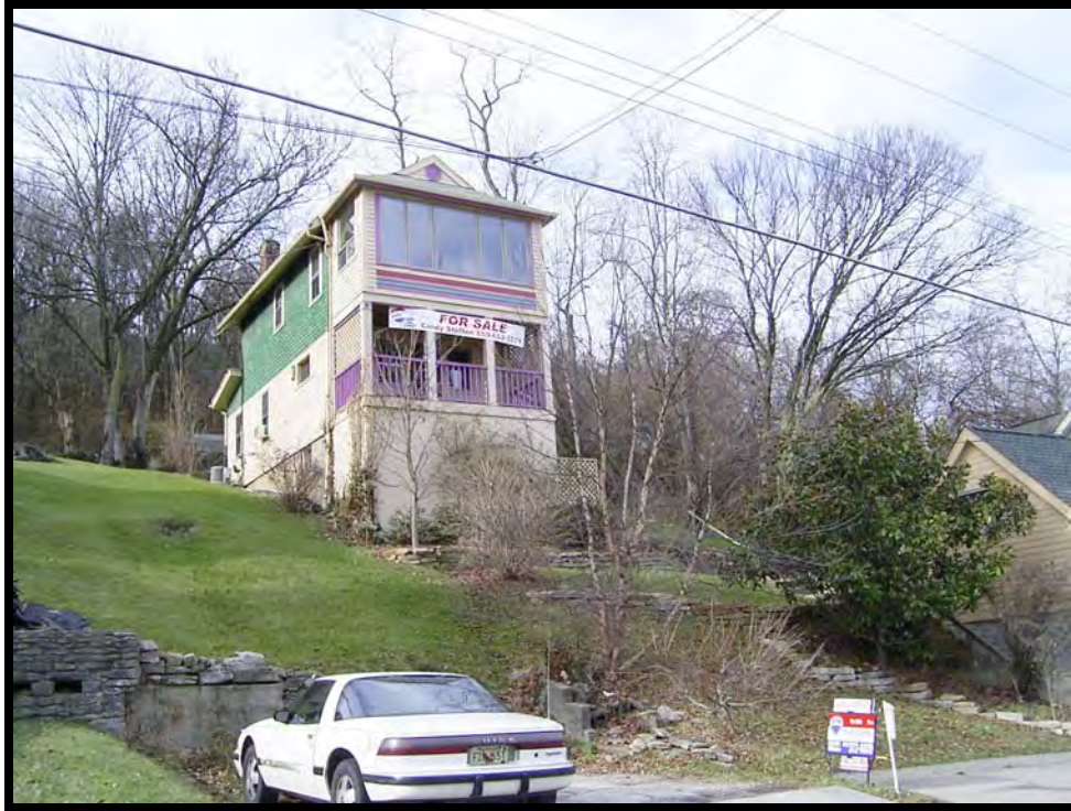
Plate 53. View of 507 Western Avenue, facing west.
