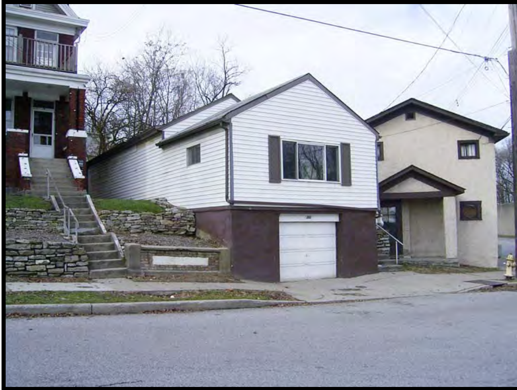
Plate 38. View of 203 Western Avenue, facing west.
