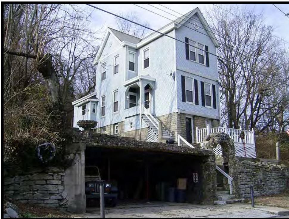
Plate 44. View of 223 Western Avenue, facing west.
