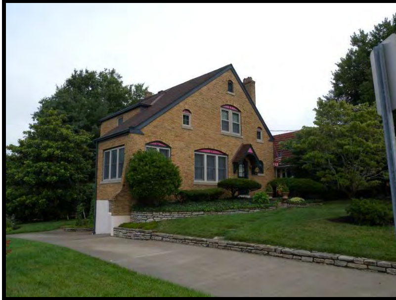
Plate 111. View of 15 Leslie Avenue, facing north.
