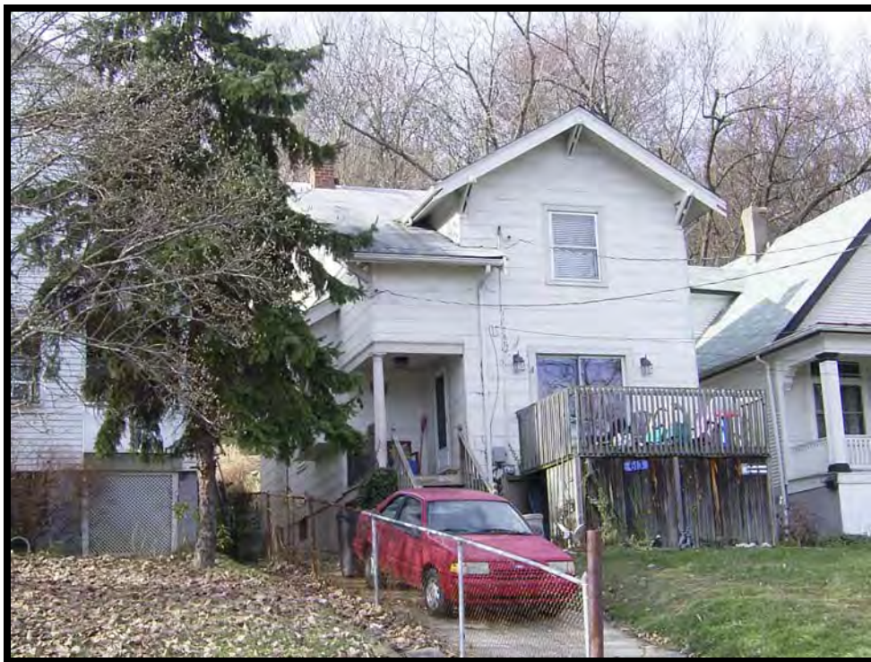
Plate 63. View of 613 Western Avenue, facing west.
