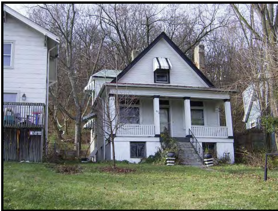
Plate 62. View of 611 Western Avenue, facing west.
