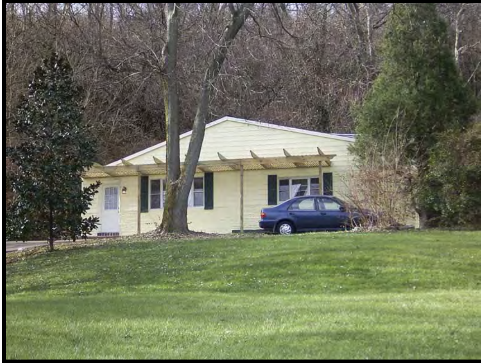
Plate 70. View of 635 Western Avenue, facing west.
