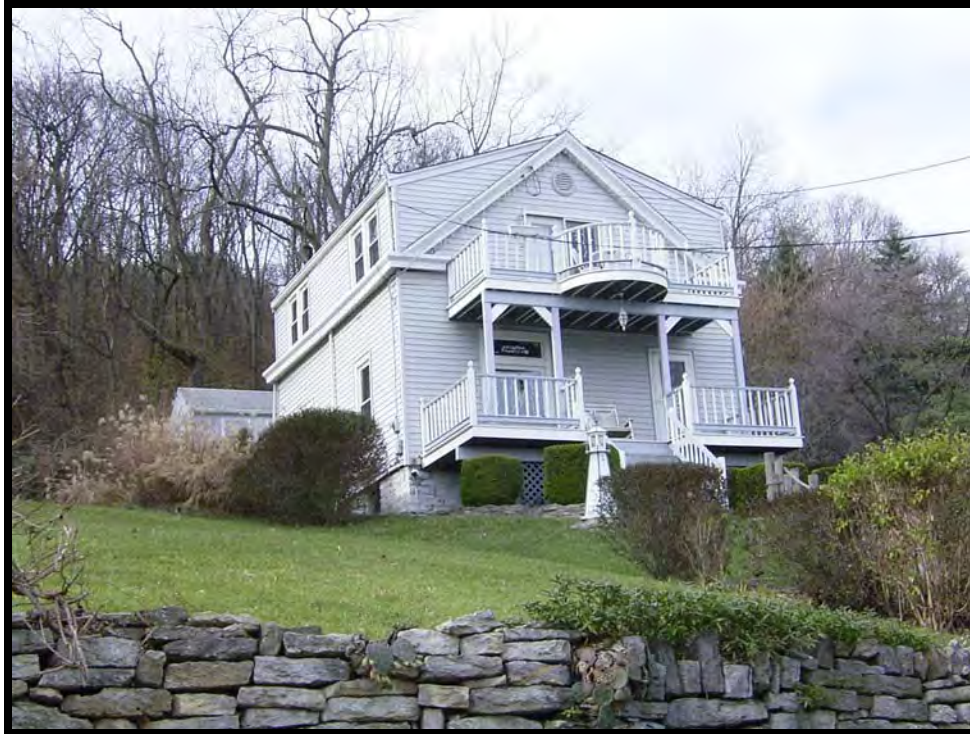
Plate 55. View of 517 Western Avenue, facing west.
