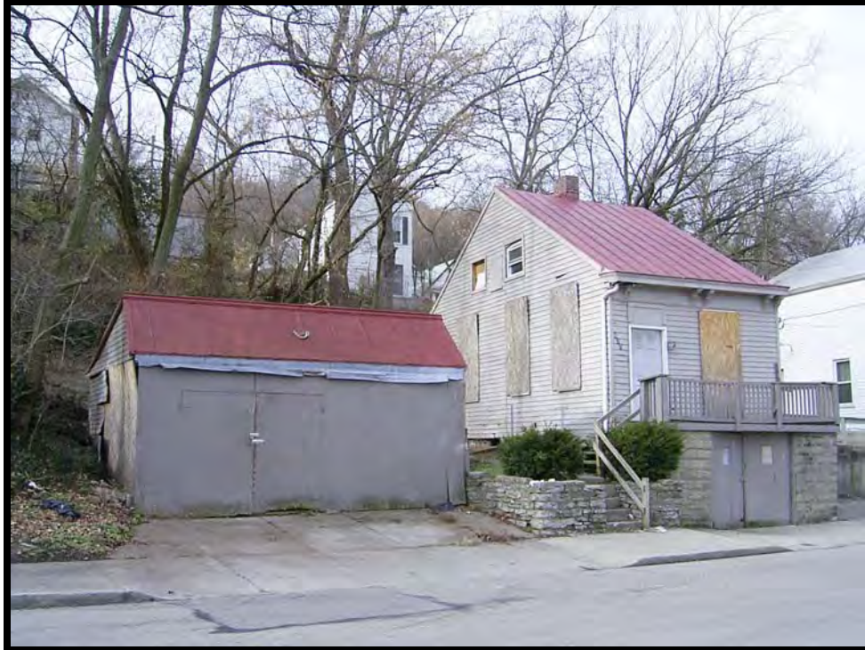
Plate 80. View of 625 Crescent Avenue, facing west.
