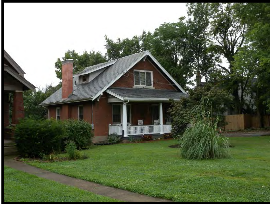
Plate 130. View of 2049 Dixie Highway, facing south.
