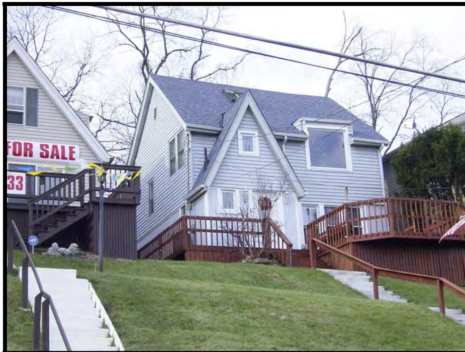
Plate 48. View of 405 Western Avenue, facing west.
