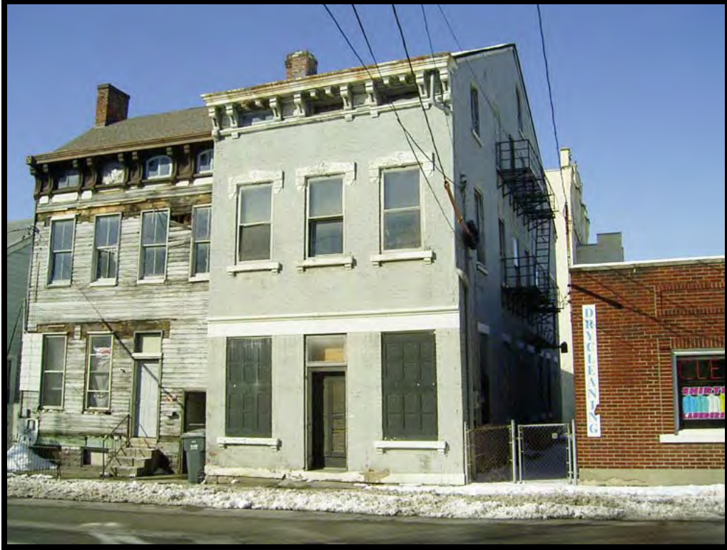
Plate 8. View of 504 West 12th Street (KECL 621), facing north.
