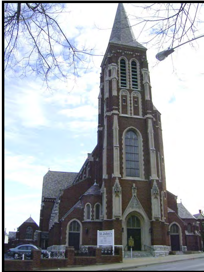
Plate 24. View of St. John's Church, within the Lewisburg Historic District, facing south.
