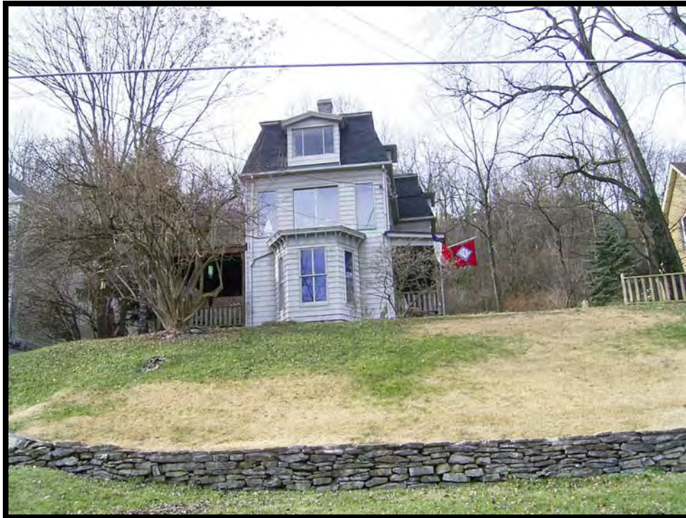
Plate 57. View of 527 Western Avenue, facing west.
