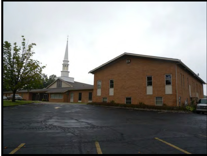
Plate 92. View of 2006 Pieck Drive, facing west.
