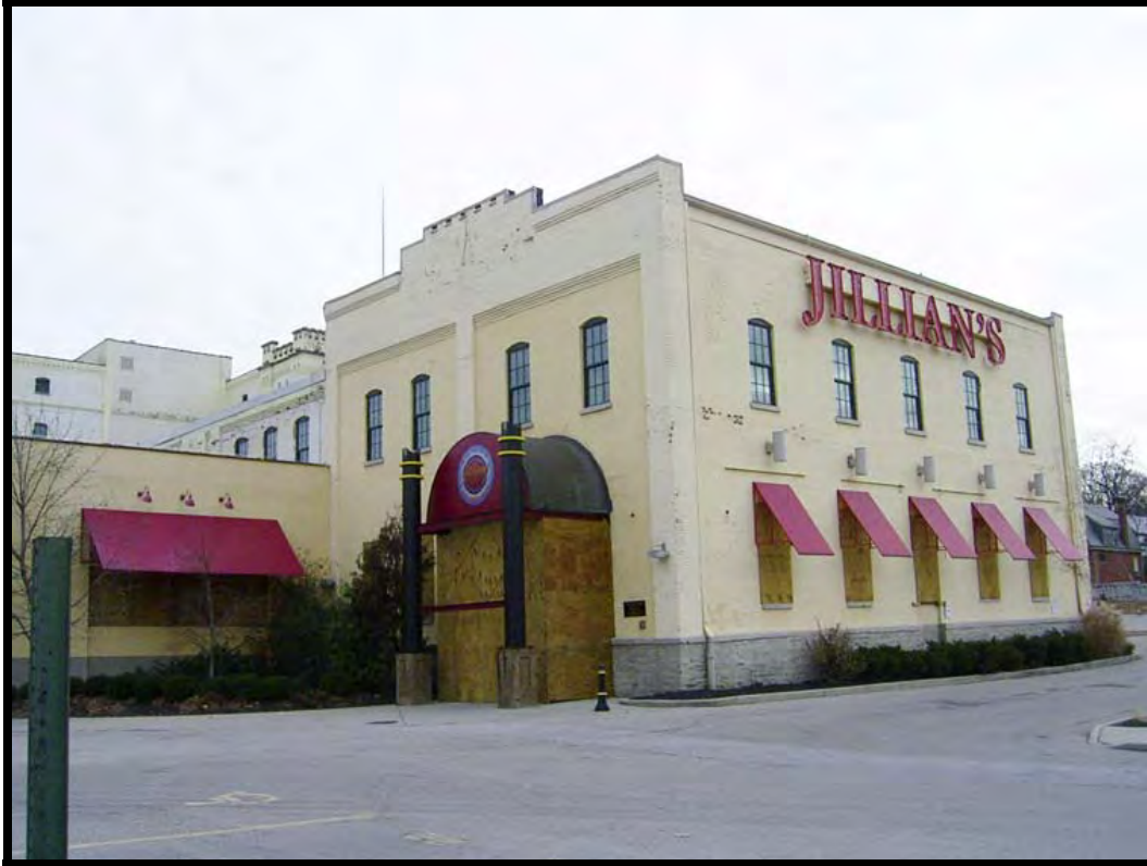
Plate 26. View of Bavarian Brewing Company (NRHP No. 96000281), facing southeast.
