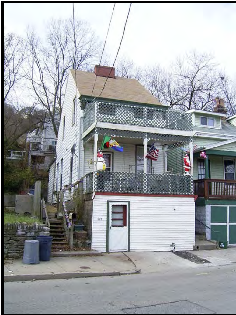
Plate 75. View of 605 Crescent Avenue, facing west.
