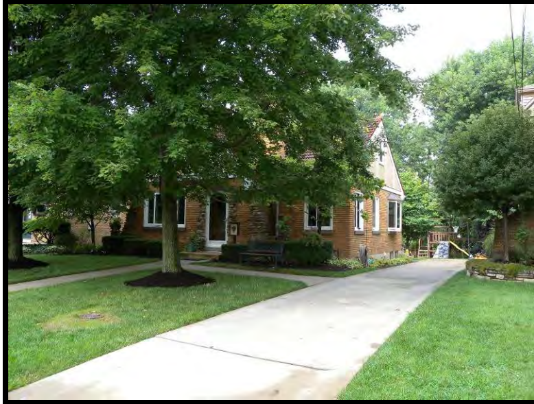
Plate 112. View of 13 Leslie Avenue, facing west.
