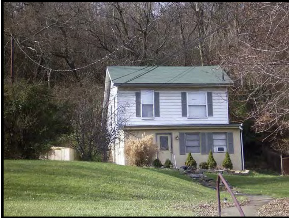
Plate 69. View of 633 Western Avenue, facing west.
