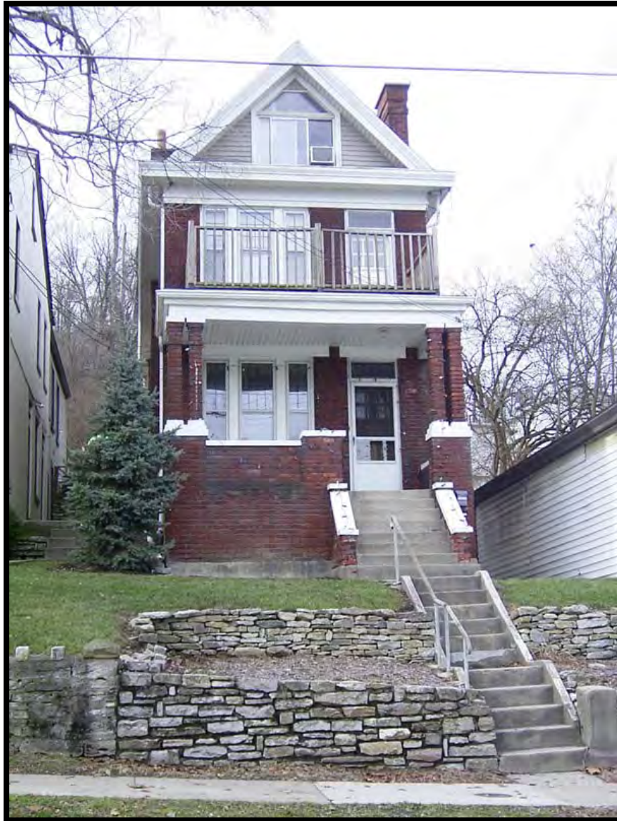
Plate 39. View of 205 Western Avenue, facing west.
