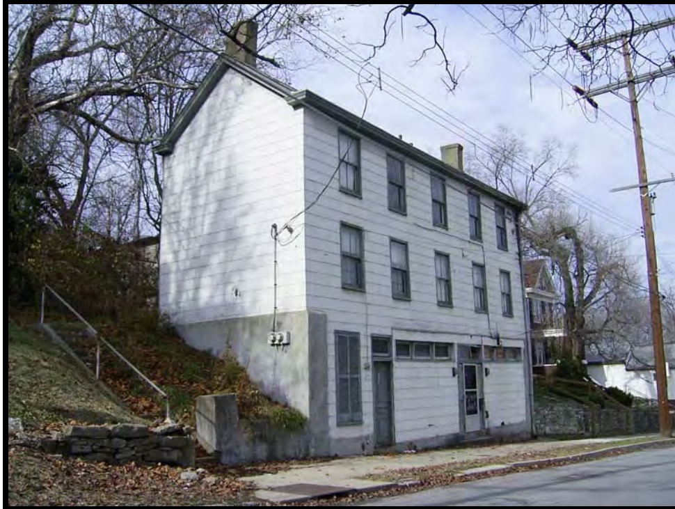
Plate 43. View of 213 Western Avenue, facing west.
