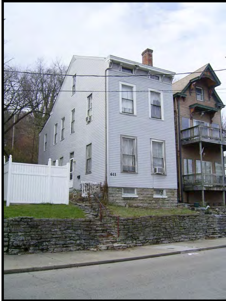
Plate 77. View of 611 Crescent Avenue, facing west.
