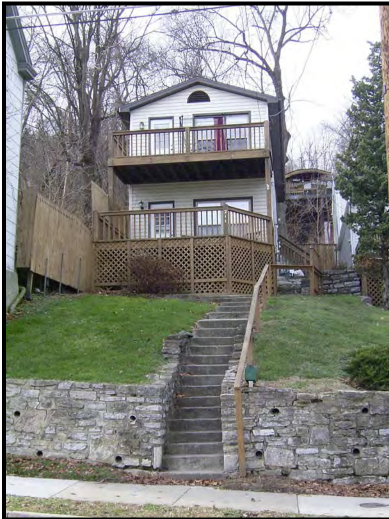
Plate 42. View of 211 Western Avenue, facing west.
