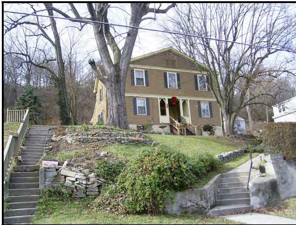
Plate 56. View of 521 Western Avenue, facing west.
