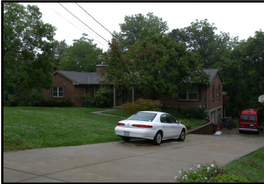
Plate 90. View of 1999 Pieck Drive, facing east.
