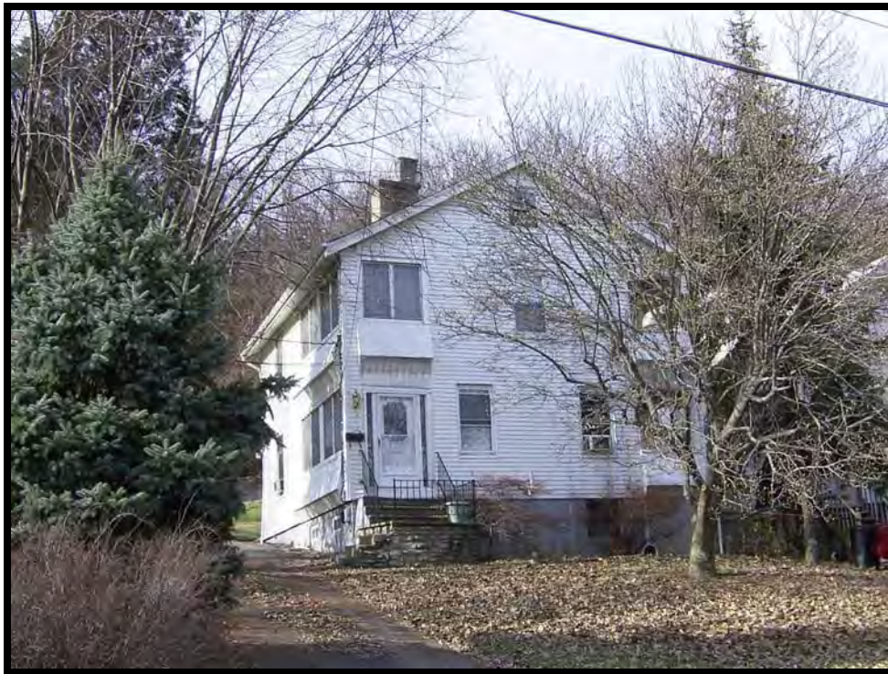
Plate 65. View of 619 Western Avenue, facing west.
