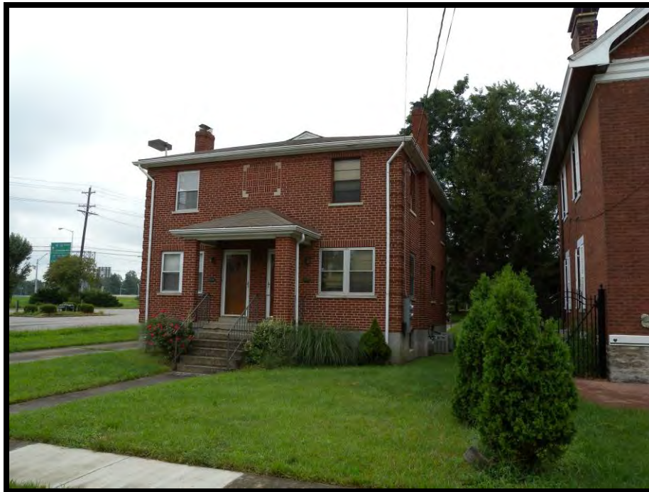
Plate 132. View of 15-17 West Maple Avenue, facing south.
