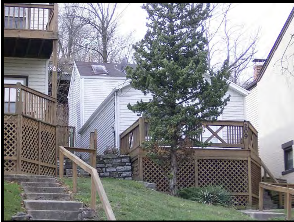
Plate 41. View of 209 Western Avenue, facing west.
