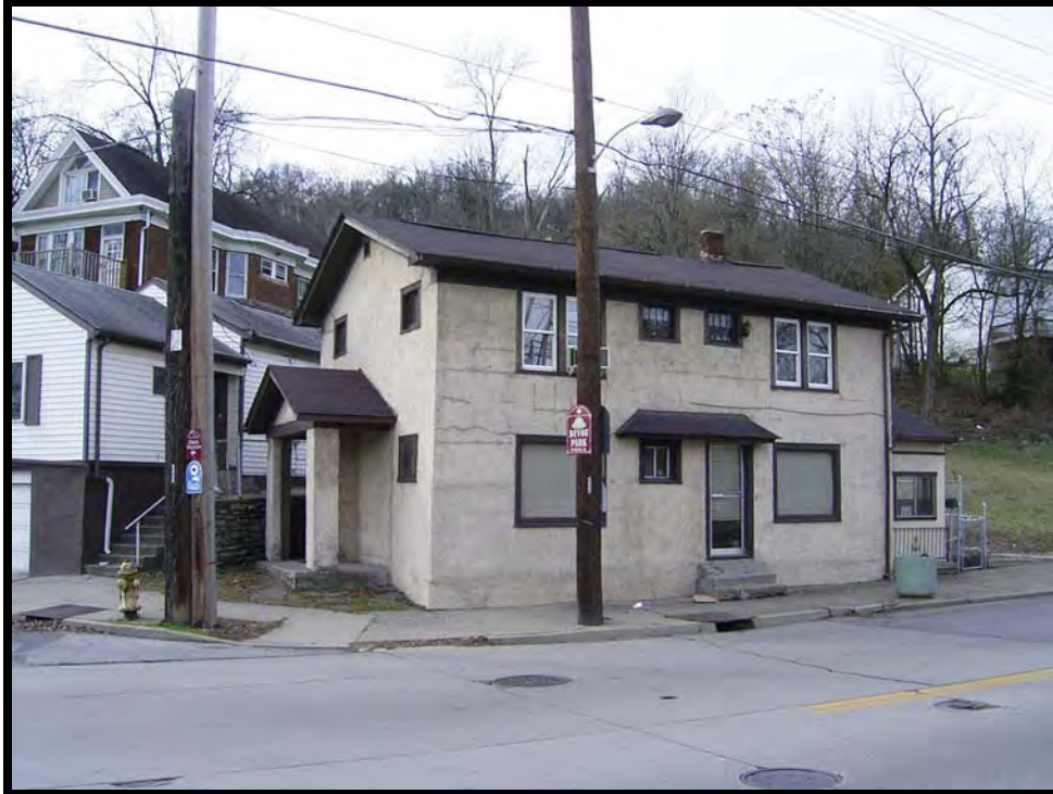
Plate 35. View of 801 Highway Avenue, facing southwest.
