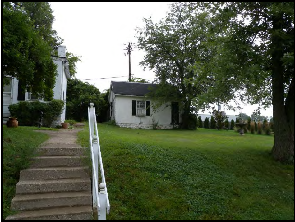
Plate 121. View of 2 East Orchard Road, outbuilding, facing northeast.
