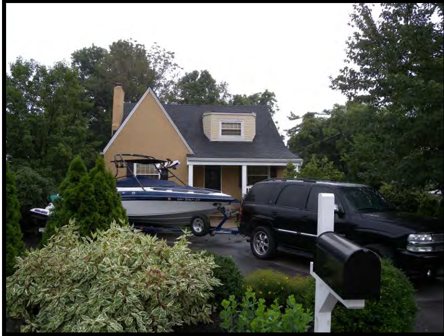
Plate 96. View of 2009 Pieck Drive, facing southeast.
