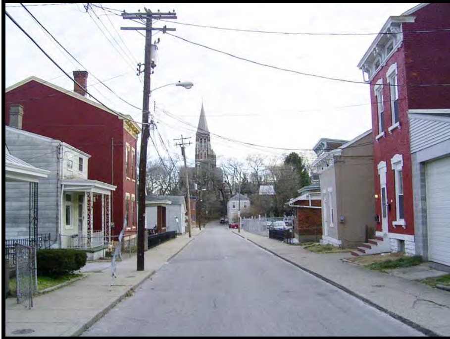
Plate 23. View of Baker Street, within the Lewisburg Historic District (NRHP No. 93001165), facing south.
