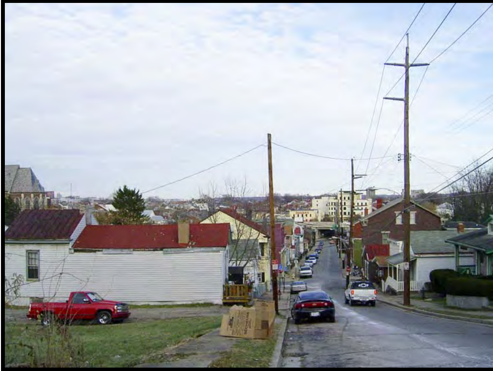
Plate 21. View of West 12 th Street, within the Lewisburg Historic District (NRHP No. 93001165), facing east.
