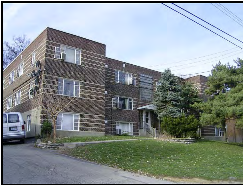
Plate 87. View of 509 St. Joseph Lane, facing northwest.
