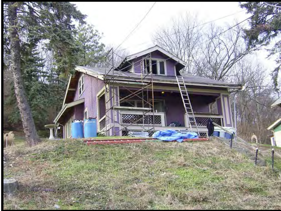
Plate 54. View of 511 Western Avenue, facing west.
