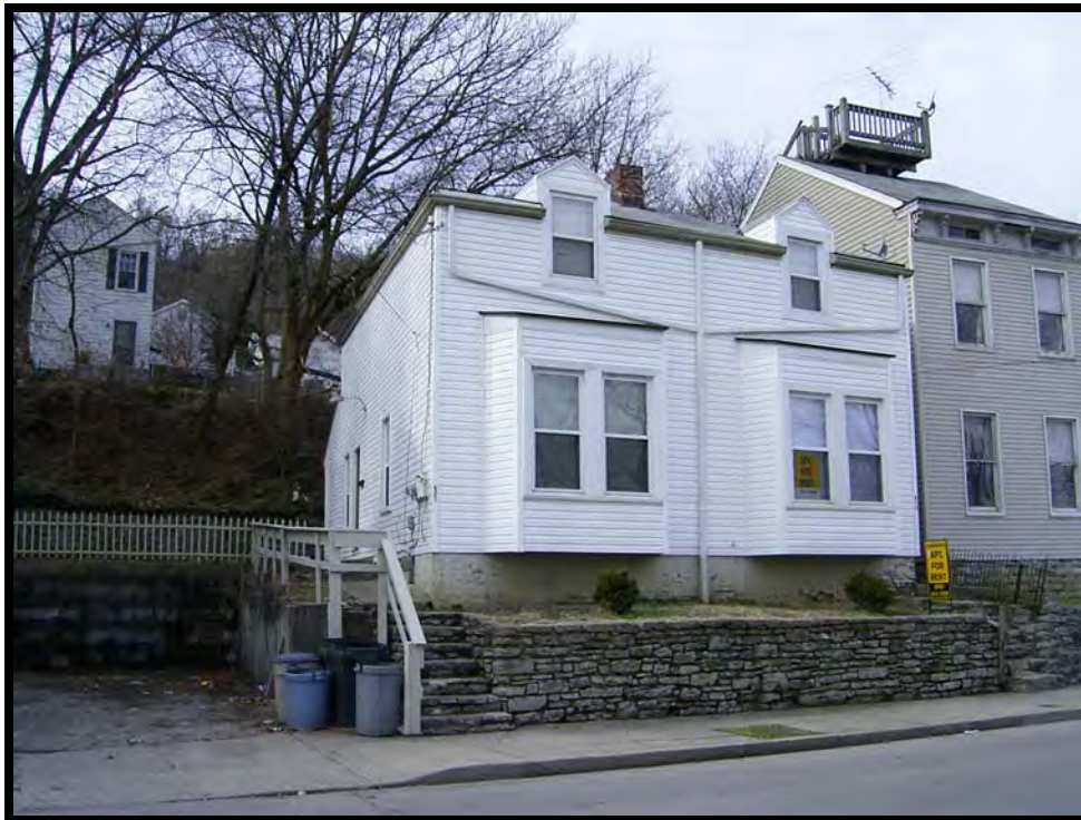
Plate 79. View of 619-621 Crescent Avenue, facing west.
