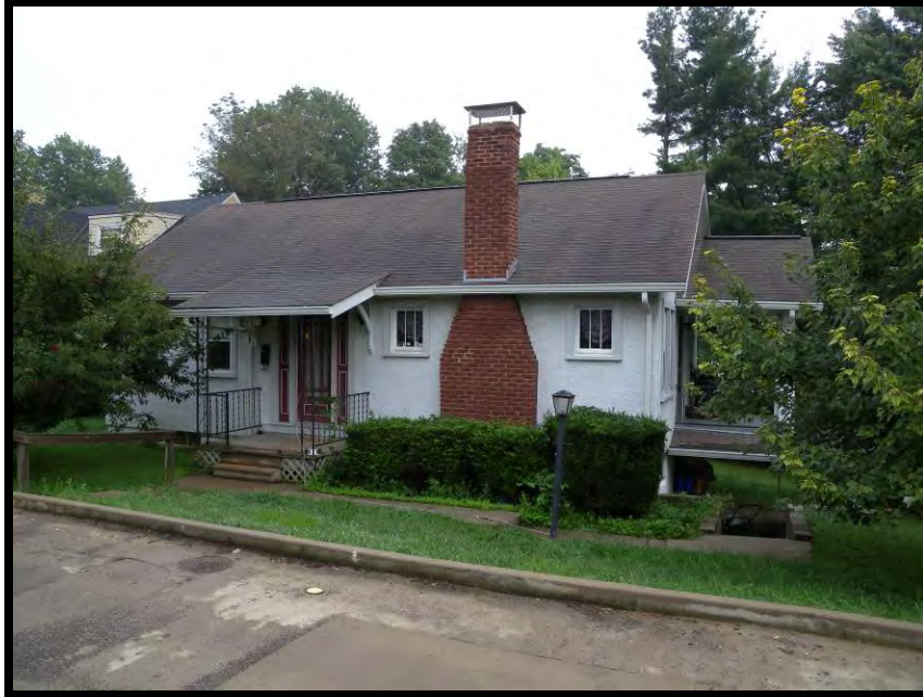
Plate 97. View of 2011 Pieck Drive, facing east.
