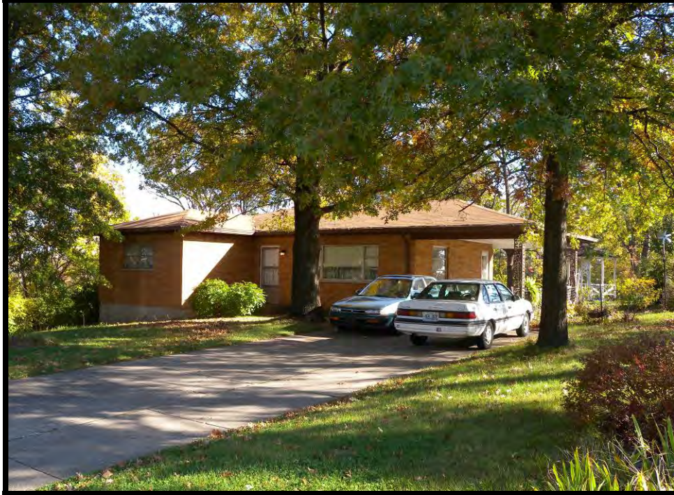
Plate 138. View of 216 Ana Jo Lane, facing northeast.
