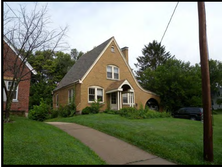
Plate 116. View of 5 Leslie Avenue, facing west.
