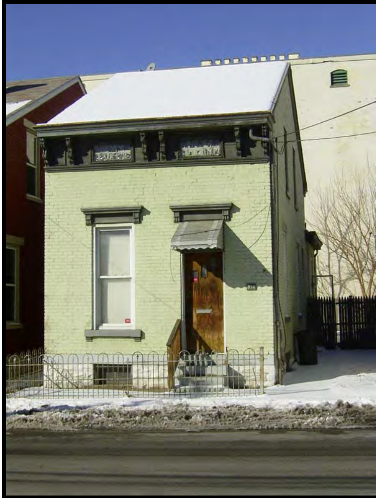
Plate 9. View of 514 West 12th Street (KECL 626), facing north.
