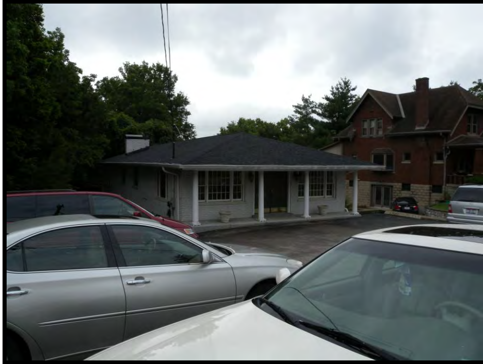
Plate 128. View of 2039 Dixie Highway, facing south.
