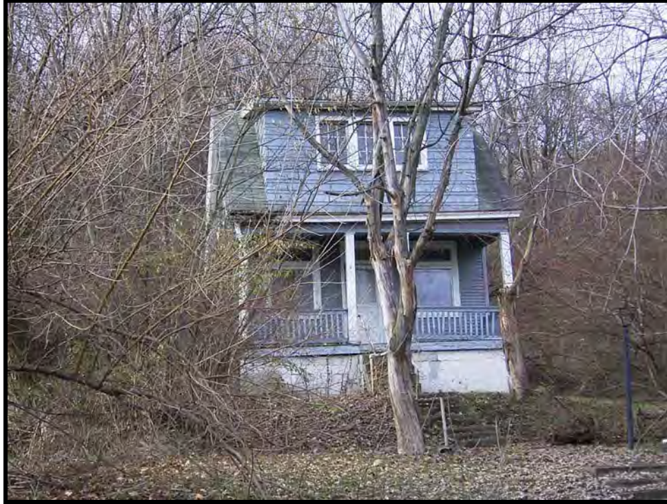
Plate 61. View of 609 Western Avenue, facing west.
