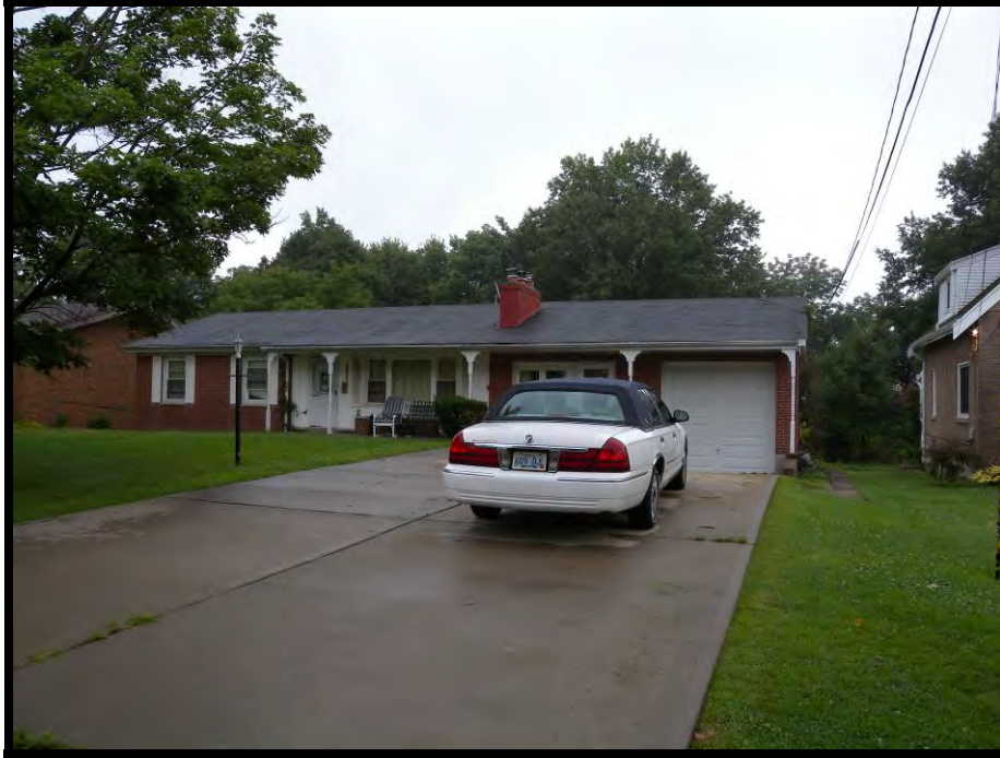
Plate 94. View of 2005 Pieck Drive, facing southeast.
