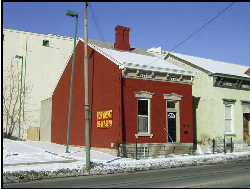
Plate 10. View of 516 West 12th Street (KECL 628), facing north.
