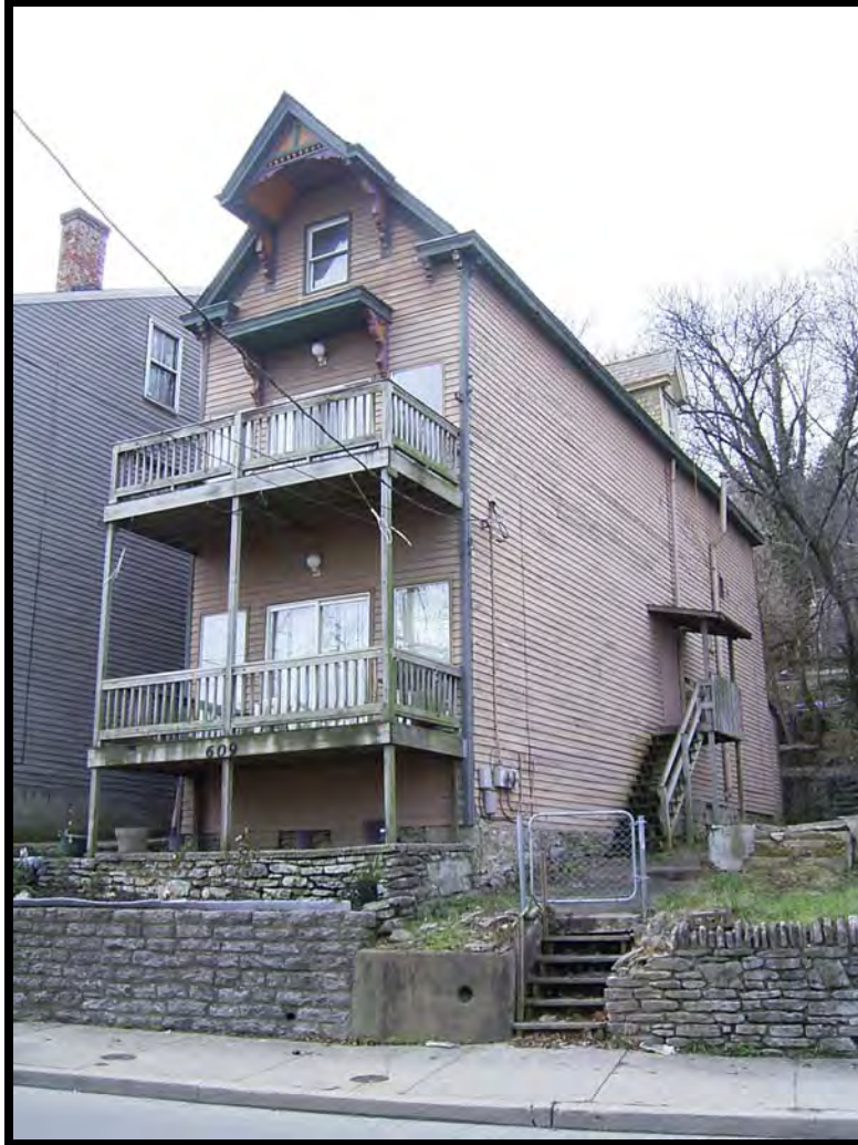
Plate 76. View of 609 Crescent Avenue, facing west.
