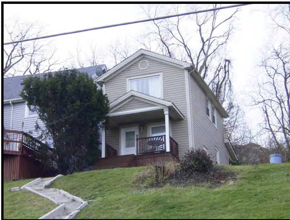
Plate 47. View of 401 Western Avenue, facing west.
