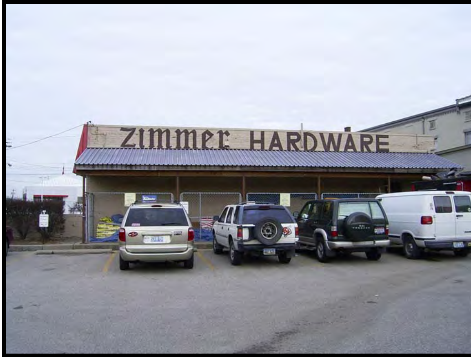
Plate 84. View of Zimmer Hardware, facing north.
