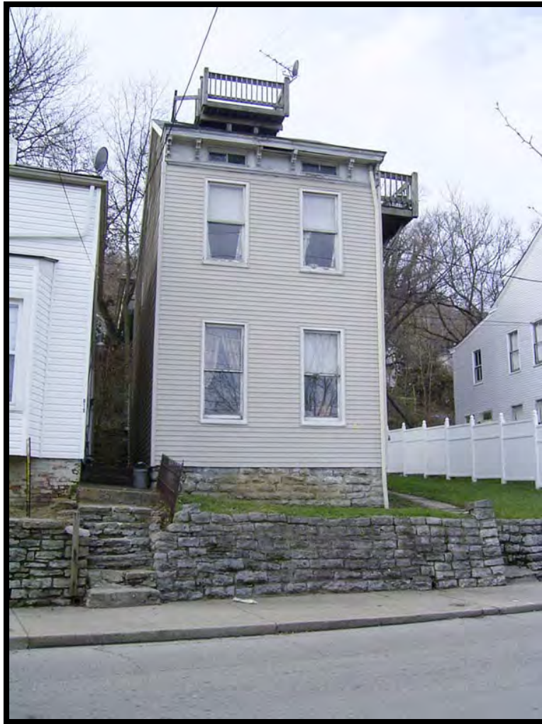
Plate 78. View of 617 Crescent Avenue, facing west.
