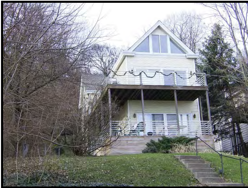
Plate 60. View of 607 Western Avenue, facing west.
