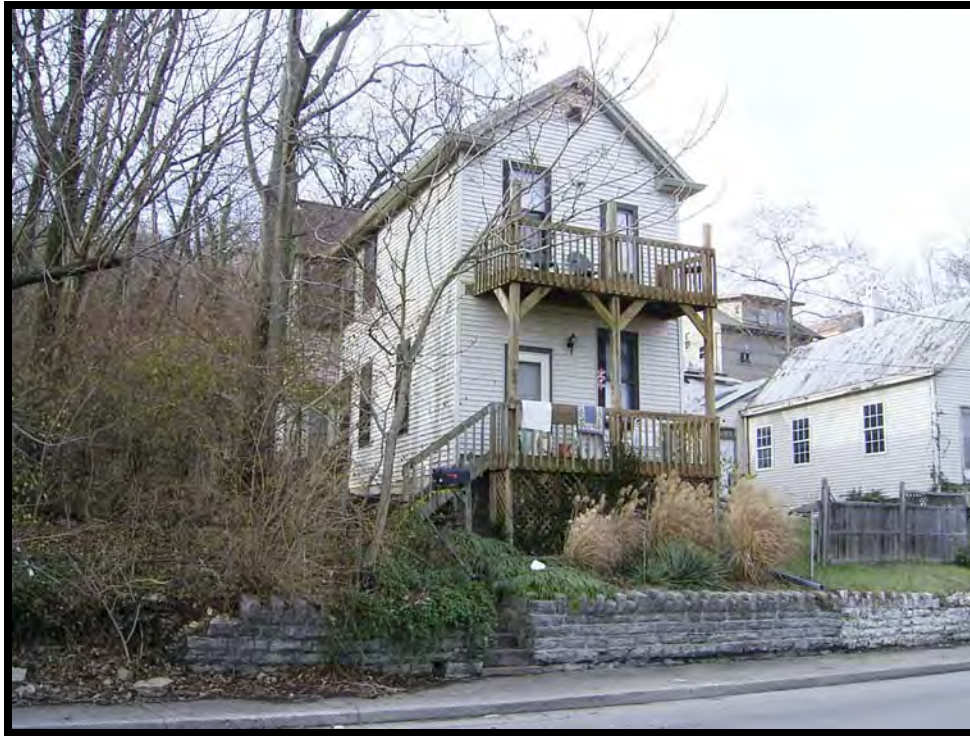
Plate 83. View of 641 Crescent Avenue, facing west.
