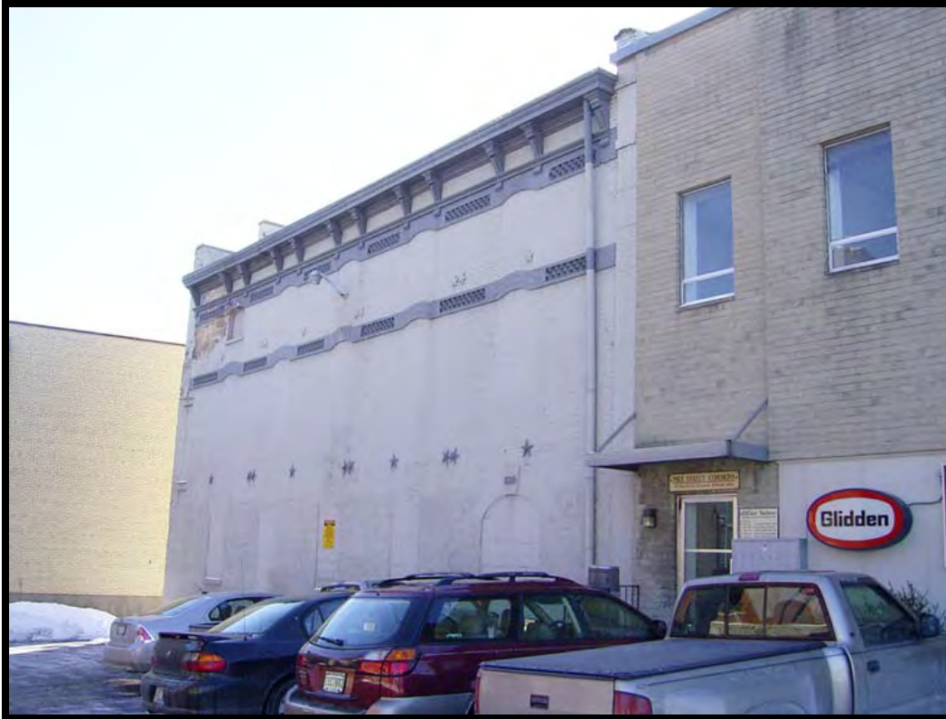
Plate 11. View of 533 Pike Street (KECL 817), facing south.
