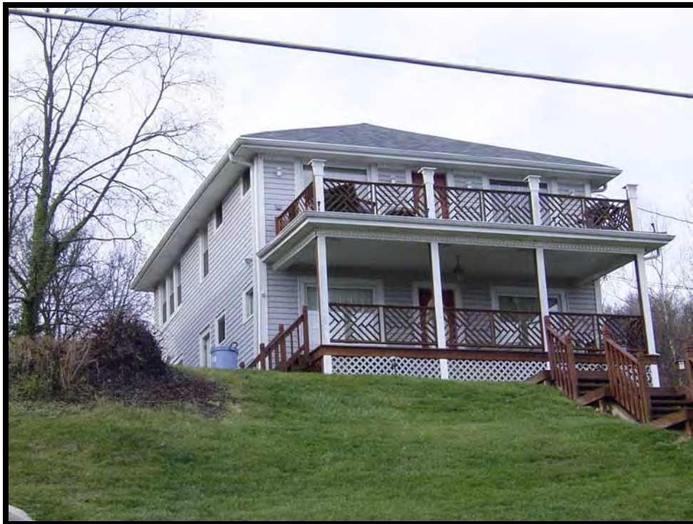
Plate 46. View of 333 Western Avenue, facing west.
