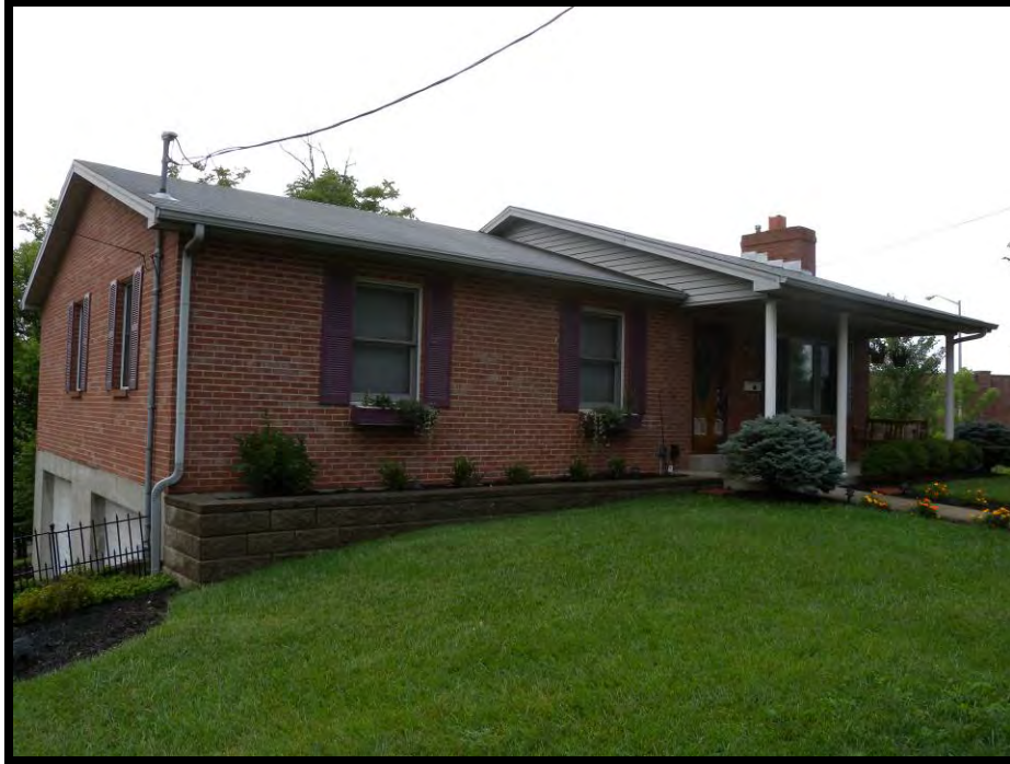
Plate 110. View of 4 Leslie Avenue, facing southeast.
