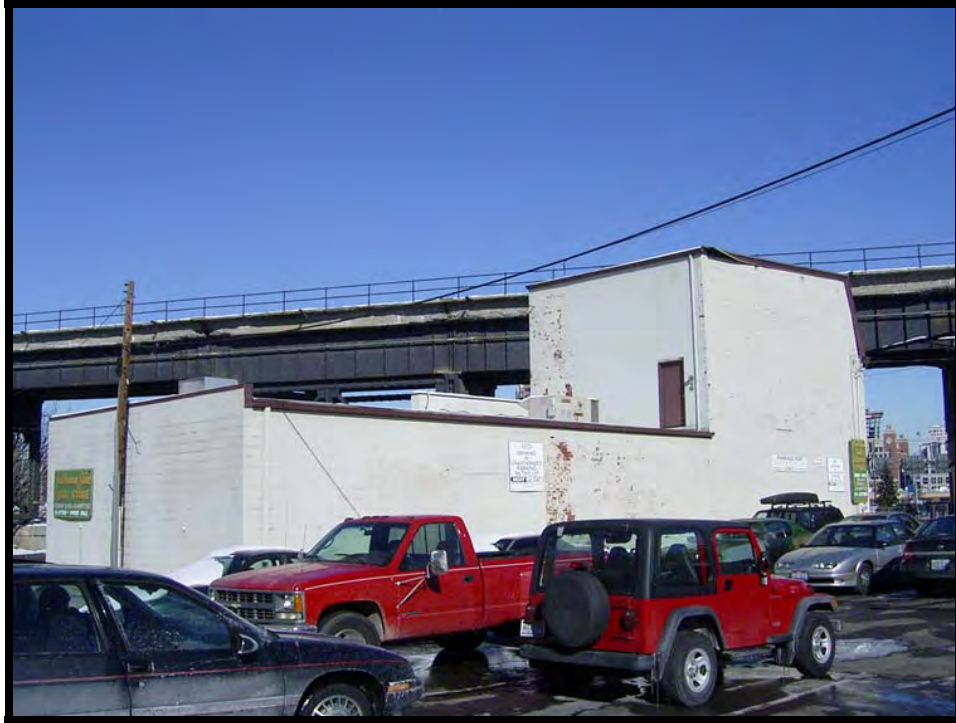
Plate 6. View of 407 Main Street (KEC 430), facing southwest.
