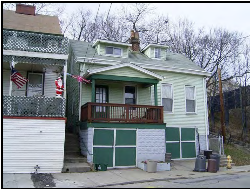
Plate 74. View of 601 Crescent Avenue, facing west.
