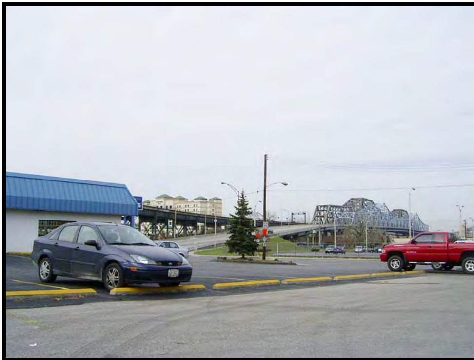
Plate 3. View of C&O Railroad Bridge (KEC 107), facing northwest.
