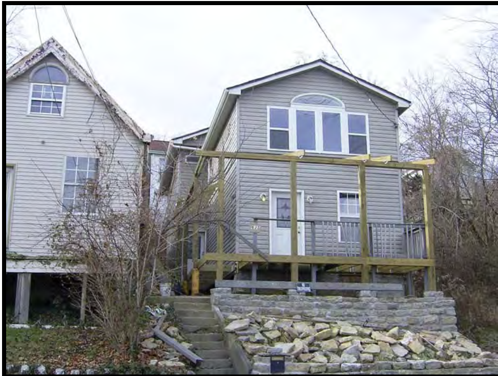
Plate 81. View of 635 Crescent Avenue, facing west.
