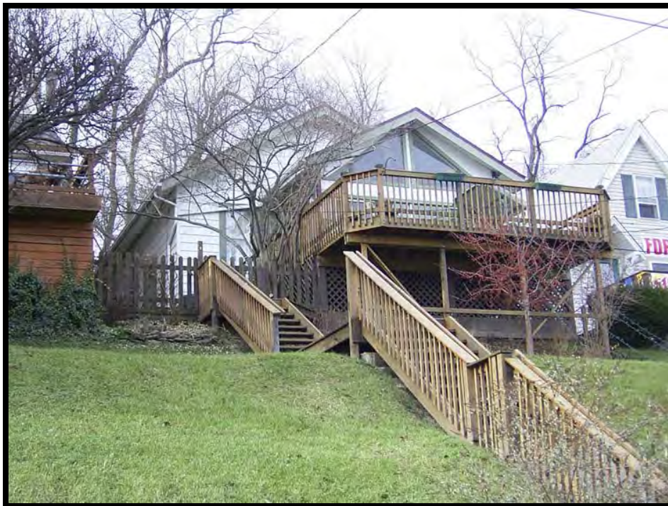
Plate 50. View of 409 Western Avenue, facing west.
