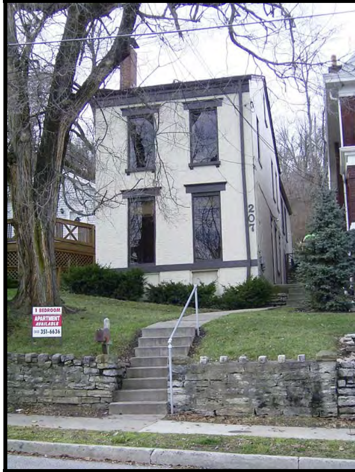
Plate 40. View of 207 Western Avenue, facing west.
