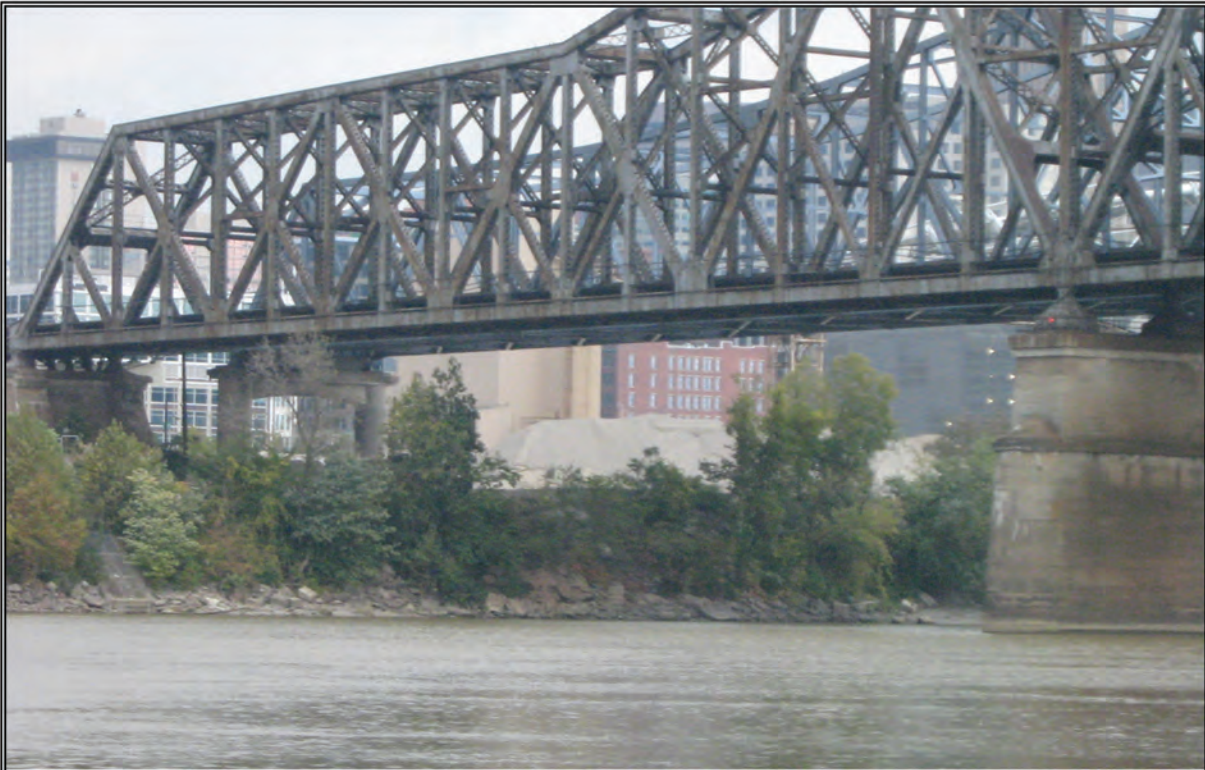
Photograph 9: Wooded riparian zone along north bank of Ohio River beneath the Bailey Bridge. View from Kentucky. Brent Spence Bridge Replacement and Rehabilitation Project. October 11, 2006.
