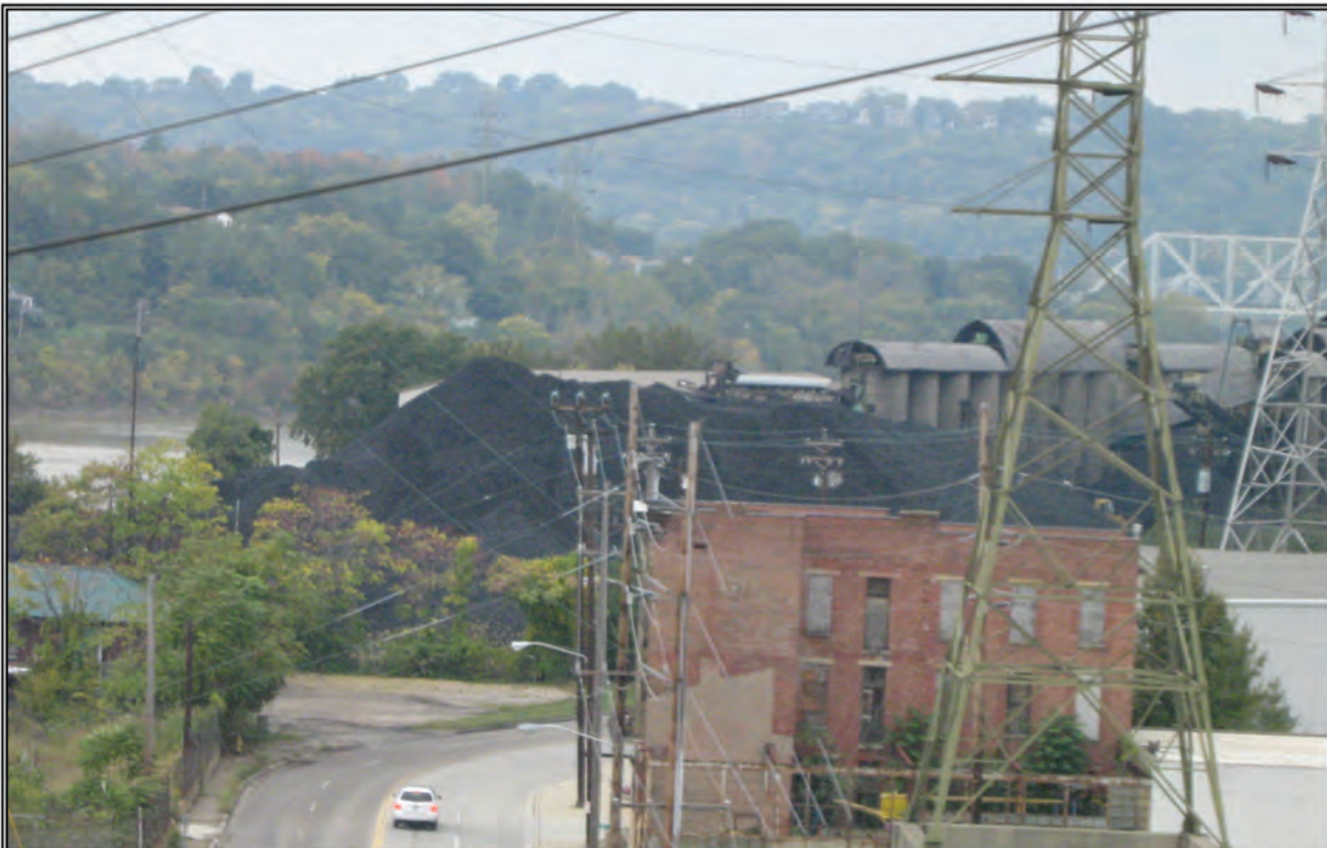
Photograph 6: Industrial portion of study area along Ohio River, facing south. Coal processing facility shown in center of frame. Brent Spence Bridge Replacement and Rehabilitation Project. October 11, 2006.
