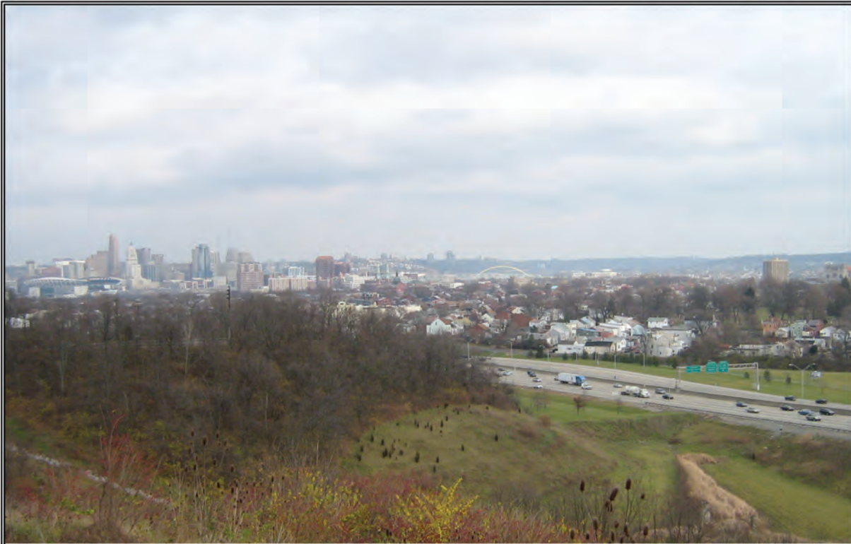
Photograph 1: General view of I-75/I-71 project corridor in northern Kentucky, facing northeast, with Cincinnati in background left portion of frame. Brent Spence Bridge Replacement and Rehabilitation Project. November 29, 2006
