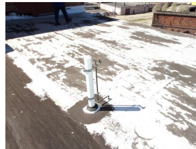
Photo 8: Plumbing Vent Pipe (noted Photo E-3 in Figure 4)
