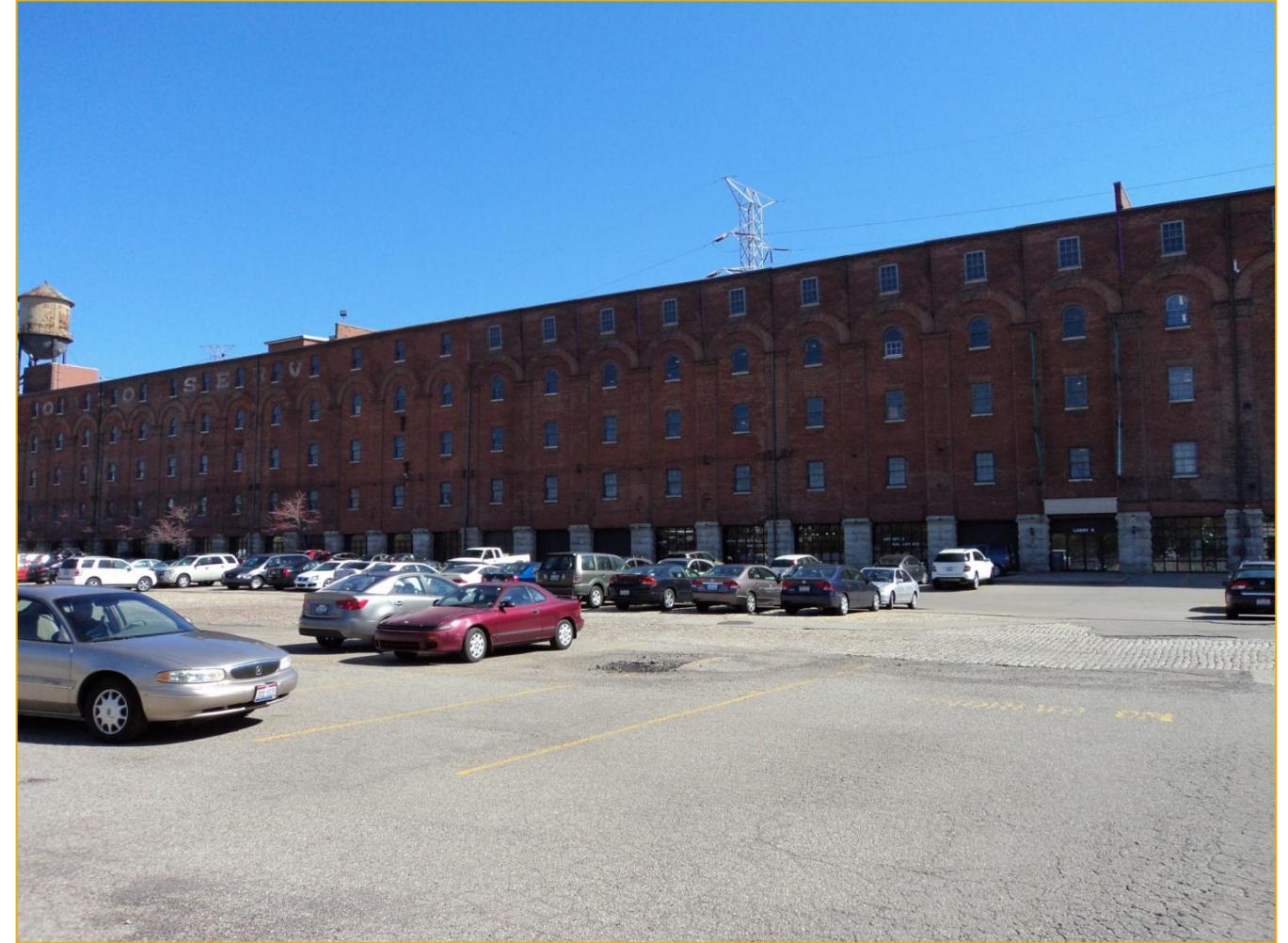
Photo 3: "After" image of Longworth Hall reconstruction at fifth floor Area "E"
