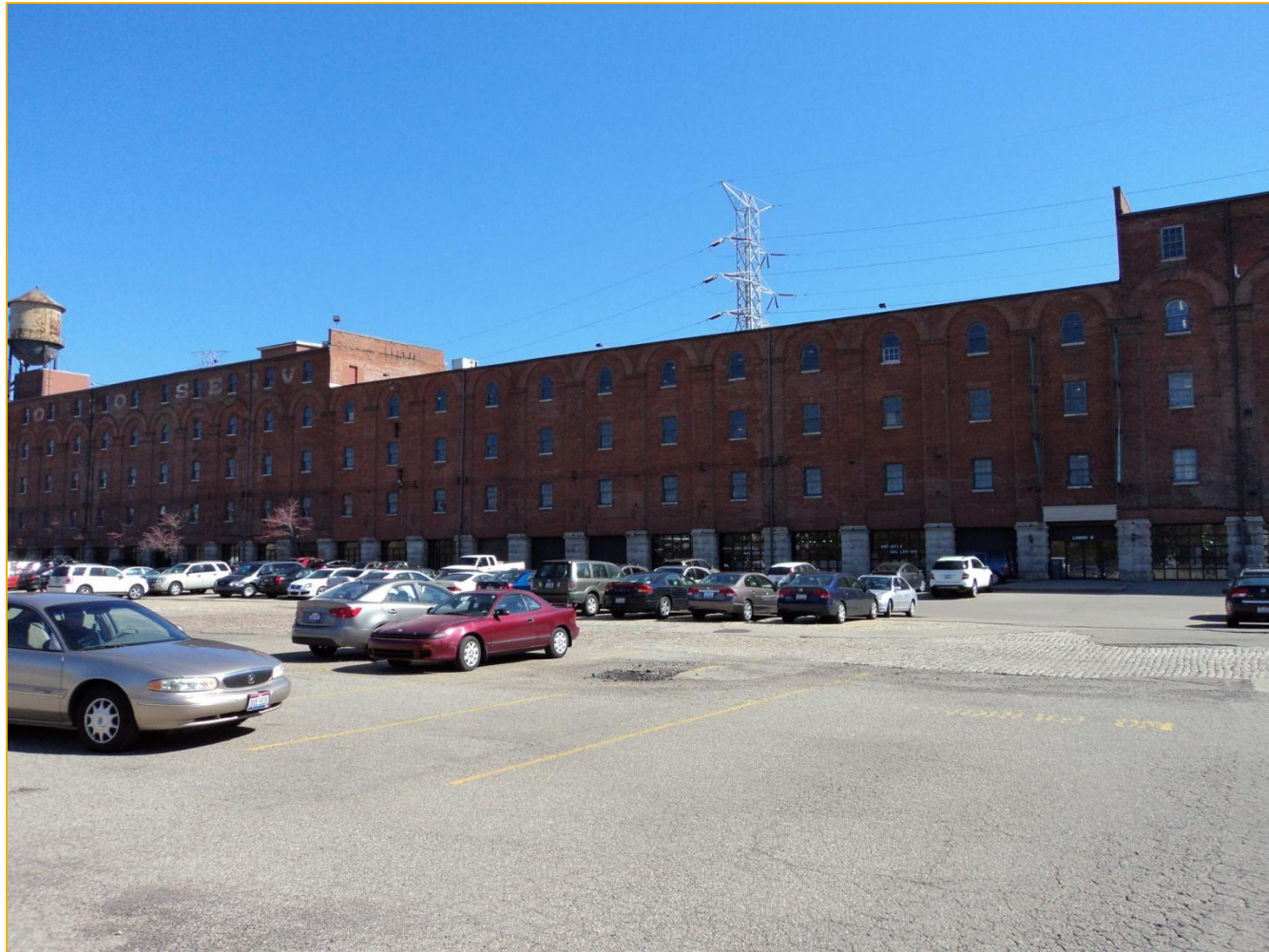
Photo 2: "Before" image of Longworth Hall showing gap at fifth floor Area "E"
