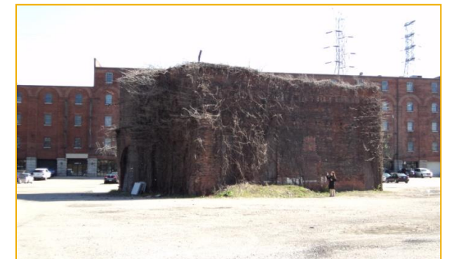
Photo 16: Boiler House: North Elevation
