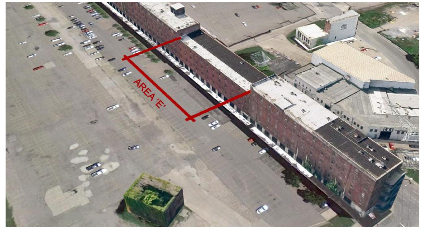
Photo 1: Aerial photo of Longworth Hall showing existing gap at Fifth Floor Area "E"
