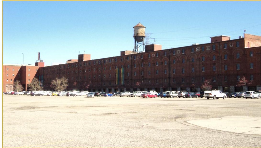
Photo 9: North Side of Longworth Hall – Existing Windows
