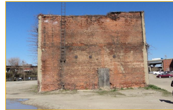
Photo 13: Boiler House: West Elevation
