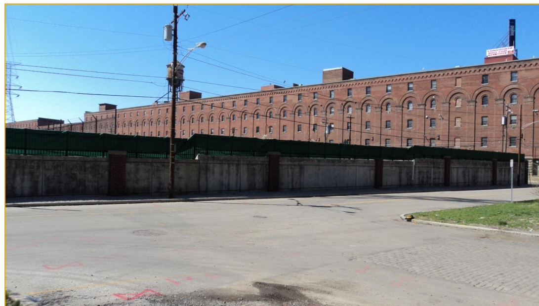
Photo 10: South Side of Longworth Hall - Existing Windows
