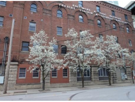
Photo 24: Incoming Communication Lines
