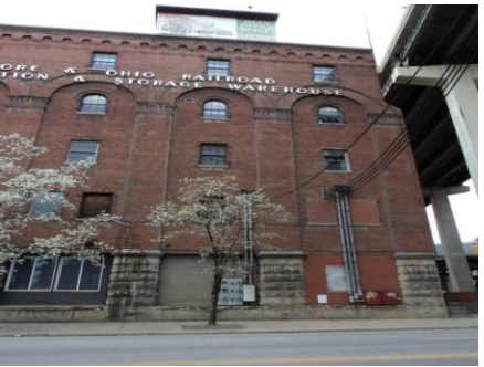
Photo 22: Area A Incoming Power
