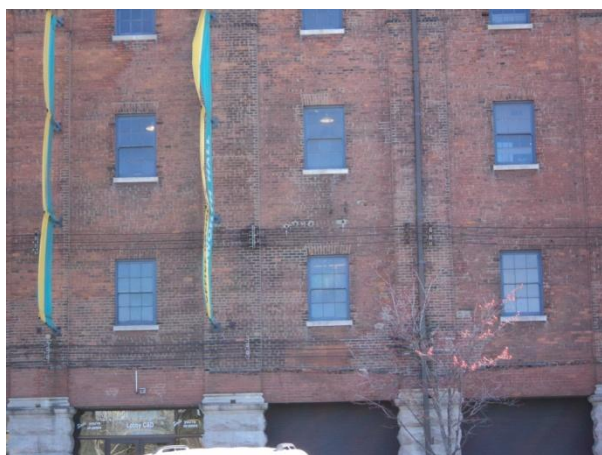
Photo 15: Elevator power lines (top set)
