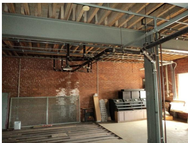
Photo 7: Area “B” Plumbing stack (noted Photo P-1 in Figure 16)
