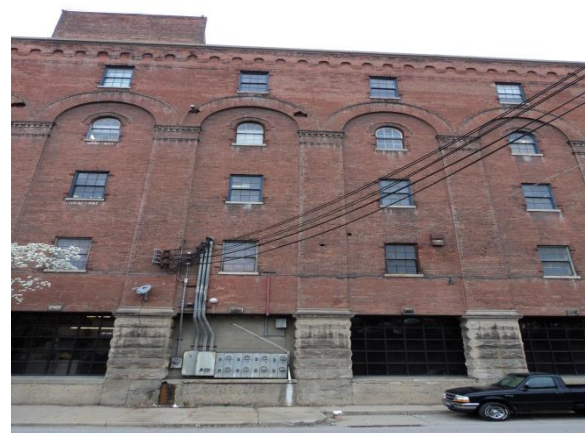
Photo 16: Area “B” incoming power (noted Photo E-2 in Figure 14)
