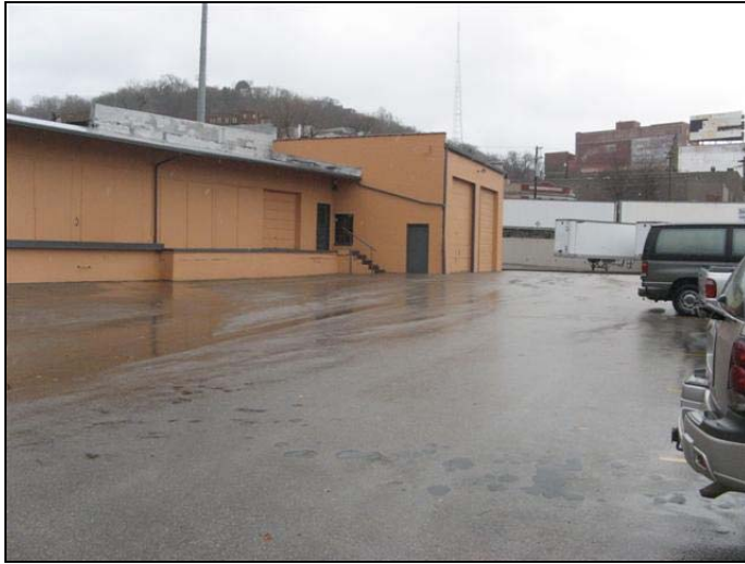
Site 3 - Back of Building
