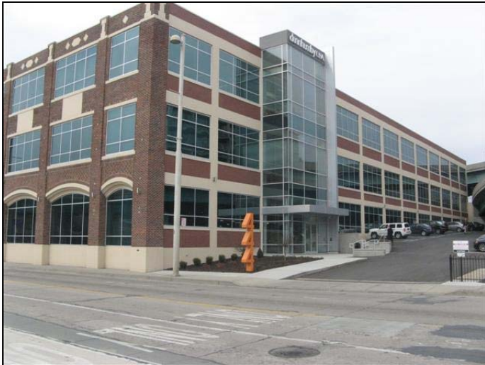
Site 55 - View From John Street
