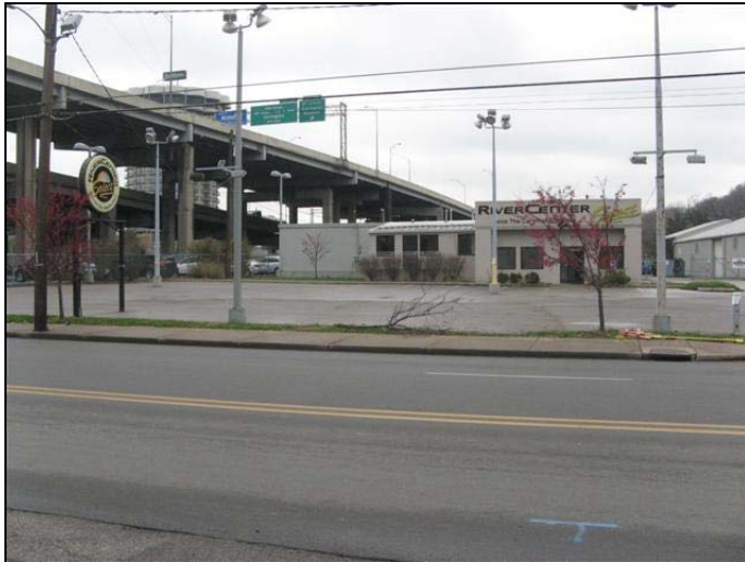
Site 74 - River City Motors
