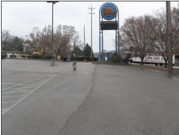
Site 80 - Former UST Location, Facing West 12'th Street
