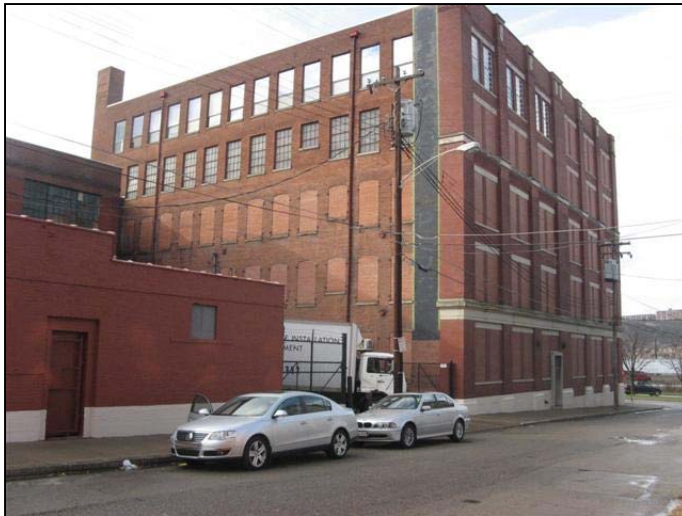
Site 9 - Warehouse. View from York Street Facing West
