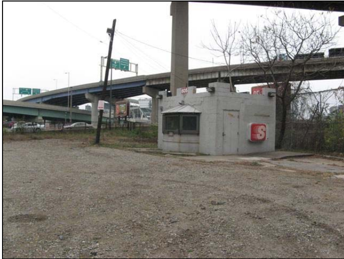
Site 53 - Old Filling Station. View from West 3 rd Street
