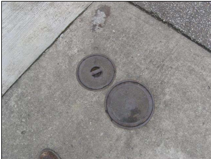
Site 53 - Suspected UST Fill Ports
