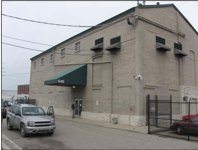
Site 60 - Building on Former MGP Location
