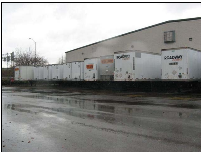
Site 4 - Back of Warehouse
