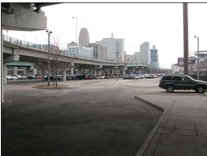
Site 58 - Former UST Location
