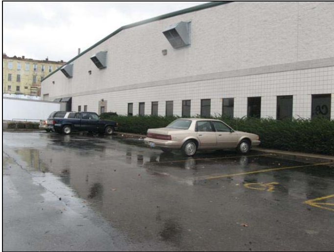
Site 4 - Front of Warehouse. View from Winchell Avenue
