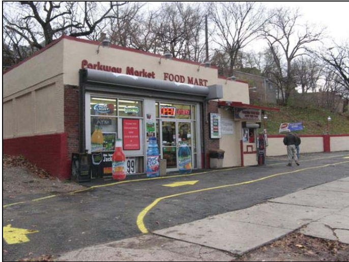
Site 1 - Along Central Parkway Parkway; UST Location Right of Building
