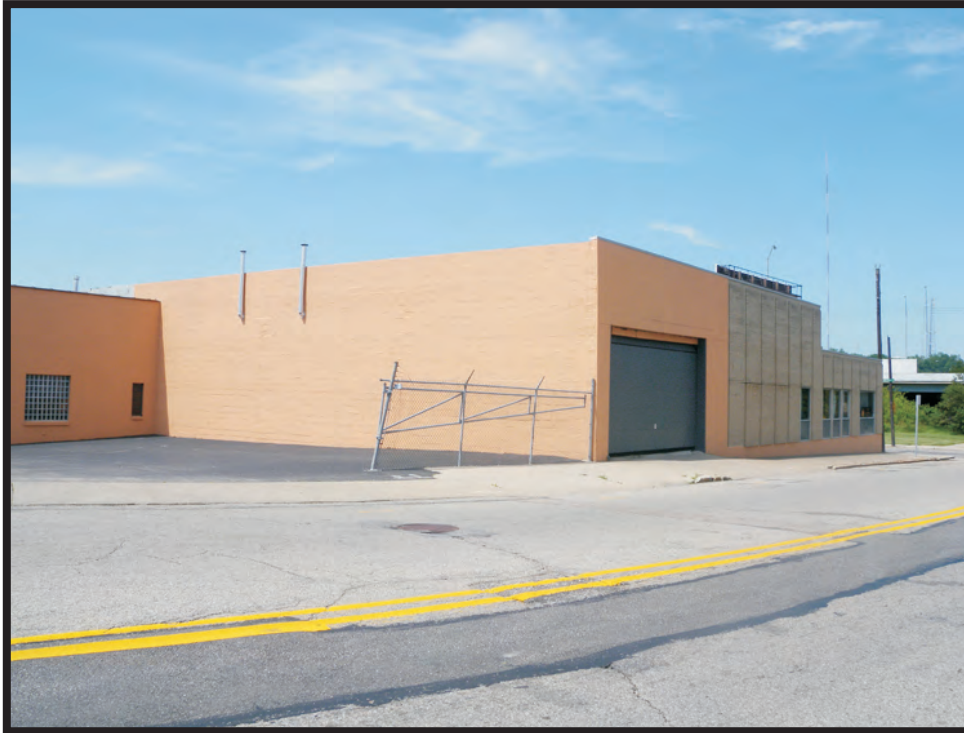
Plate B89. Building at 1155 Harrison Avenue, facing southwest.
