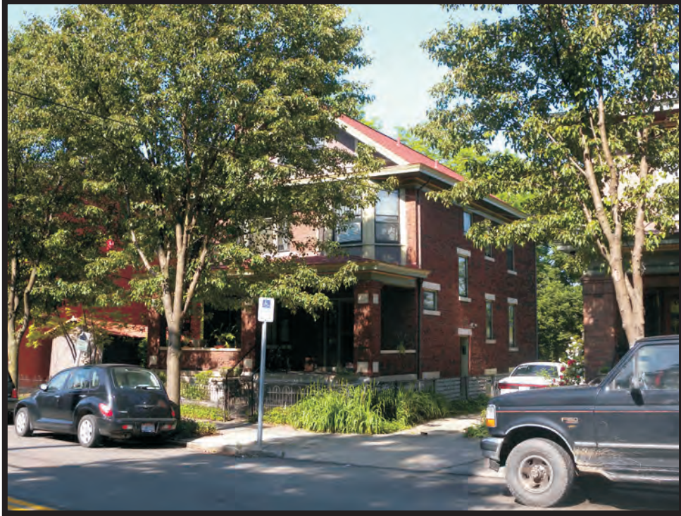
Plate B17. Building at 2403 West McMicken Avenue, facing southwest.
