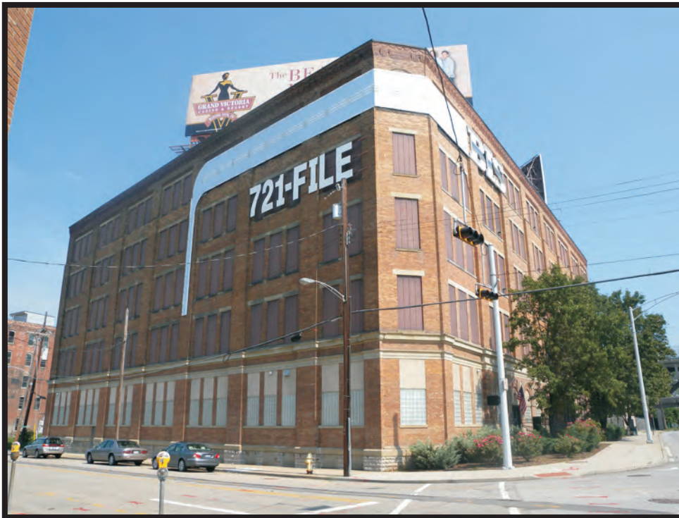
Plate B94. Building at 2201 Spring Grove Avenue, facing northwest.
