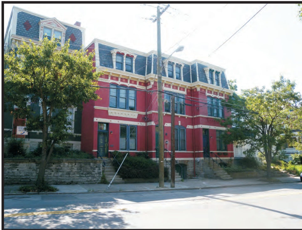
Plate B20. Building at 2358-2362 West McMicken Avenue, facing southeast.
