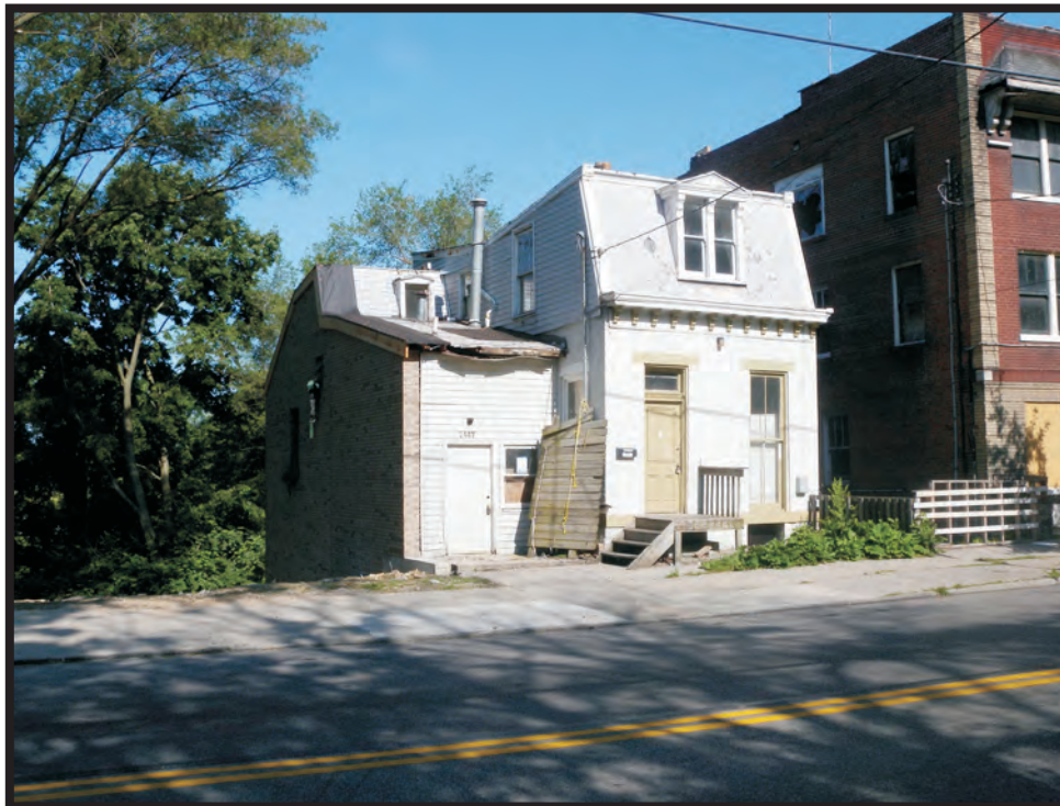
Plate B6. Building at 2447 West McMicken Avenue, facing west.
