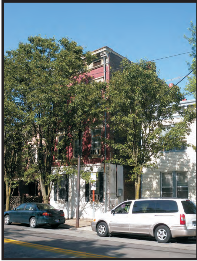
Plate B13. Building at 2411 West McMicken Avenue, facing southwest.
