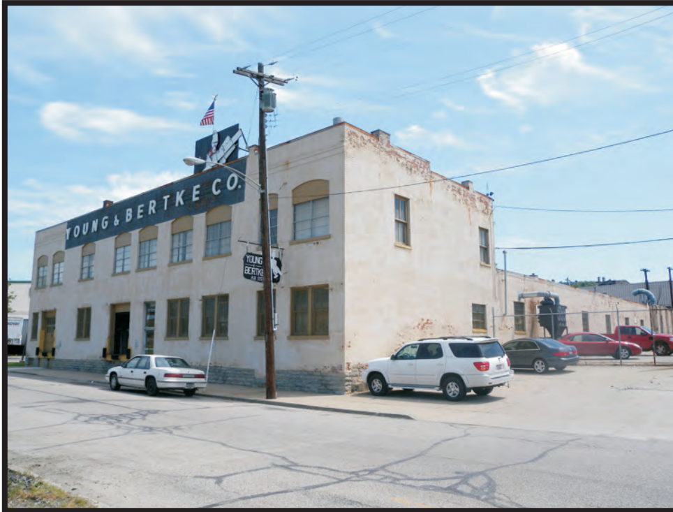
Plate B91. Building at 2124 Winchell Avenue, facing northeast.
