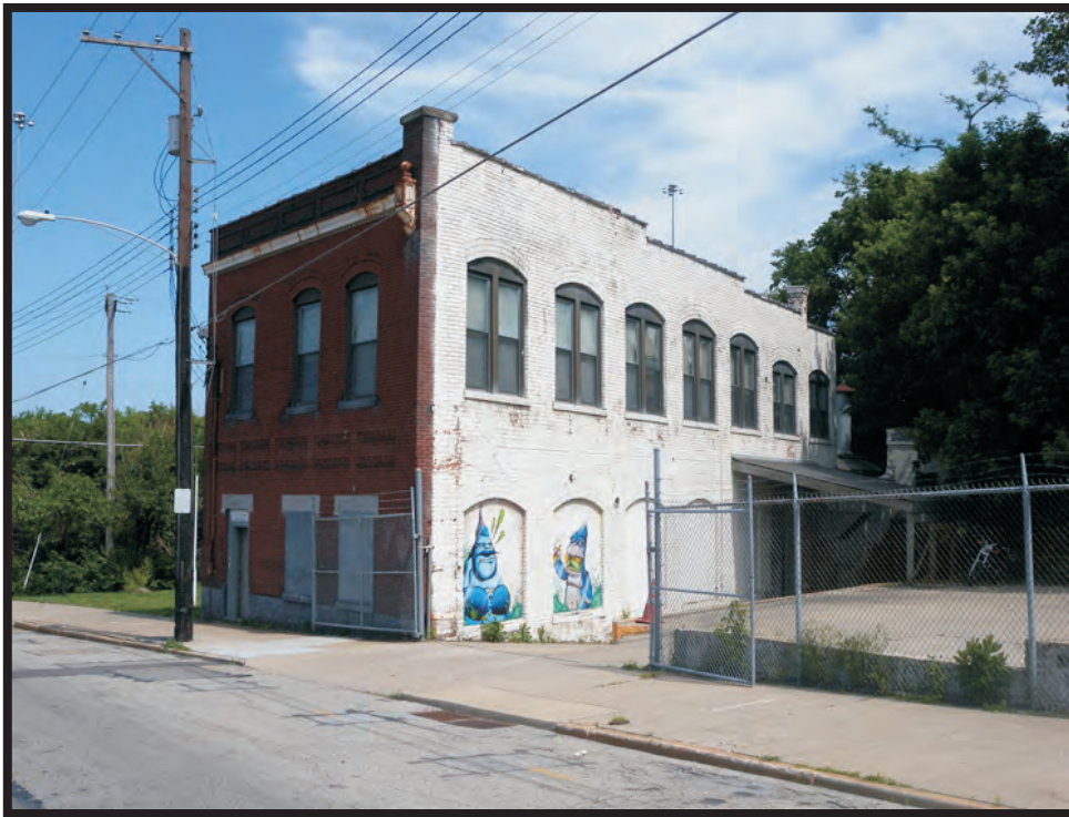
Plate B88. Building at 1136 Harrison Avenue, facing northwest.
