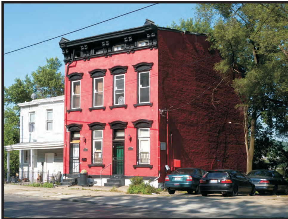
Plate B8. Building at 2437-2439 West McMicken Avenue, facing southwest.
