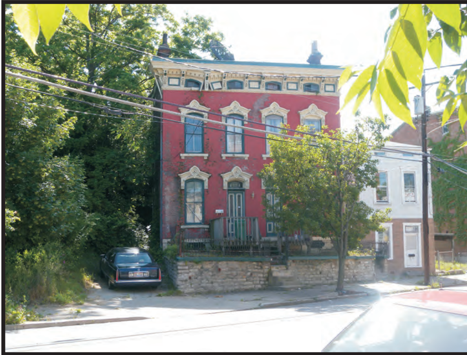
Plate B49. Building at 650 West McMicken Avenue (HAM-484-06), facing east.
