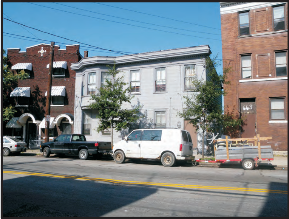
Plate B43. Building at 661 West McMicken Avenue, facing southwest.
