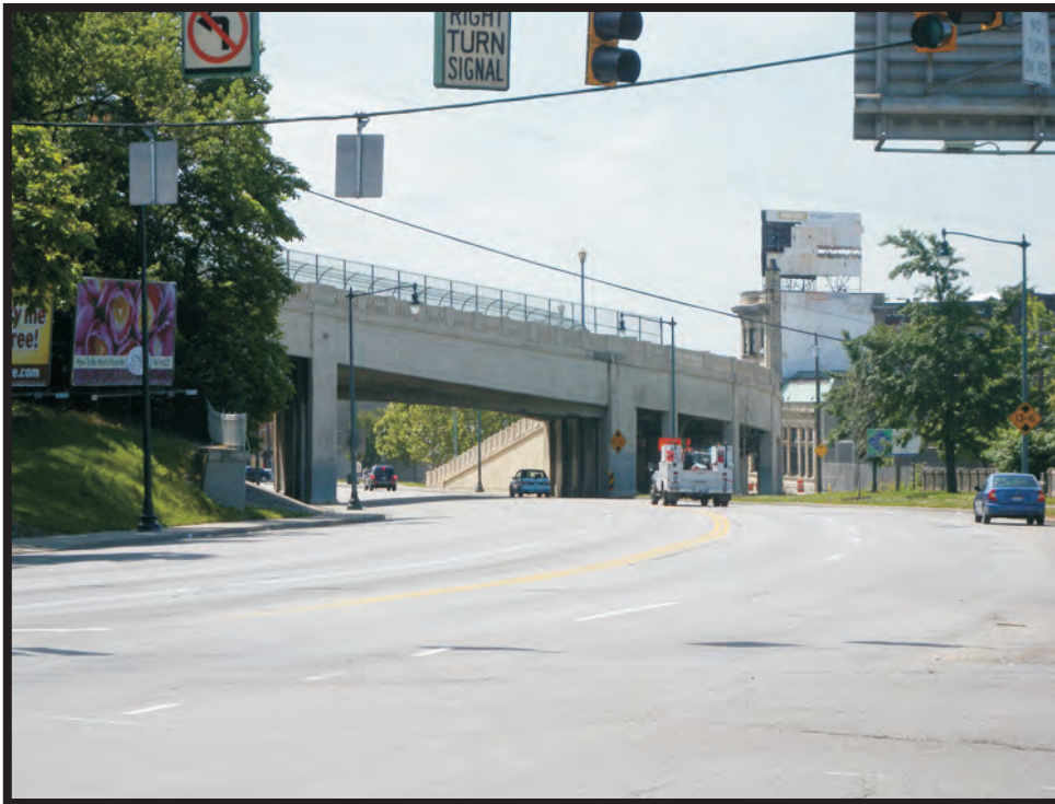
Plate B82. Brighton Bridge (SFN 3101533) at Central Parkway, facing south.
