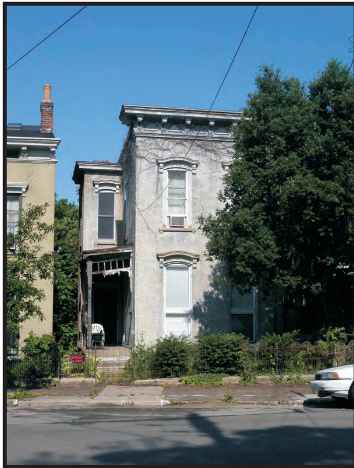
Plate B34. Building at 2323 West McMicken Avenue, facing west.
