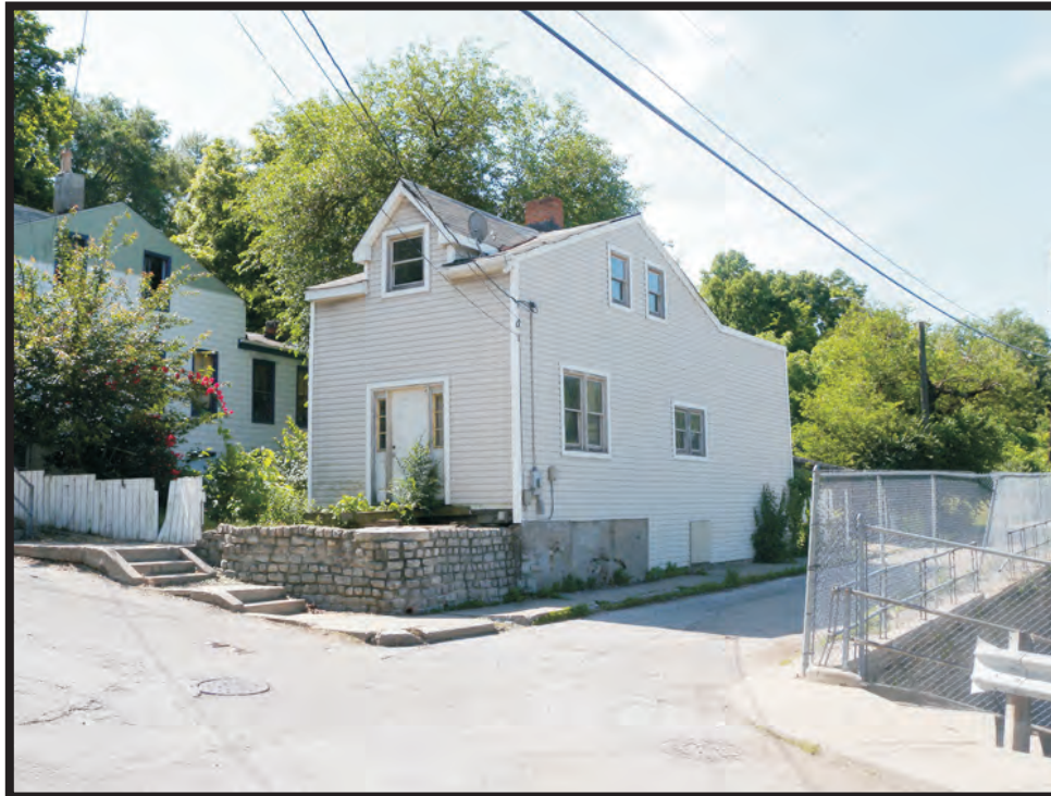
Plate B62. Building at 1061 Rush Street, facing southeast.
