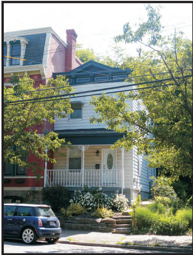
Plate B22. Building at 2356 West McMicken Avenue, facing east.
