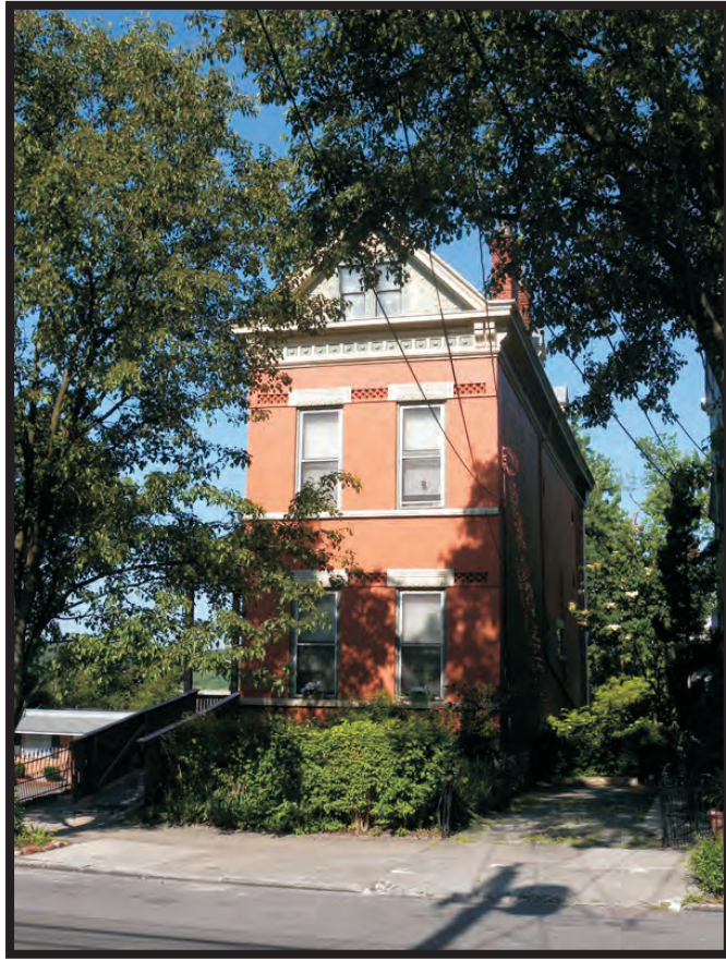
Plate B23. Building at 2355 West McMicken Avenue, facing west.
