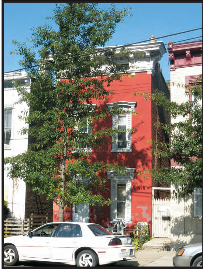
Plate B1. Building at 2459 West McMicken Avenue, facing southwest.
