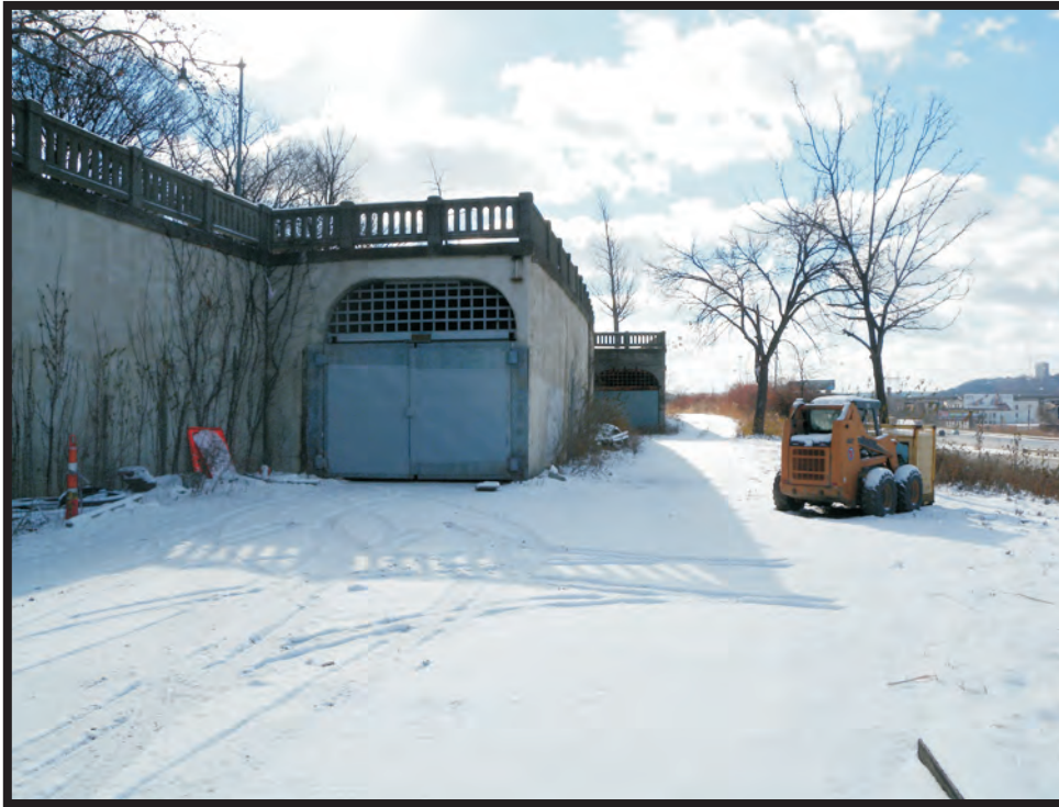
Plate B98. Western Hills Viaduct Subway Portals, facing south.
