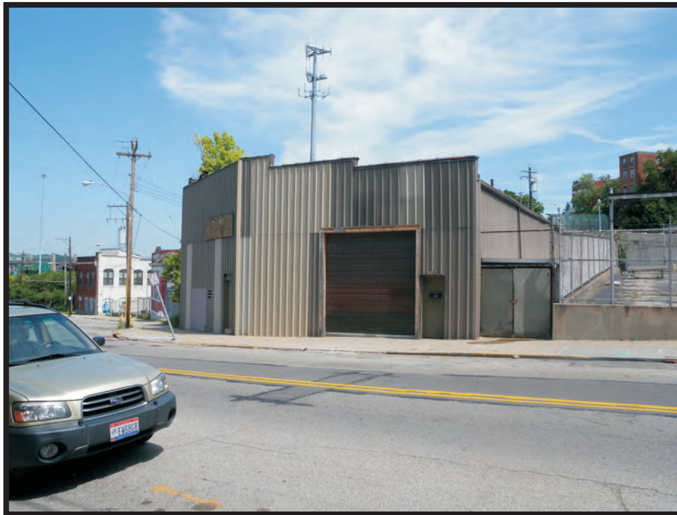
Plate B86. Building at 1112 Harrison Avenue, facing north.
