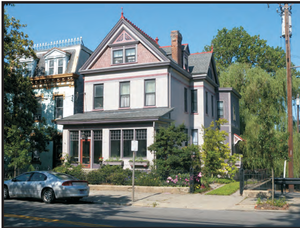
Plate B30. Building at 2343 West McMicken Avenue, facing southwest.
