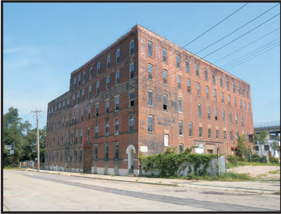
Plate B96. Building at 1220 Harrison Avenue, facing northwest.
