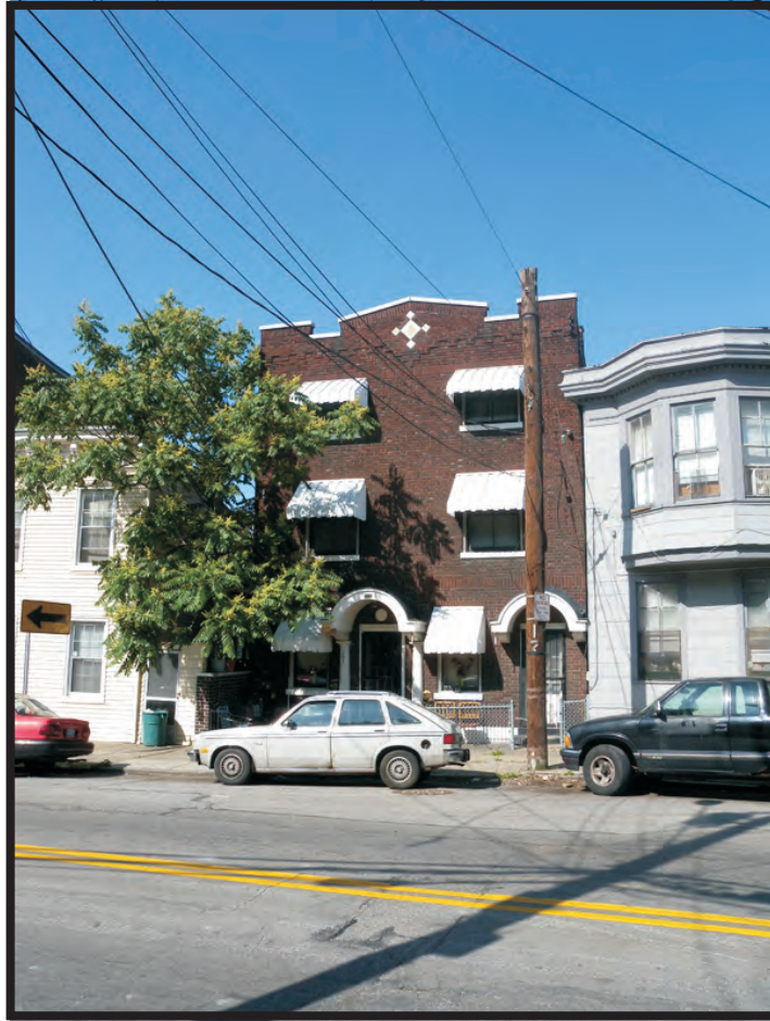
Plate B45. Building at 657 West McMicken Avenue, facing southwest.
