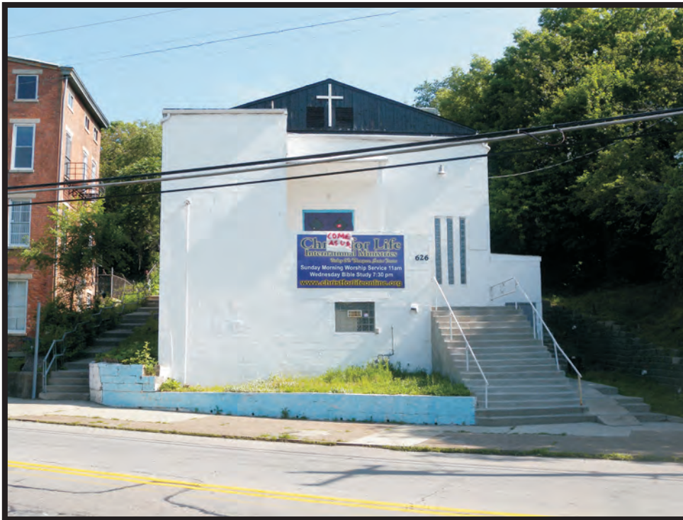
Plate B54. Building at 626 West McMicken Avenue, facing north.
