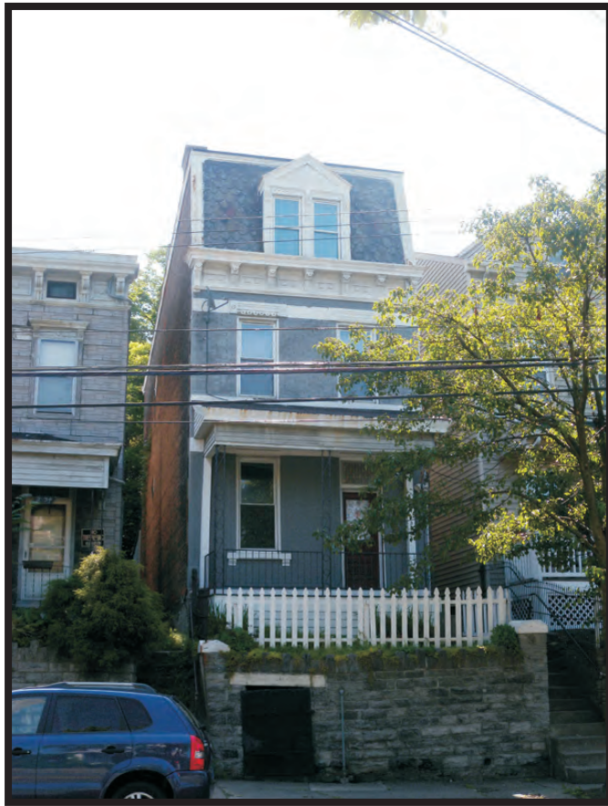
Plate B38. Building at 2332 West McMicken Avenue, facing east.
