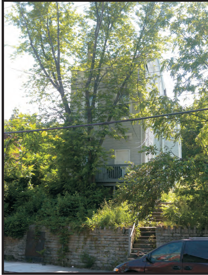
Plate B5. Building at 2450 West McMicken Avenue, facing east.
