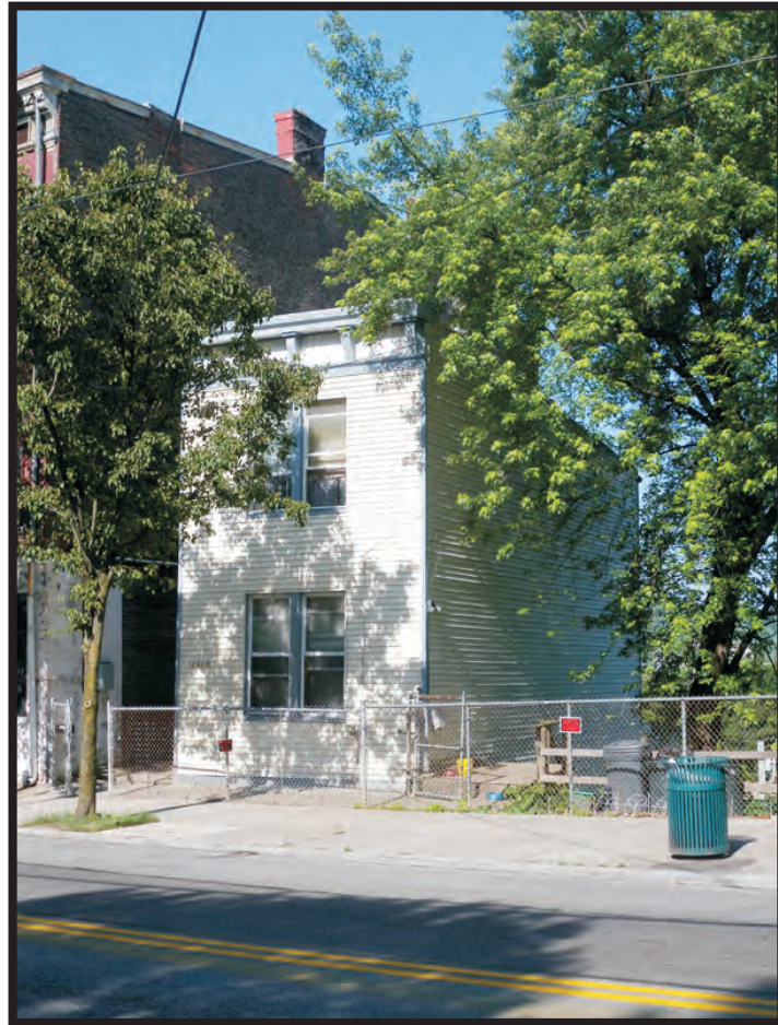
Plate B10. Building at 2413 West McMicken Avenue, facing southwest.
