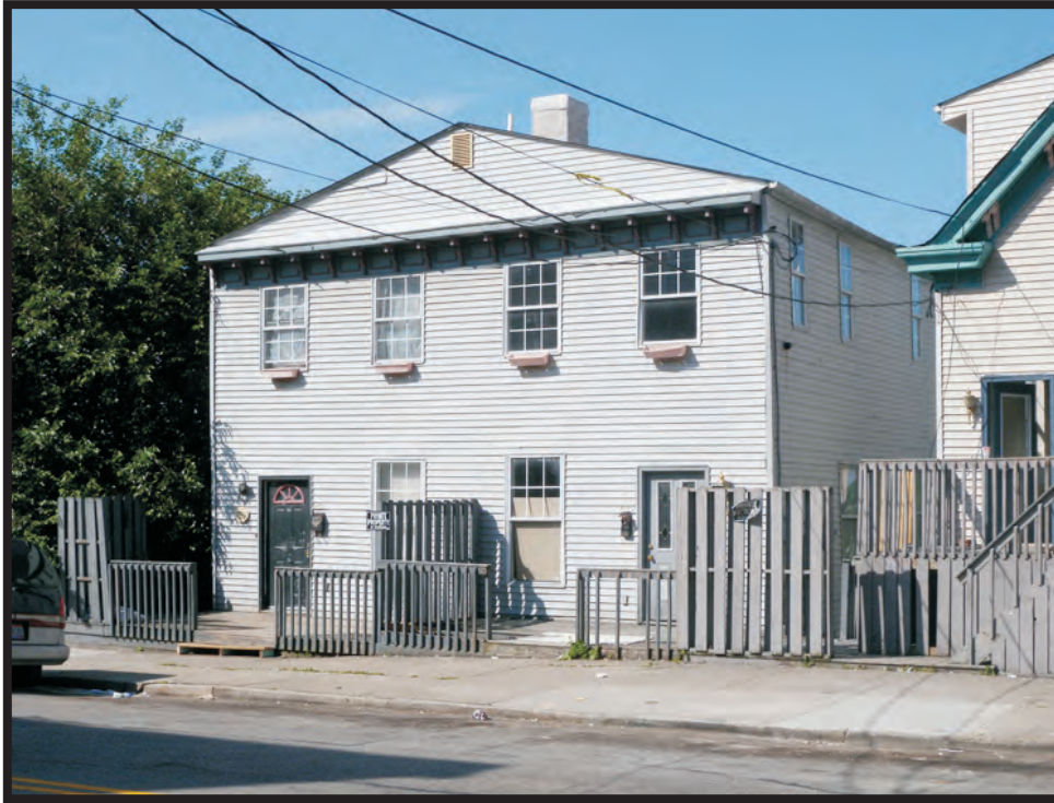
Plate B51. Building at 645 West McMicken Avenue, facing southwest.
