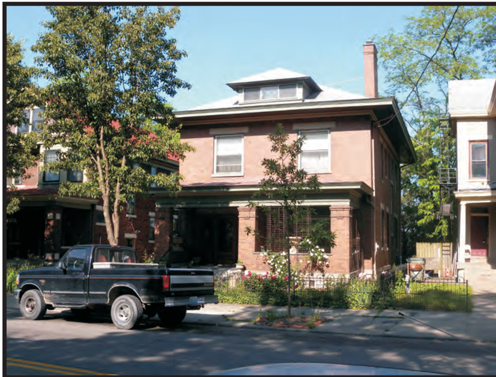
Plate B16. Building at 2405 West McMicken Avenue, facing southwest.
