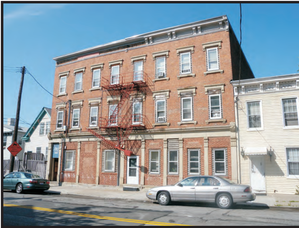
Plate B48. Building at 649 West McMicken Avenue, facing southwest.
