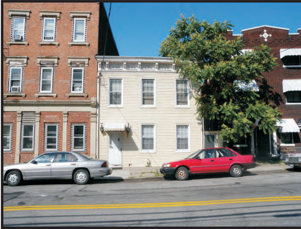
Plate B47. Building at 655 West McMicken Avenue, facing west.
