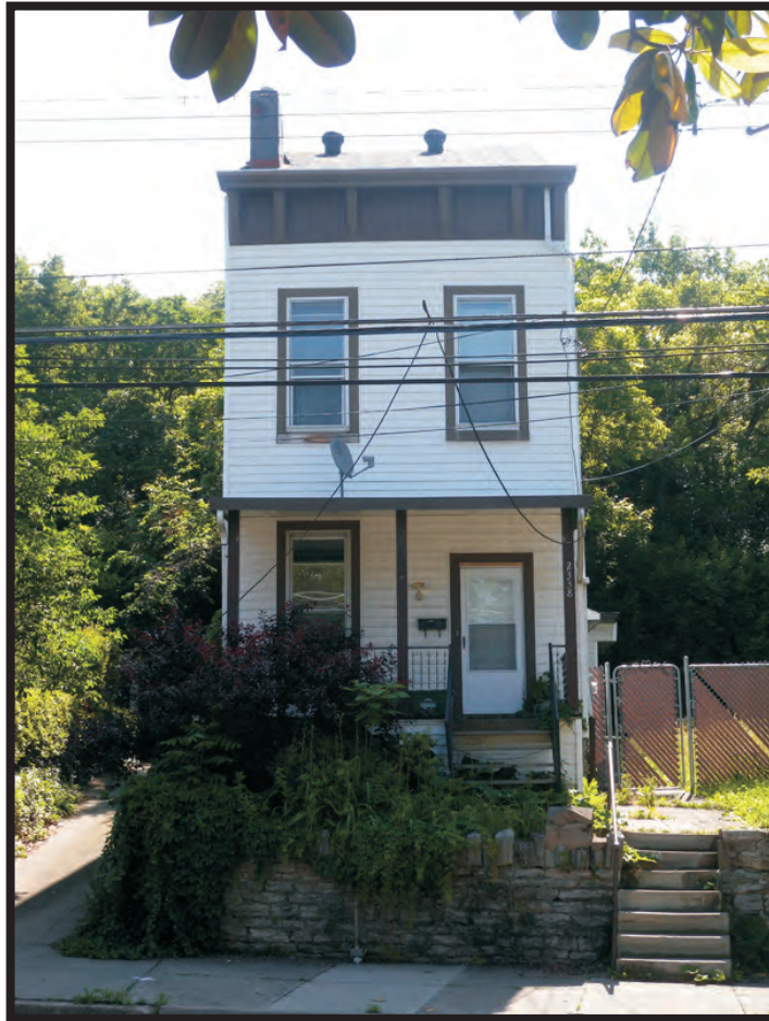
Plate B36. Building at 2338 West McMicken Avenue, facing east.
