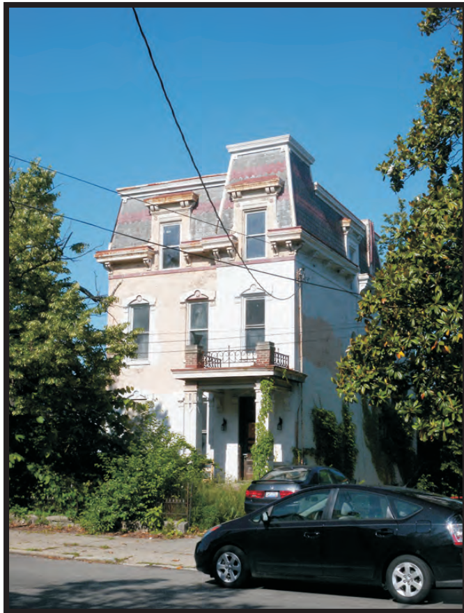
Plate B32. Building at 2335 West McMicken Avenue, facing west.
