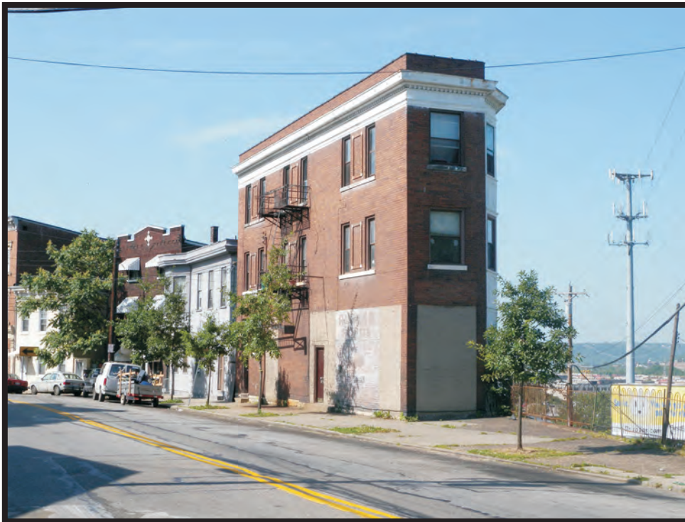
Plate B42. Building at 663-665 West McMicken Avenue, facing southwest.
