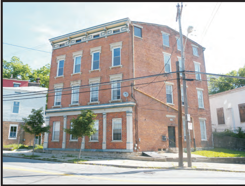
Plate B53. Building at 642 West McMicken Avenue, facing north.
