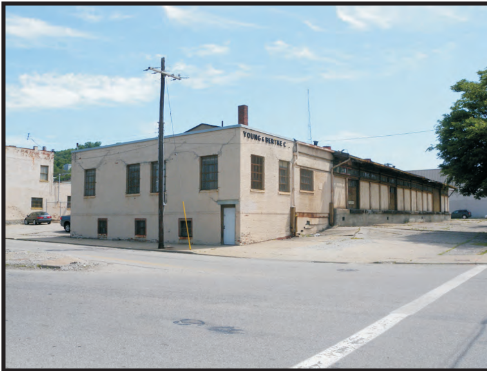
Plate B92. Building at 2108 Winchell Avenue, facing northeast.
