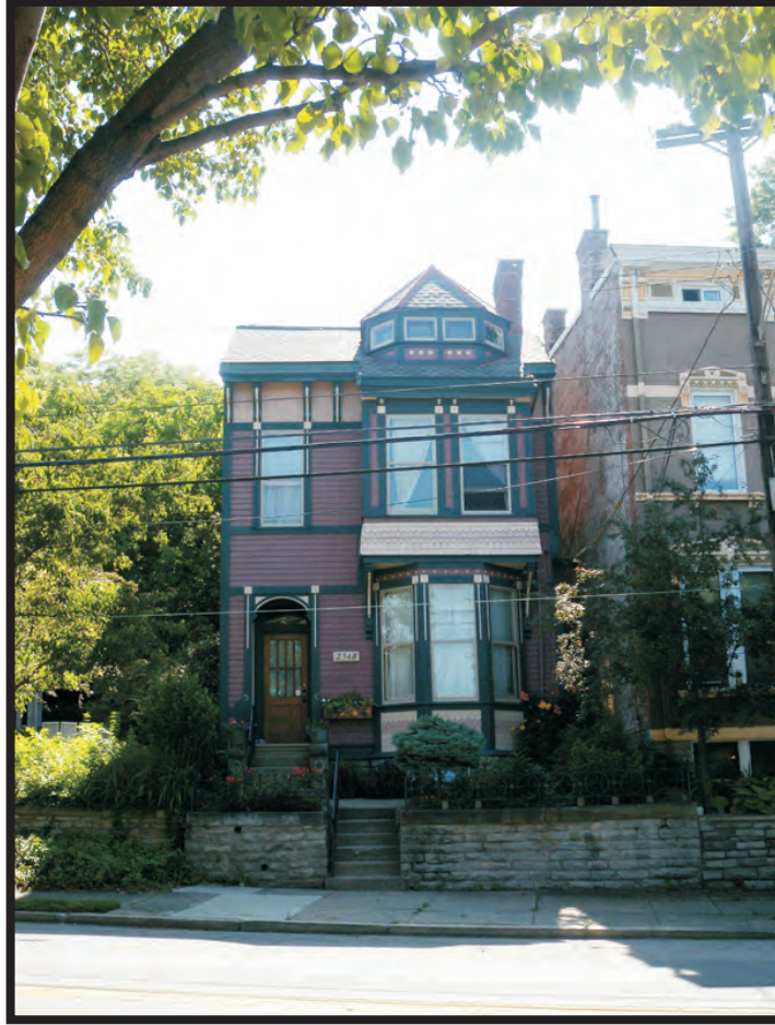
Plate B25. Building at 2348 West McMicken Avenue, facing east.
