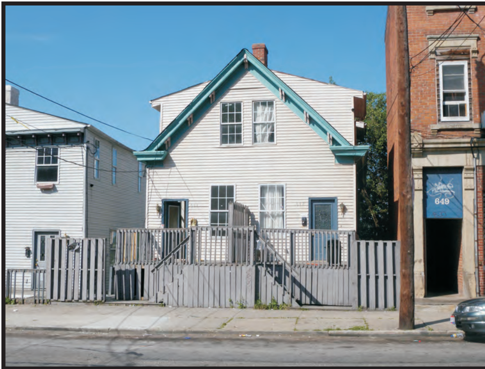
Plate B50. Building at 647 West McMicken Avenue, facing southwest.
