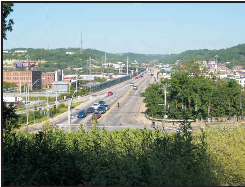
Plate B78. Western Hills Viaduct (SFN 3105458) from West McMicken Avenue, facing west.
