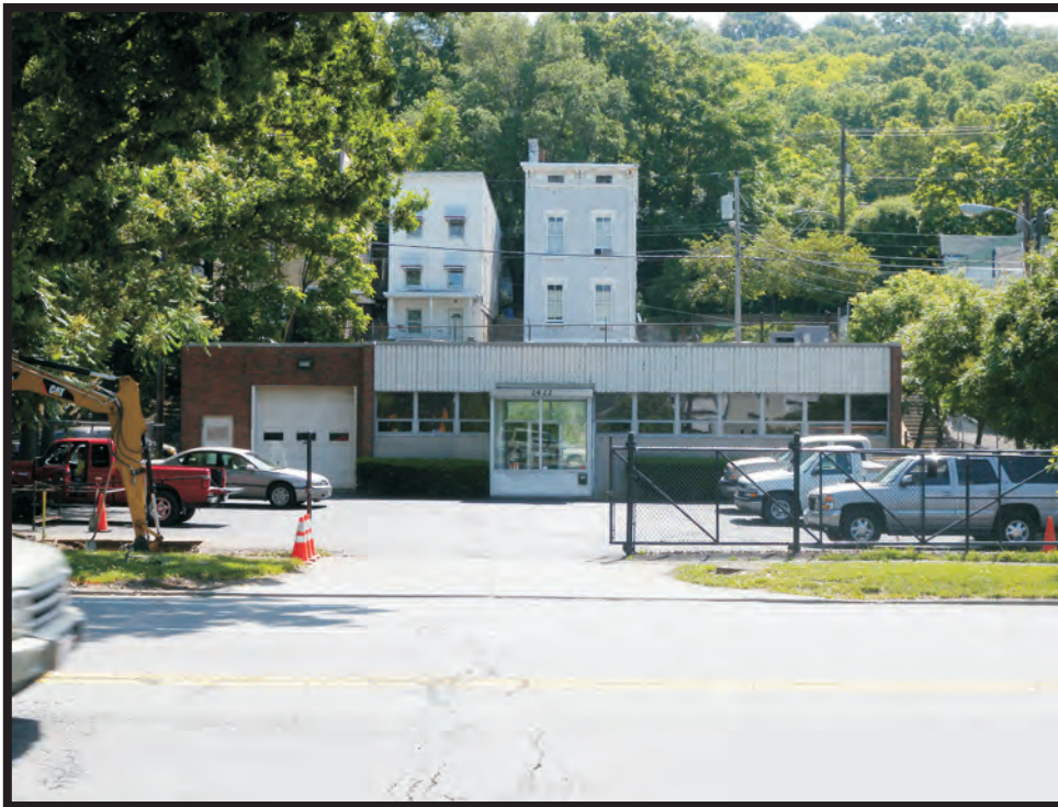
Plate B68. Building at 2422 Central Parkway, facing east.
