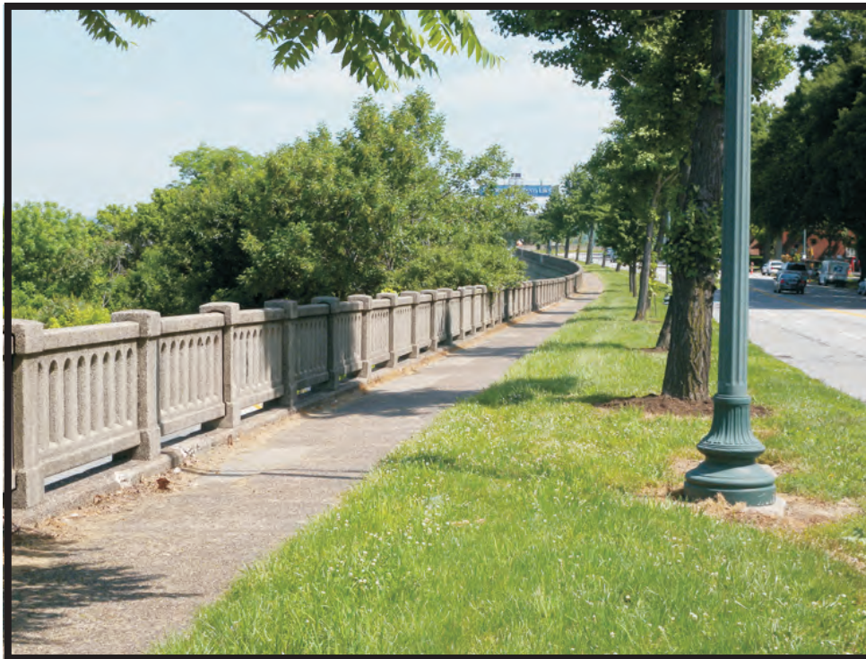
Plate B76. Central Parkway (HAM-7571-40) and concrete guardrail, facing north.
