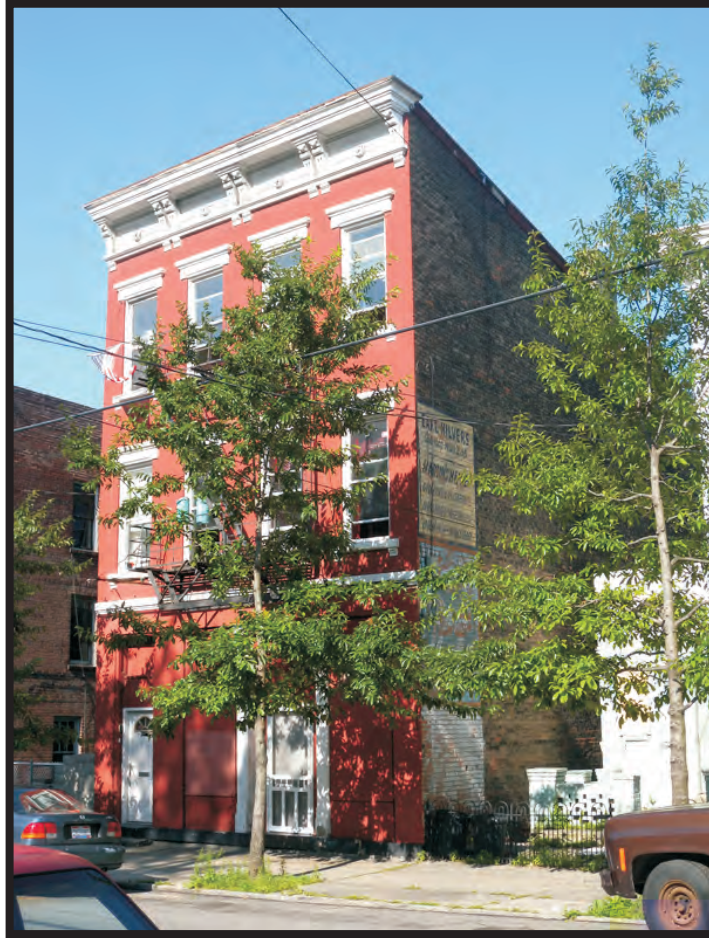
Plate B3. Building at 2455 West McMicken Avenue, facing southwest.
