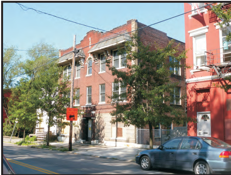
Plate B4. Building at 2453 West McMicken Avenue, facing southwest.
