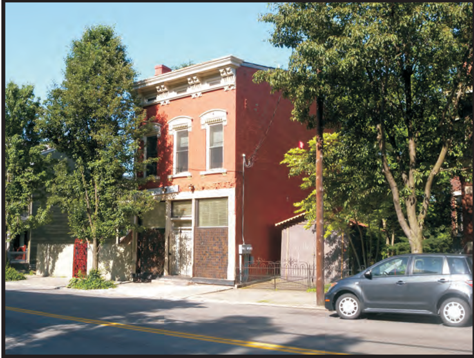
Plate B18. Building at 2365 West McMicken Avenue, facing southwest.
