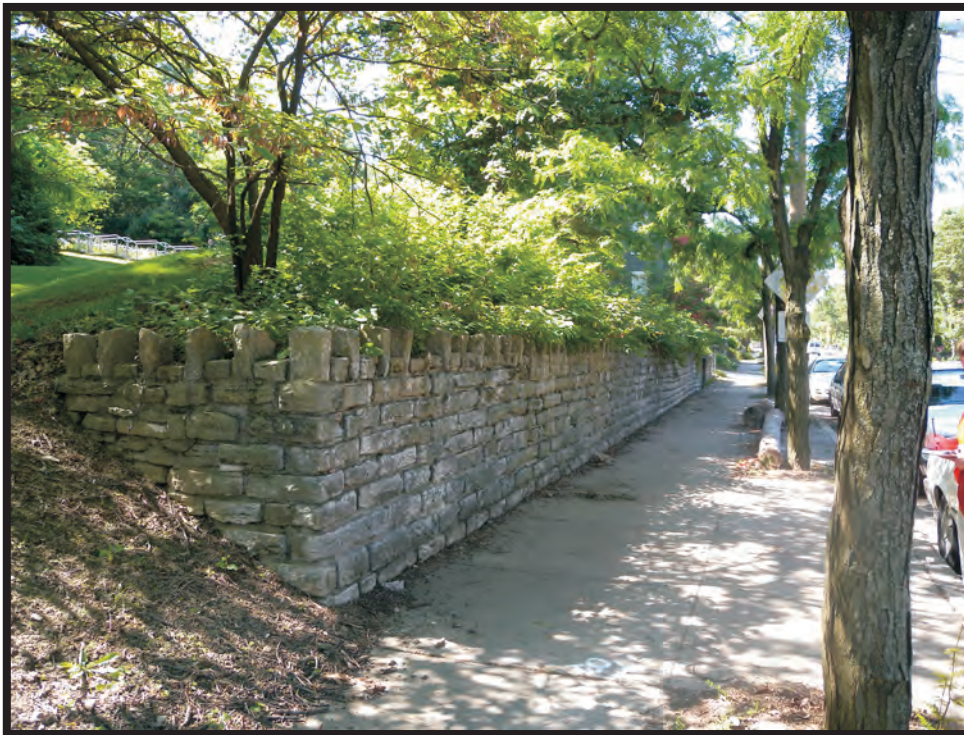
Plate B12. Stone wall along West McMicken Avenue, facing south.
