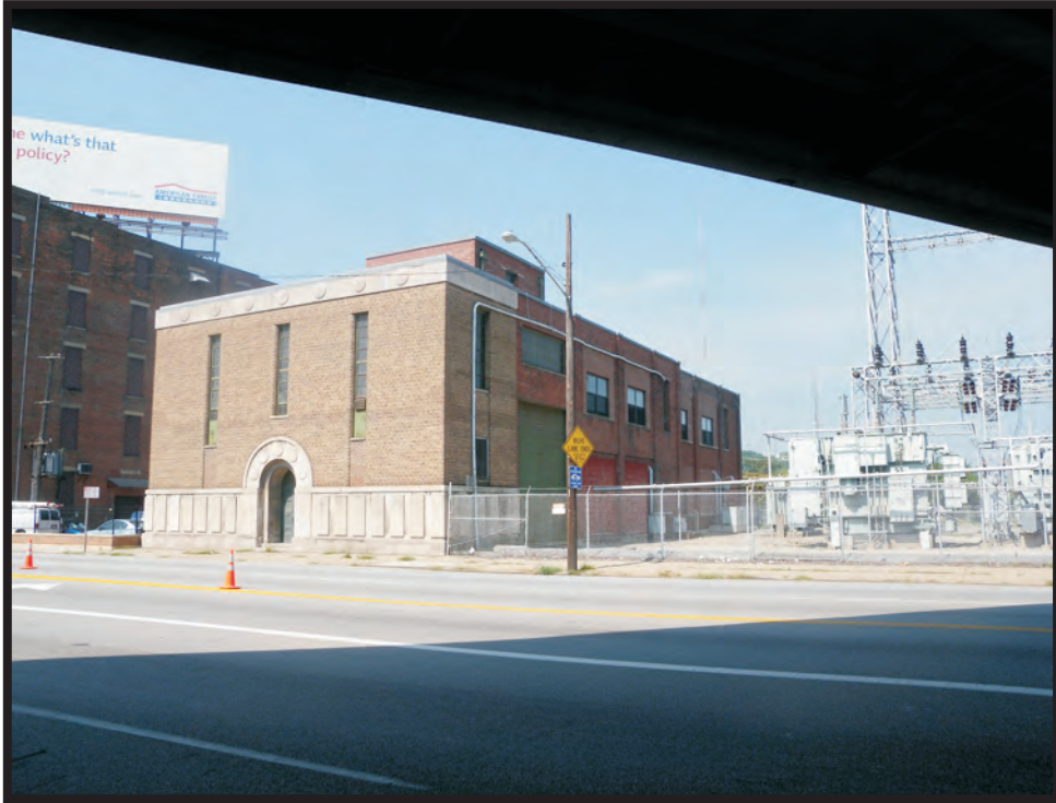
Plate B95. Duke Energy Brighton Substation at 2229 Spring Grove Avenue, facing southwest.
