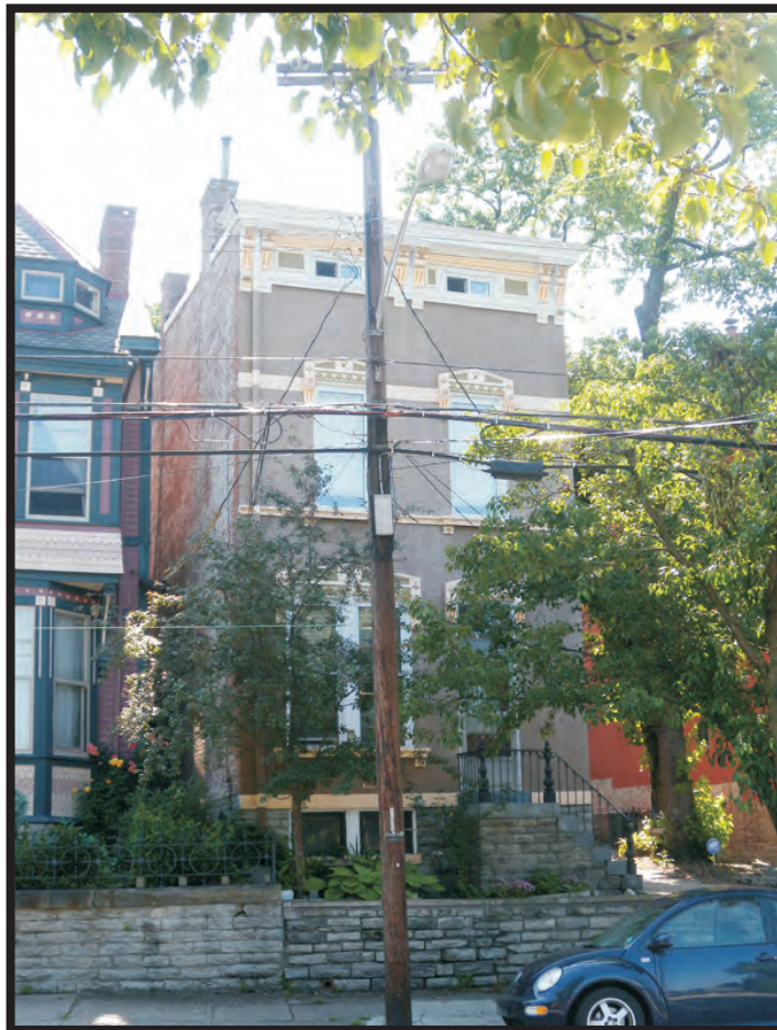
Plate B28. Building at 2346 West McMicken Avenue, facing southeast.
