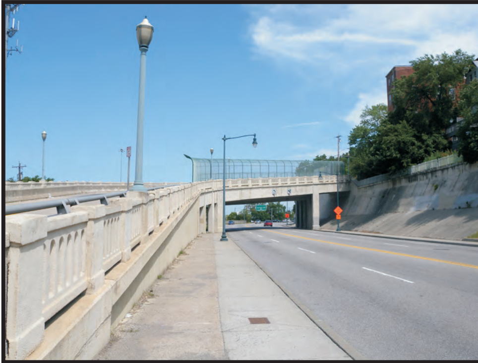
Plate B83. Brighton Bridge (SFN 3101533) at Central Parkway, facing north.
