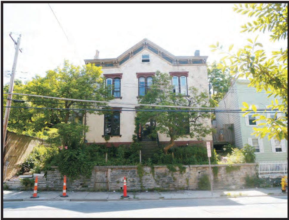
Plate B44. Building at 635 Kress Alley (HAM-1462-06), facing east.
