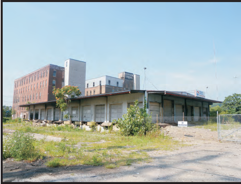
Plate B97. Building at 1220 Harrison Avenue, facing southwest.
