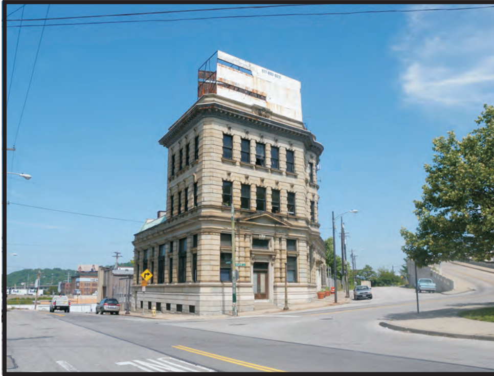
Plate B85. Building at 1110 Harrison Avenue(HAM-2164-28), facing northwest.
