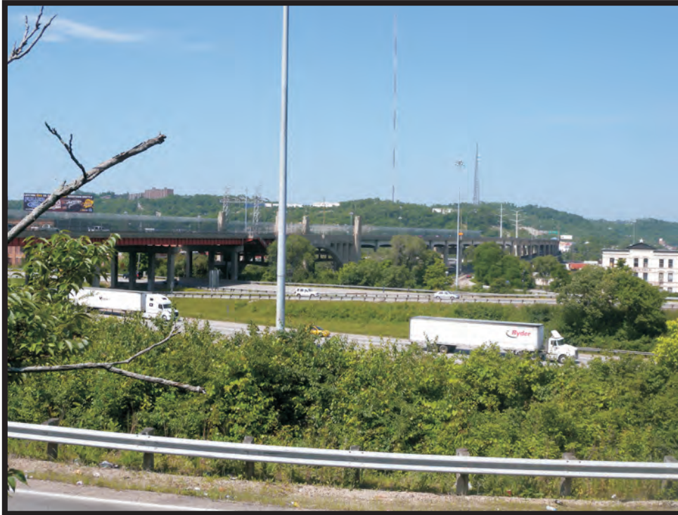
Plate B77. View of the Western Hills Viaduct (SFN 3105458) from Central Parkway, facing southwest.
