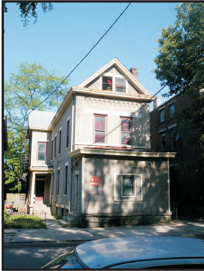
Plate B15. Building at 2407 West McMicken Avenue, facing west.
