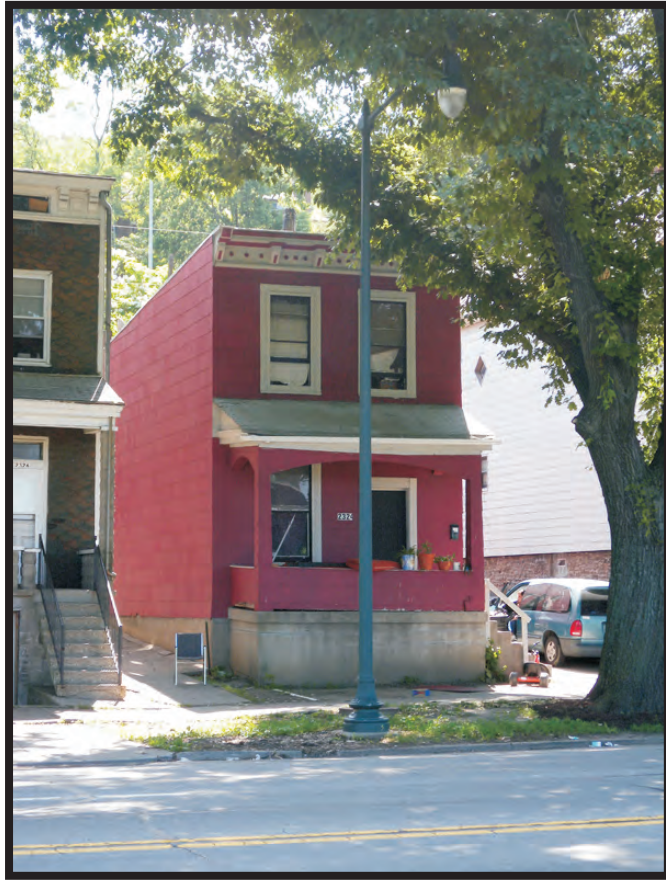
Plate B71. Building at 2324 Central Parkway, facing east.
