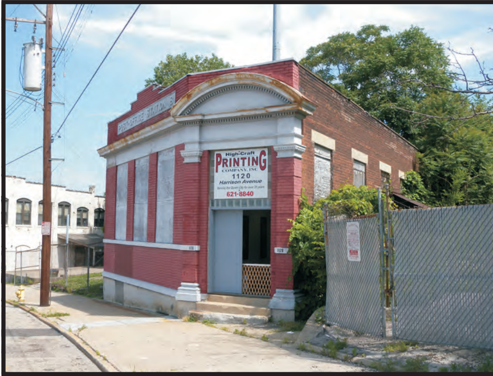
Plate B87. Building at 1120 Harrison Avenue (HAM-7366-28), facing north.
