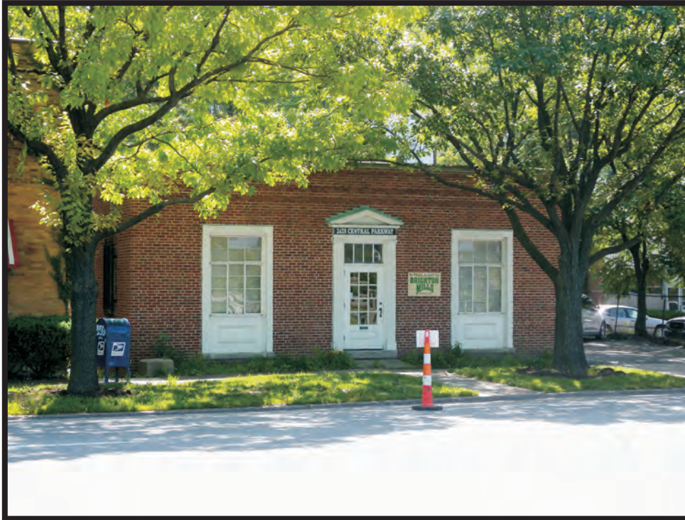
Plate B67. Building at 2428 Central Parkway, facing east.
