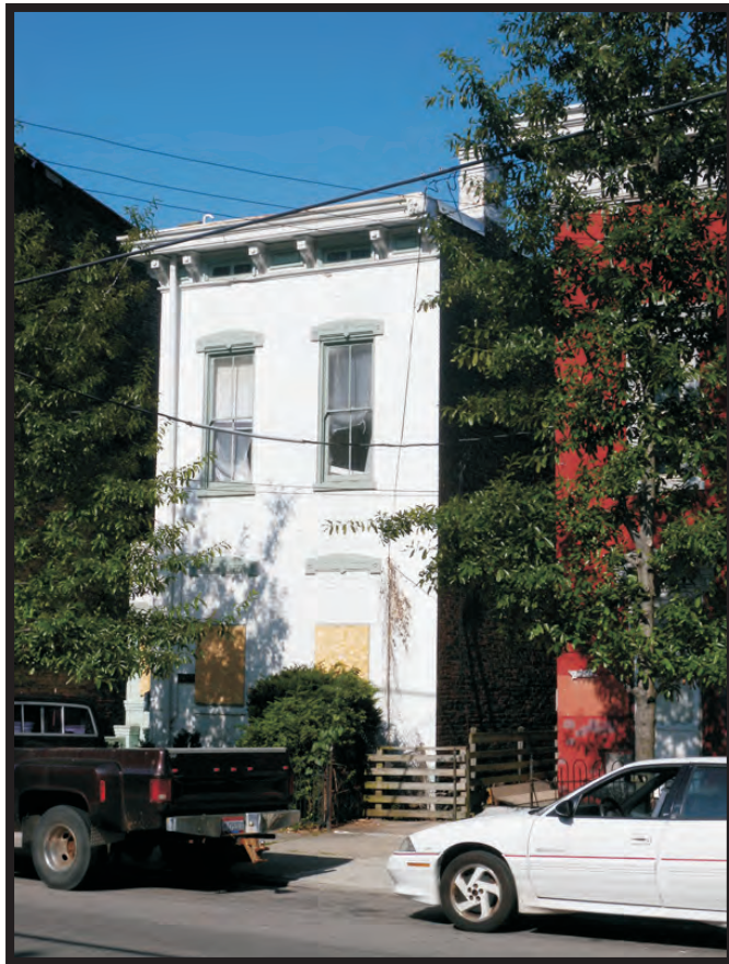
Plate B2. Building at 2457 West McMicken Avenue, facing southwest.
