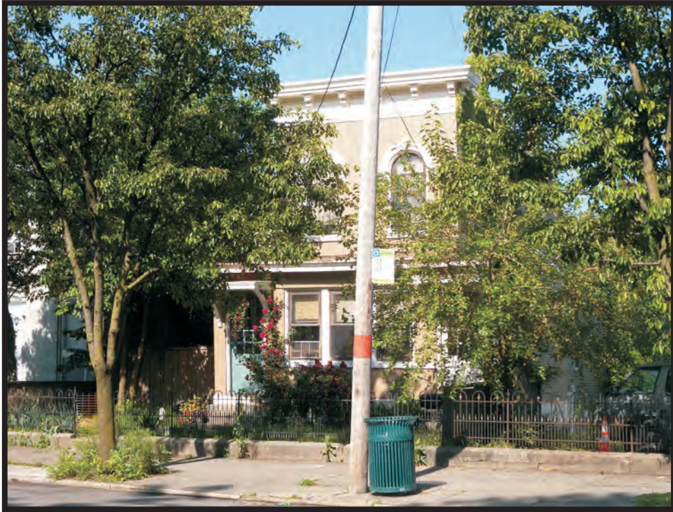
Plate B33. Building at 2325 West McMicken Avenue, facing west.
