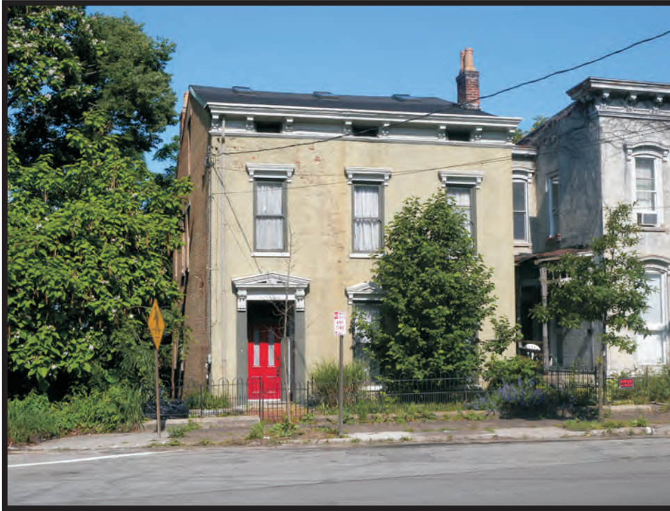
Plate B35. Building at 2321 West McMicken Avenue, facing west.
