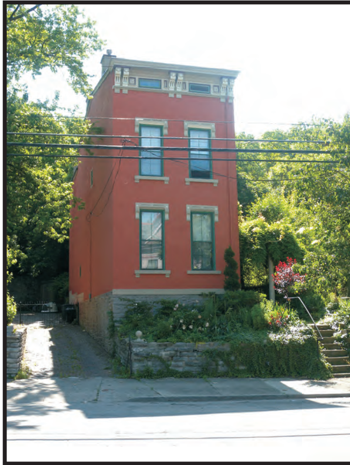
Plate B29. Building at 2342 West McMicken Avenue, facing southeast.
