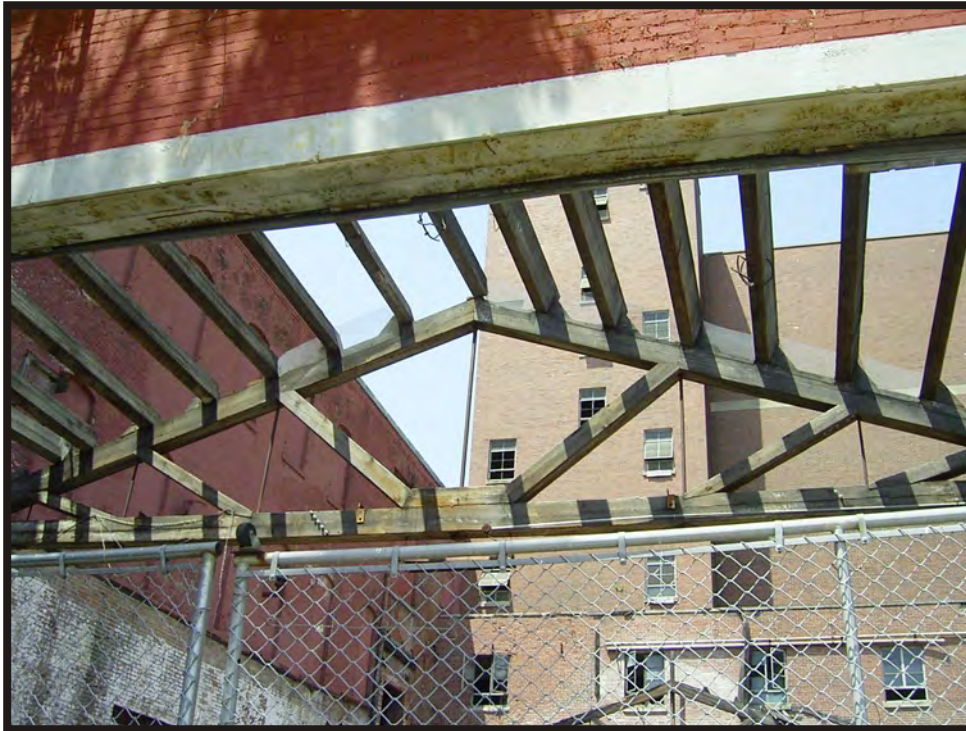
Plate B113. View of Hudepohl Brewery at 801 West 6th Street, facing north.
