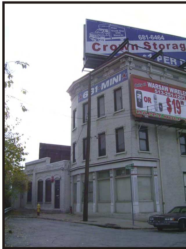
Plate B28. View of building at 1101 Alfred Street, facing south.
