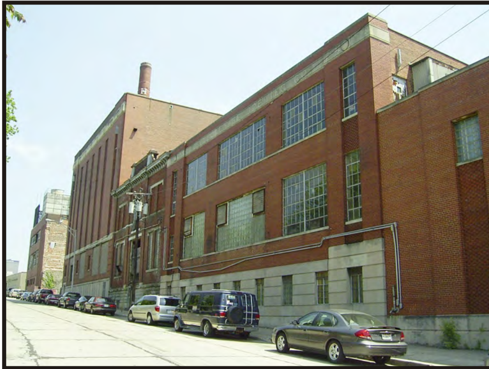
Plate B117. View of Hudepohl Brewery at 801 West 6th Street, facing east.
