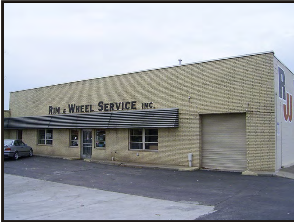
Plate B37. View of building at 1100 Gest Street, facing northwest.
