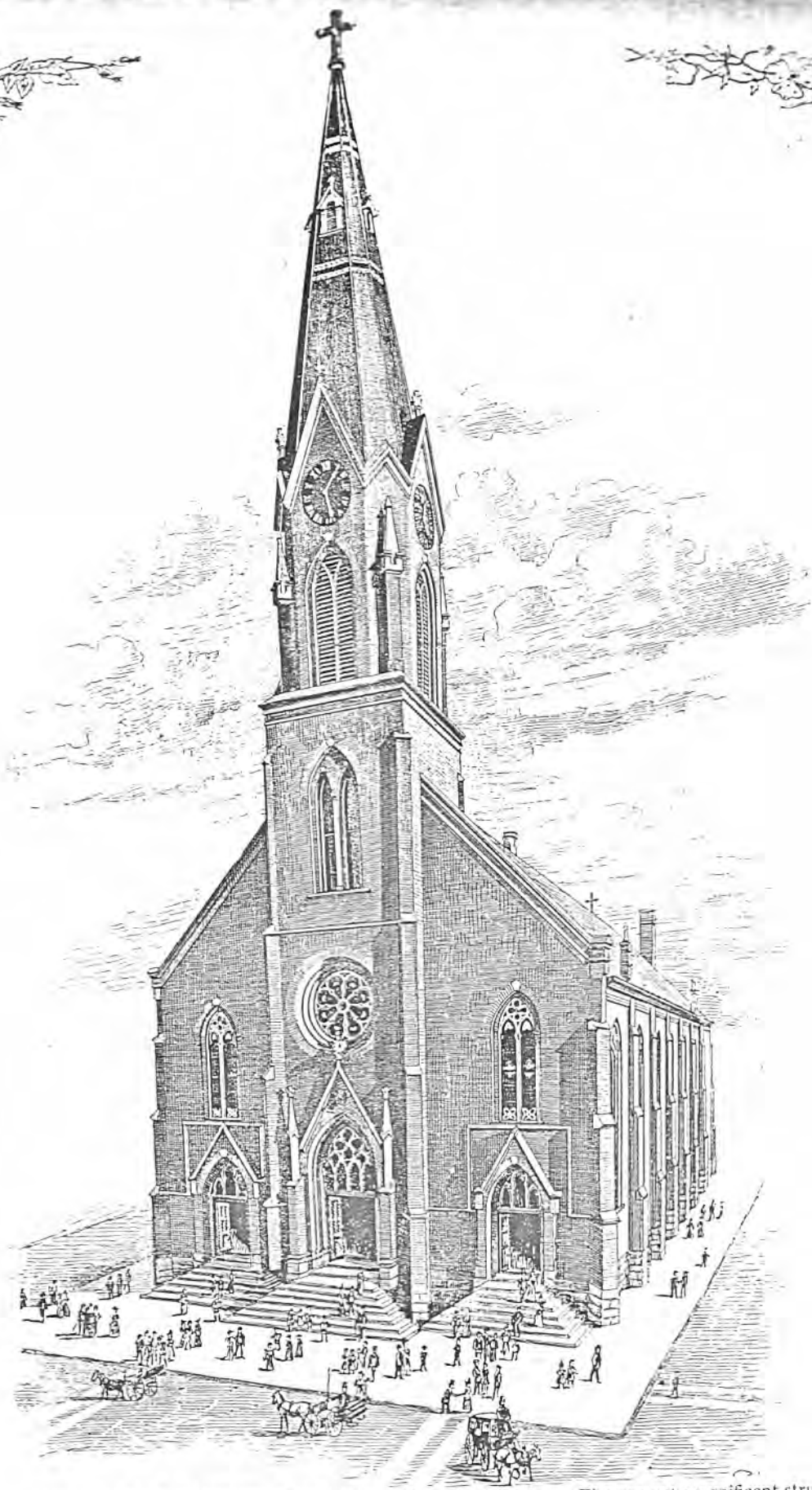
ST. HENRY'S CHURCH, Flint Street. —Organized in 1873. The present magnificent structure was dedicated July 20, 1893, is of the gothic style, 70 x 173 feet, cost $65,000, including ground. The original church was a three-story brick, containing church, school and parsonage, and was dedicated December 14, 1873. The first pastor was Rev. Anthony Ulrich, who died November 22, 1881, and was succeeded by the present incumbent, Rev. John M. Schuchardt. The assistant pastor is Rev. John H. Vogedes. The congregation has a membership of 400 families.
