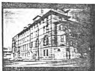
South facade, Looking Northwest
