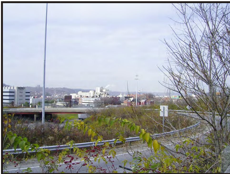
Plate B74. View of I-75 off-ramp to Western Hills Viaduct, facing northwest.
