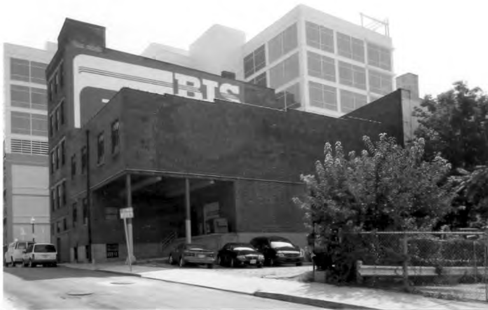
VIEW TO SOUTHEAST, REAR OF BUILDING
