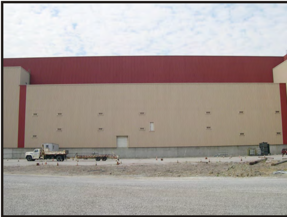
Plate B126. View of West End Electric Generating Station (HAM-5508-43), facing south.
