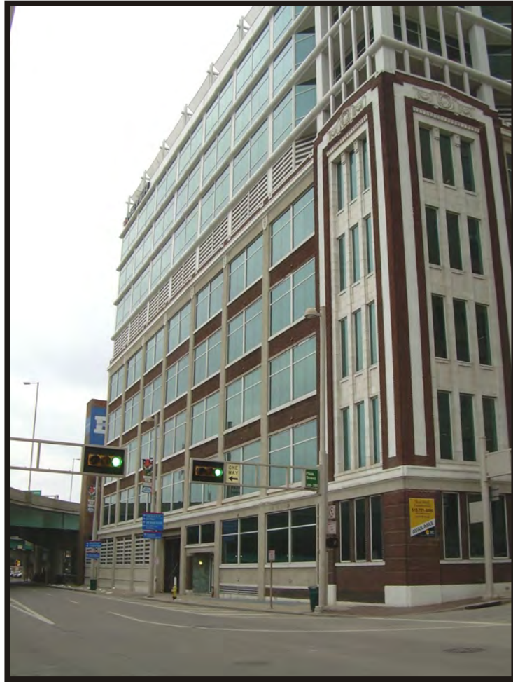
Plate B103. View of 302 West 3 rd Street, facing northwest.
