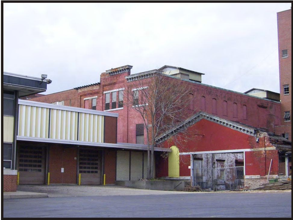
Plate B45. View of building at 801 West 6 th Street, facing northwest.
