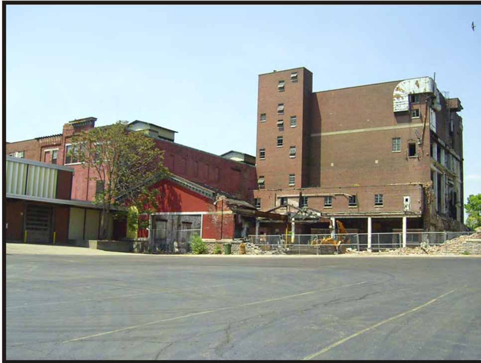
Plate B111. View of Hudepohl Brewery at 801 West 6th Street, facing northwest.
