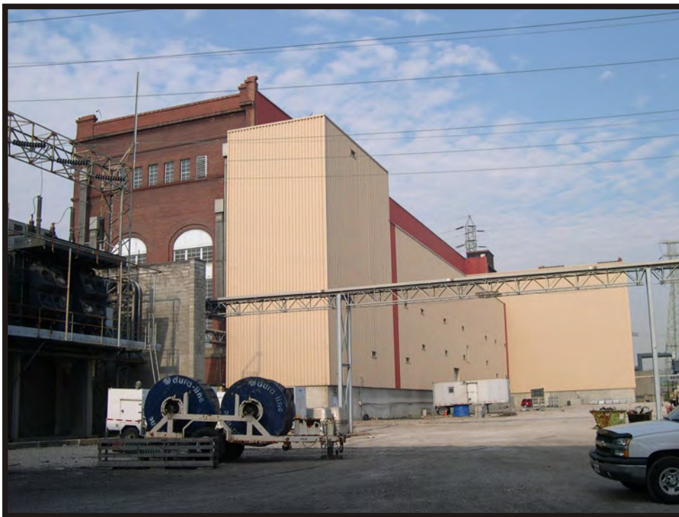
Plate B122. View of West End Electric Generating Station (HAM-5508-43), facing southwest.
