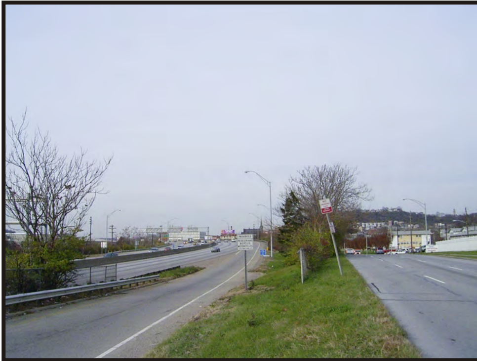
Plate B65. View of I-75 onramp from Winchell Avenue, facing north.
