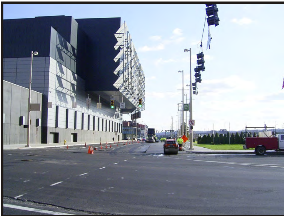
Plate B54. Streetscape of Central Avenue from West 6 th Street, facing south.
