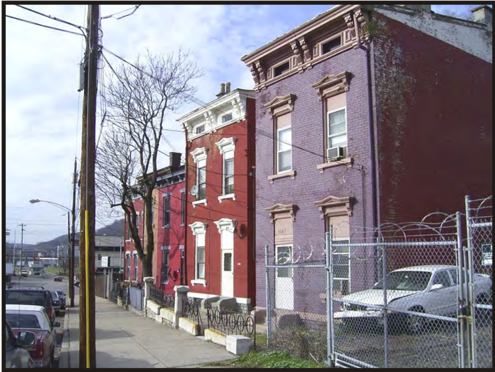
Plate B29. View of buildings at 1130-1132 Draper Street, facing west.
