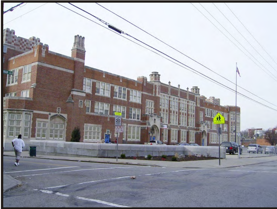
Plate B69. View of Heberle School at Freeman Avenue and Dayton Street, facing northwest.
