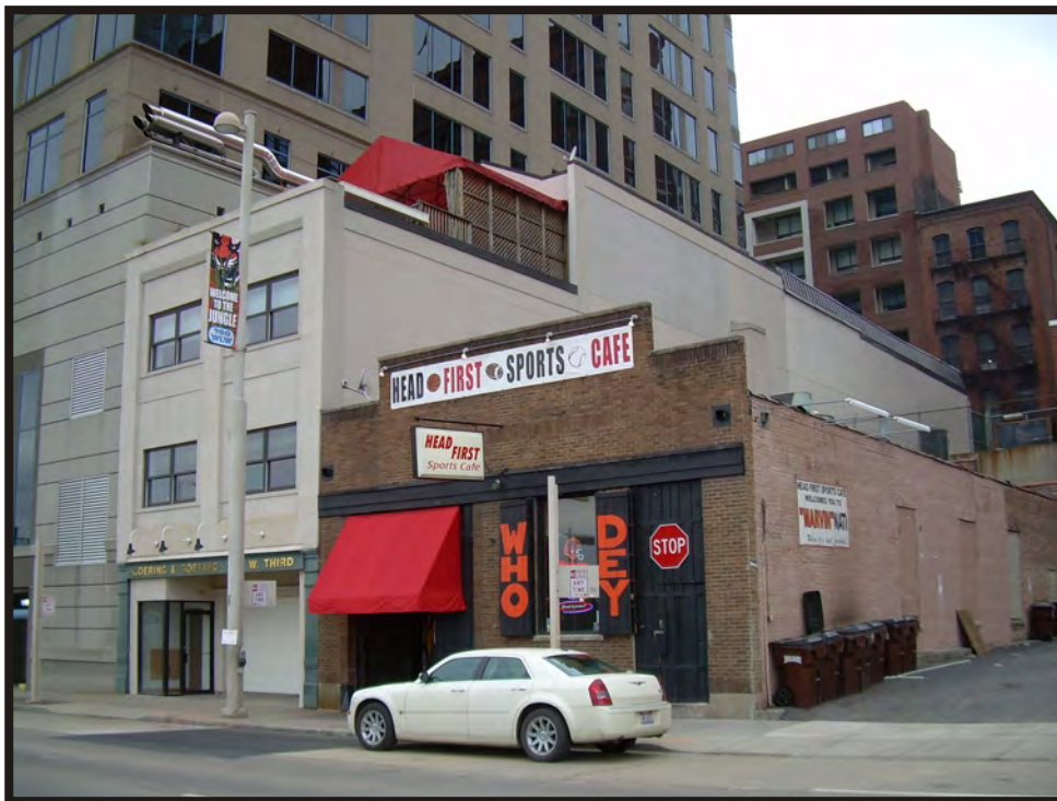
Plate B102. View of Resources HAM-0080-44 and HAM-5540-44 at 220 and 218 West 3 rd Street, facing northwest.
