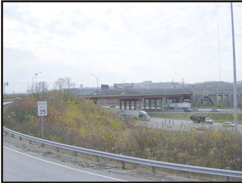
Plate B73. Overview of I-75 and the Western Hills Viaduct from Central Parkway, facing southwest.
