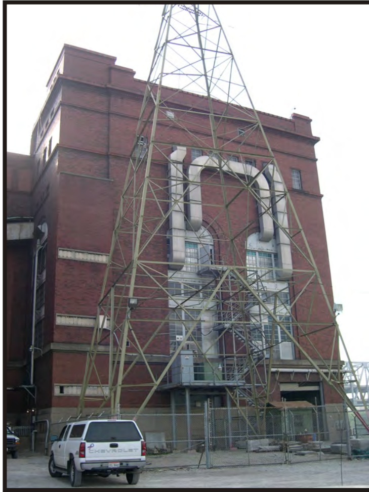
Plate B123. View of West End Electric Generating Station (HAM-5508-43), facing east.
