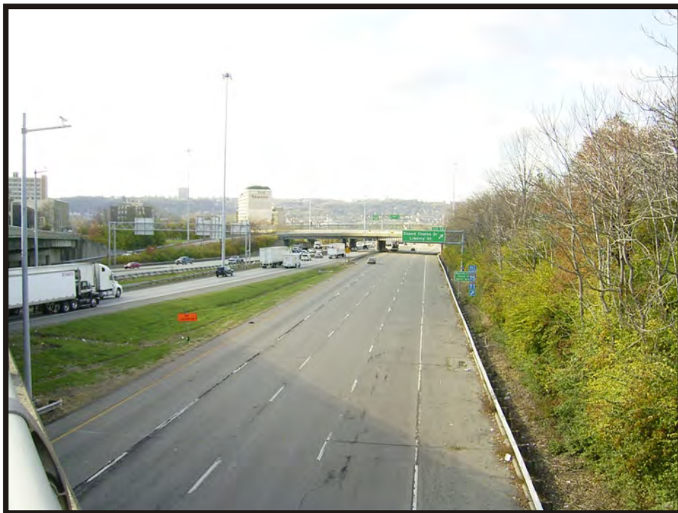
Plate B56. Overview of I-75 from West 7 th Street overpass, facing north.
