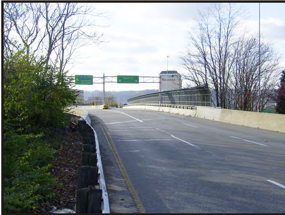
Plate B57. View of West 8 th Street Viaduct, facing west.
