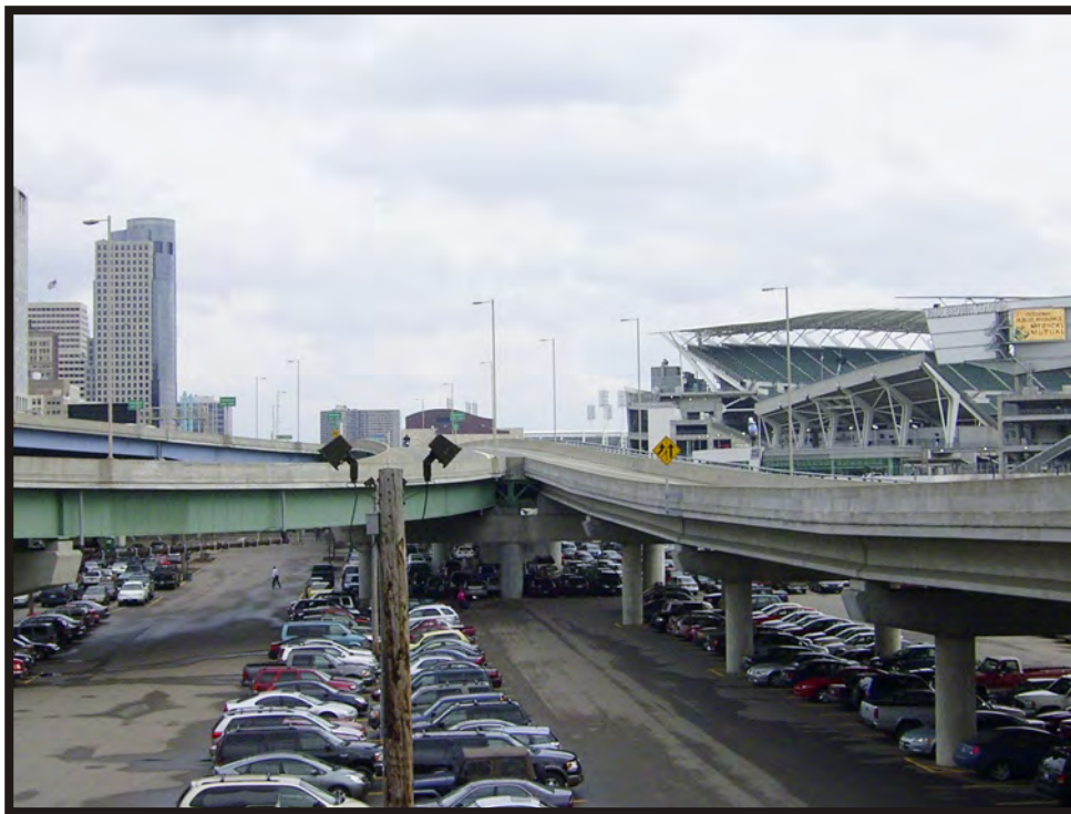
Plate B100. Overview of West 2 nd Street onramps from Clay Wade Bailey Bridge approach, facing east.
