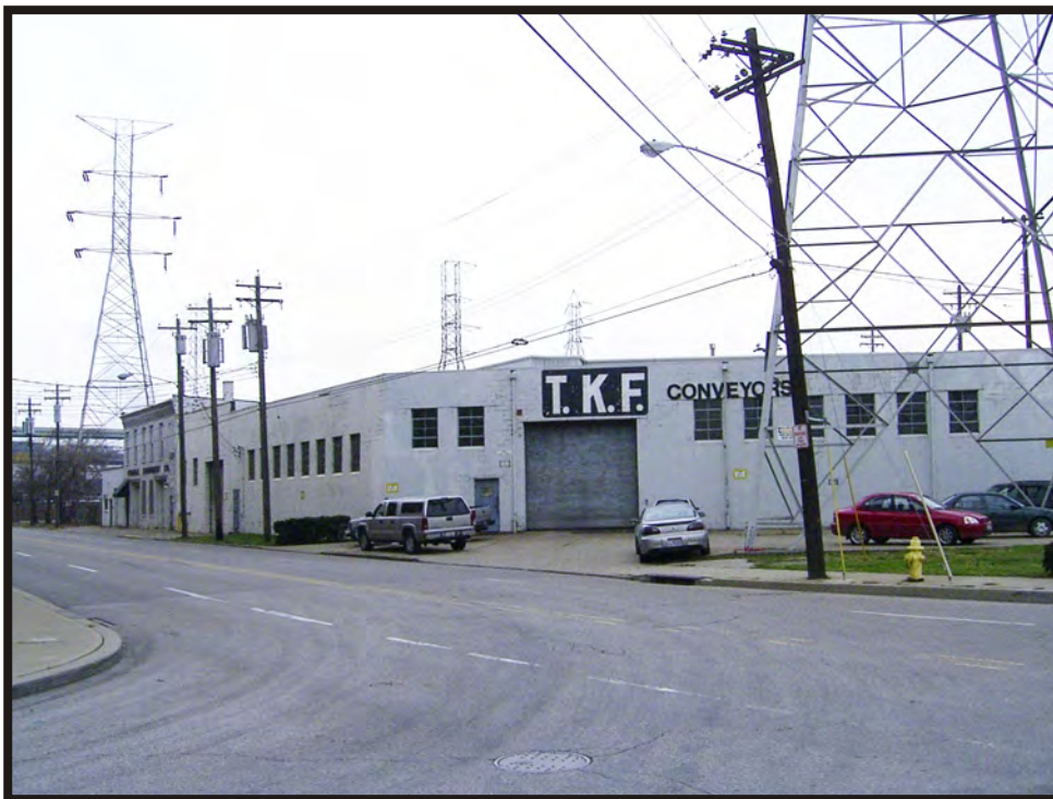
Plate B16. View of building at 726 Mehring Way, facing southeast.
