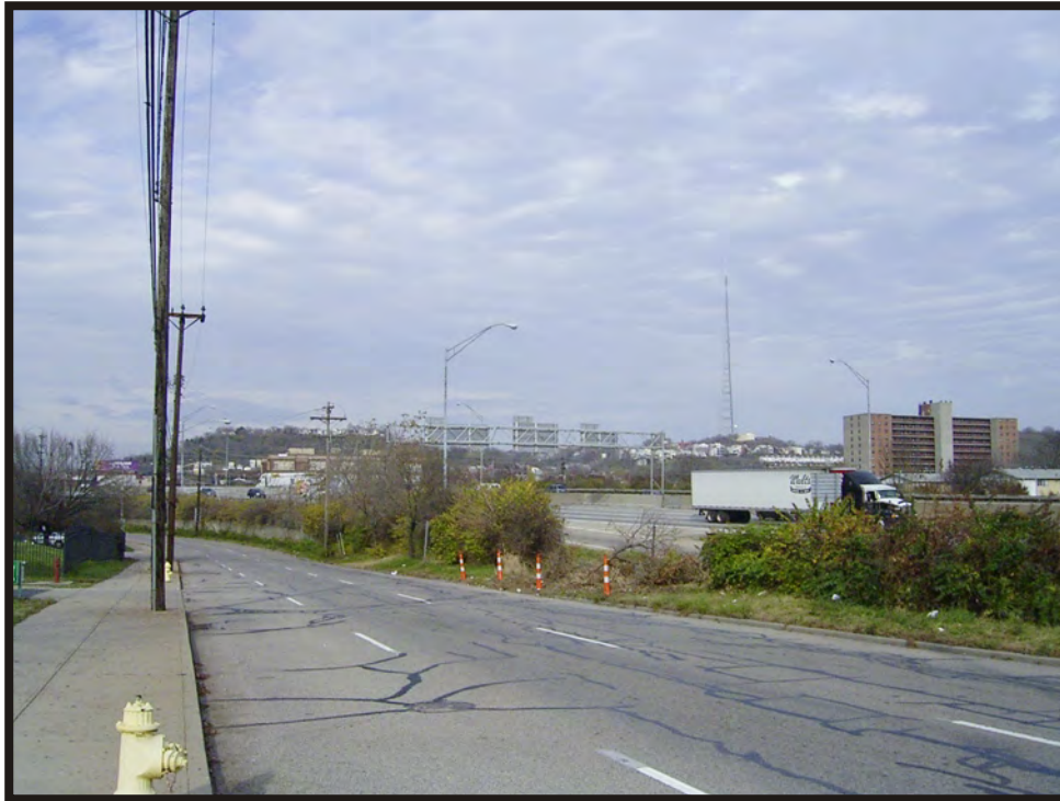
Plate B81. View of Western Avenue and I-75, facing north.
