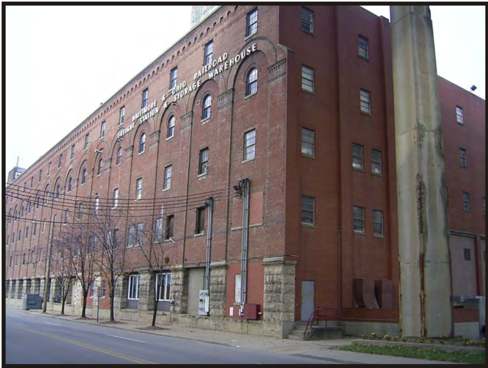
Plate B12. Detail of Longworth Hall (HAM-1656-43), facing northwest.
