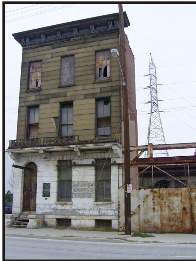
Plate B18. View of building at 724 Mehring Way, facing north.
