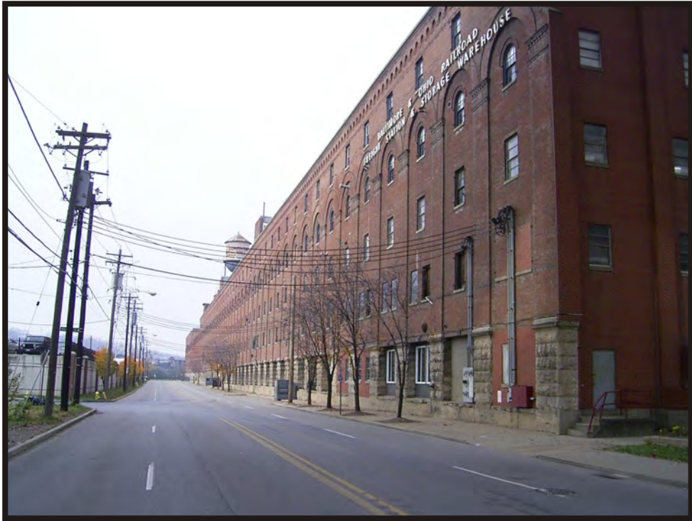
Plate B11. View of Longworth Hall (HAM-1656-43), facing west.
