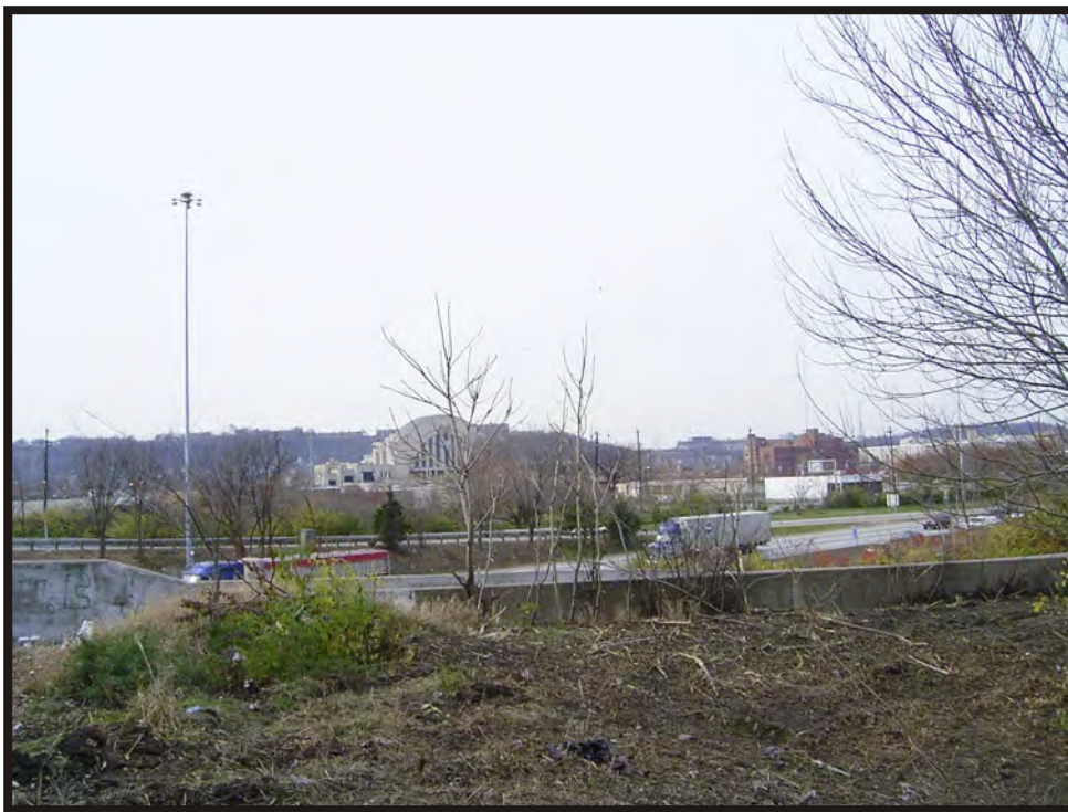
Plate B62. Overview of I-75 and Union Terminal from West Court Street terminus, facing northwest.
