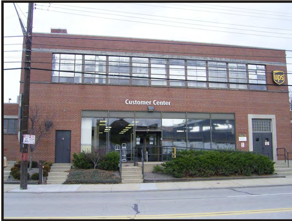
Plate B5. View of building at 690 West 3 rd Street, facing north.
