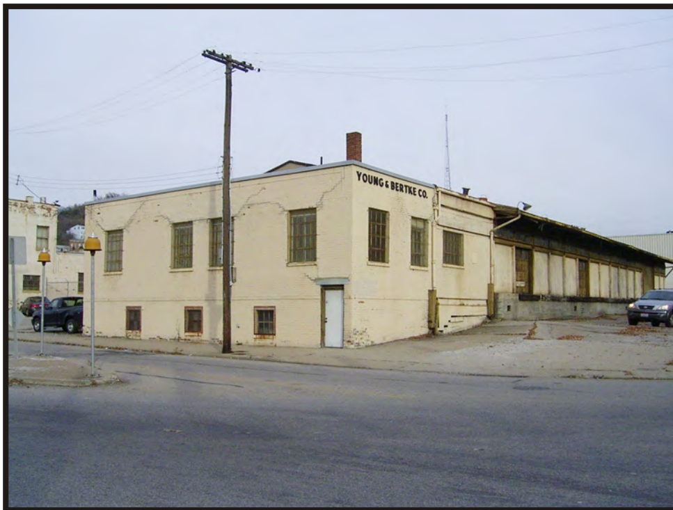
Plate B26. View of secondary building at 2108 Winchell Avenue, facing east.
