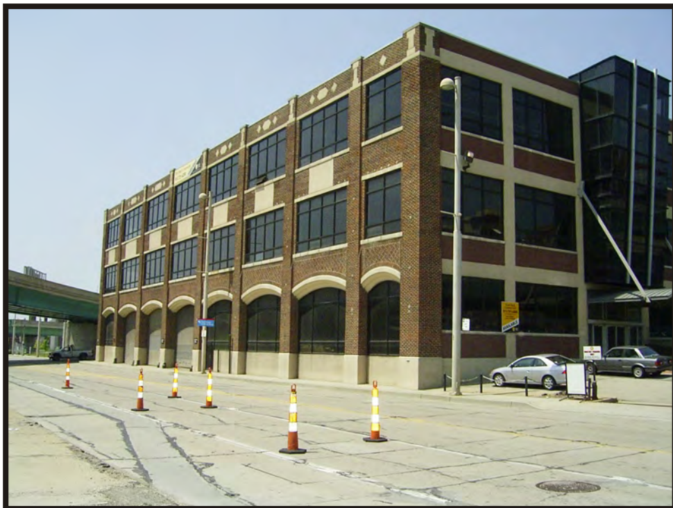
Plate B104. View of Hennegan Warehouse (HAM-5571-44), facing northwest.
