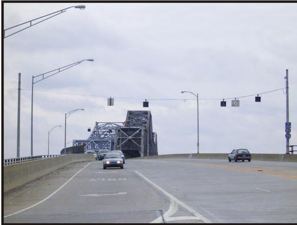
Plate B101. View of Clay Wade Bailey Bridge and CSX Rail Bridge from West 2 nd Street, facing south.
