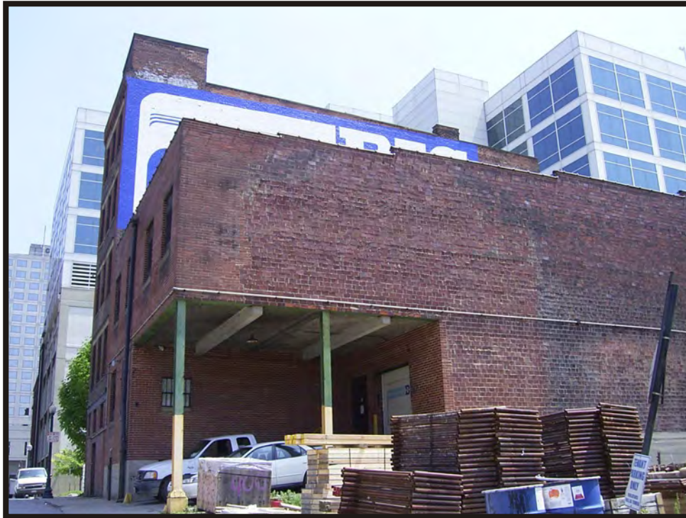
Plate B107. View of Business Information Storage Building (HAM-5572-44) at 318 West 3rd Street, facing east.
