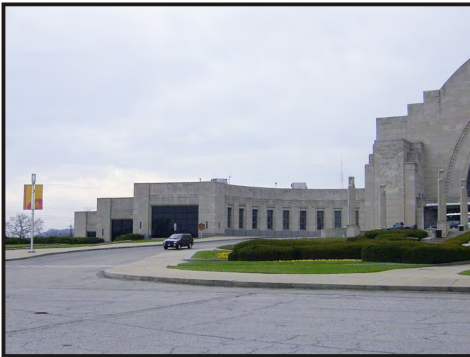
Plate B36. Detail of Cincinnati Union Terminal (HAM-1295-43), facing southwest.
