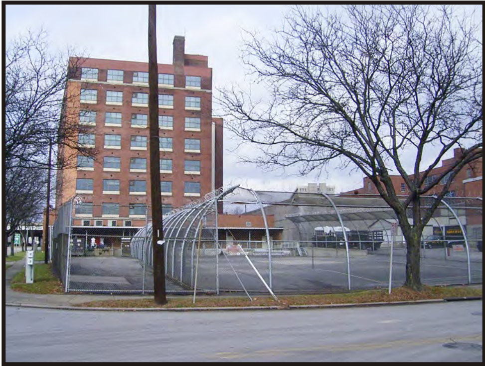
Plate B41. View of building at 516-528 Linn Street, facing north.
