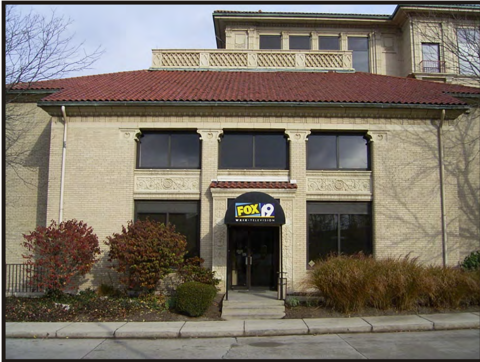
Plate B39. Detail of Harriet Beecher Stowe Elementary School (HAM-1342-43), facing north.
