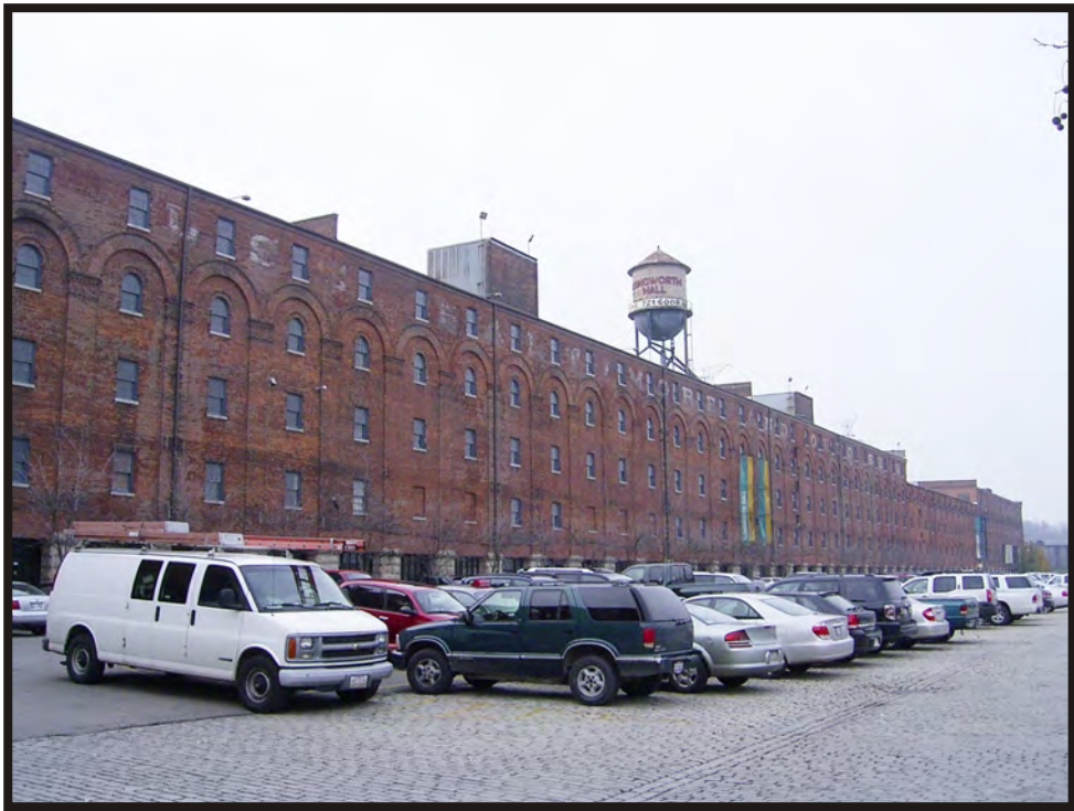
Plate B10. View of Longworth Hall (HAM-1656-43), facing southwest.
