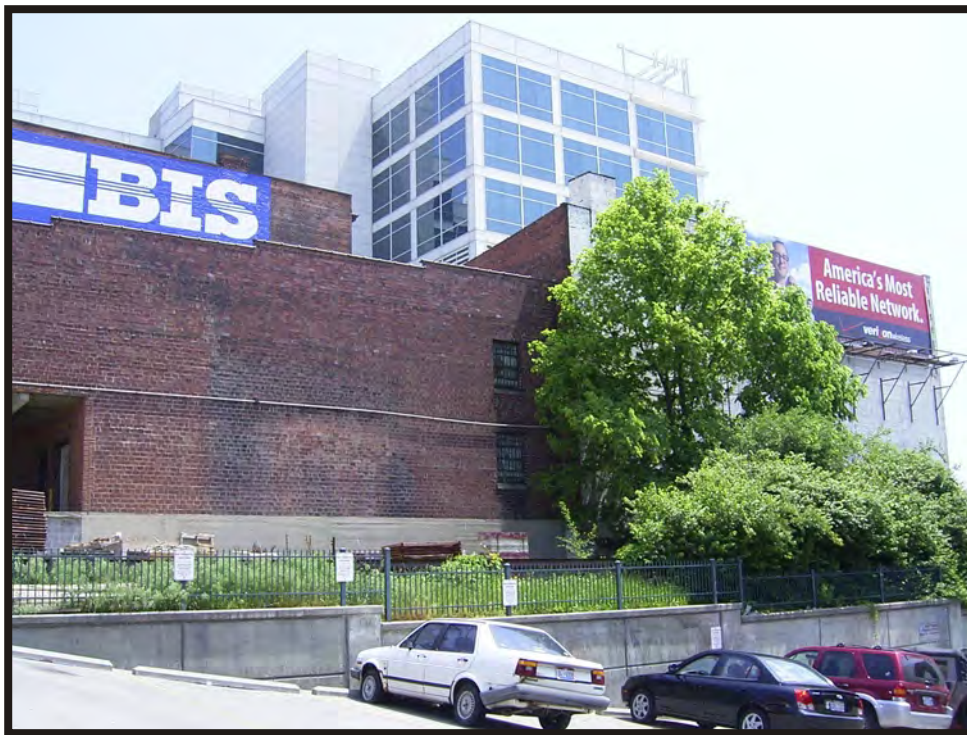
Plate B108. View of Business Information Storage Building (HAM-5572-44) at 318 West 3rd Street, facing southeast.
