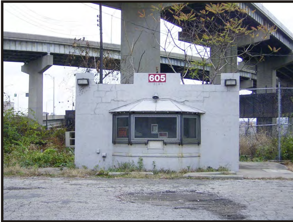
Plate B7. View of building at 605 West 3 rd Street, facing south.
