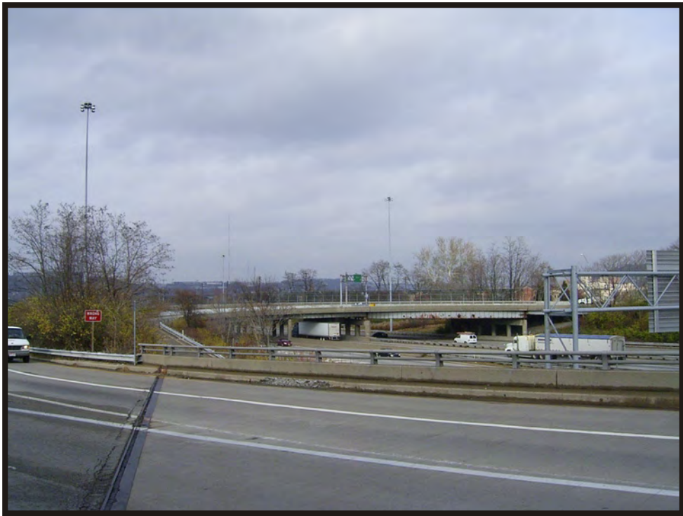
Plate B90. Overview of I-75 from W. 7 th Street, facing northwest.
