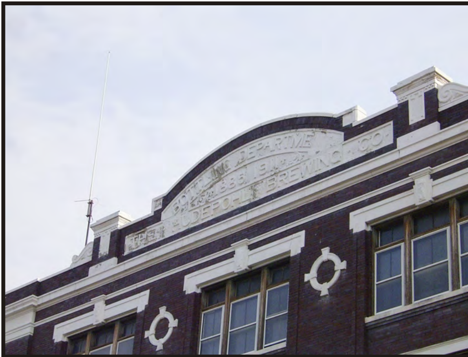
Plate B15. Detail of the former Hudepohl Brewing Company Bottling Plant at 40 East McMicken Avenue, facing north.
