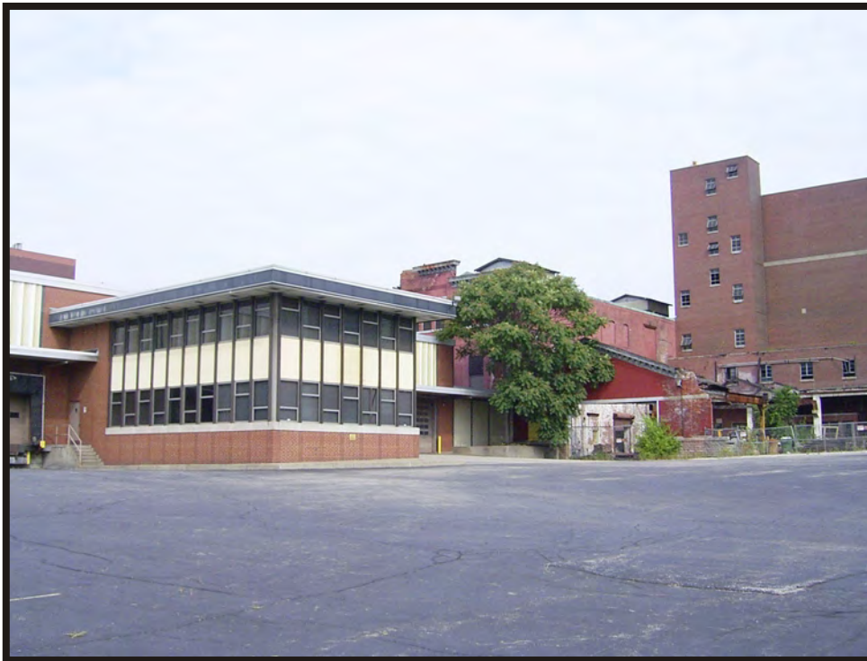
Plate B39. Rear of Hudepohl Brewing Company complex, facing northwest.
