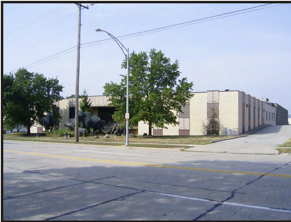
Plate B17. The 1966 Hudepohl office building at 505 Gest Street, facing southwest.
