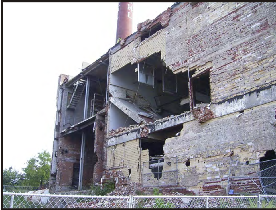
Plate B44. Detail of Hudepohl Brewing Company demolition site, facing northeast.
