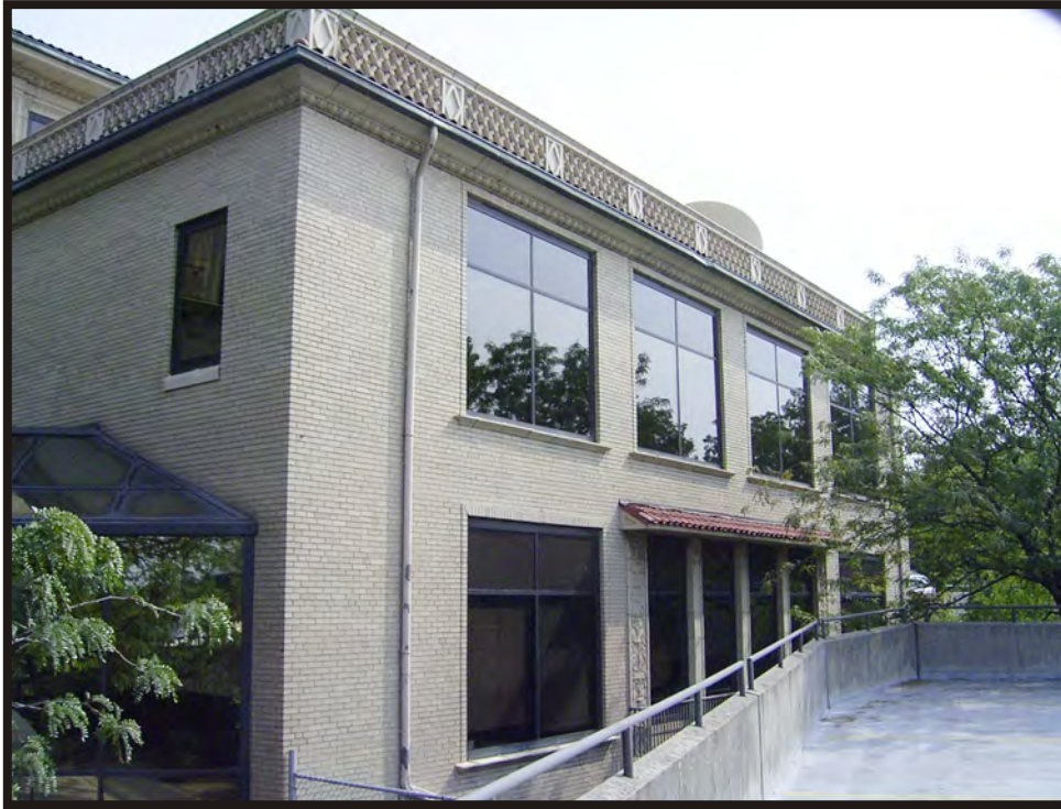
Plate B3. Southeast wing of Harriet Beecher Stowe School (HAM-1342-43) from parking garage, facing northeast.
