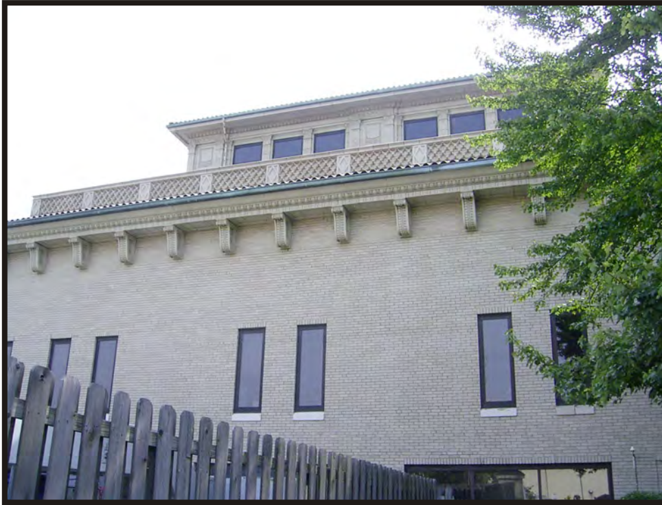
Plate B5. Harriet Beecher Stowe School (HAM-1342-43), west façade, facing east.
