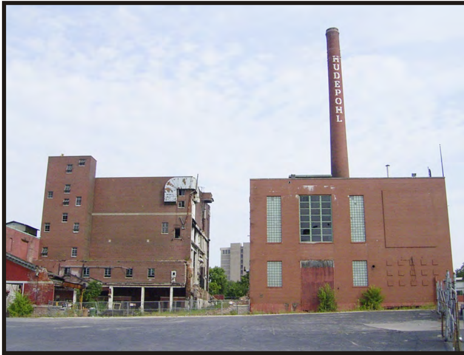
Plate B42. Rear of Hudepohl Brewing Company complex, showing 1960 addition on right, 1947 addition on left, and demolition site, facing north.
