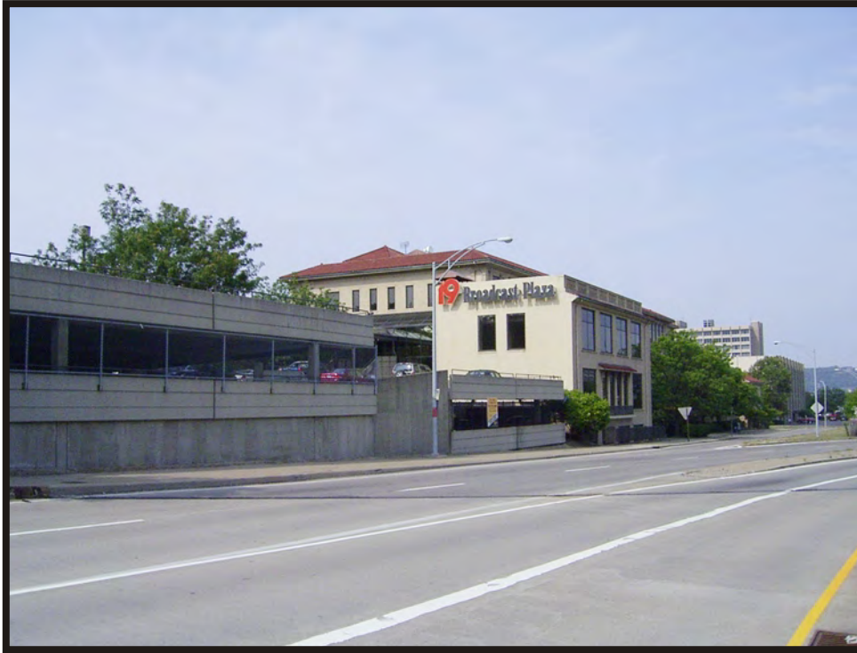
Plate B13. Harriet Beecher Stowe School (HAM-1342-43) and parking garage addition, facing southwest.
