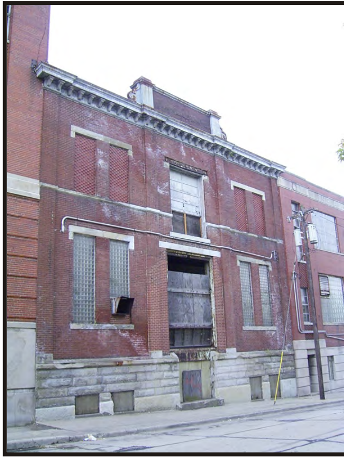
Plate B30. Hudepohl Brewing Company complex, original Lackman Brewery building, facing south.
