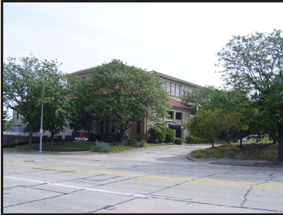
Plate B1. Harriet Beecher Stowe School (HAM-1342-43), facing northeast.
