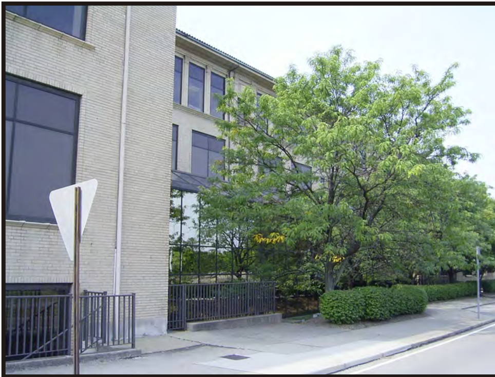
Plate B10. North façade of Harriet Beecher Stowe School (HAM-1342-43), facing southwest.
