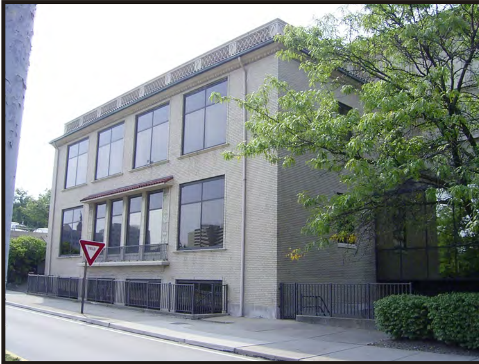
Plate B9. Northeast wing of Harriet Beecher Stowe School (HAM-1342-43), facing southeast.
