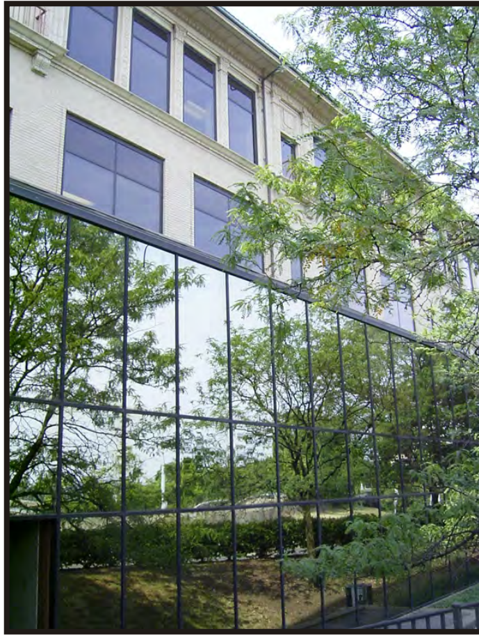
Plate B11. Detail of solarium addition on north façade of Harriet Beecher Stowe School (HAM-1342-43), facing southwest.
