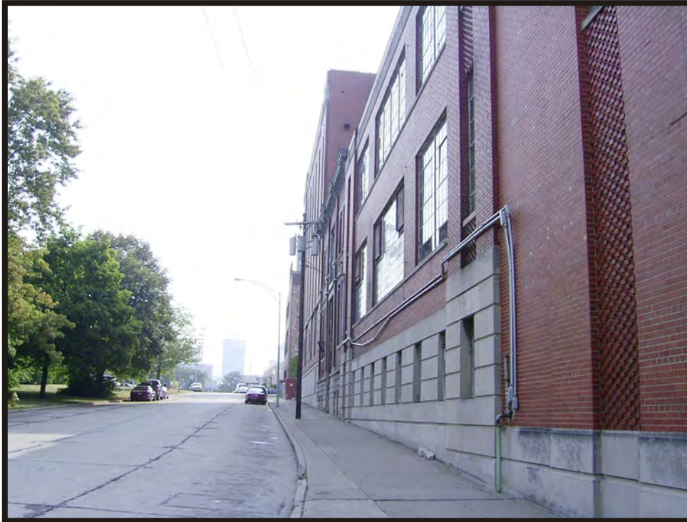
Plate B34. Hudepohl Brewing Company complex and West Sixth Street, facing east.
