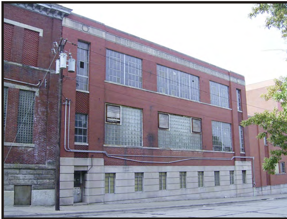
Plate B31. The Hudepohl Brewing Company 1940 addition, facing south.
