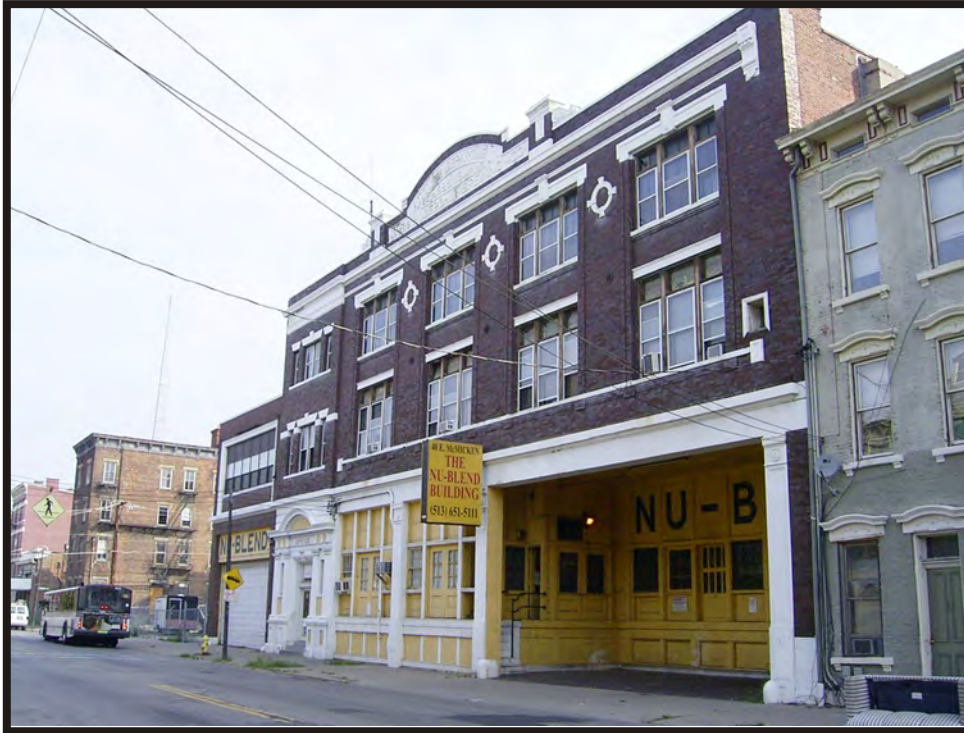
Plate B14. The former Hudepohl Brewing Company Bottling Plant at 40 East McMicken Avenue, facing north.
