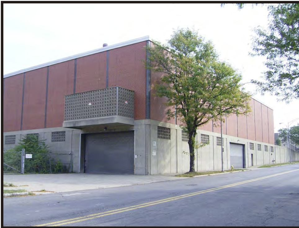
Plate B45. Hudepohl Brewing Company 1980s addition from West Fifth Street, facing northeast.
