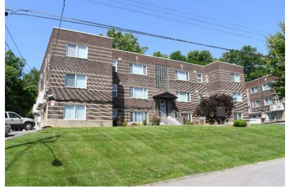
H-shaped, three story, brick veneer apartment building with Art Deco features in the proposed Elberta Apartments Historic District.
