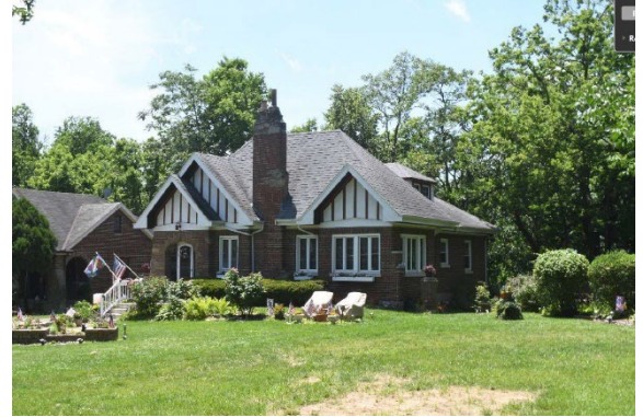
Tudor Revival House at 51 Rivard Drive in Covington (Kentucky): a contributing element to the Hillsdale Subdivision Historic District to have 0.06 acre of strip right-of-way acquired from the rear of the property.
