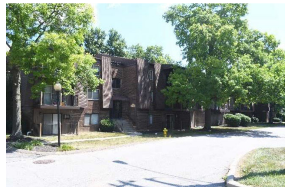
More contemporary brick veneer apartment building in the proposed Elberta Apartments Historic District.
