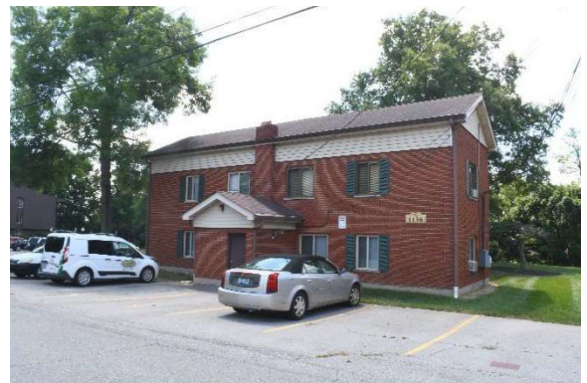
Colonial Revival-inspired four-plex apartment building in the proposed Elberta Apartments Historic District.
