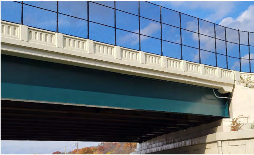
Steel girder example
