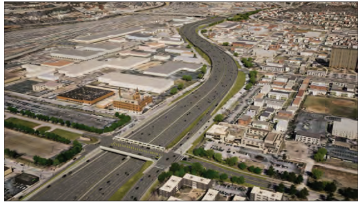
This view shows what the finished project will look like from Ezzard Charles Drive looking north. Notice the 8-foot-tall extended traffic safety barriers for noise reduction. Also notice the ashlar stone treatments on the retaining walls.
