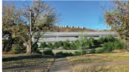
Goebel Park Clock Tower with Noise Wall (looking west)
