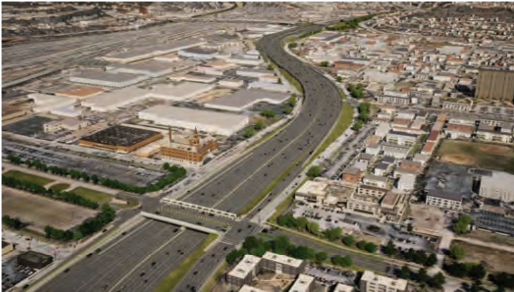
Brent Spence Bridge Corridor - Ohio (Looking North Near Ezzard Charles Drive)
