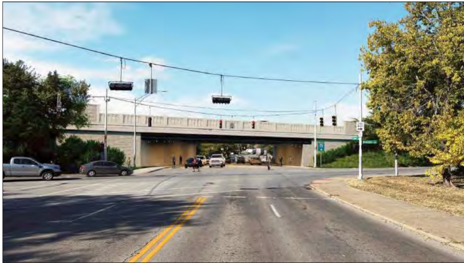
This is a view of what Findlay Street will look like when the project is built. Notice the 57-inch barrier on the I-75 bridge and the 8-foot extended traffic safety barriers on both sides of the bridge to reduce traffic noise. This also shows what the barriers and bridge walls will look like with the ashlar stone treatment. Also notice the rebuilt sidewalks, added bike lanes, and underpass lighting.
