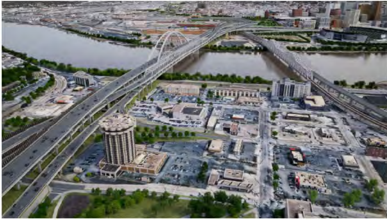
Brent Spence Bridge Corridor (Looking Northwest from Kentucky)
