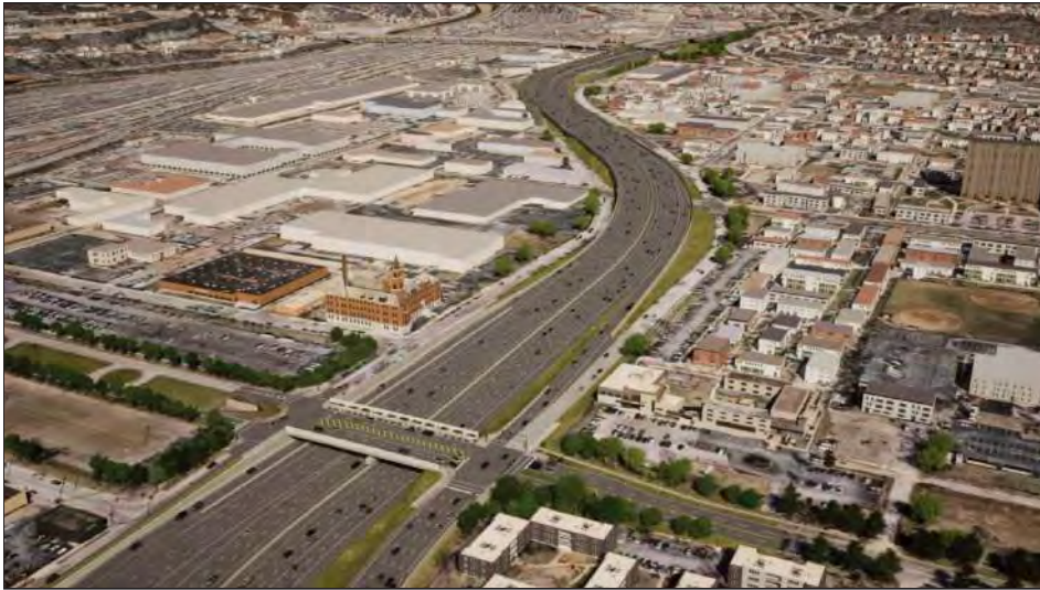
This view shows what the finished project will look like from Ezzard Charles Drive looking north. Notice the 8-foot-tall extended traffic safety barriers for noise reduction. Also notice the ashlar stone treatments on the retaining walls.
