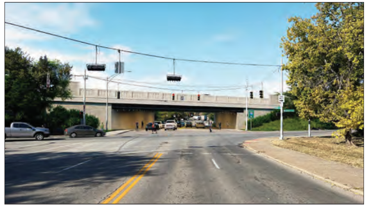
This is a view of what Findlay Street will look like when the project is built. Notice the 57-inch barrier on the I-75 bridge and the 8-foot extended traffic safety barriers on both sides of the bridge to reduce traffic noise. This also shows what the barriers and bridge walls will look like with the ashlar stone treatment. Also notice the rebuilt sidewalks, added bike lanes, and underpass lighting.
