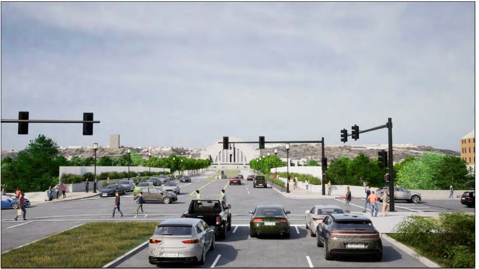
This view shows what the new, two-way bridge on Ezzard Charles Drive will look like. Notice the wide shared use path on the right and the sidewalk on the left. Also notice the planters, screenwall, and decorative lighting on the bridge. The bridge lights and traffic signal supports will be black and meet City aesthetic standards.
