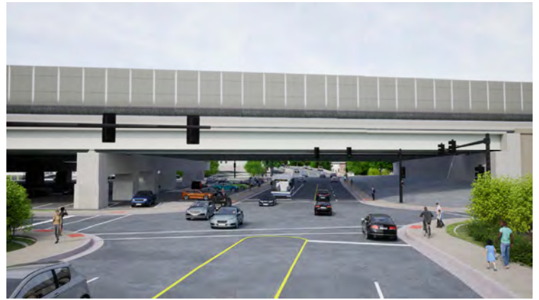
Pike Street With Noise Wall (looking east) 64 dBA (average)
