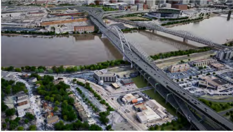
Brent Spence Bridge Corridor (Looking Northeast from Kentucky)
