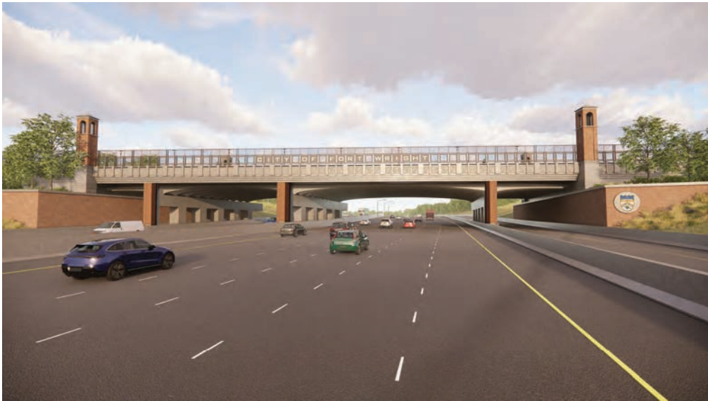
Kyles Lane Overpass (Looking South)
